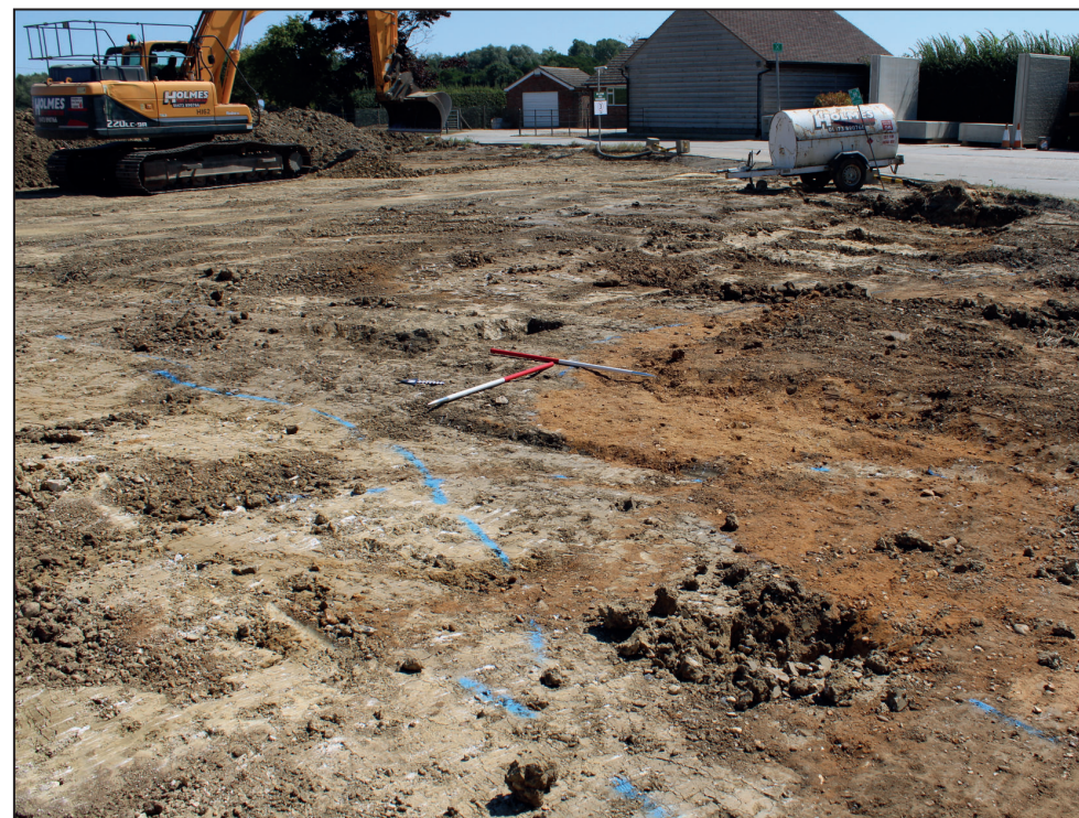
Site, modern disturbance, looking east (scales 1m)
