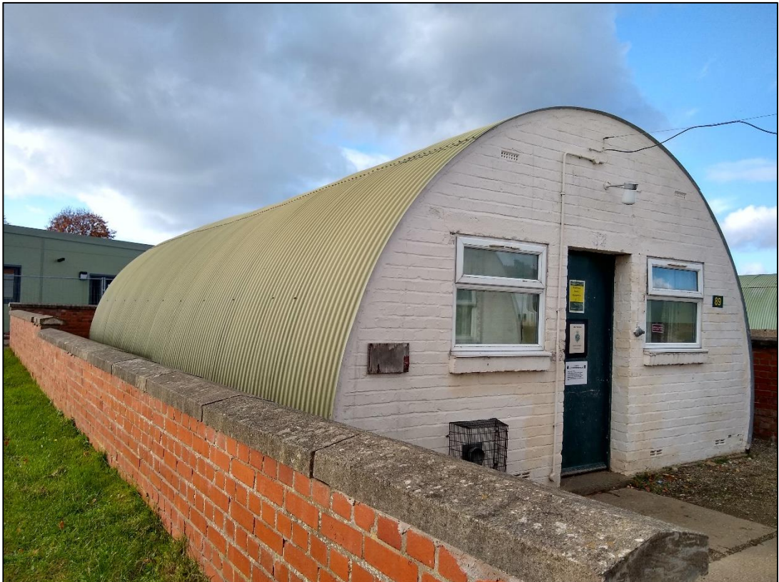
Photo 3: Close up image of a Nissen Hut within the Site
