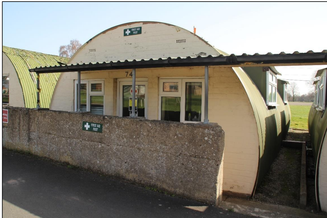
Photo 38: View of the front (west) elevation of the Medical hut
