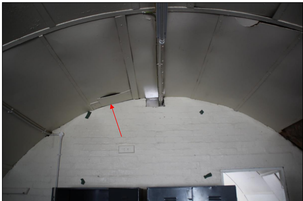
Photo 13: View of the roof apex with flue hole cover arrowed
