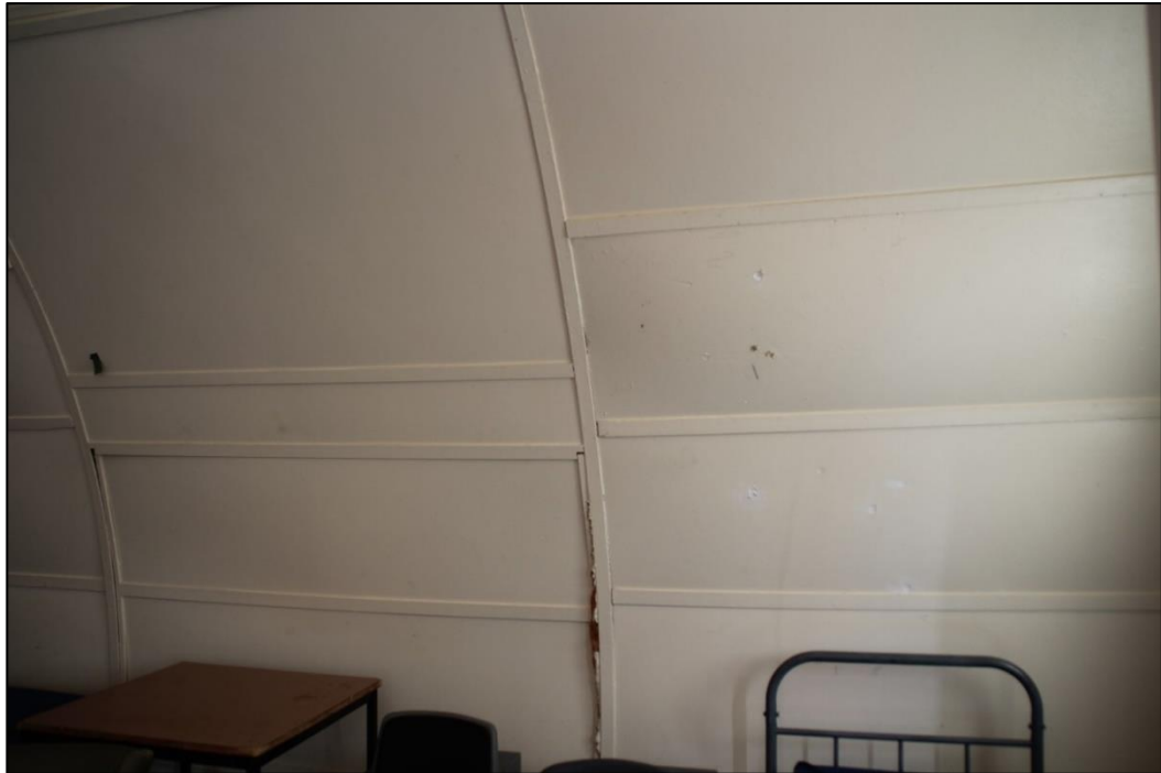
Photo 12: View of cladding to wall in Hut 105
