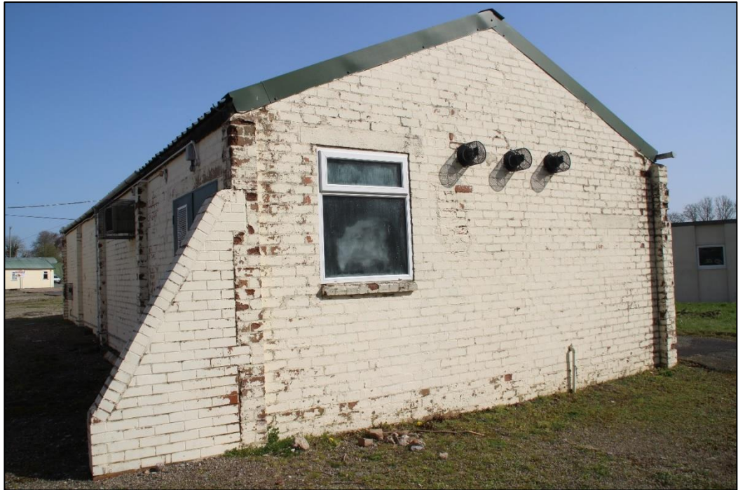
Photo 19: View of southern elevation of Block 106
