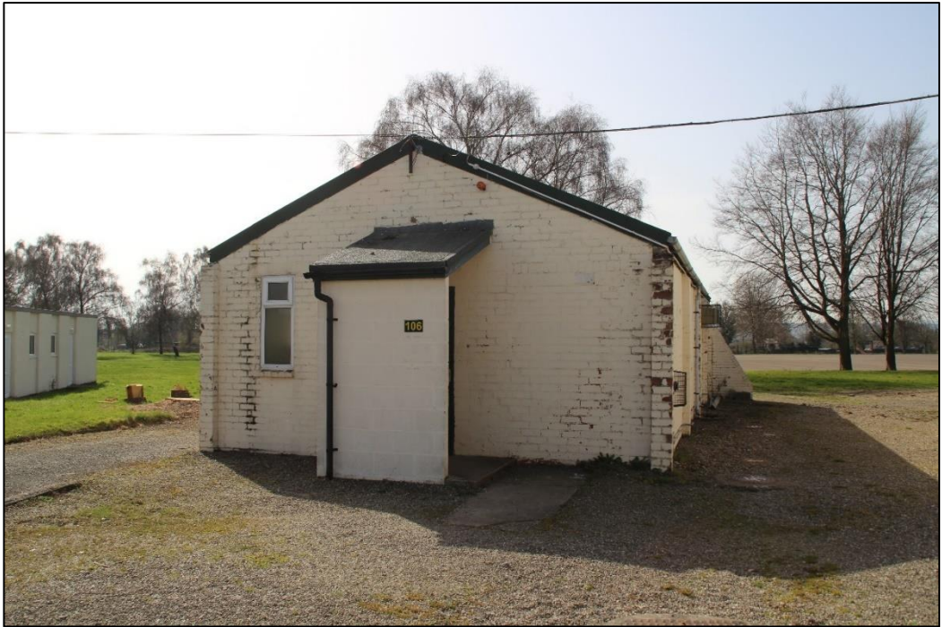
Photo 17: View of toilet and wash block 106, image taken looking south
