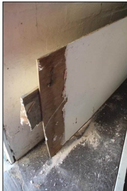
Photo 15: Detail of match boarding used as internal cladding
