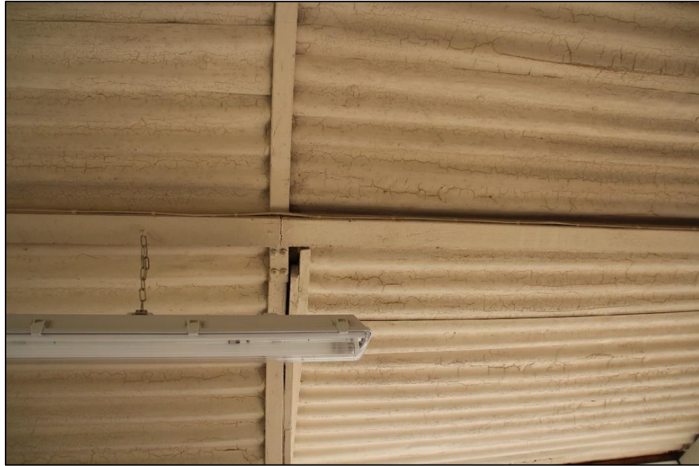
Photo 29: View of the roof apex with longitudinal rib
