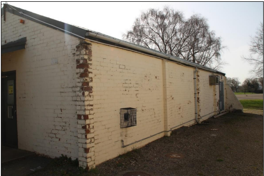
Photo 18: View of western elevation of Block 106
