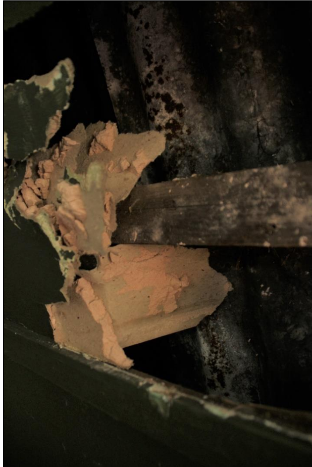
Photo 36: Internal detail view in office hut 77
