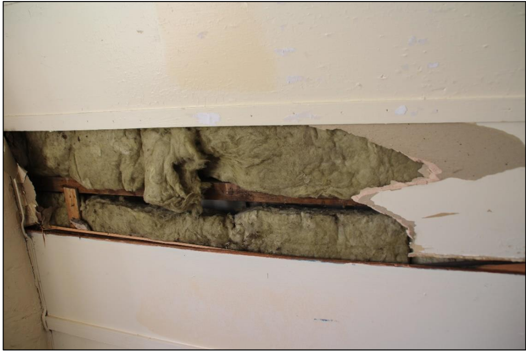
Photo 42: Detail of rock wool insulation and plasterboard cladding – Medical hut
