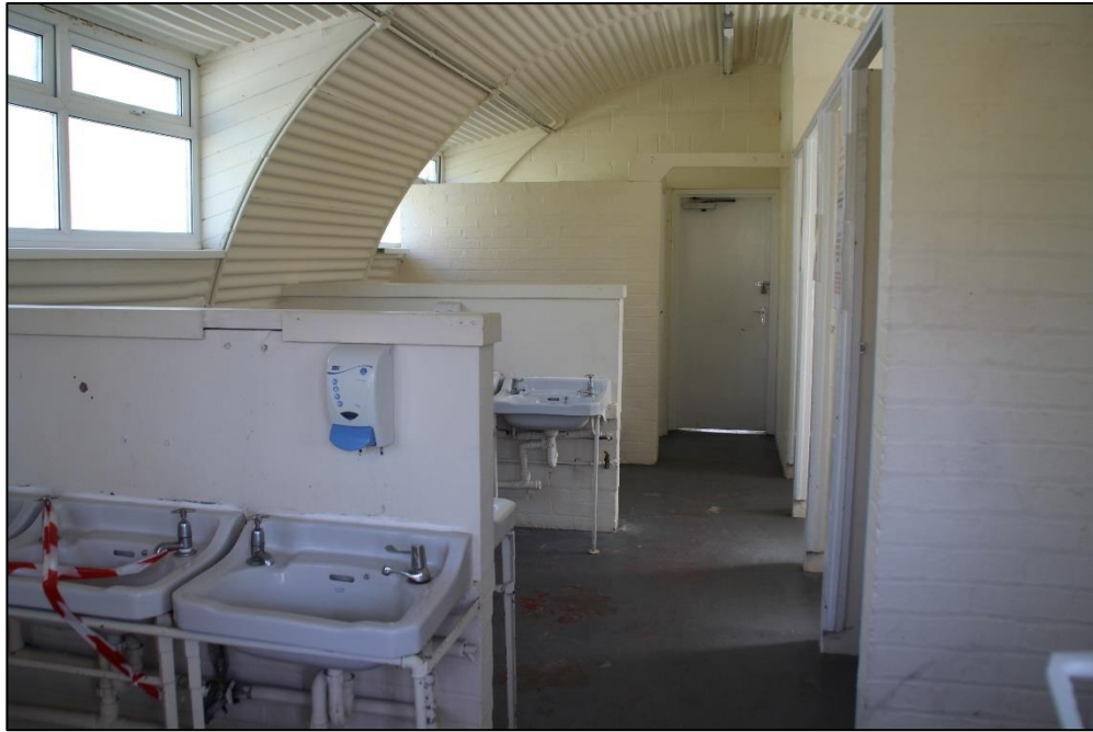
Photo 43: Internal view of the Toilet hut looking east
