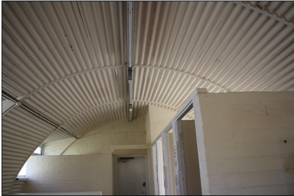
Photo 45: Internal view of the upper areas of the Toilet hut
