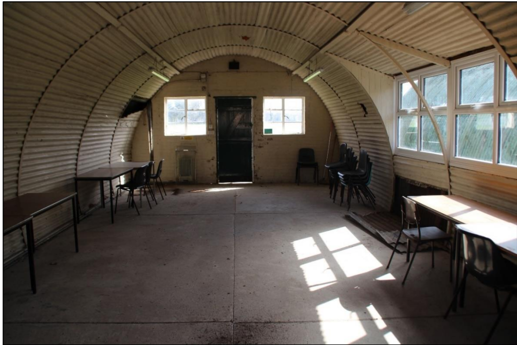
Photo 27: View of the interior of Hut 79 – classroom hut – looking east
