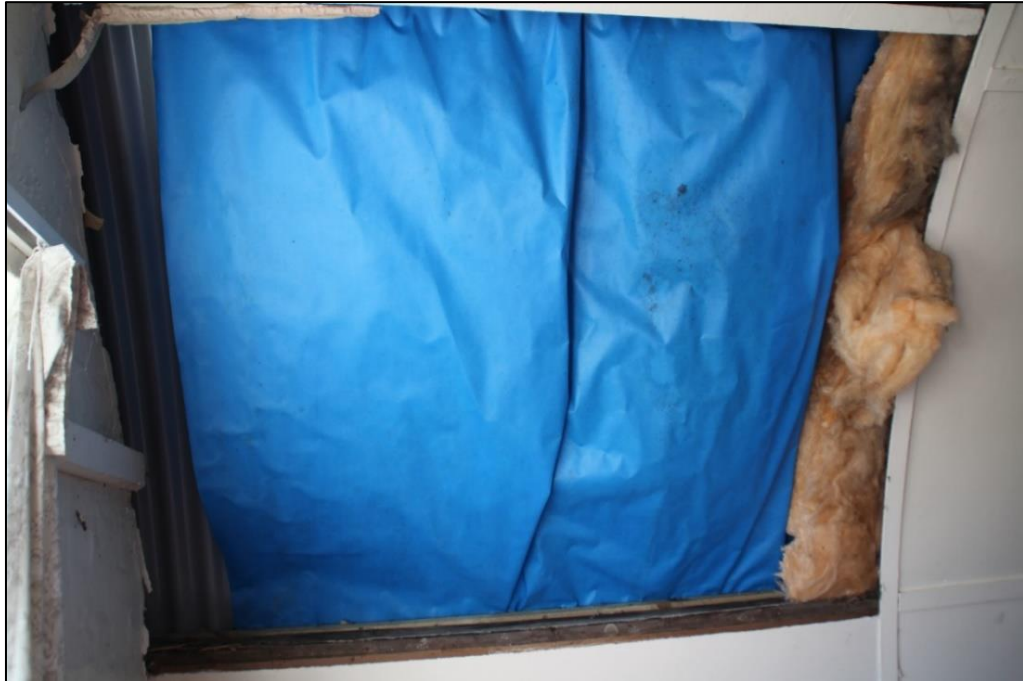
Photo 14: View of the plastic lining and rock wool in Hut 103
