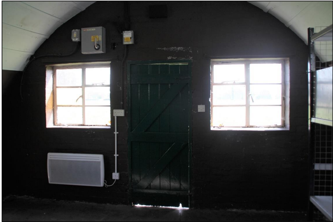
Photo 37: Eastern room of office hut (77)
