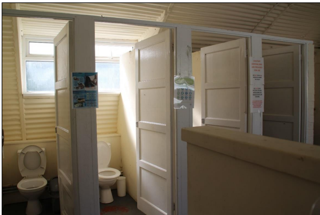
Photo 46: View of toilet cubicles with panelled doors
