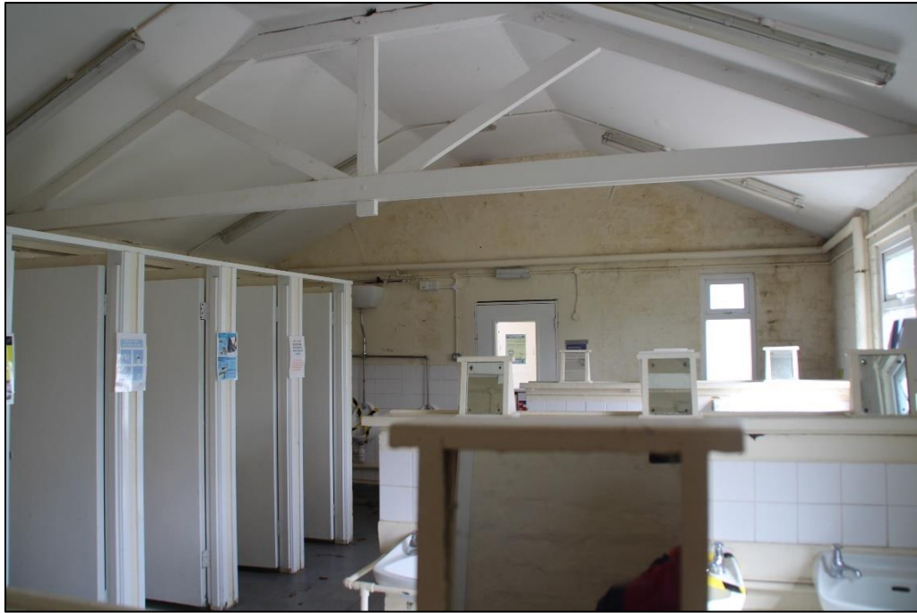
Photo 22: View of the interior of Block 106 looking north
