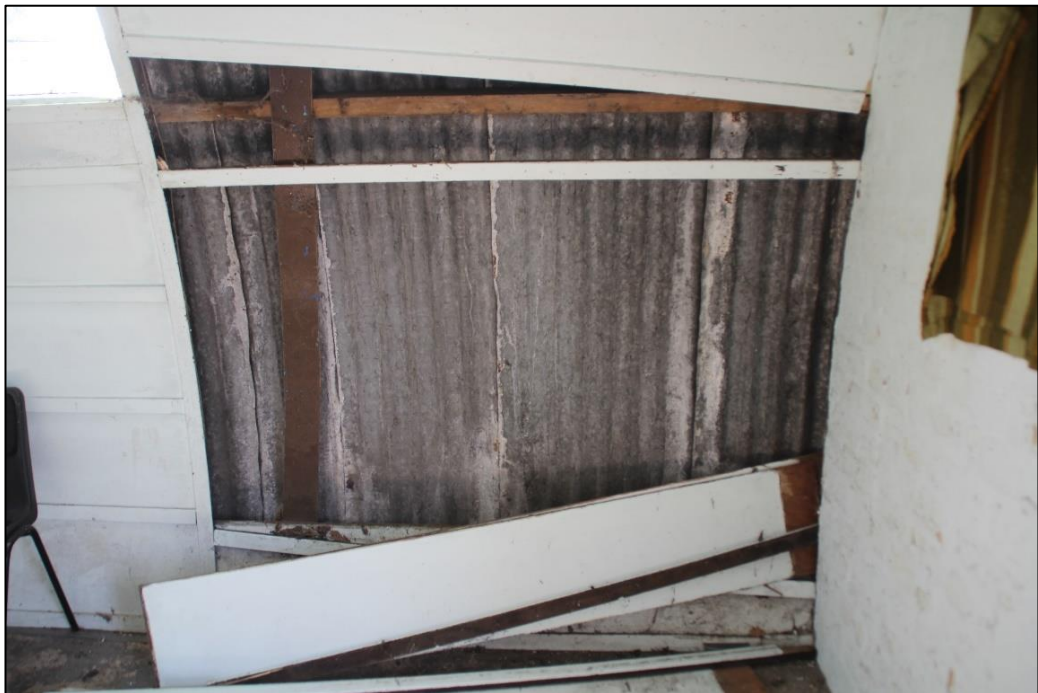
Photo 51: Detail of internal and external cladding in hut 71
