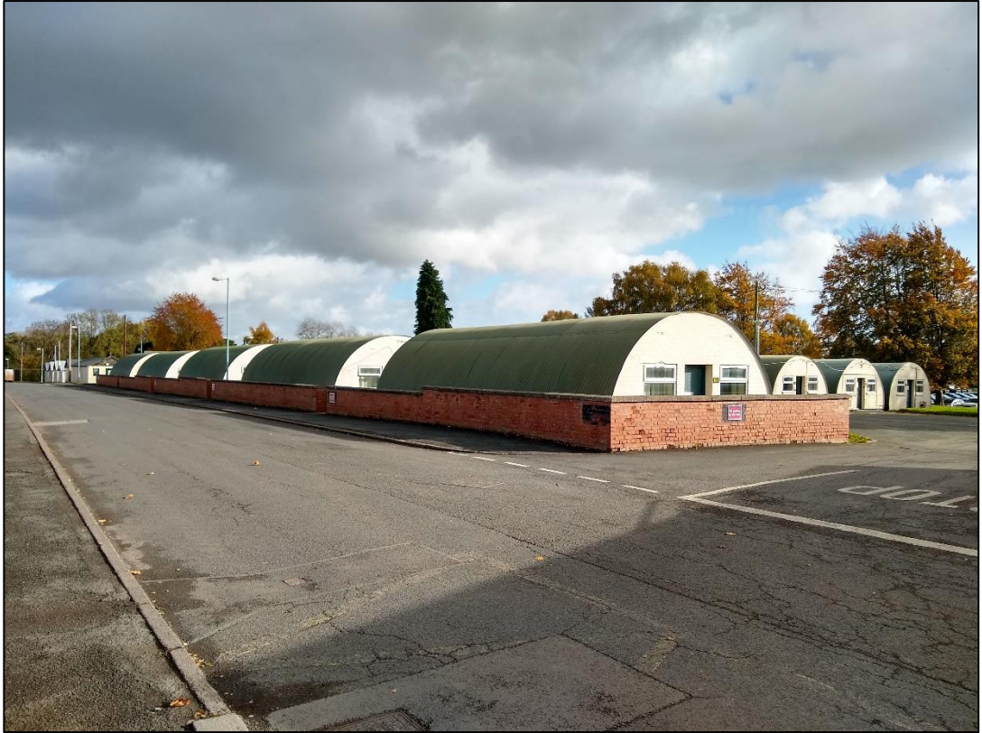
Photo 2: Image taken from the centre of the Site looking south-west at the Nissen Huts in the south of the Site
