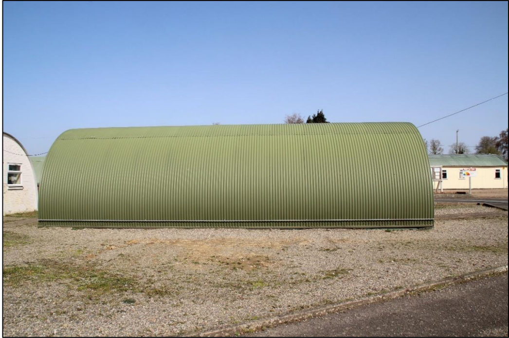
Photo 9: View of Hut 105 from the side angle
