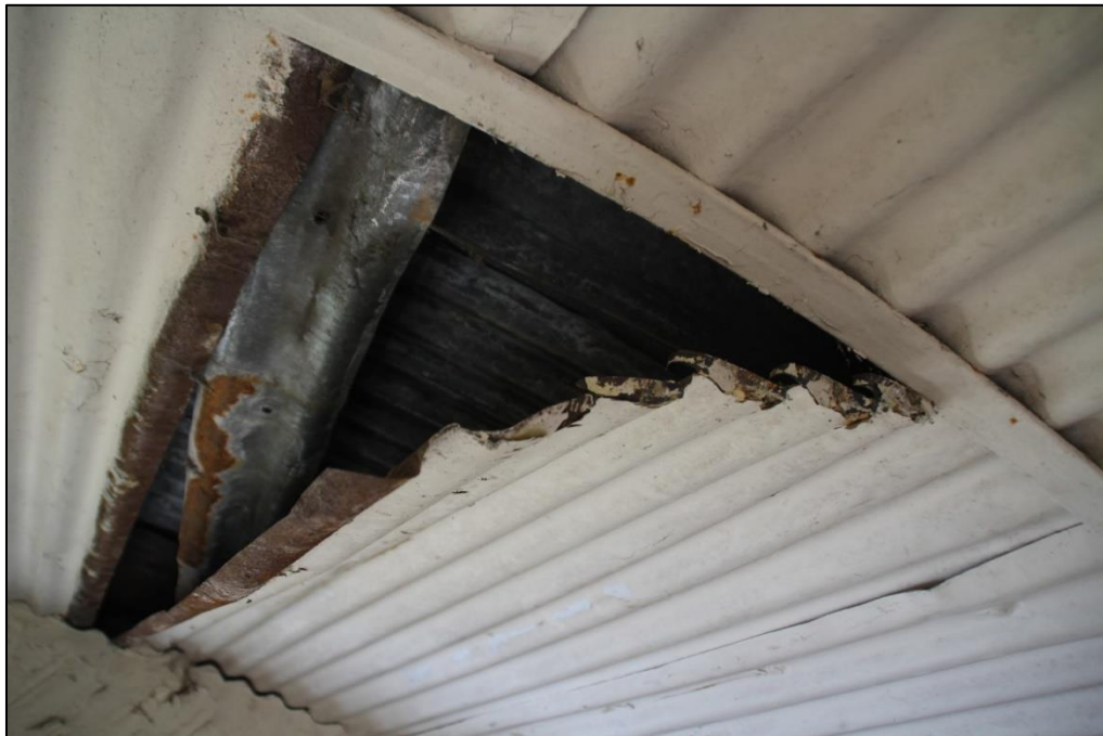
Photo 30: View of cladding and interior void
