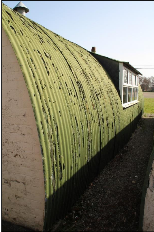
Photo 25: External view of south side of Hut 79
