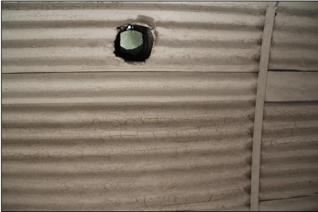
Photo 31: View of the former stove flue hole
