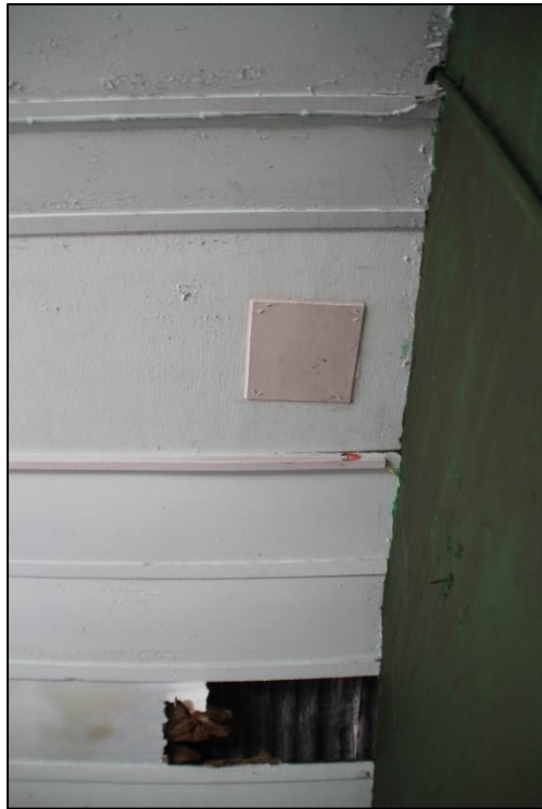
Photo 34: Interior view of the covered flue hole in the office hut (77
