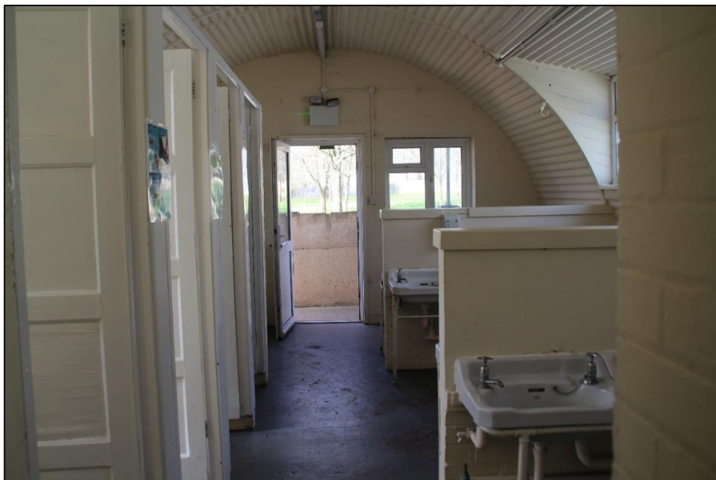
Photo 44: Internal view of the Toilet hut looking west
