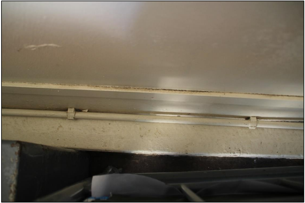
Photo 16: Detail of concrete 'rim' to floor
