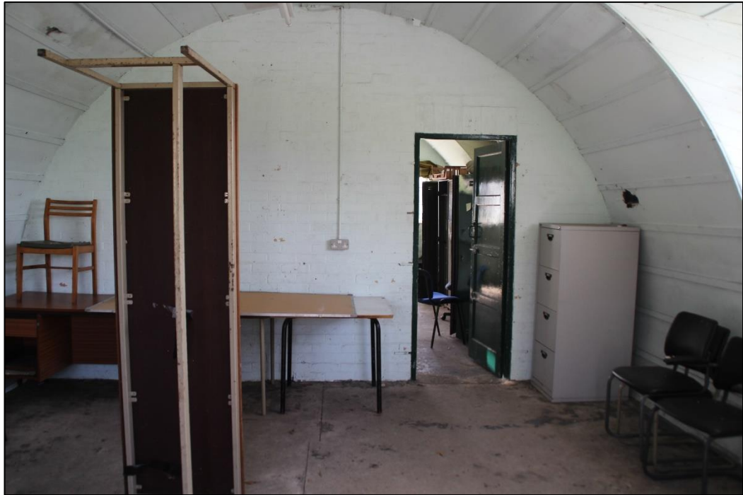
Photo 50: Internal view of hut 71 looking east
