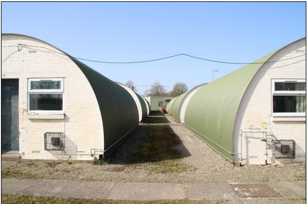
Photo 7: View through Huts 103 and 102
