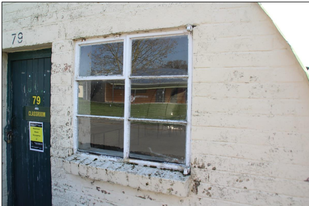
Photo 26: Detail of metal Crittall window in Hut 79
