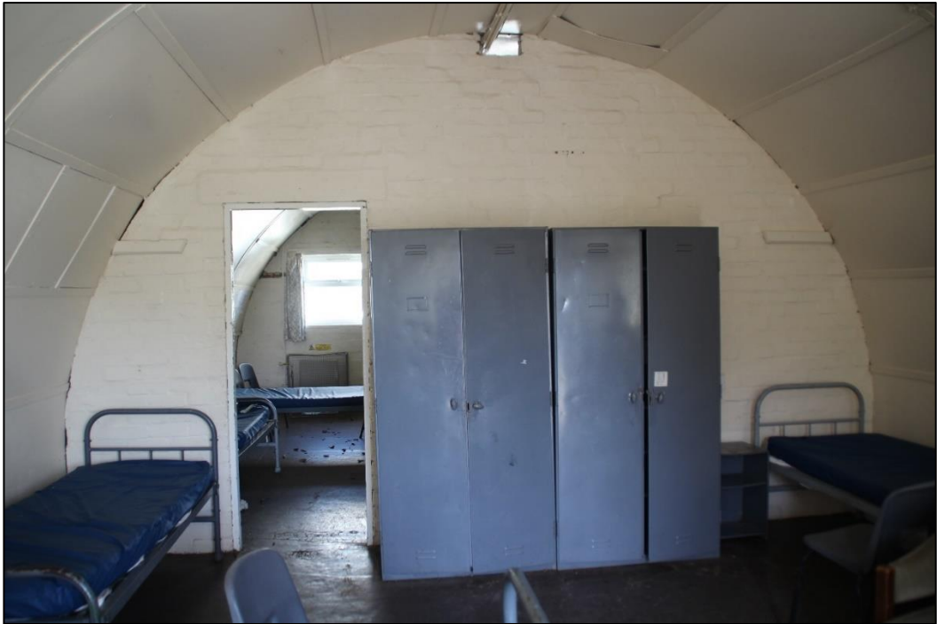
Photo 10: Internal view of Hut 105 looking west
