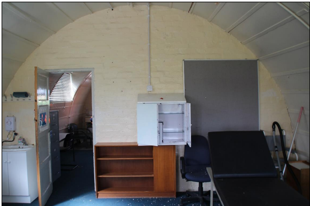
Photo 41: View of internal central wall – Medical Hut
