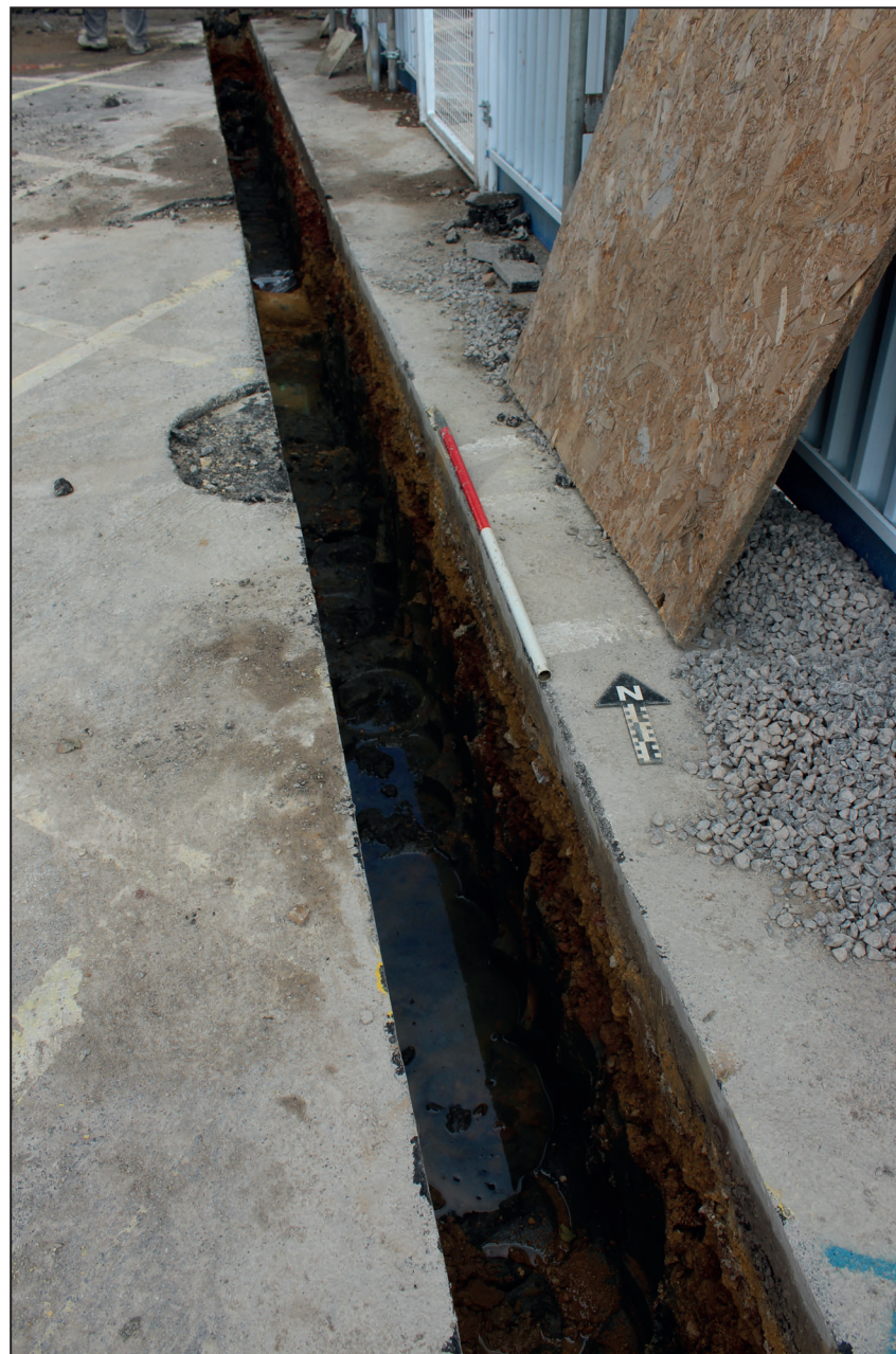
General view of Trench 8, looking north (1m scale)
