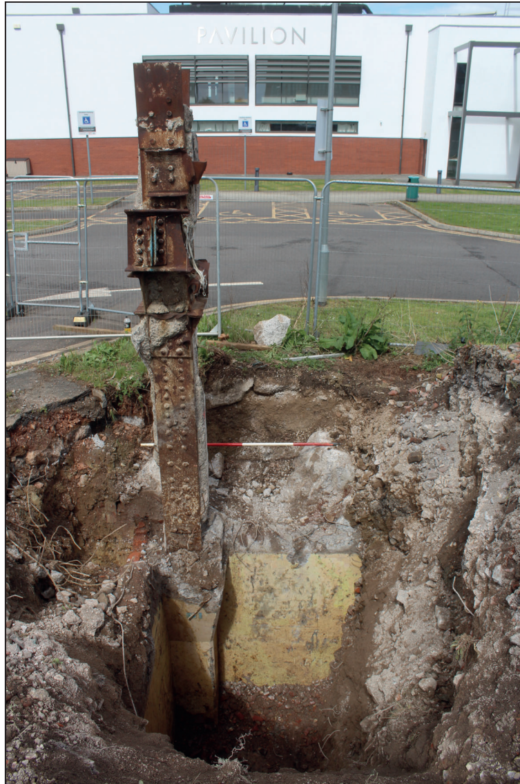
Trench 3, looking north-west (2m scale)
