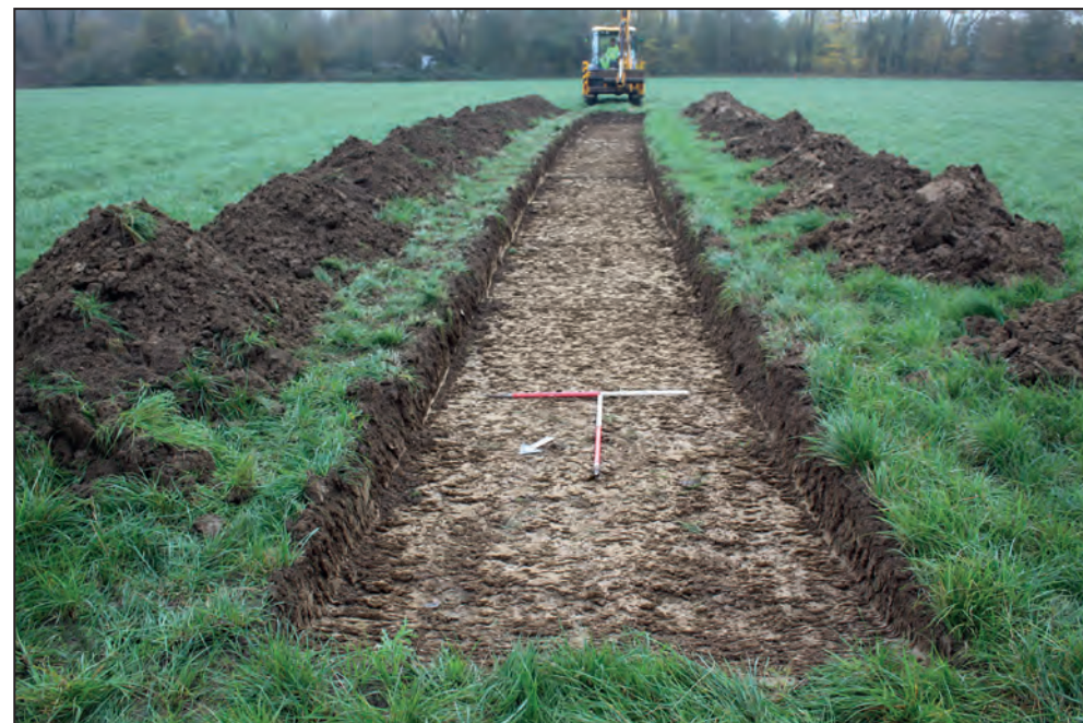
Trench 71, looking south-east (1m scales)
