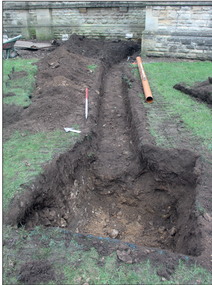
Trench 101, looking north-east (scale 1m)
