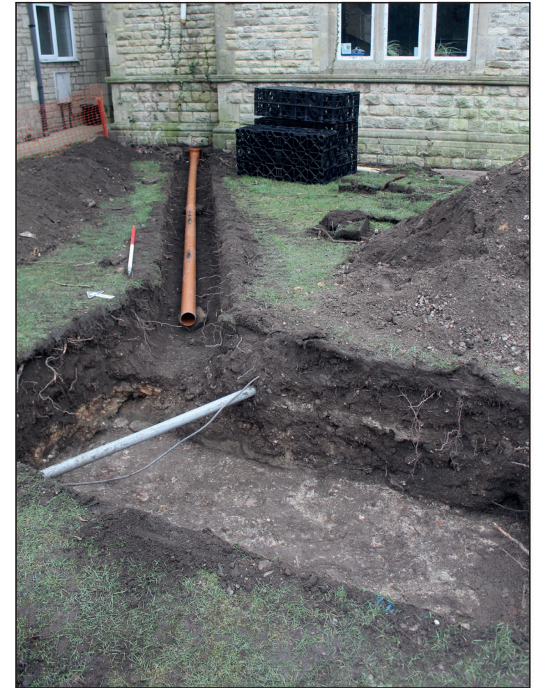
Trench 102, looking north-east (scale 1m)
