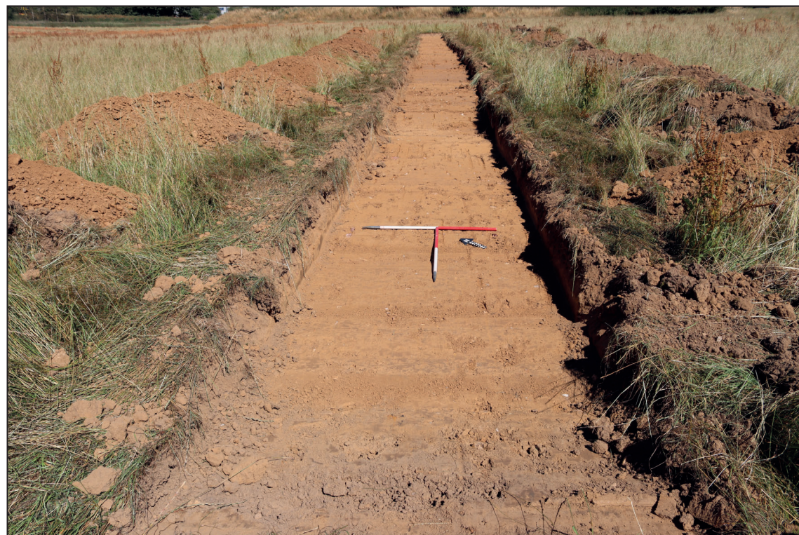
Trench 23, looking north-east (1m scales)
