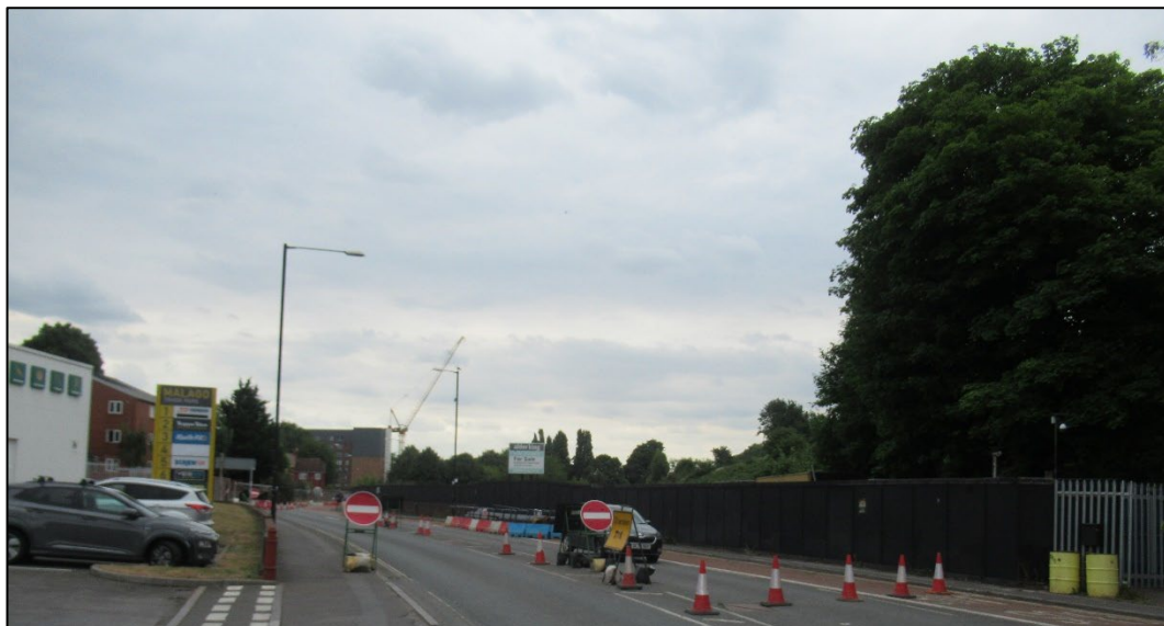
Photo 10 P3 Looking north-east along Malago Road
