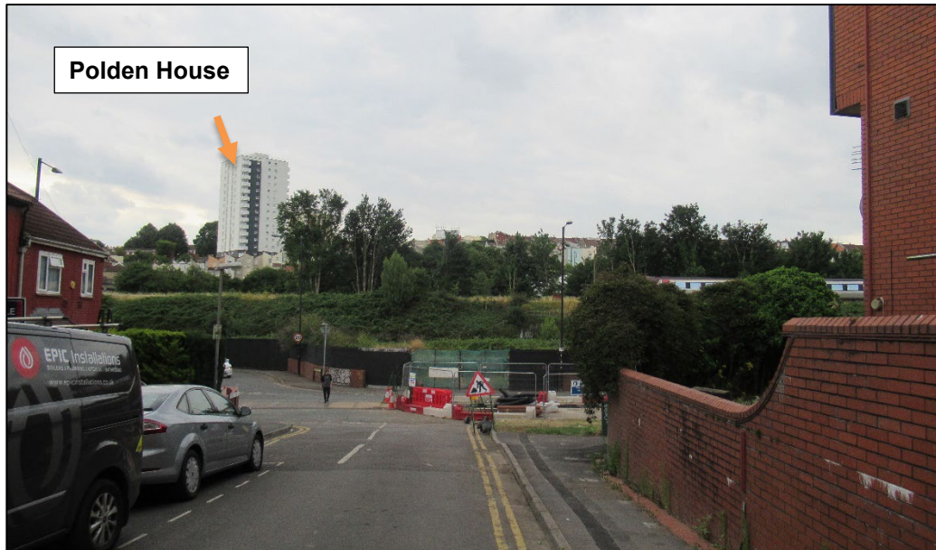
Photo 9 P8 Looking south along Church Lane towards the Site
