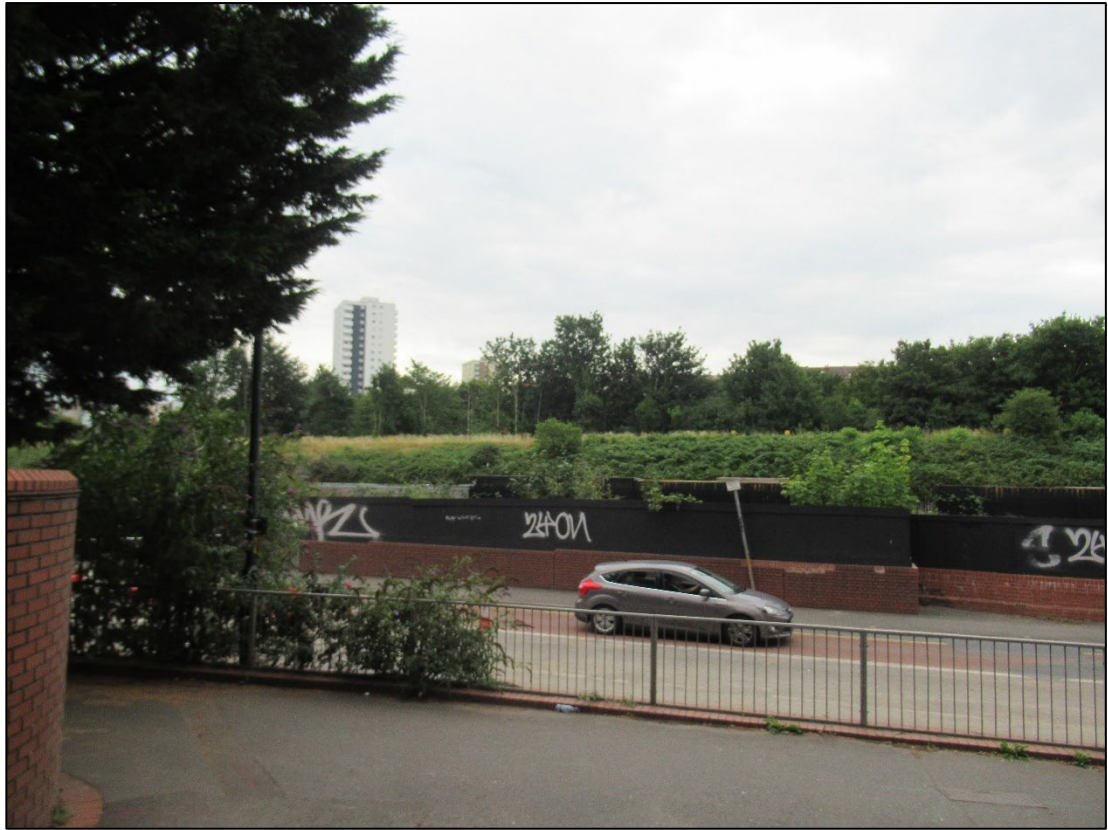
Photo 4 The Site from the Malago Road flats, facing south
