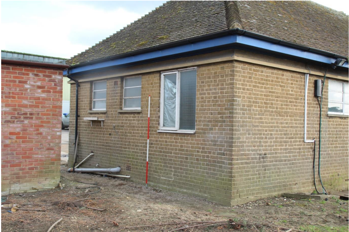
Figure 37 The north elevation of Building 3 (scale 2m)
