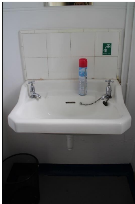
Photo 85 Detail of sink in Ladies toilet
