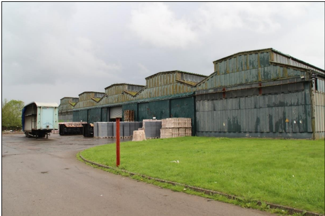
Photo 13 View of the west elevation of store block 2 viewed looking north-west
