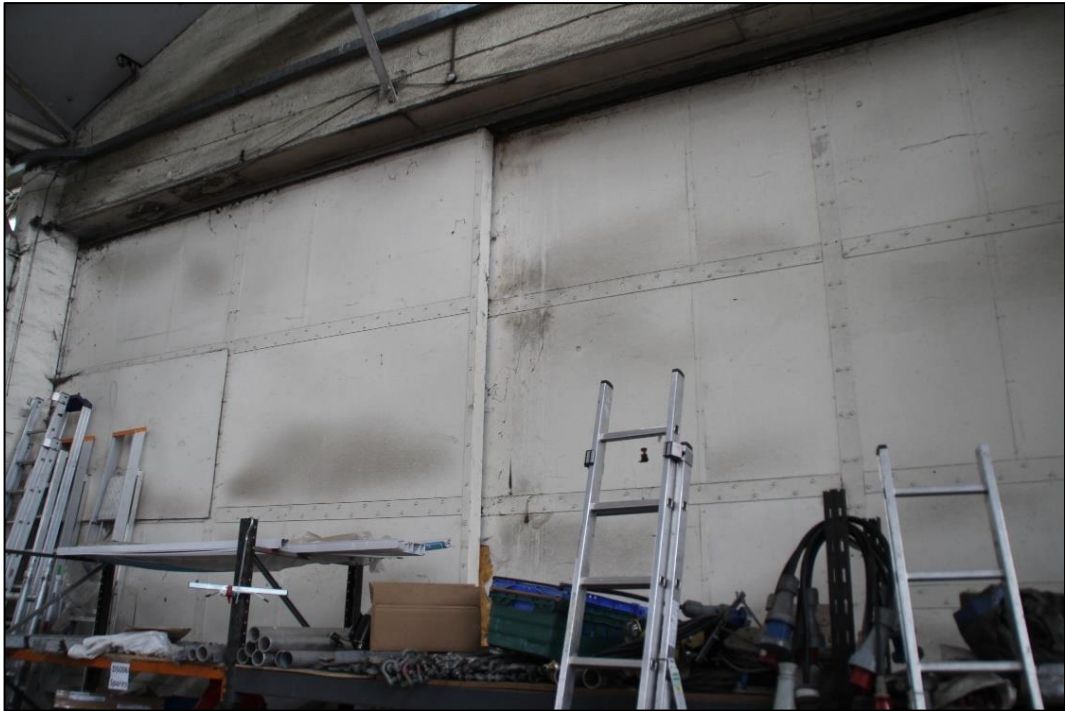
Photo 20 View of the interior of sliding metal framed doors
