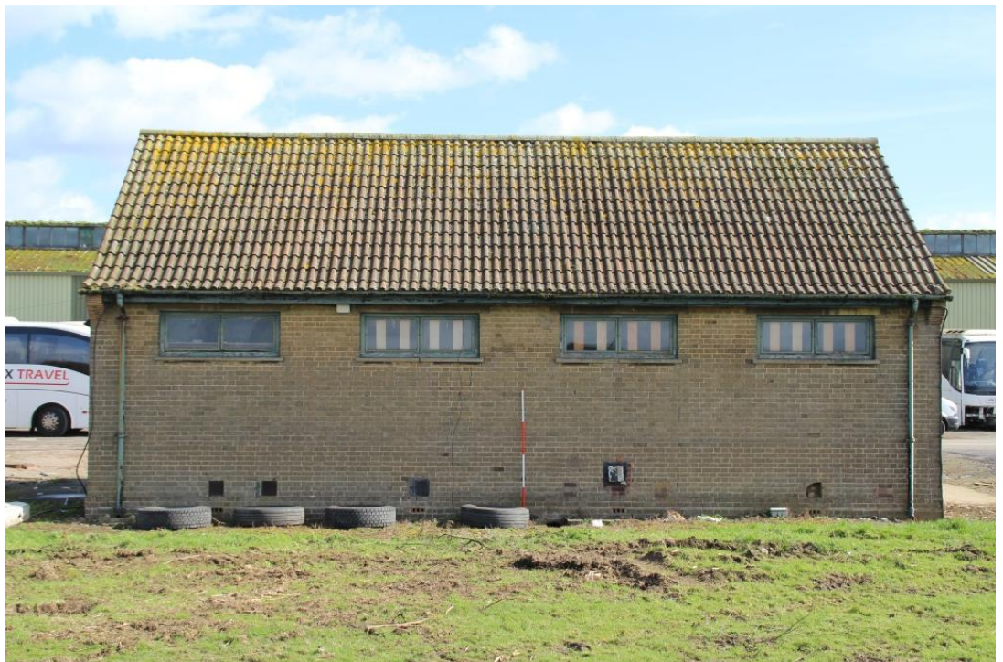
Figure 26 The west elevation of Building 2 (scale 2m)
