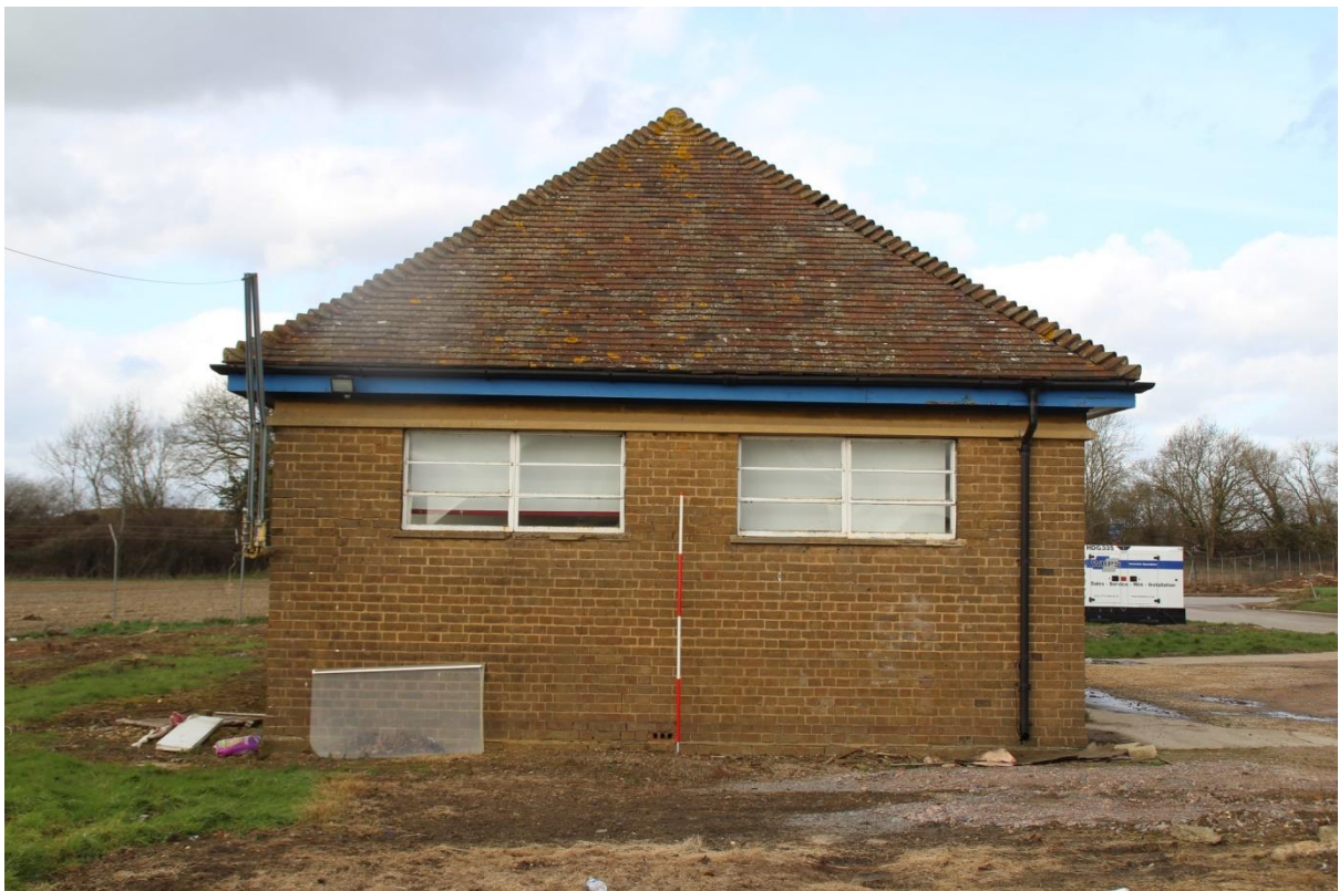
Figures 35 and 36 The west and south elevations of Building 3 (scale 2m)
