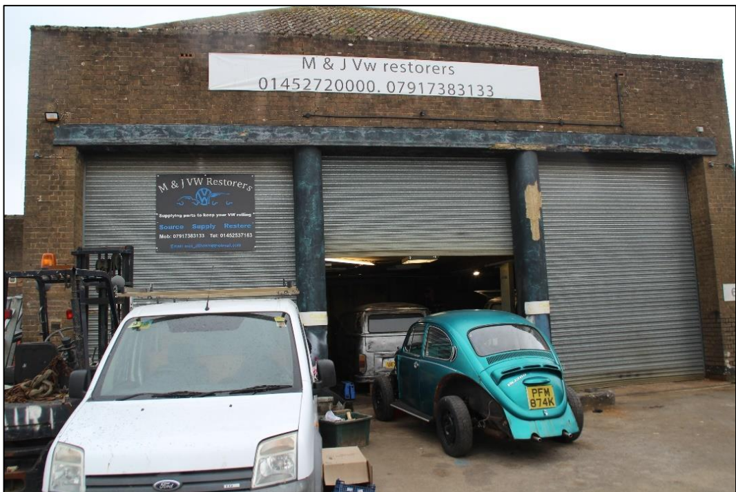
Photo 59 Close view of the vehicle openings to the main south elevation of the repair garage
