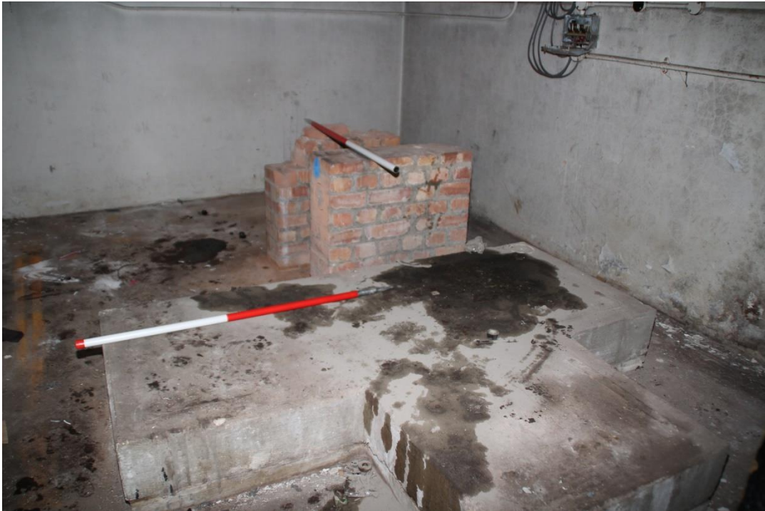
Figure 19 The machinery bases in G8 looking north-west (scale 2m)
