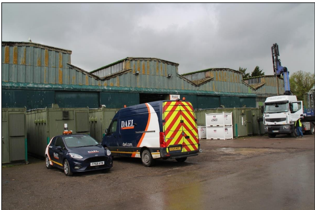
Photo 14 View of the northern elevation of store block 2
