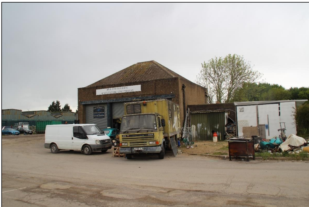
Photo 57 View of the front (south) elevation of the repair garage
