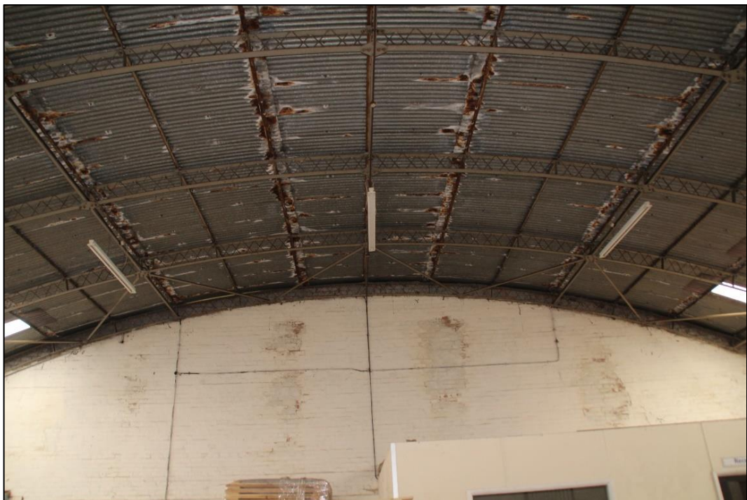
Photo 47 Internal view of the roof structure of the blister hangar
