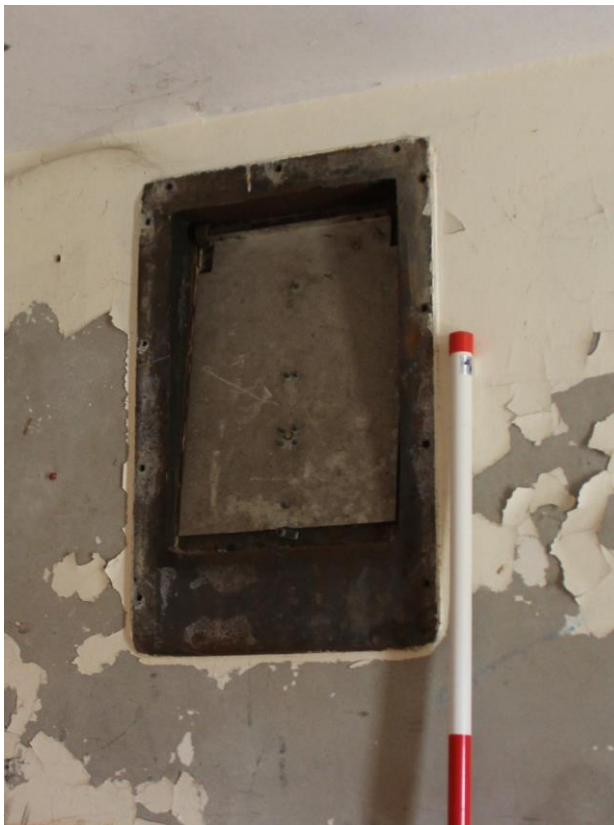
Figure 14 Room G in Building 1, showing the glass block window in the east wall and the heavy hatch closing the louvre under it, cf Fig. 6. Also visible is the black plastic cladding (scale 2m)
