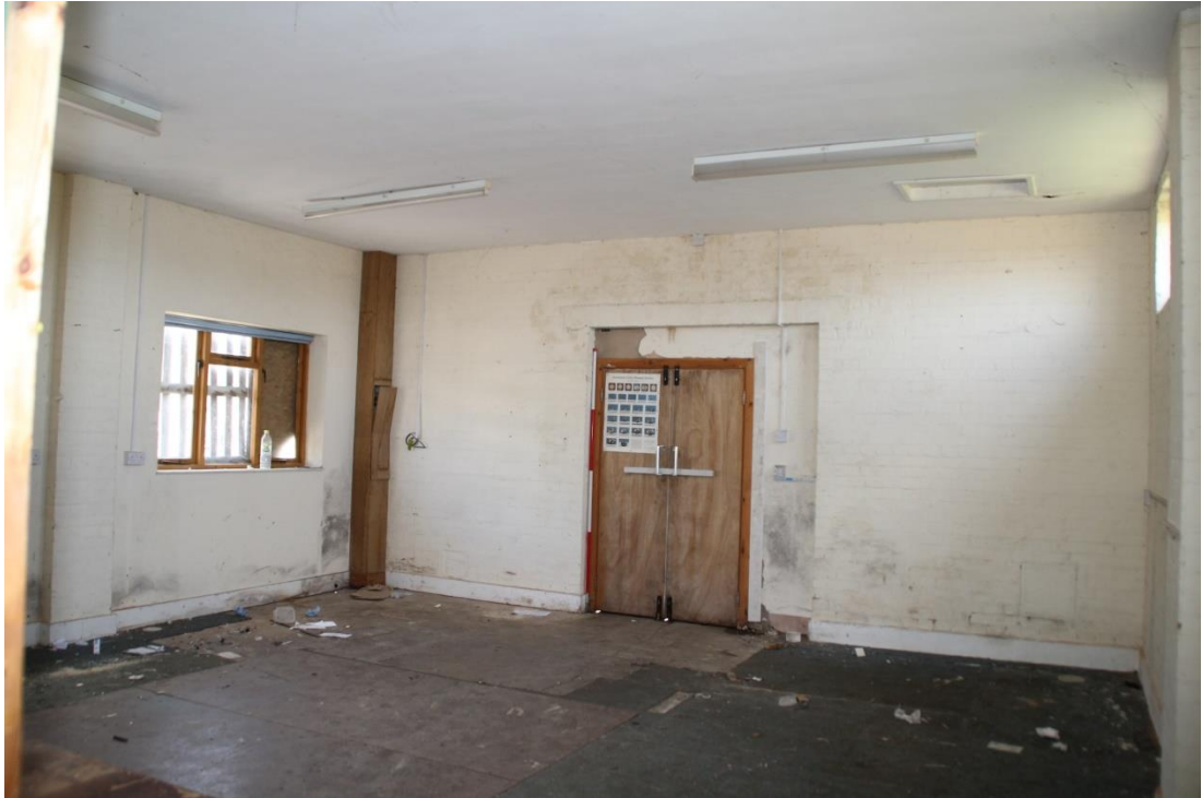
Figure 29 Building 2: Room G4 looking south-east (scale 2m)
