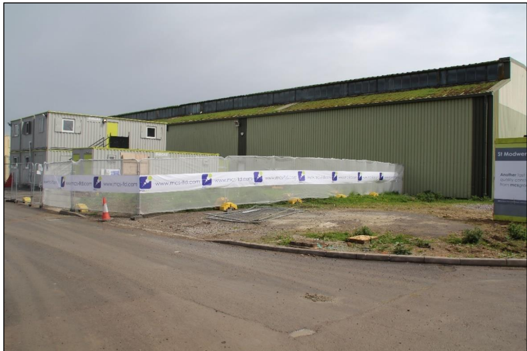
Photo 3 Store block 1 western elevation viewed looking north
