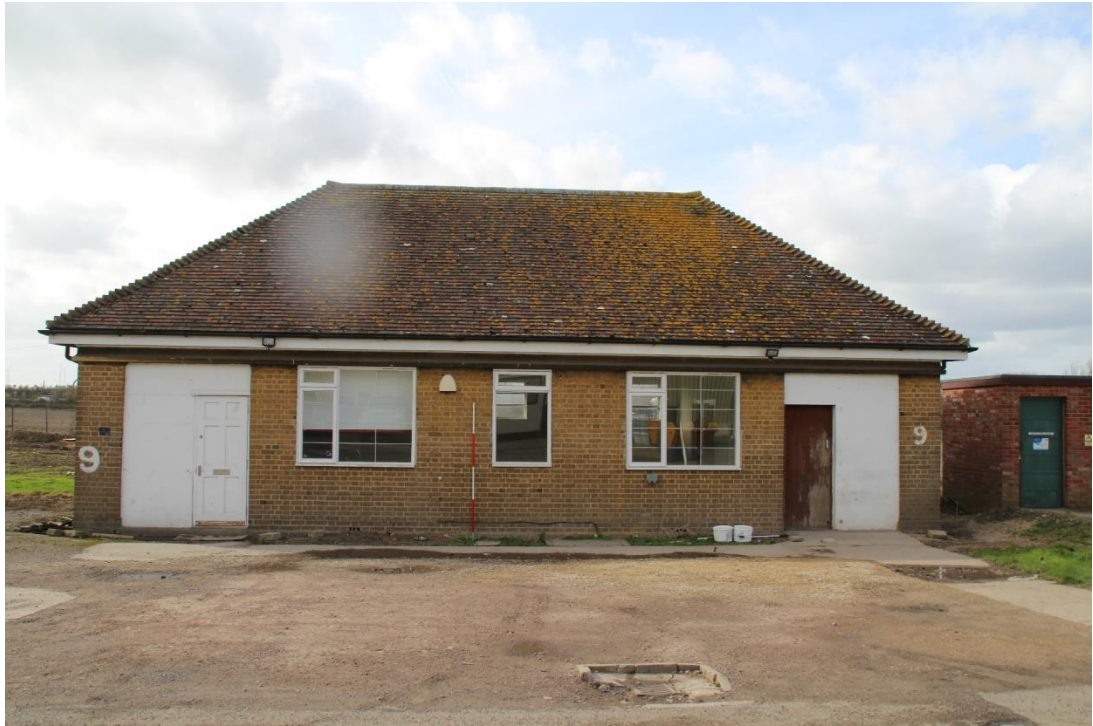
Figure 31 East elevation of Building 3 (scale 2m)
