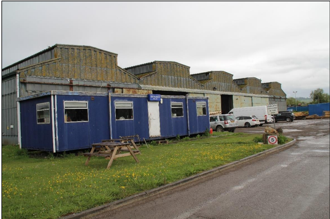
Photo 34 View of the southern elevation of store block 3
