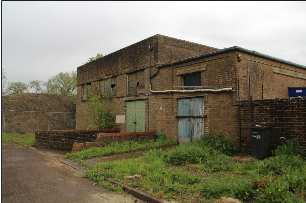
Photo 51 View of the western elevation of the CHS with entrances
