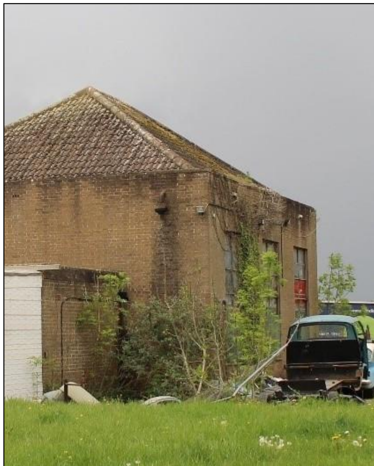
Photo 63 View of the rear (north) of the repair garage
