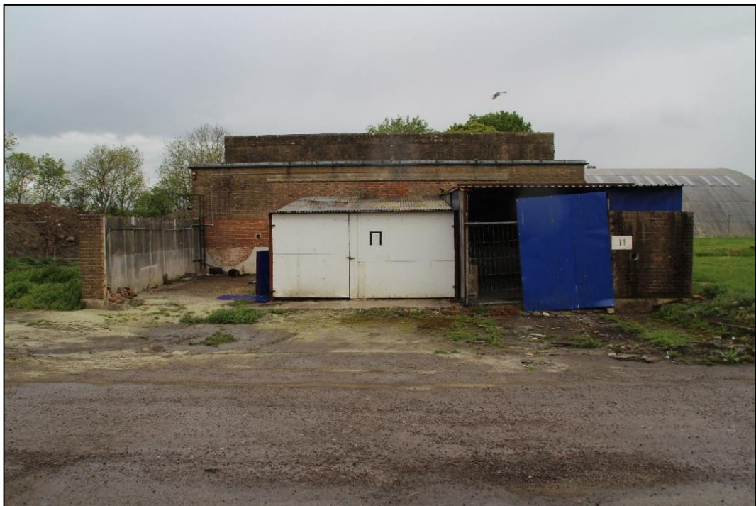
Photo 50 View of the former fuel tank storage compound
