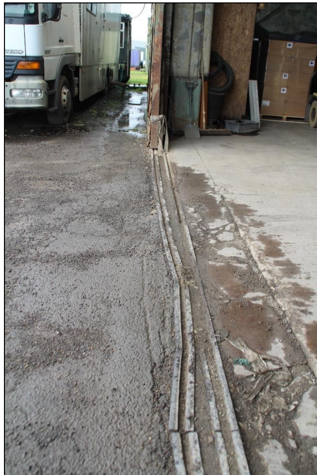
Photo 38 View of the sliders of the doors to store block 3
