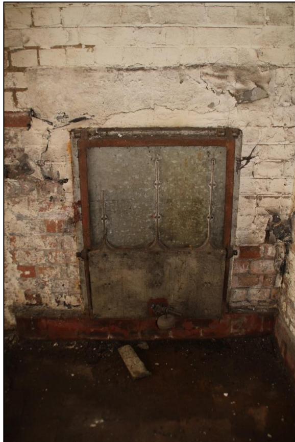
Photo 53 View of the metal door of the coal chute
