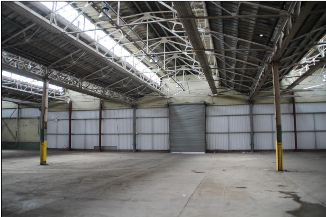
Photo 7 View of internal south elevation (former sliding door area)
