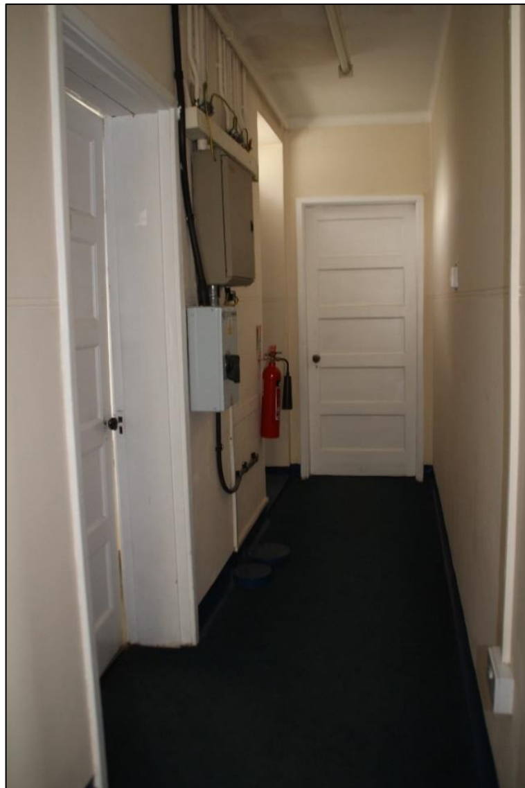
Photo 78 View of internal corridor crossing the main arm of the T plan
