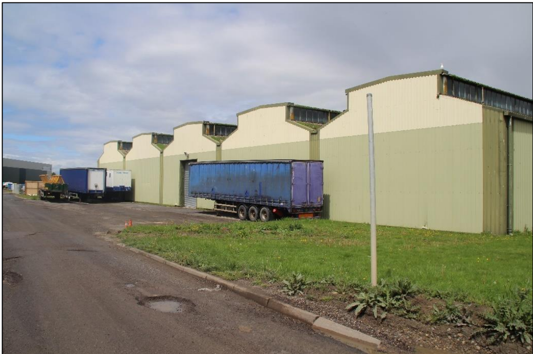
Photo 1 Store block 1 viewed looking north-west
