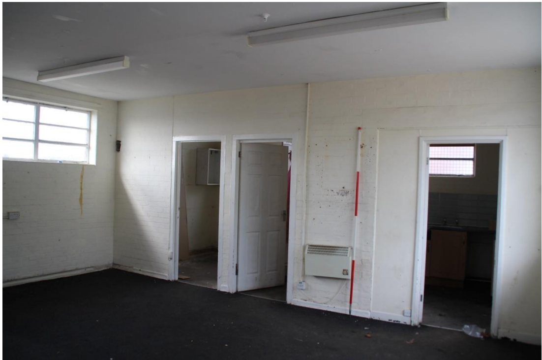
Figure 32 Building 3, Room G2, looking north-west and doors to G1-G3 (scale 2m)
