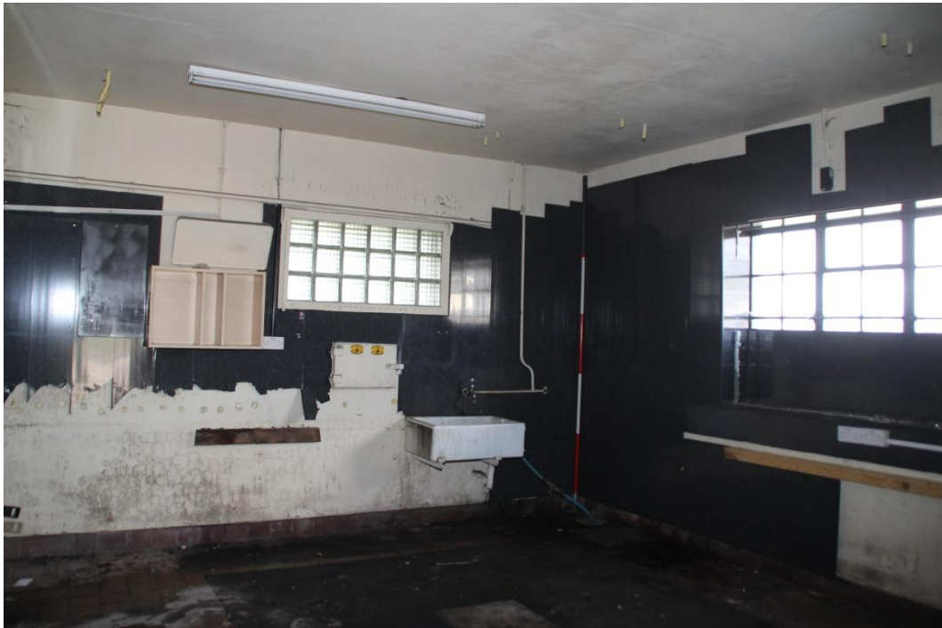
Figure 14 Room G in Building 1, showing the glass block window in the east wall and the heavy hatch closing the louvre under it, cf Fig. 6. Also visible is the black plastic cladding (scale 2m)
