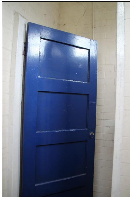
Photo 83 Detail of panelled door to cubicle in Ladies toilet
