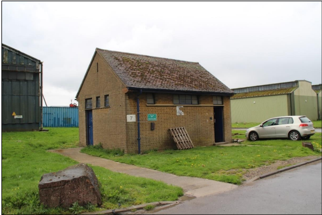
Photo 82 View of Building 9, toilet block, image taken looking south-west
