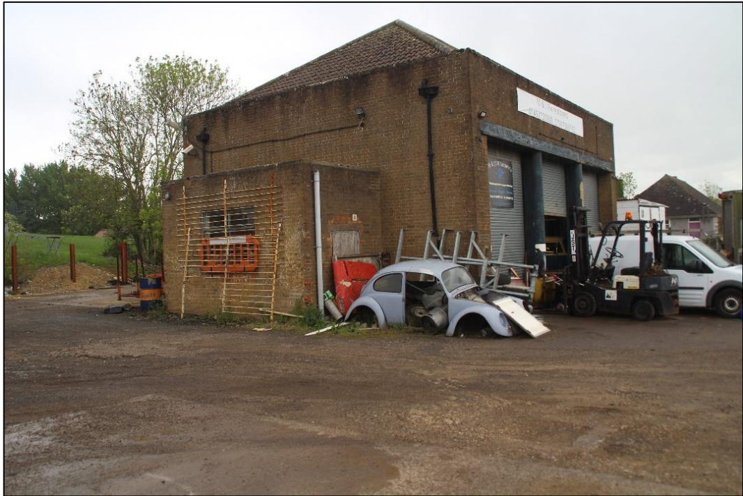
Photo 58 View of the west elevation of the repair garage
