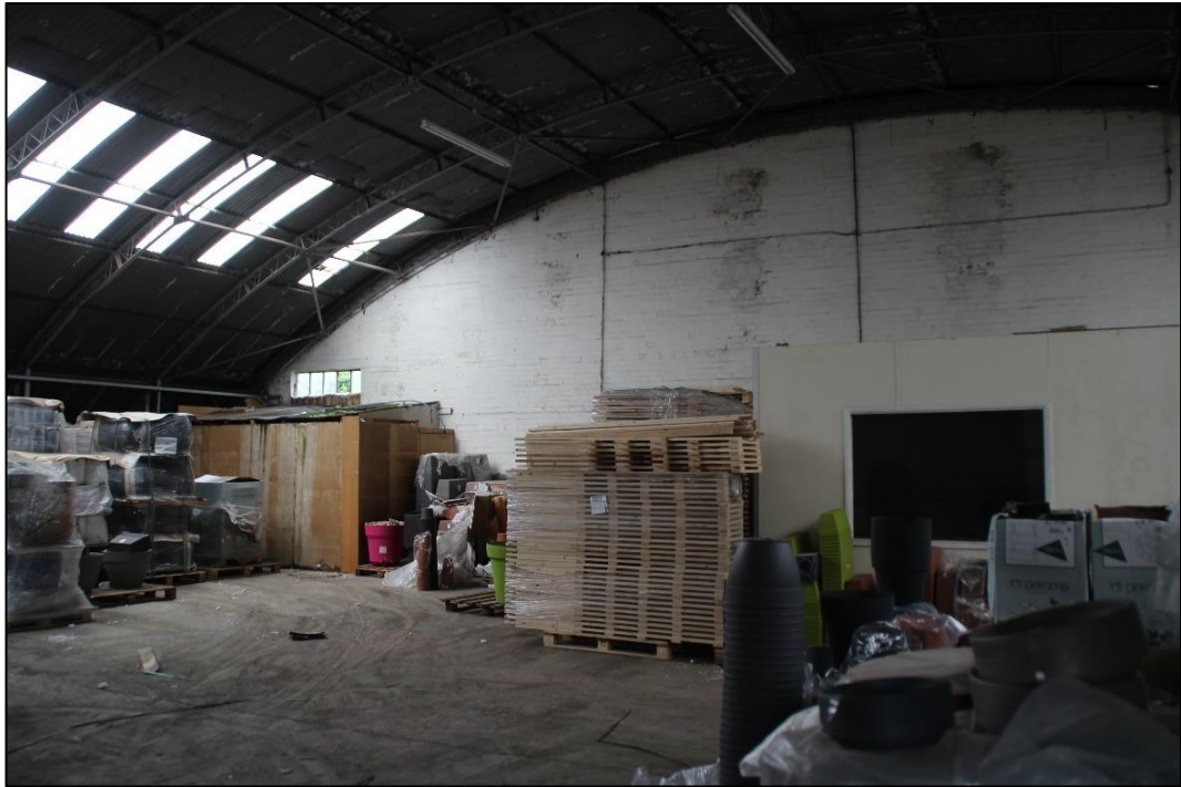
Photo 48 Internal view of the blister hangar looking south-west
