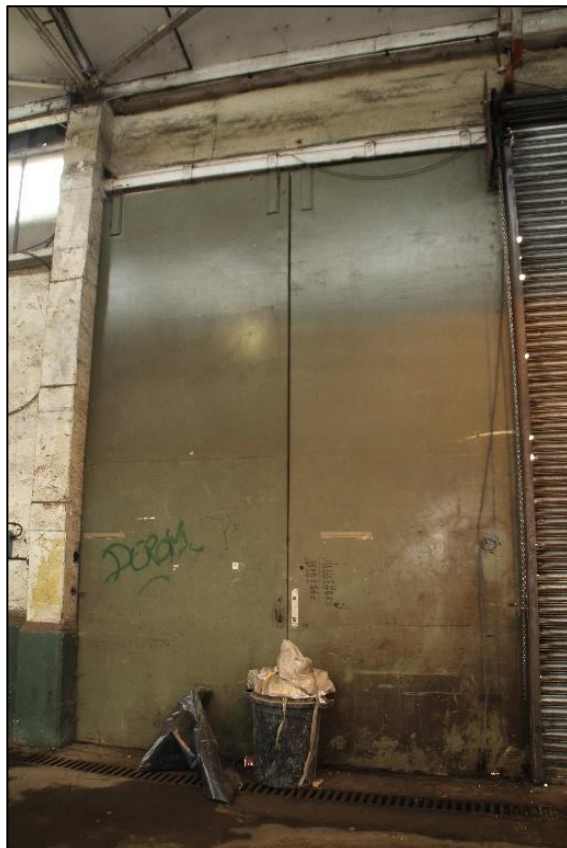
Photo 43 Internal view of metal side door of store block 3 (eastern side)
