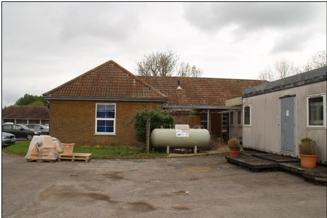
Photo 76 View of the southern elevation of the canteen
