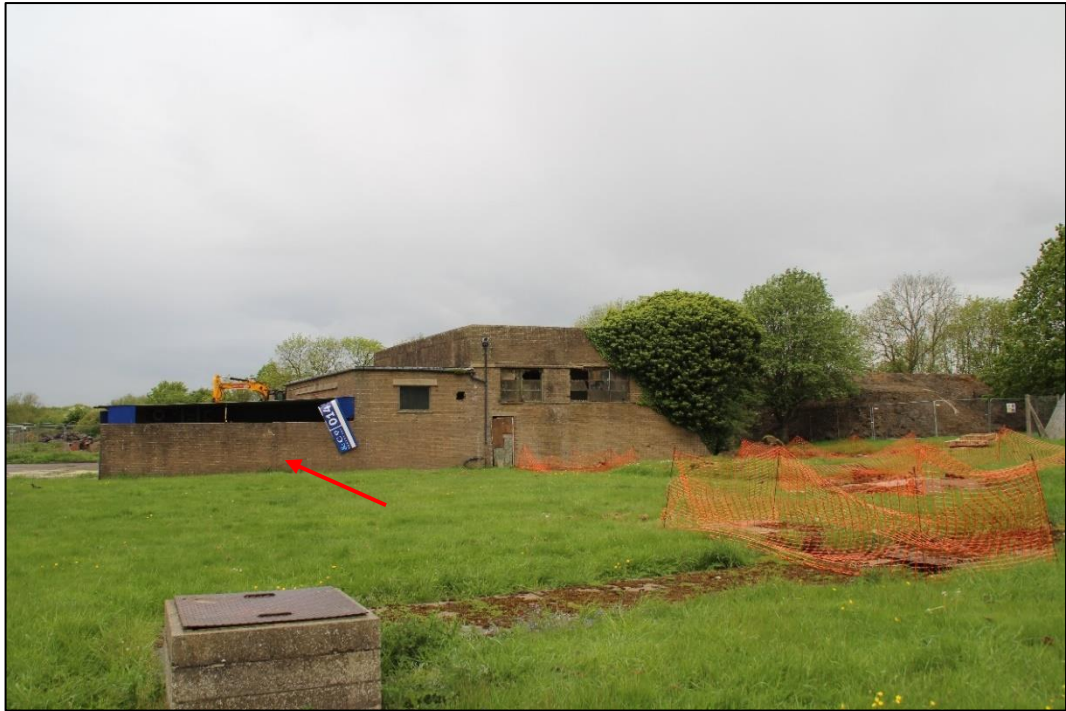
Photo 49 External view of the eastern elevation of the Central Heating Station with fuel tank storage compound arrowed
