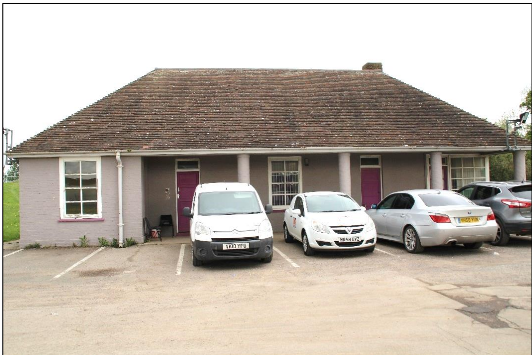
Photo 67 View of the front (south) elevation of the Warden's building
