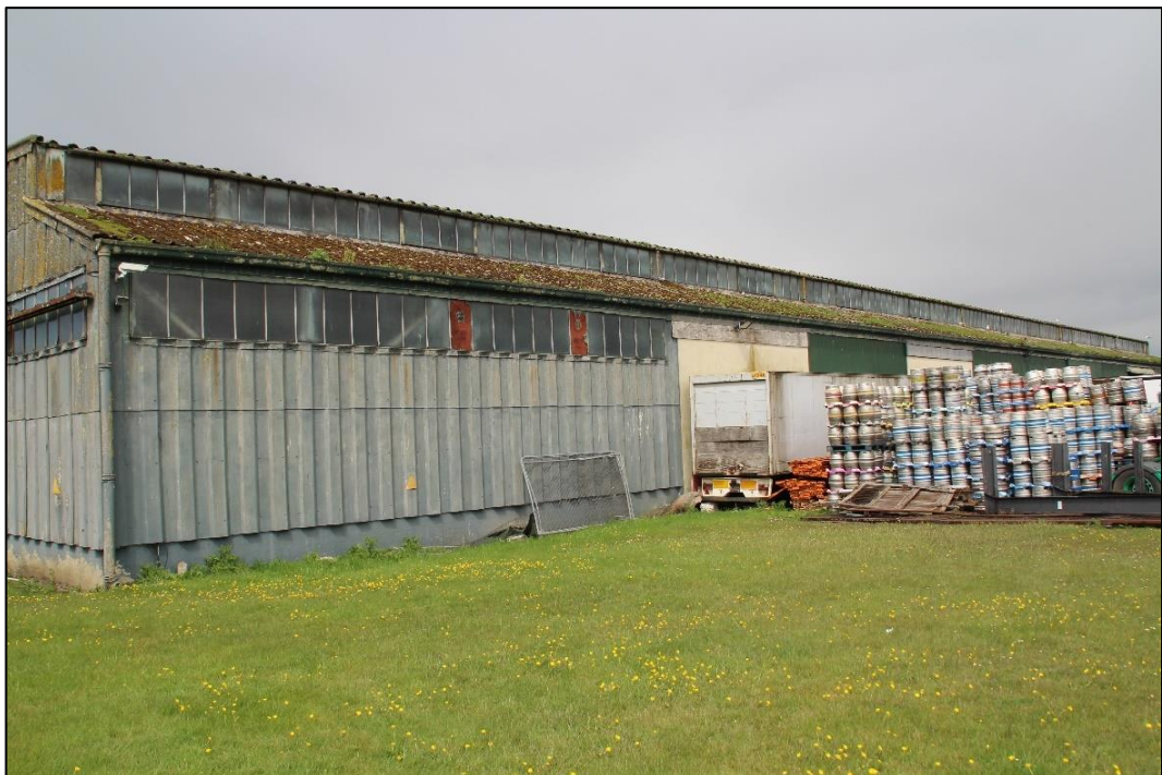
Photo 35 View of the eastern elevation of store block 3
