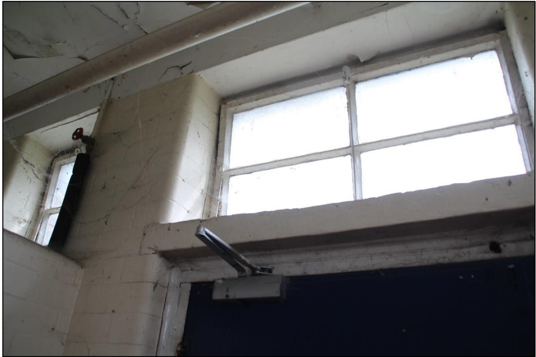
Photo 84 Detail of high-level metal windows in Ladies toilet
