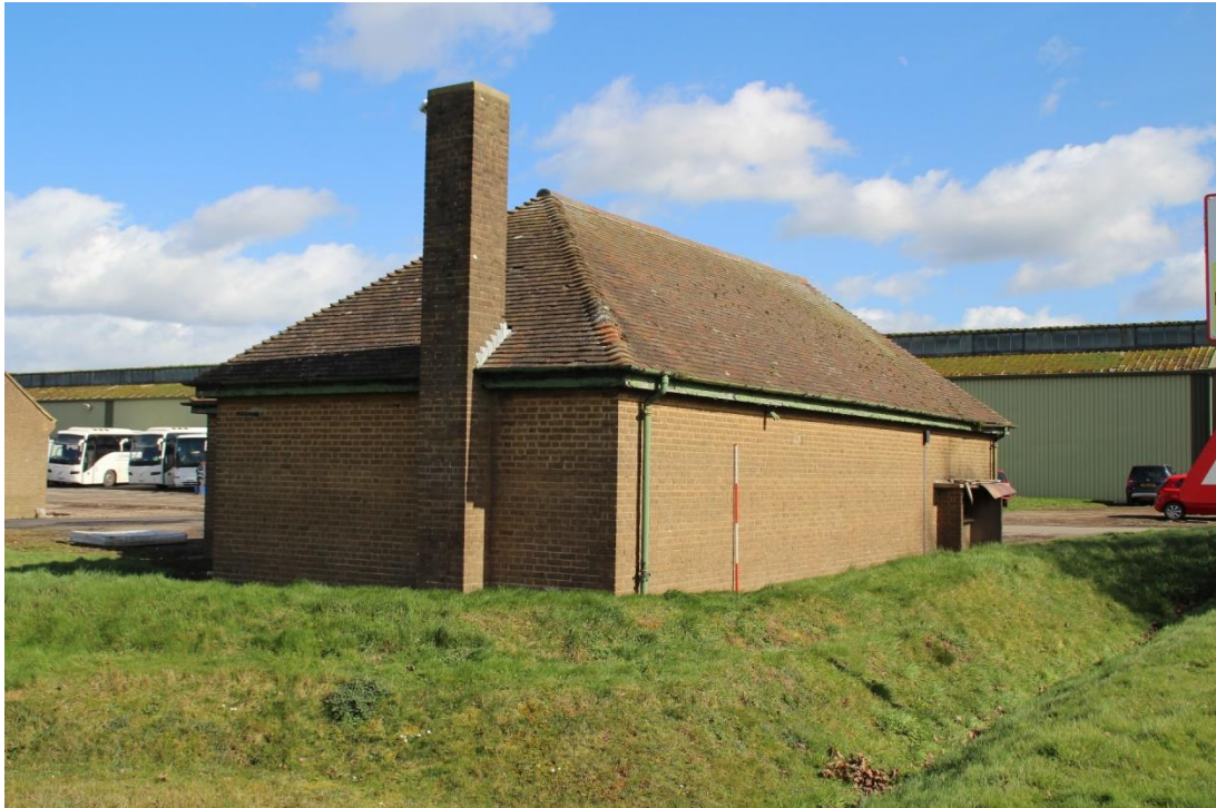
Figure 4 Building 1 looking north-east (scale 2m)
