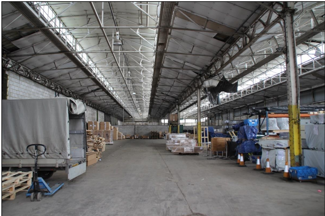
Photo 42 Internal view of store block 3 looking north in the eastern section
