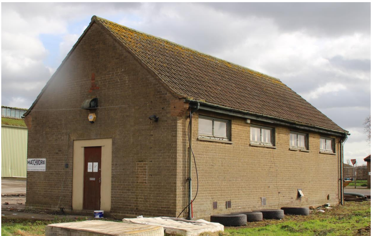
Figure 21 Building 2 looking south-east (scale 2m)
