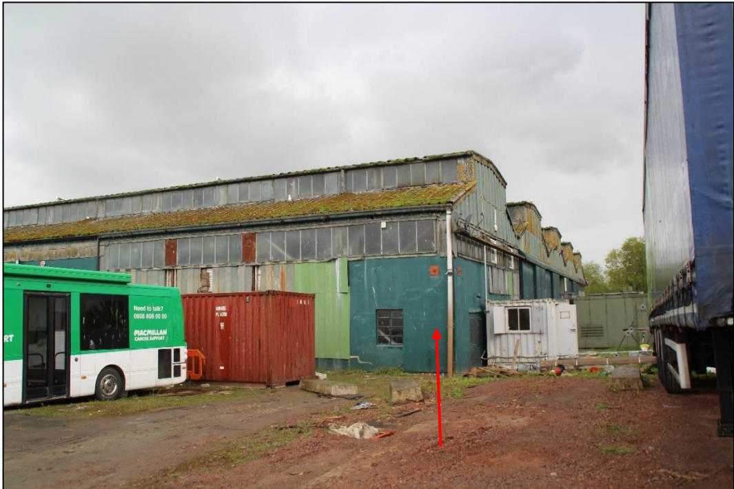
Photo 15 View of the south-west corner of store block 1 (unusual anomaly arrowed)
