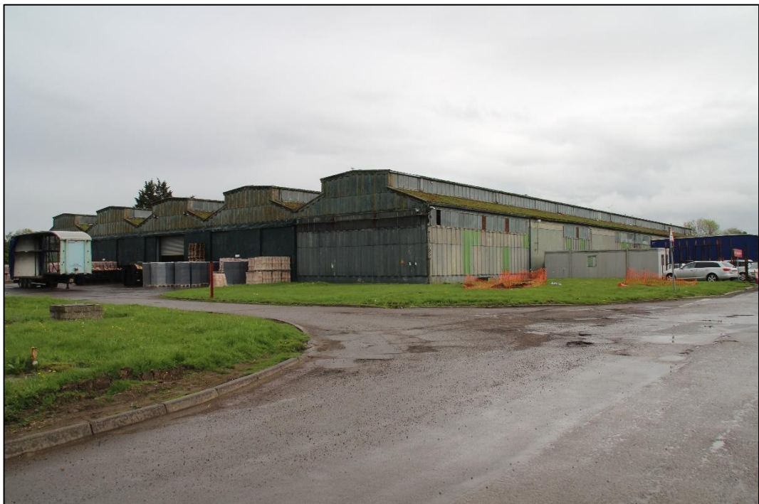
Photo 33 View of the northern elevation of store block 3, image taken looking south
