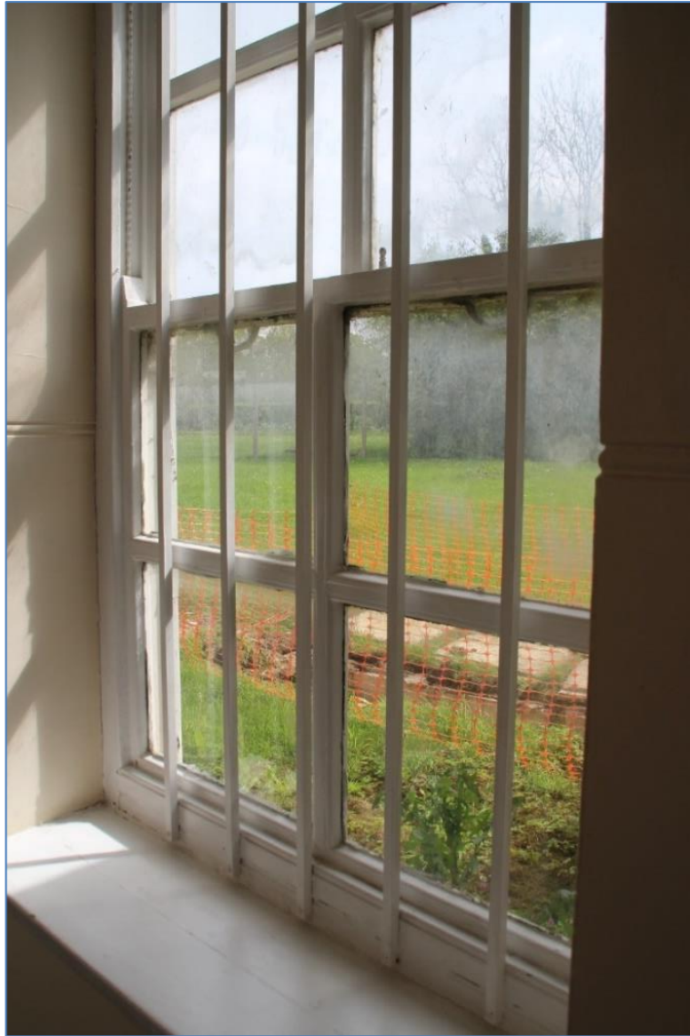
Photo 81 Detail of original timber window with bars on the canteen kitchen
