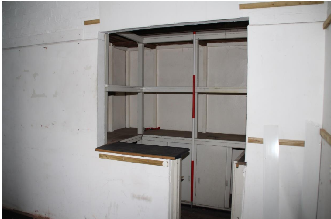
Figure 18 G4 seen from G2 looking south-east (scale 2m)
