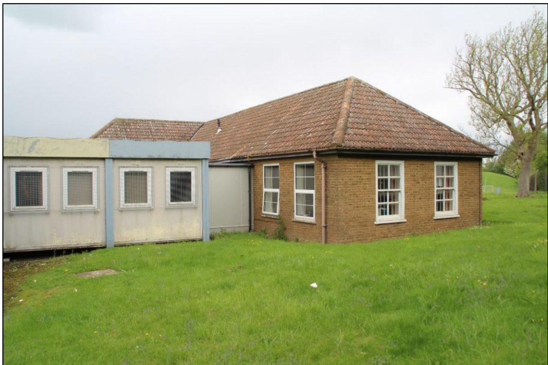
Photo 75 View of the rear (eastern) elevation of the canteen
