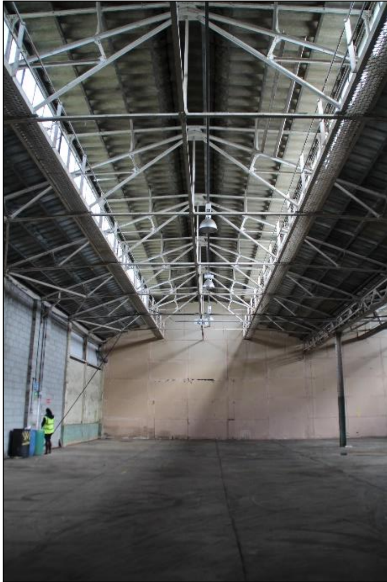
Photo 6 View of the roof truss running north-south
