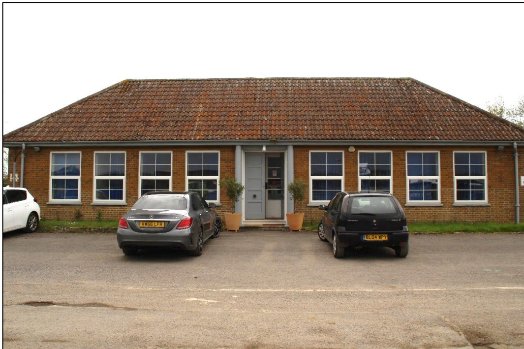
Photo 73 Front (western) elevation of the canteen building
