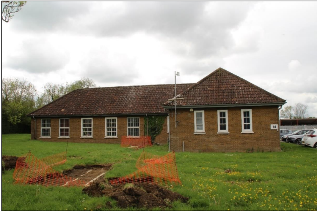
Photo 74 View of the north elevation of the canteen
