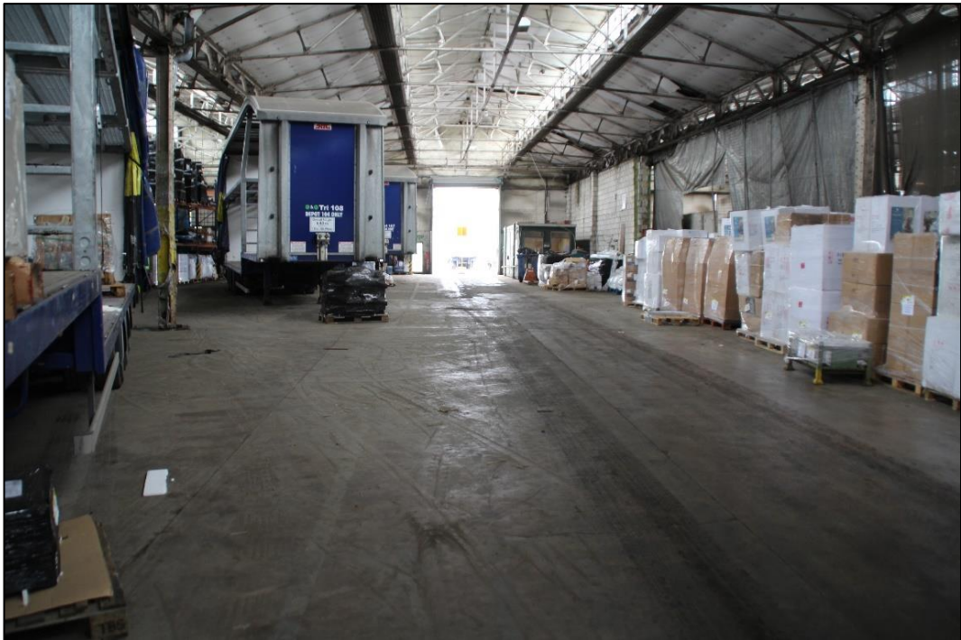
Photo 41 Internal view of store block 3 looking north
