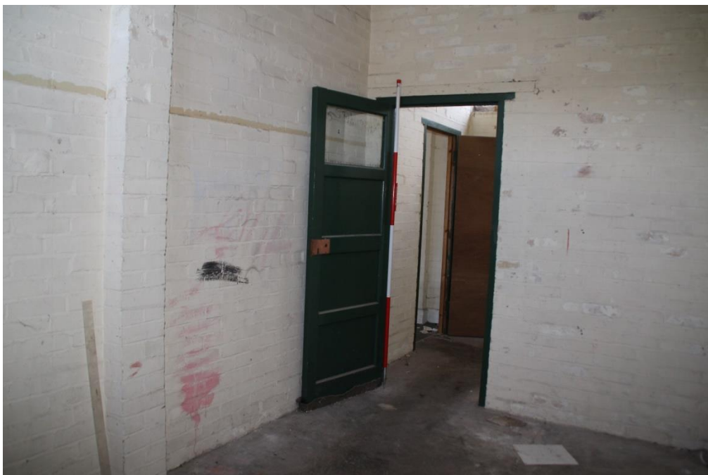
Figure 28 Building 2: Room G2 looking into G3 (scale 2m)
