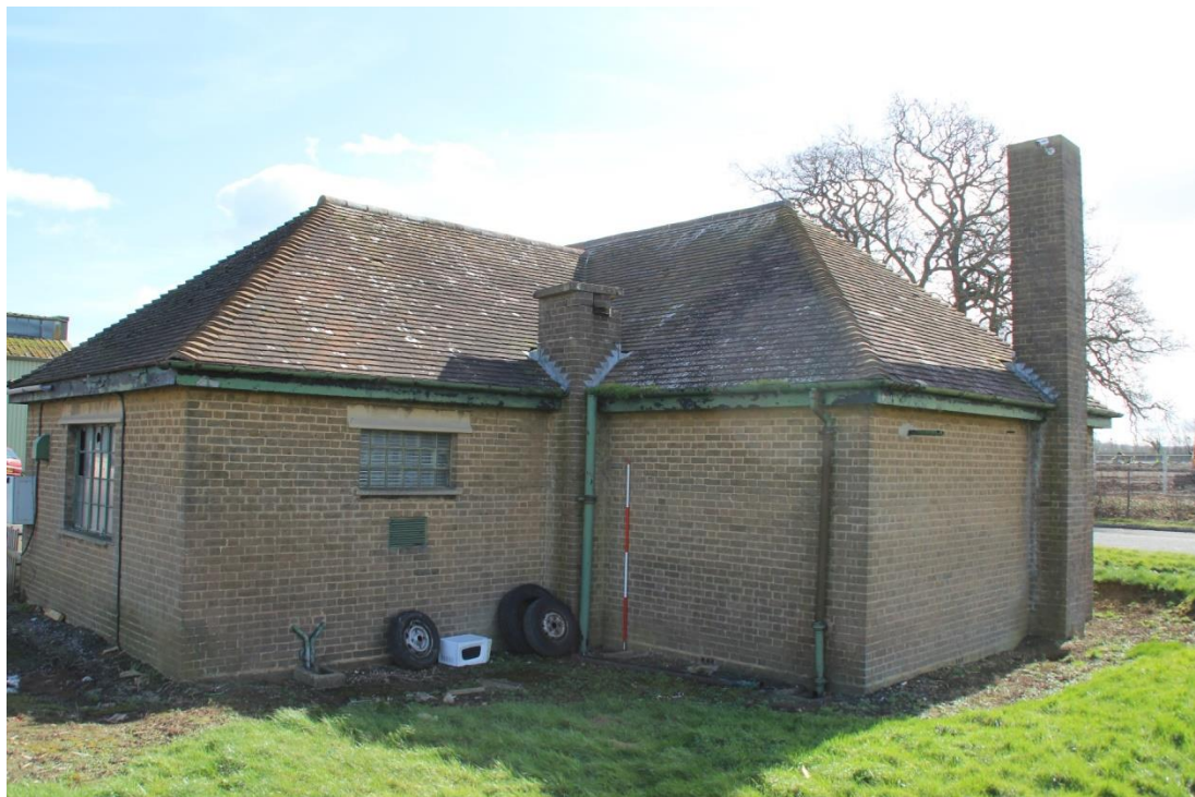
Figure 6 Building 1 looking south-east (scale 2m)
