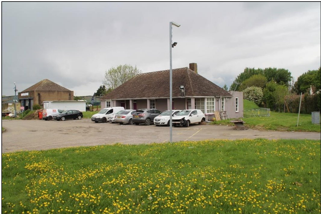
Photo 64 View of the front elevation of the Warden's building looking north
