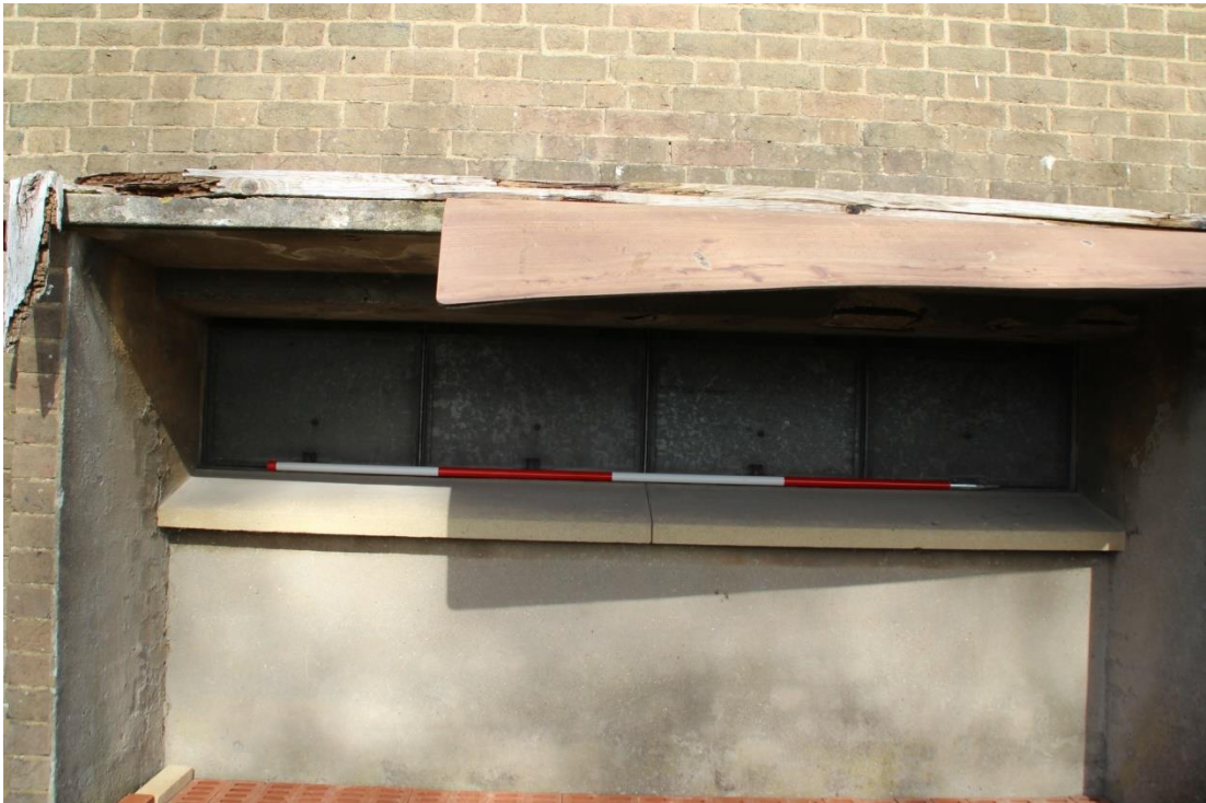
Figure 7 The steel shutters of the “delivery bay” in the south side of Building 1, cf Fig. 8 (scale 2m)
