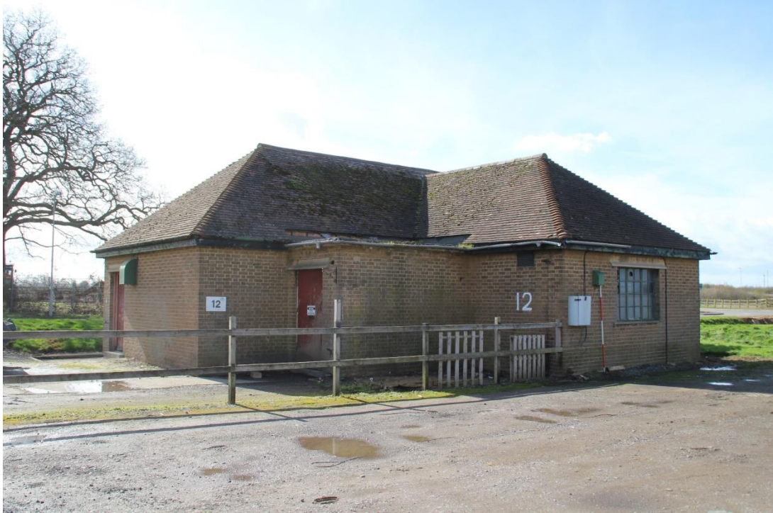
Figure 3 Building 1 looking south-west (scale 2m)
