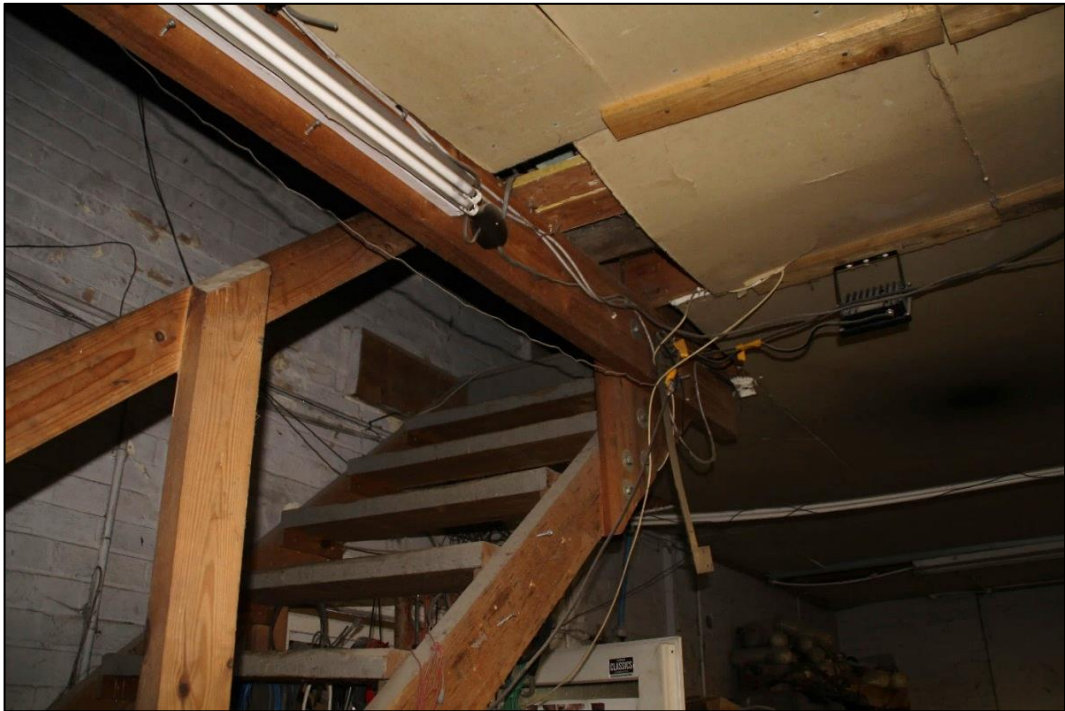
Photo 60 Timber staircase to the first-floor mezzanine, likely a later addition
