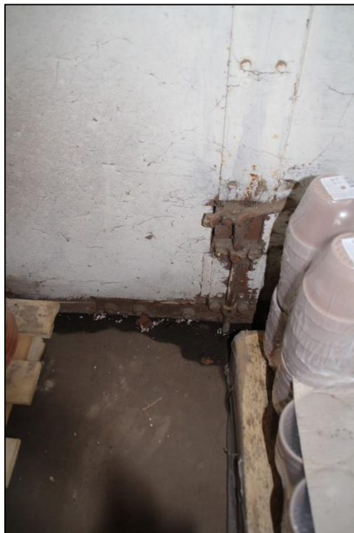
Photo 22 Detail of floor bolt on sliding door of store block 2
