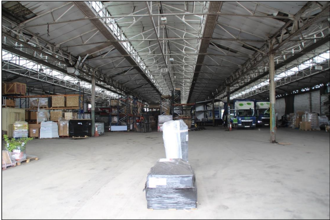
Photo 40 Internal view of store block 3 looking north
