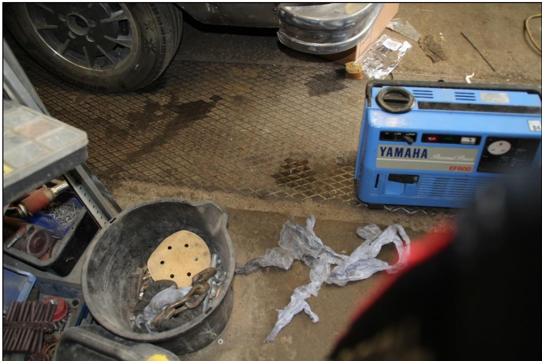
Photo 61 Metal coverings to probable former repair pits
