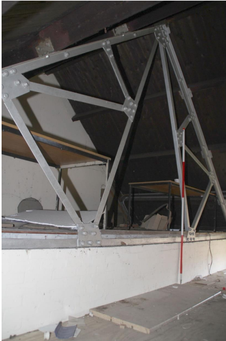
Figure 24 The northern roof truss in Building 2, looking south-west (scale 2m)
