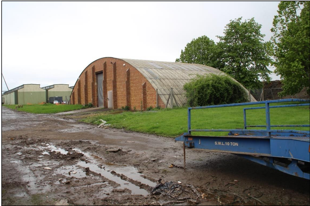
Photo 46 View of the blister hangar looking south-west
