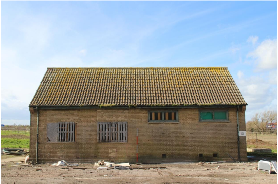
Figure 25 The east elevation of Building 2 (scale 2m)
