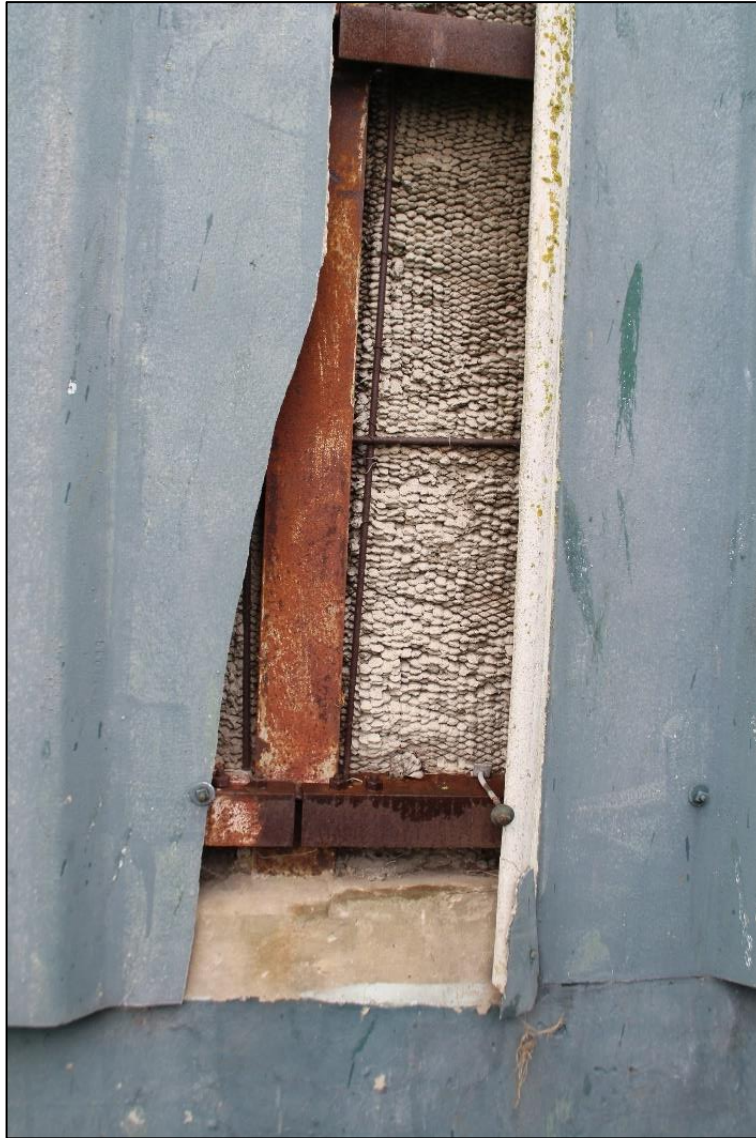
Photo 36 Detail of internal and external wall construction on store block 3
