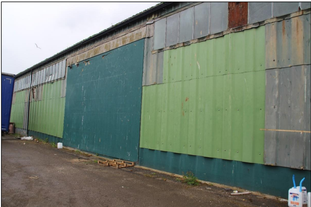
Photo 17 Detail of former opening and cladding on the south elevation of store block 2
