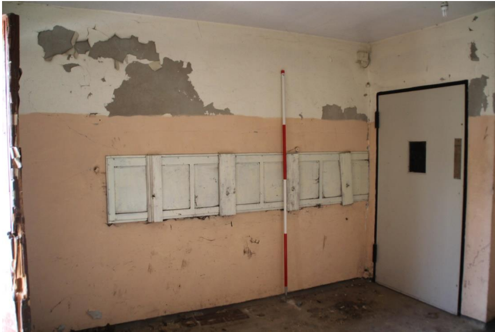
Figure 8 The steel shutters of the “delivery bay” seen within G3, looking south-west, cf Fig. 7. The wooden planks are later fixings (scale 2m)
