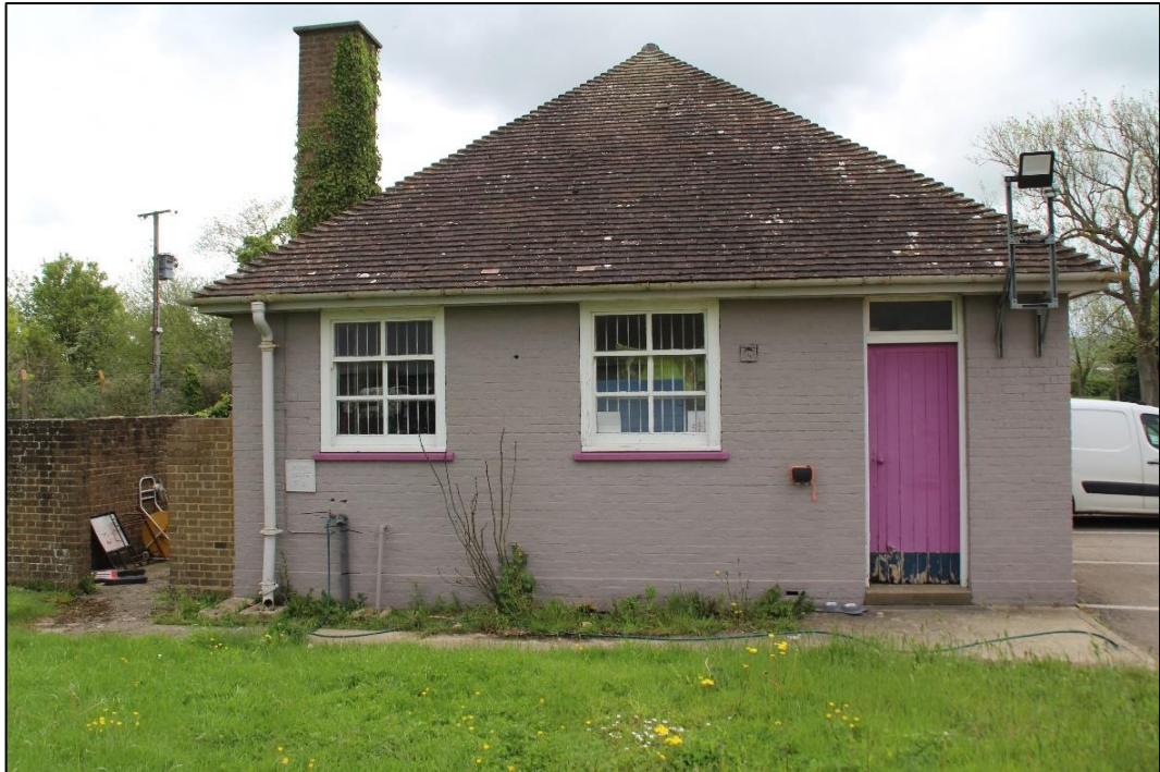
Photo 66 View of the western elevation of the Warden's building showing the small rear yard
