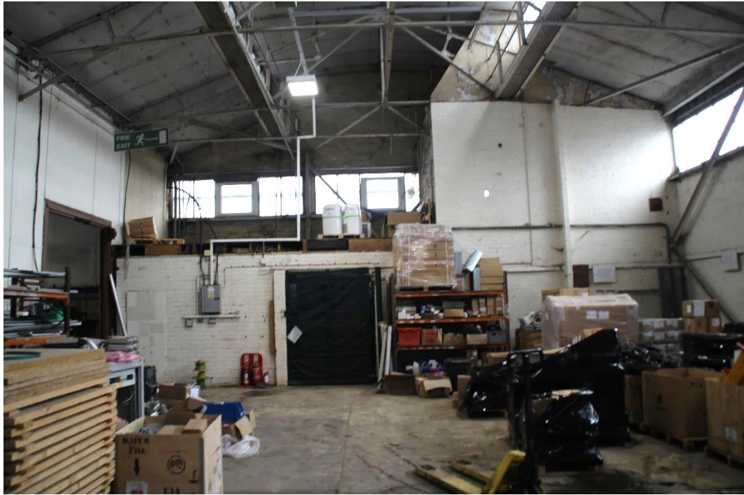
Photo 28 View looking south towards the internal brick structure
