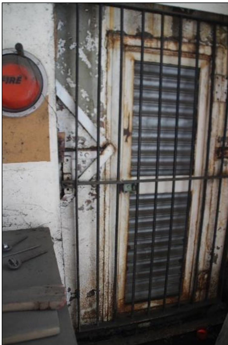
Photo 44 Internal view of barred wicket door in store block 3
