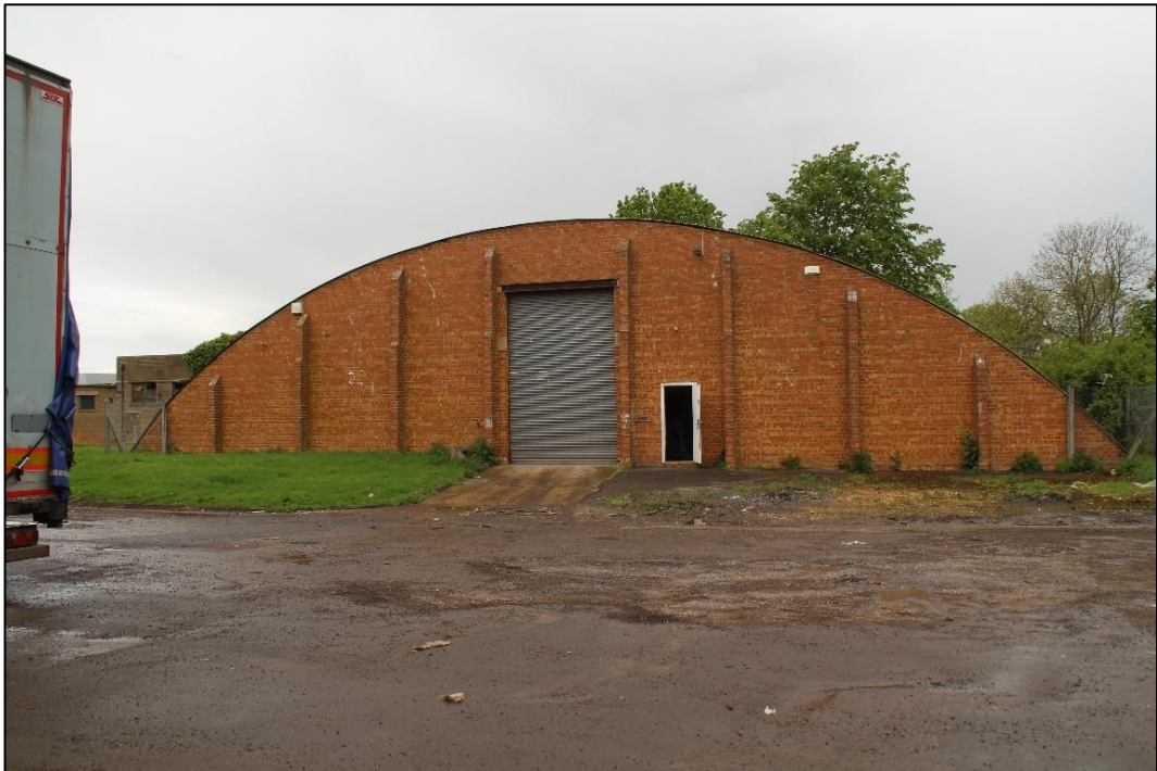
Photo 45 View of the front (eastern) elevation of the blister hangar
