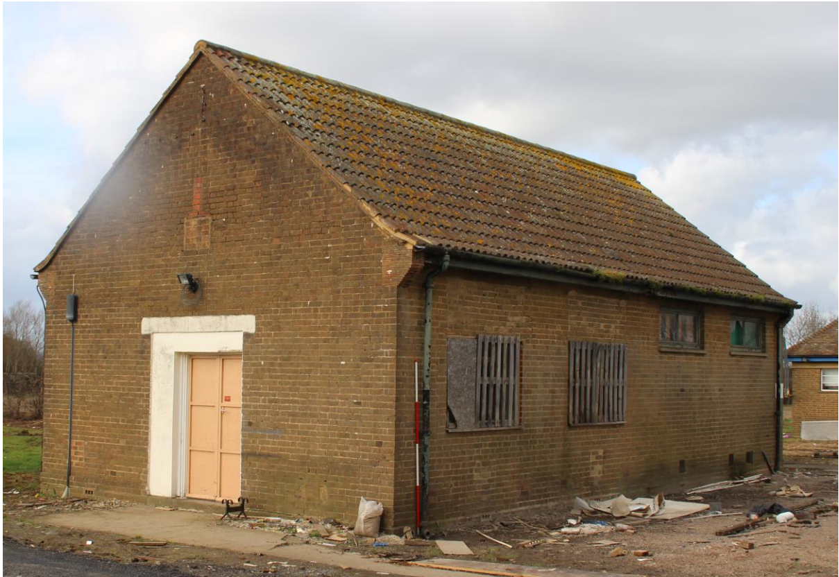
Figure 20 Building 2 looking north-west (scale 2m)
