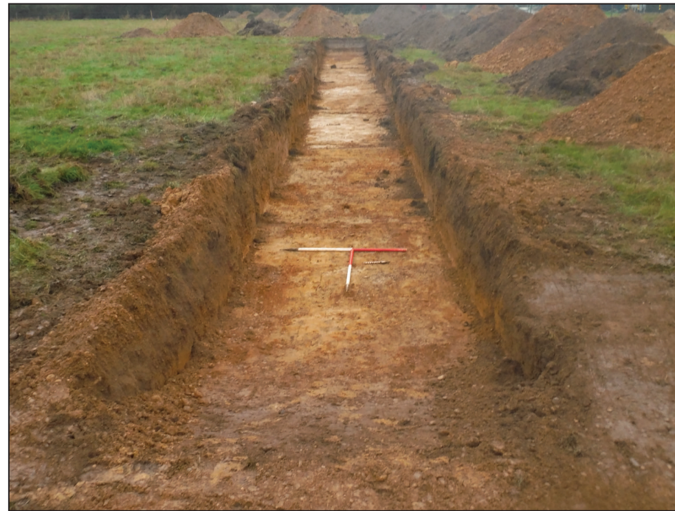
Trench 4, looking south-west (1m scales)
