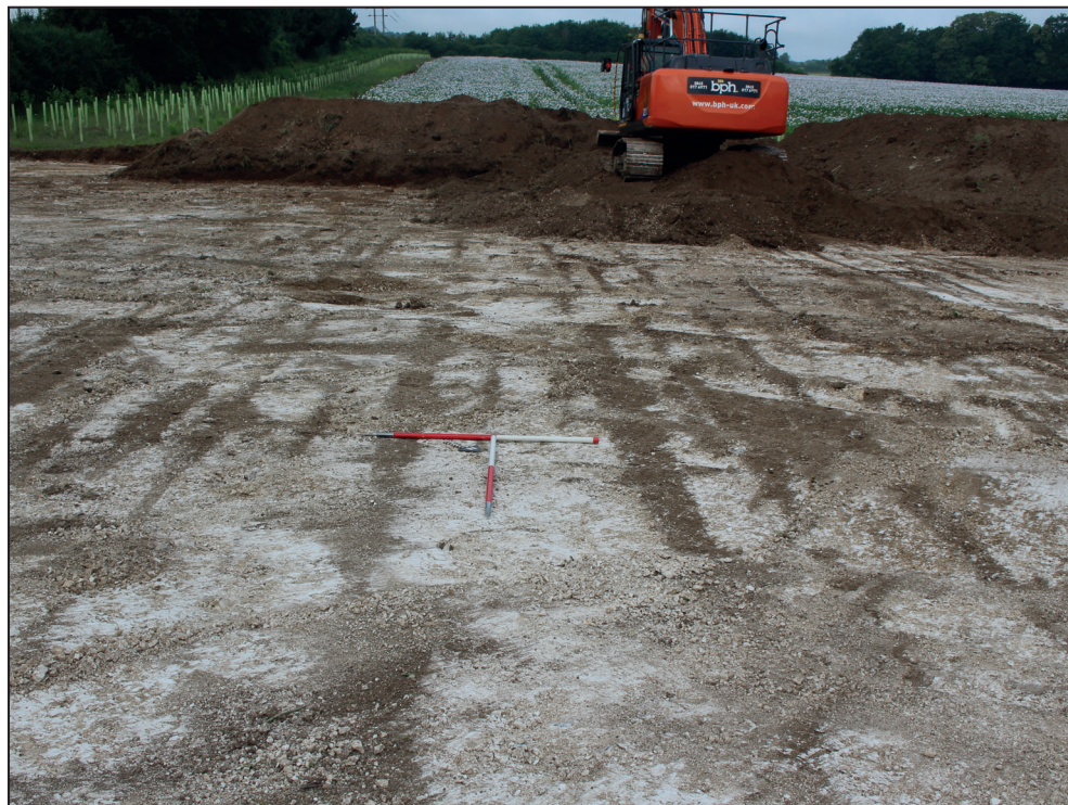
Working shot, looking south-west (scales 1m)
