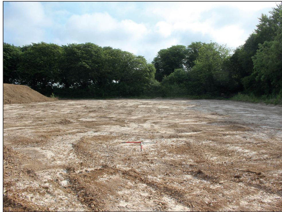
Working shot, looking north-east (scales 1m)
