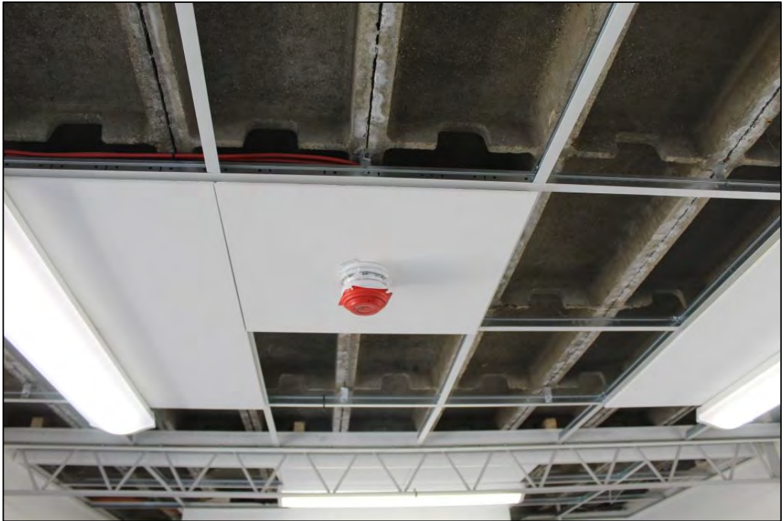
Photo 53: Acoustic grid system, partially installed in Room 16
