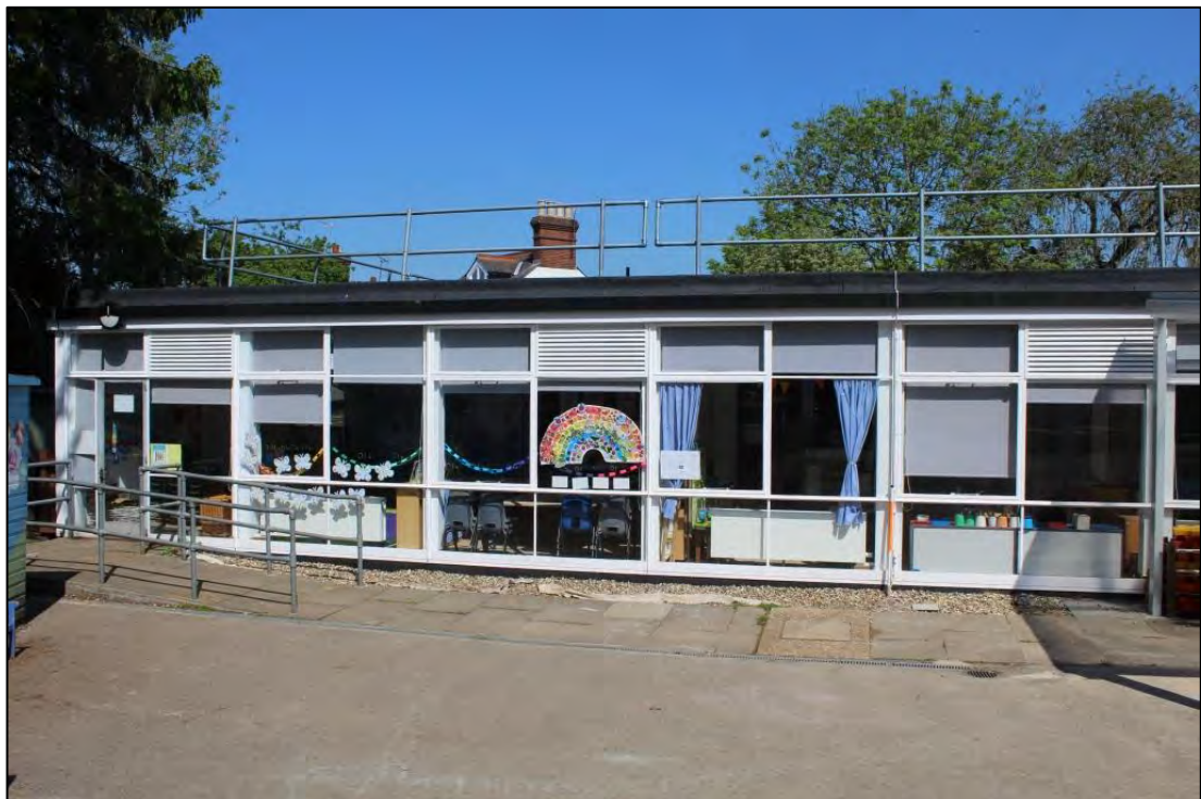
Photo 59: Louvred panels within southern elevation of nursery block
