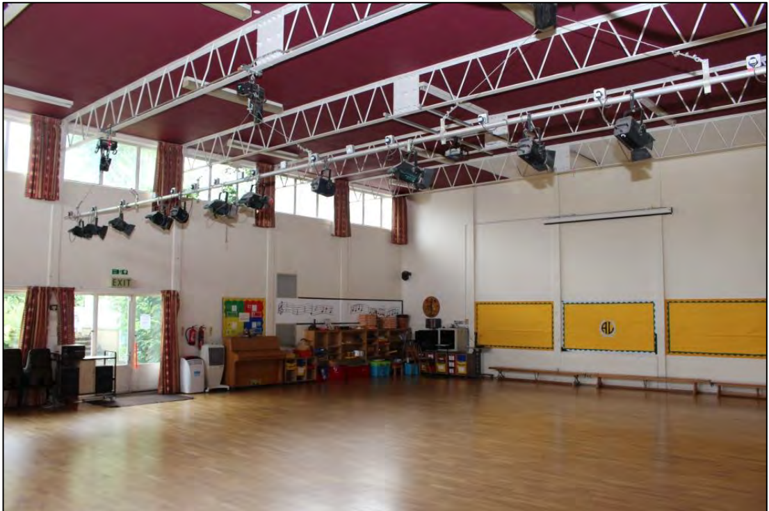
Photo 26: Overview of Room 8, looking south-eastwards
