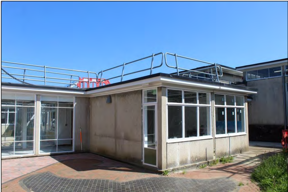
Photo 60: Fold-down roof rail system in 'up' position
