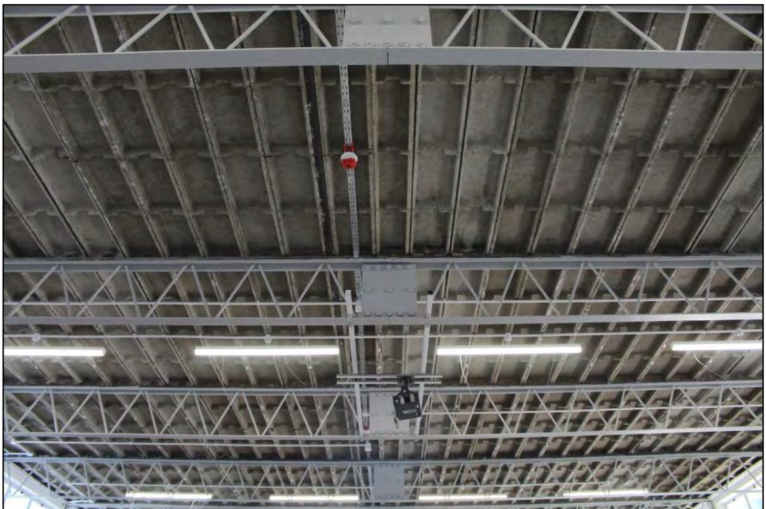
Photo 54: Exposed concrete roof structure in Room 8
