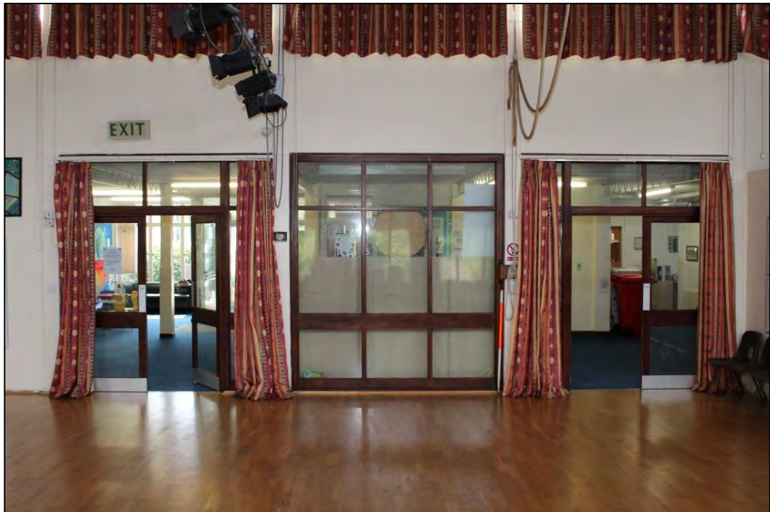
Photo 27: Overview of timber screen and double doors to western extent of Room 8
