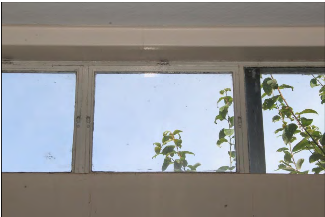
Photo 30: Detail of clerestory window in Room 13
