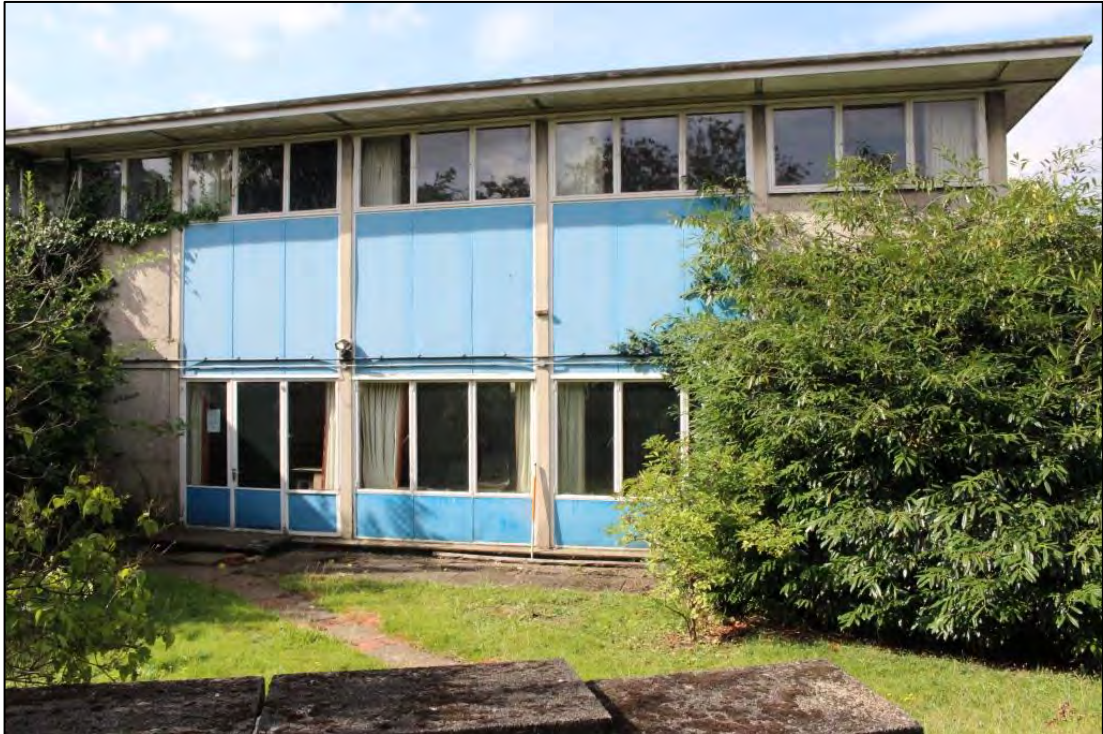
Photo 6: Overview of the eastern elevation of the main hall (Room 8)
