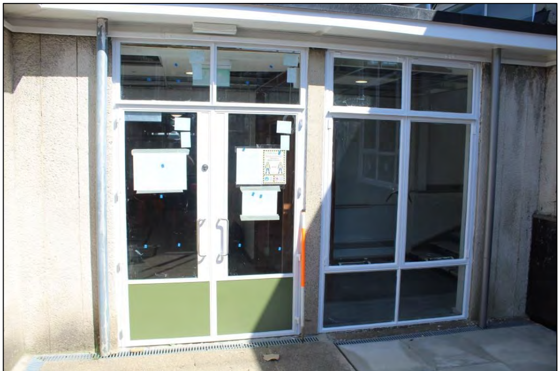
Photo 51: Steel replacement door at southern extent of Room 1
