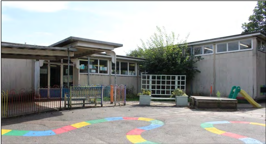
Photo 11: Overview of southern extent of Western elevation
