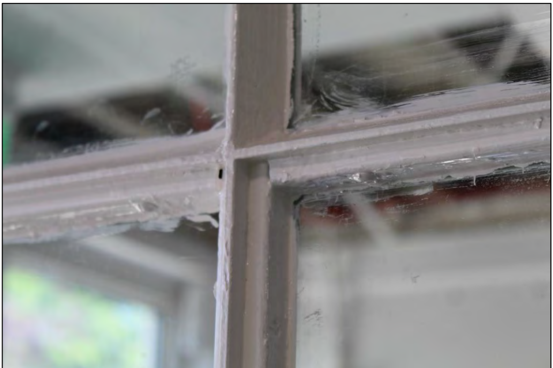
Photo 47: Replacement glazing and putty in internal windows, Room 1
