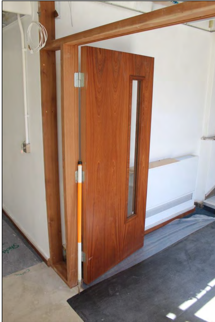
Photo 49: Internal door between Rooms 1 and 15
