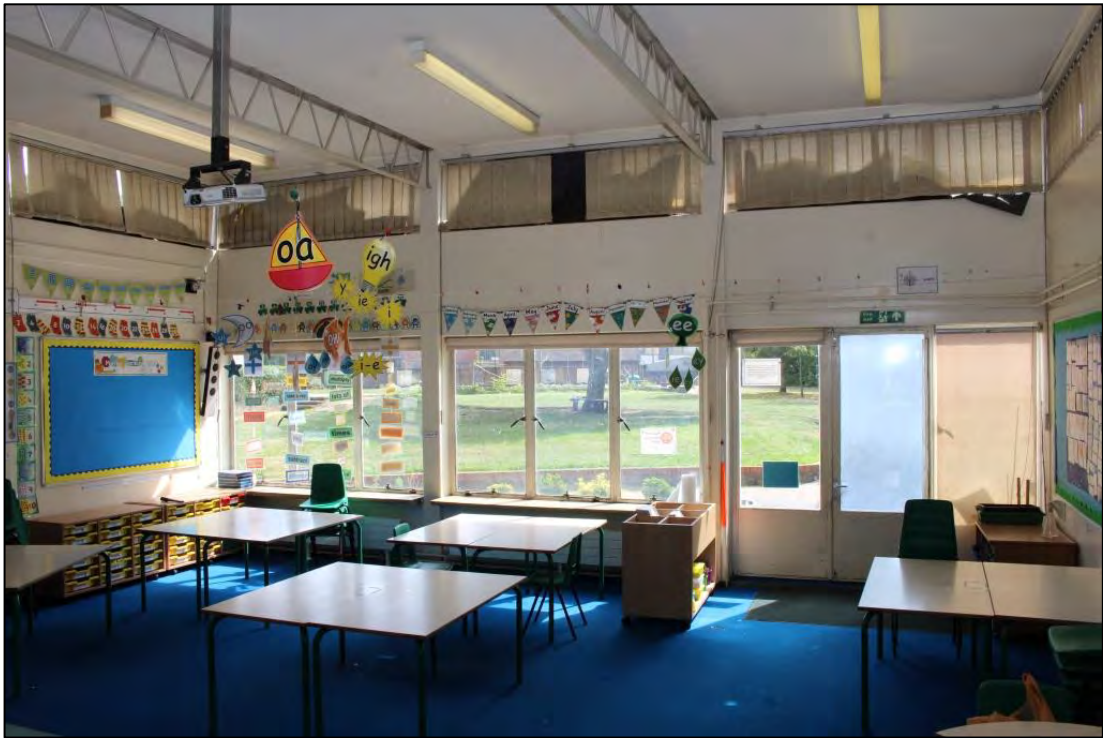
Photo 29: Overview of Room 11, looking southwards
