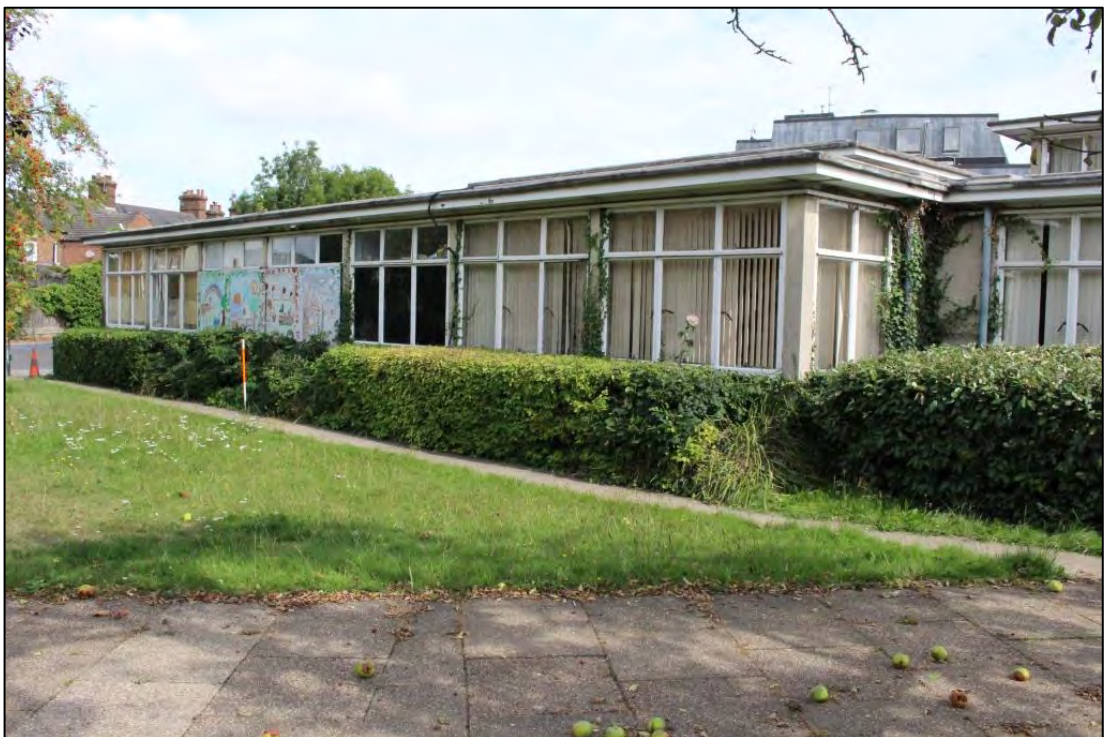
Photo 2: Overview of the northern extent of the western elevation
