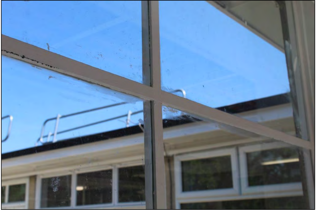
Photo 48: Replacement glazing in Room 10
