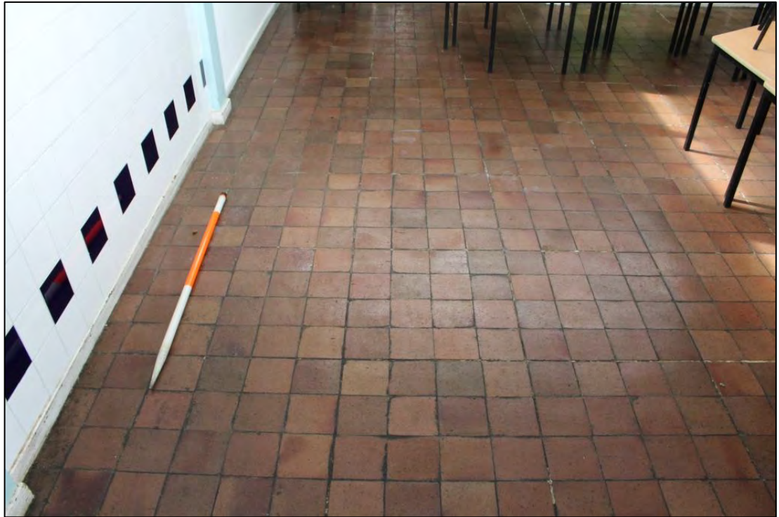
Photo 24: Quarry tiles in Room 6
