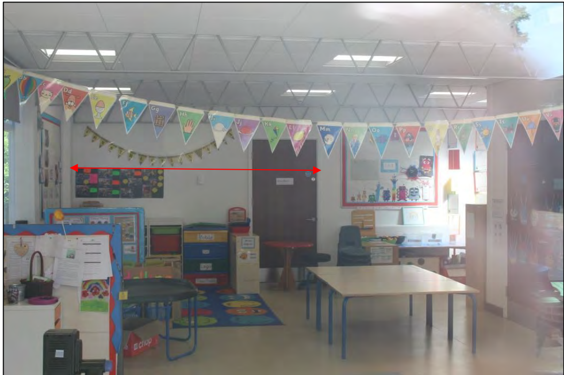
Photo 43: Extent of new server room (indicated by red arrows)
