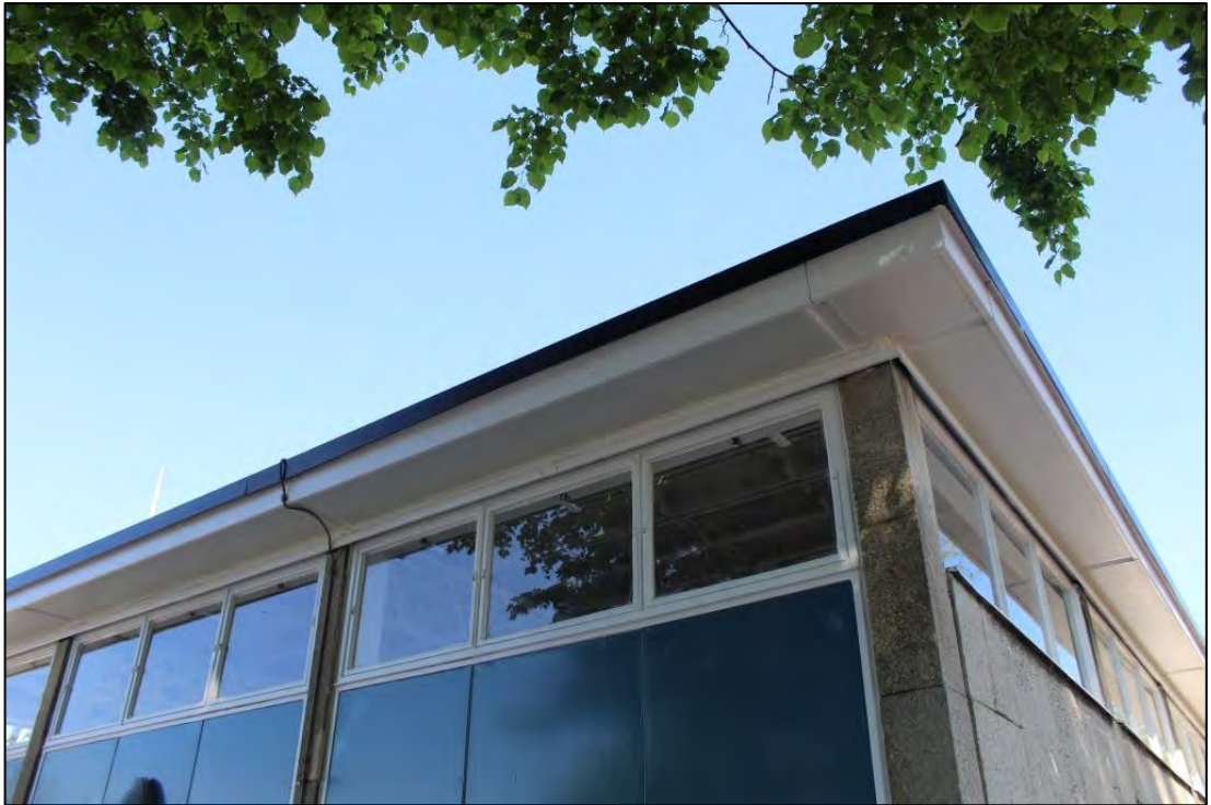
Photo 62: Detail of replacement soffits
