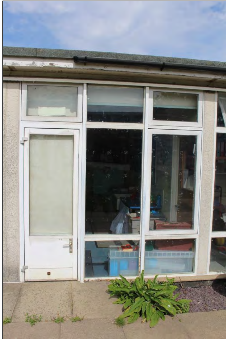
Photo 33: Detail of external door to Room 19
