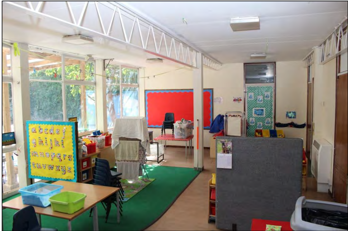
Photo 38: Overview of Room 21, looking south-westwards. Note the free standing post between roof trusses
