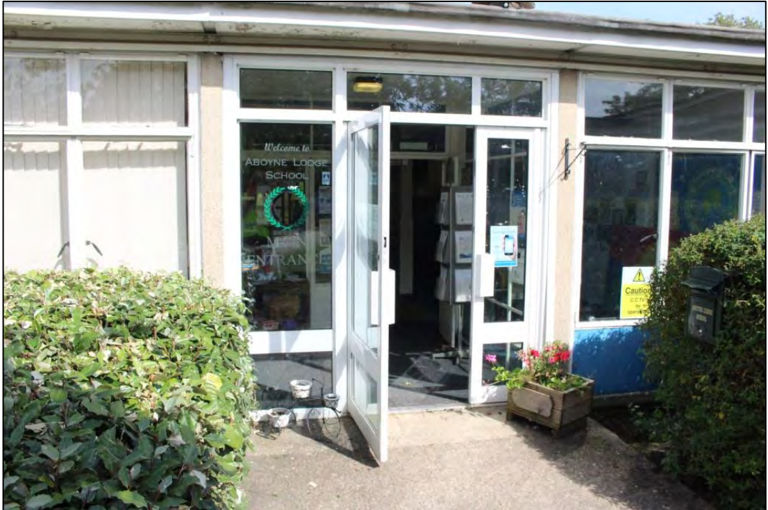
Photo 1: uPVC main entrance door
