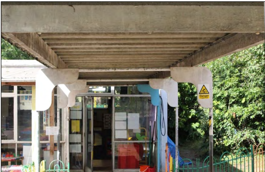
Photo 12: Covered walkway linking Phases 1 and 2, looking northwards towards Room 21
