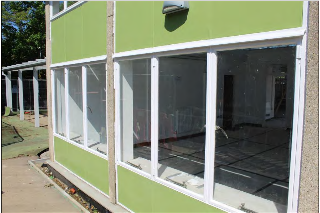
Photo 46: New safety glass in windows at south-western corner extent of Room 14
