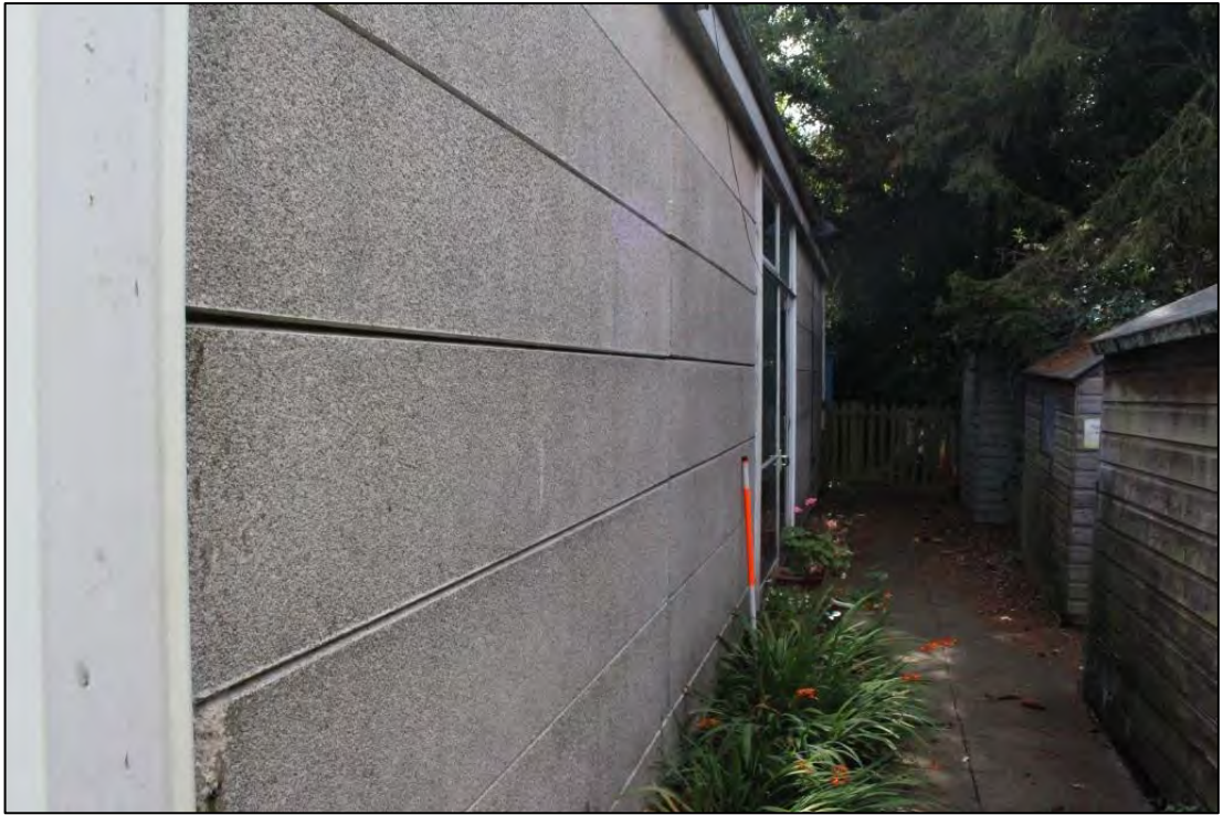
Photo 37: Overview of concrete cladding to eastern elevation of Room 23
