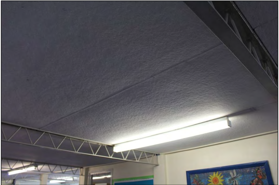
Photo 14: Detail of ceiling boards between lattice roof trusses
