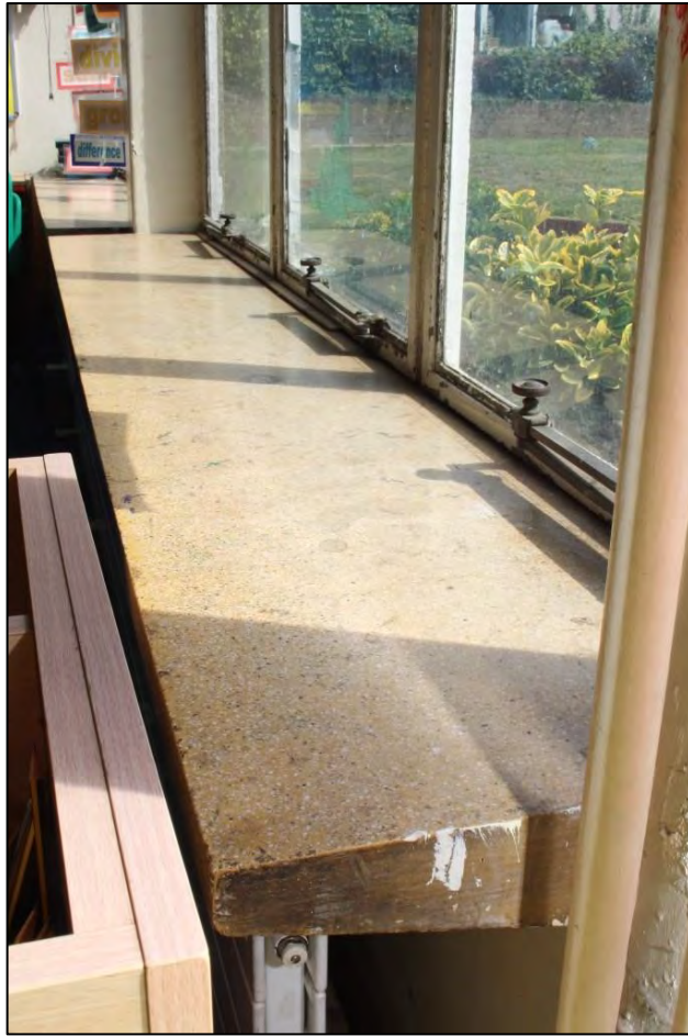
Photo 31: Detail of window shelf in Room 11
