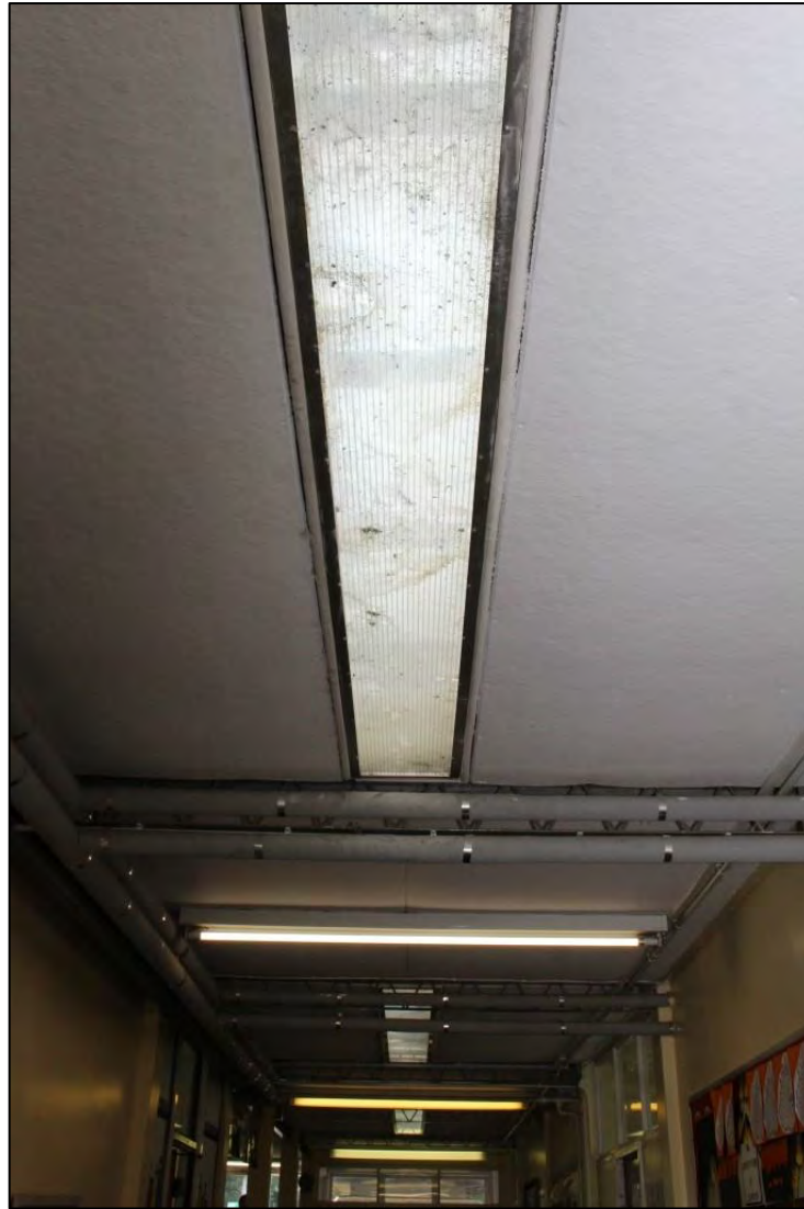
Photo 28: Detail of roof lights within Room 10
