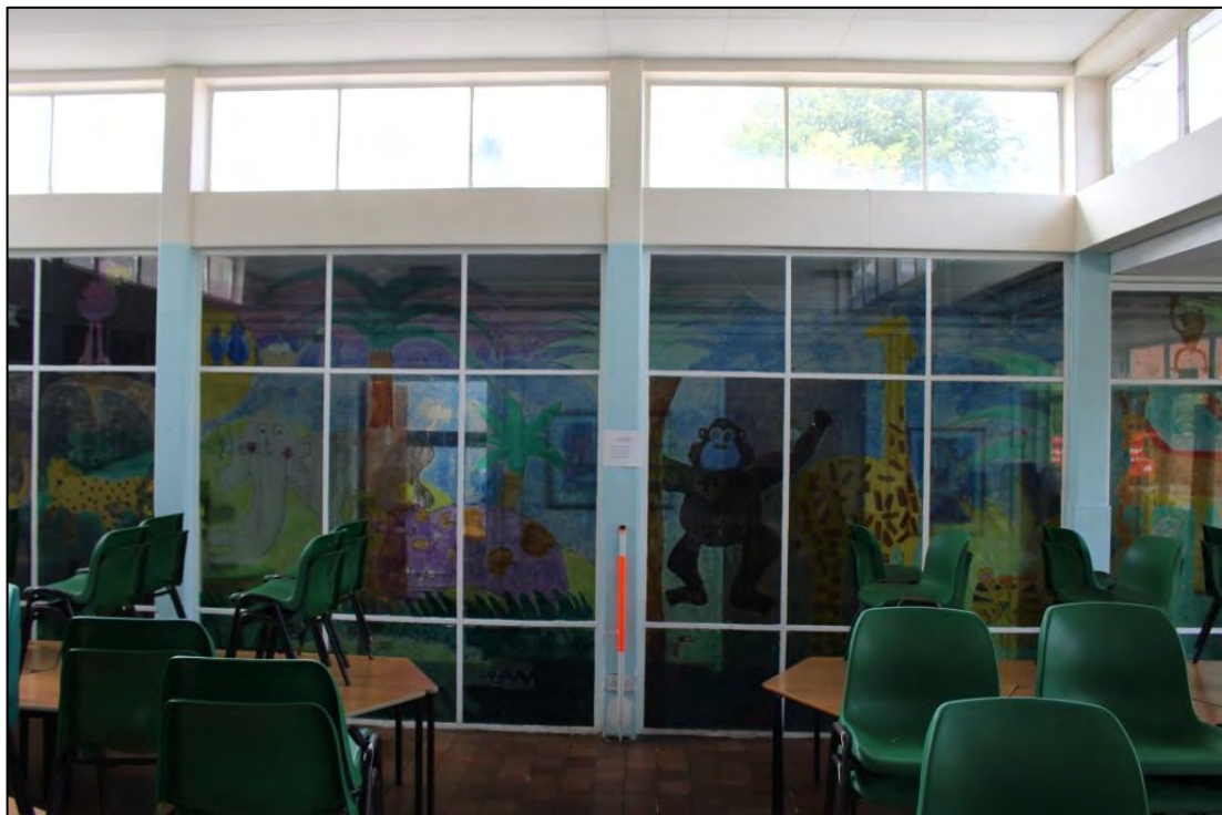
Photo 23: Glazed screen to western extent of Room 6
