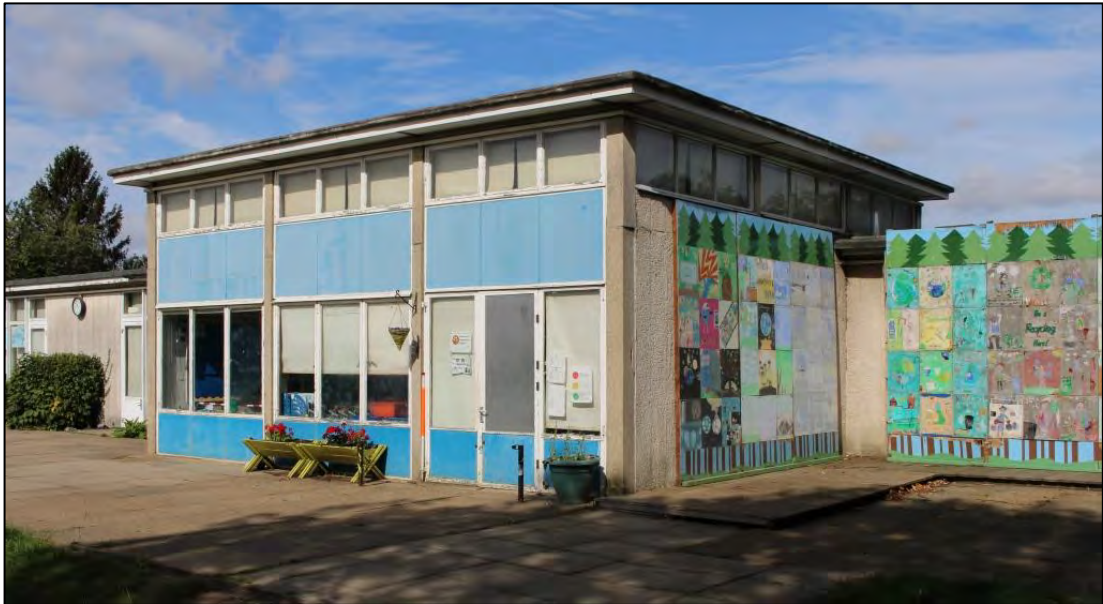
Photo 8: Overview of southern elevation of Room 18
