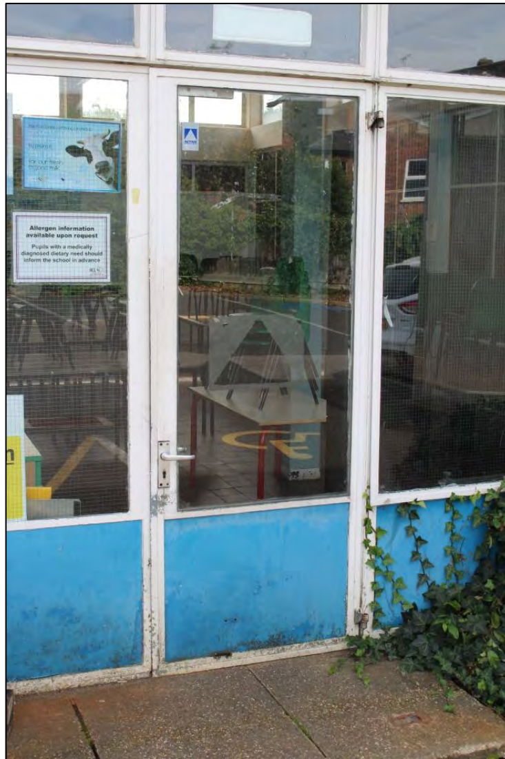
Photo 5: Door to dining hall within northern elevation
