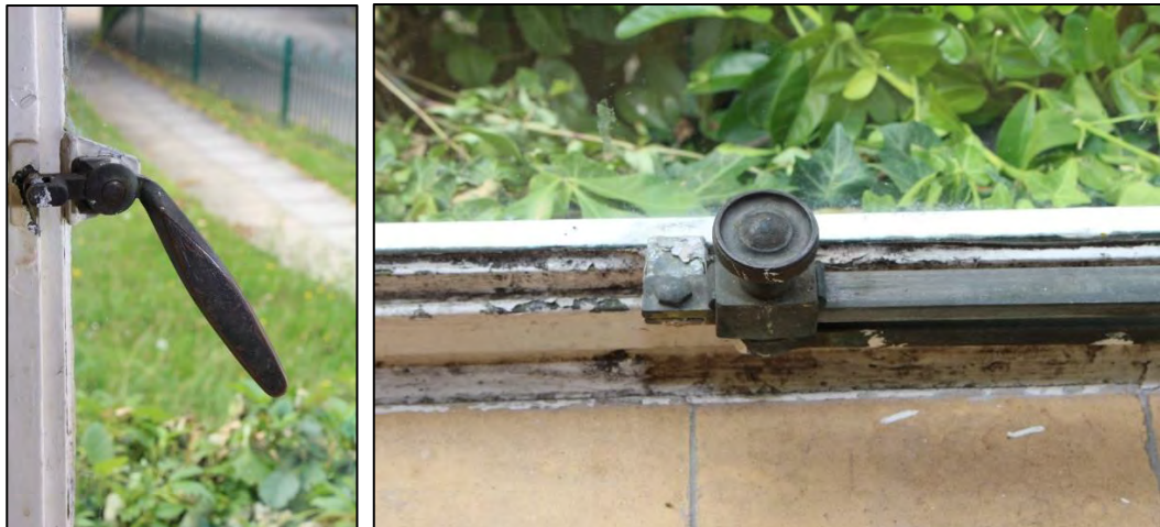
Photos 20 and 21: Detail of window fixtures in Room 5
