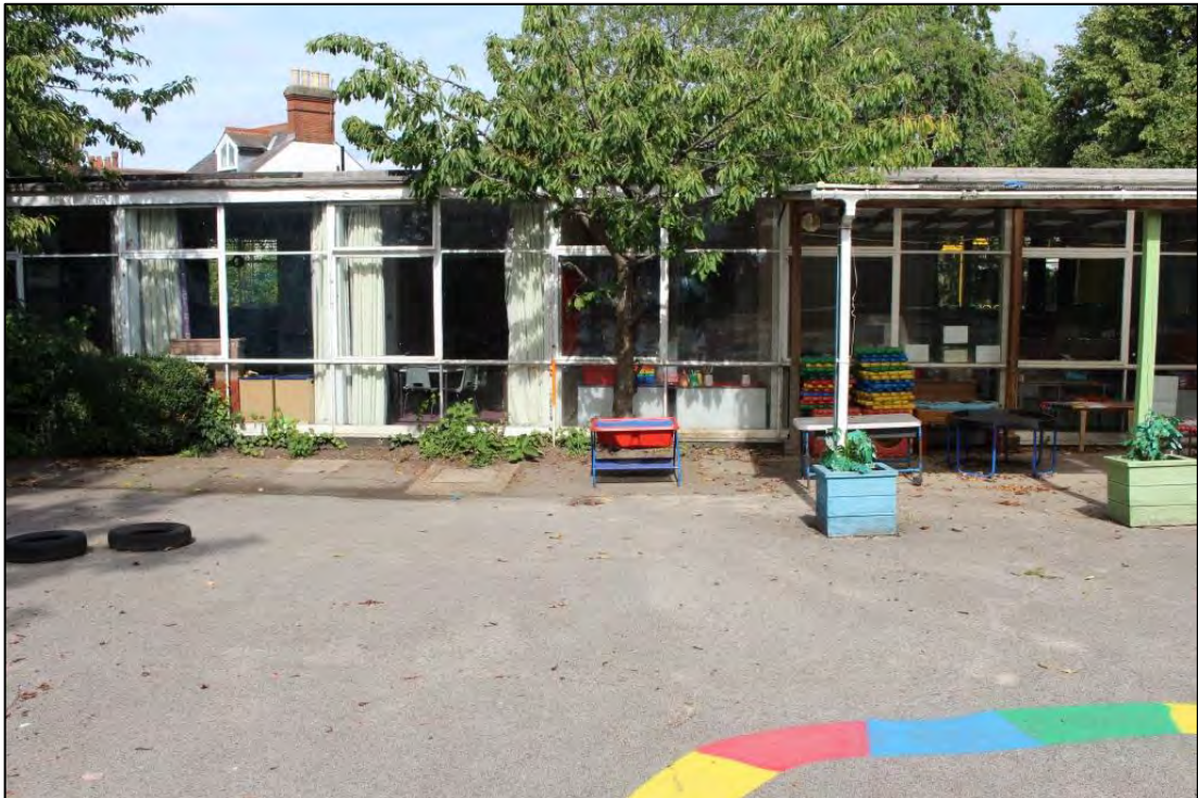
Photo 36: Overview of southern elevation of Rooms 21 and 23
