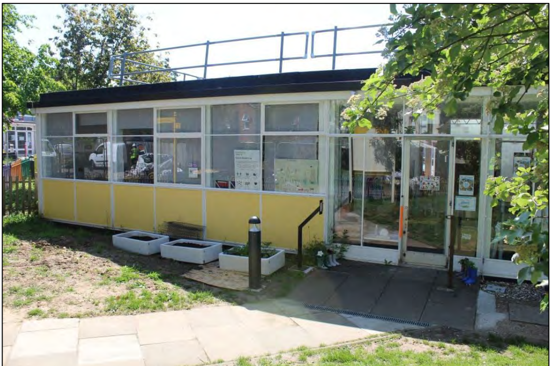
Photo 63: Nursery block, northern elevation
