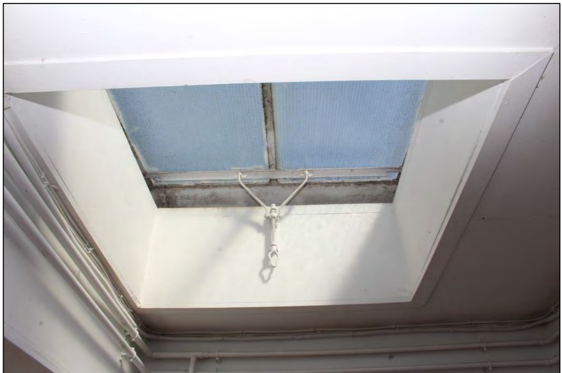
Photo 40: Detail of typical rooflight within the nursery block
