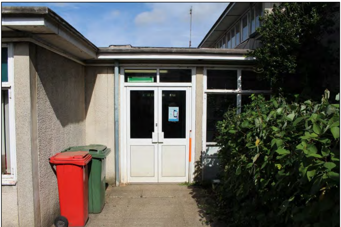
Photo 10: uPVC door within southern elevation
