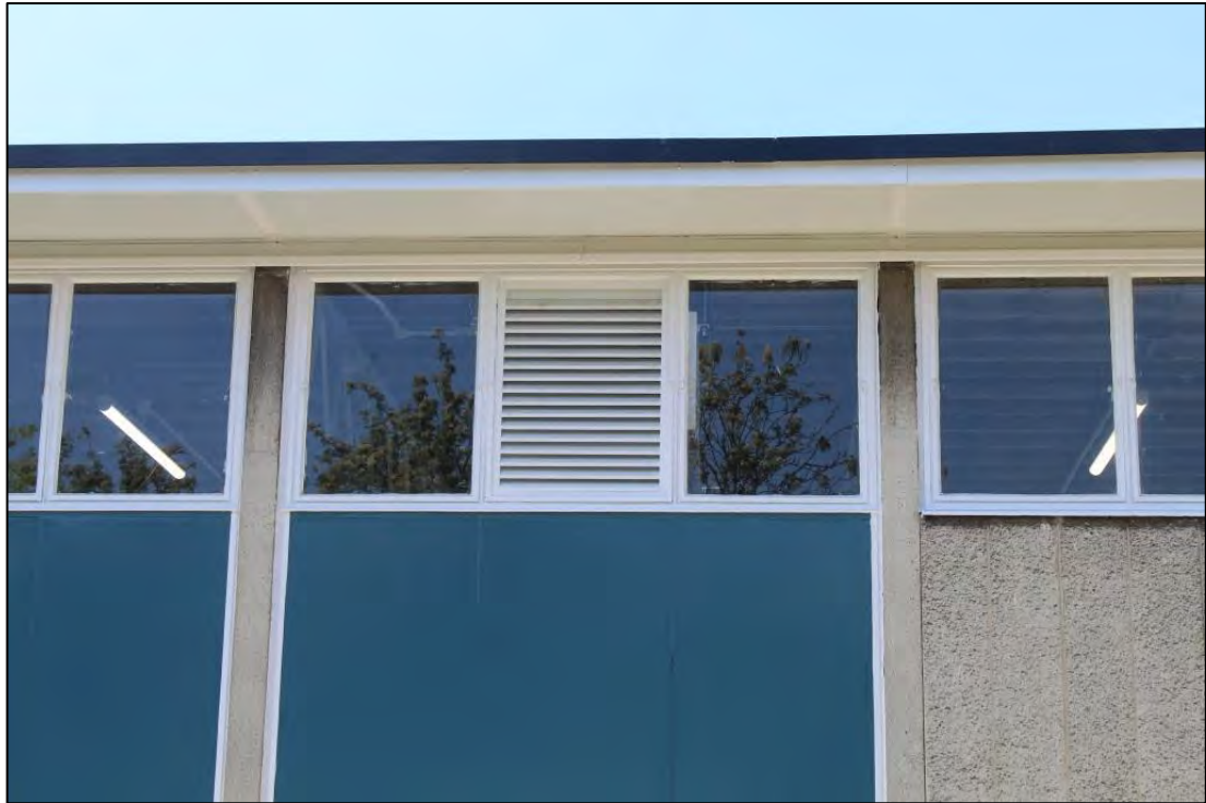
Photo 58: Louvred ventilation panel, Room 8, eastern elevation
