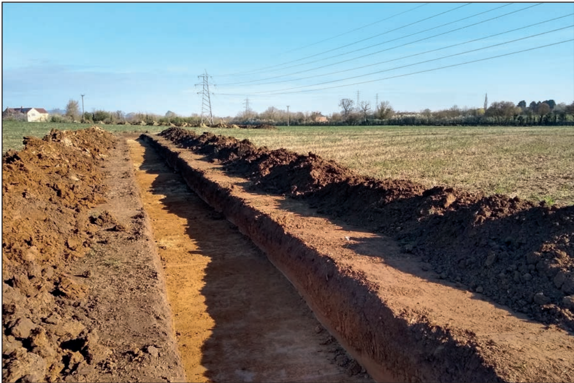
Field 9, looking north-west
