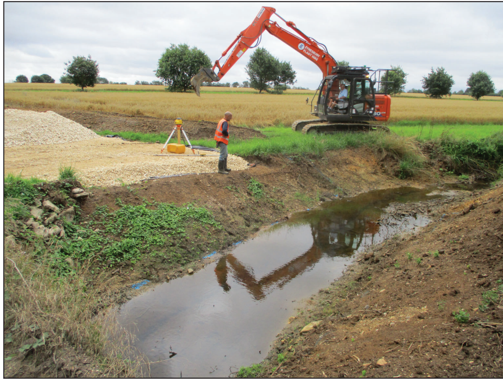
Culvert ditch pre-excavation, looking north-east
