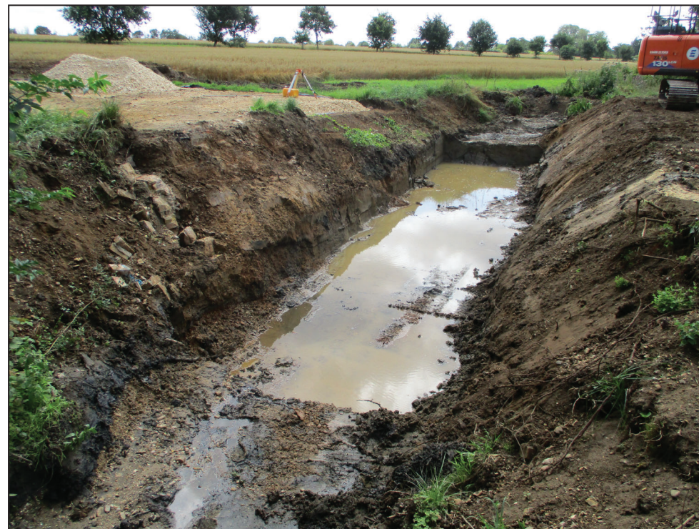
Culvert 2 post-excavation, looking south
