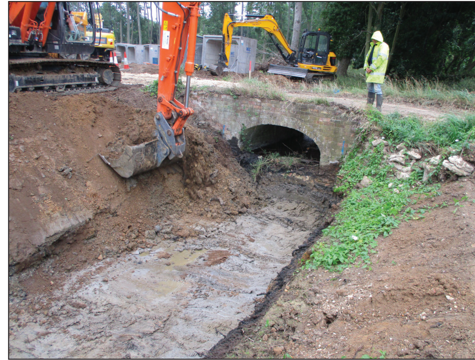
Culvert 2 under excavation, showing existing 20th century bridge
