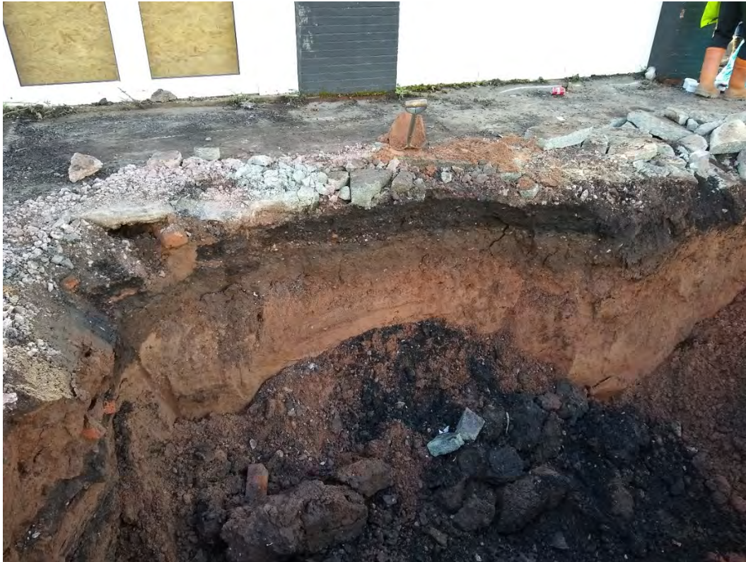
Fig. 9. Forecourt area following removal of petrol tanks, looking south
