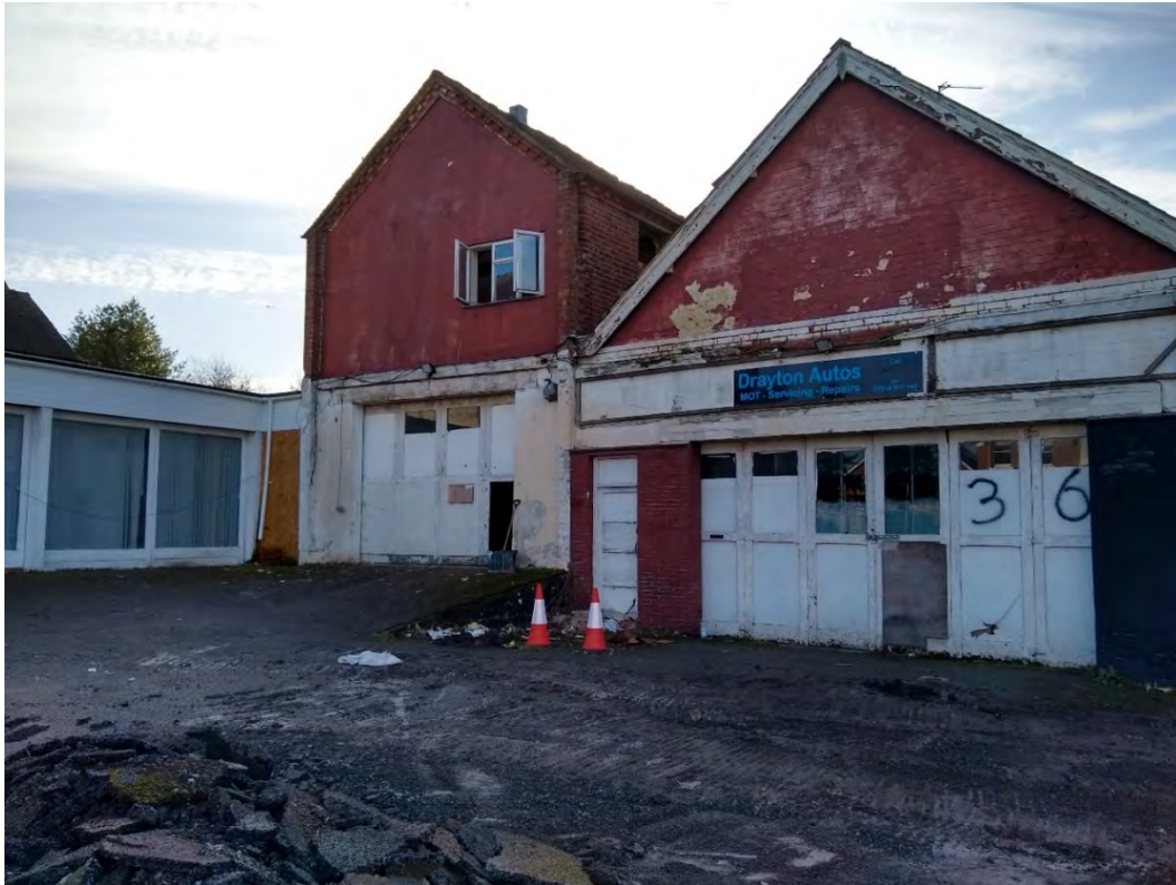
Fig. 3. No.36 and forecourt area, looking southeast
