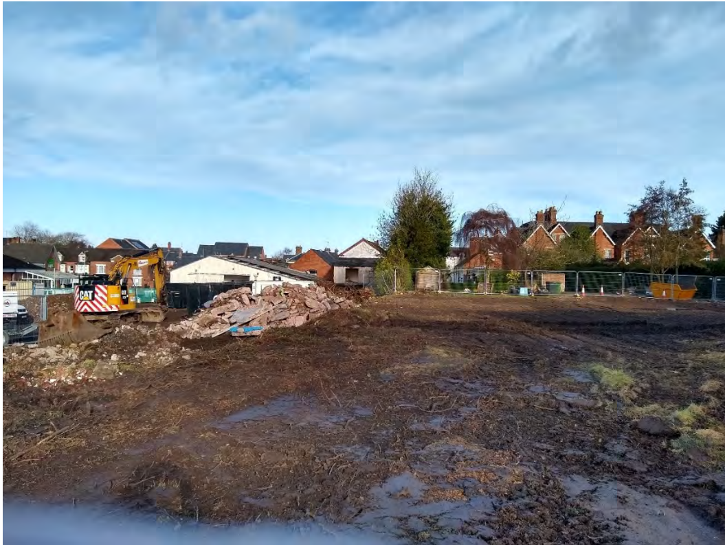
Fig. 5. Site looking north toward Stafford Road
