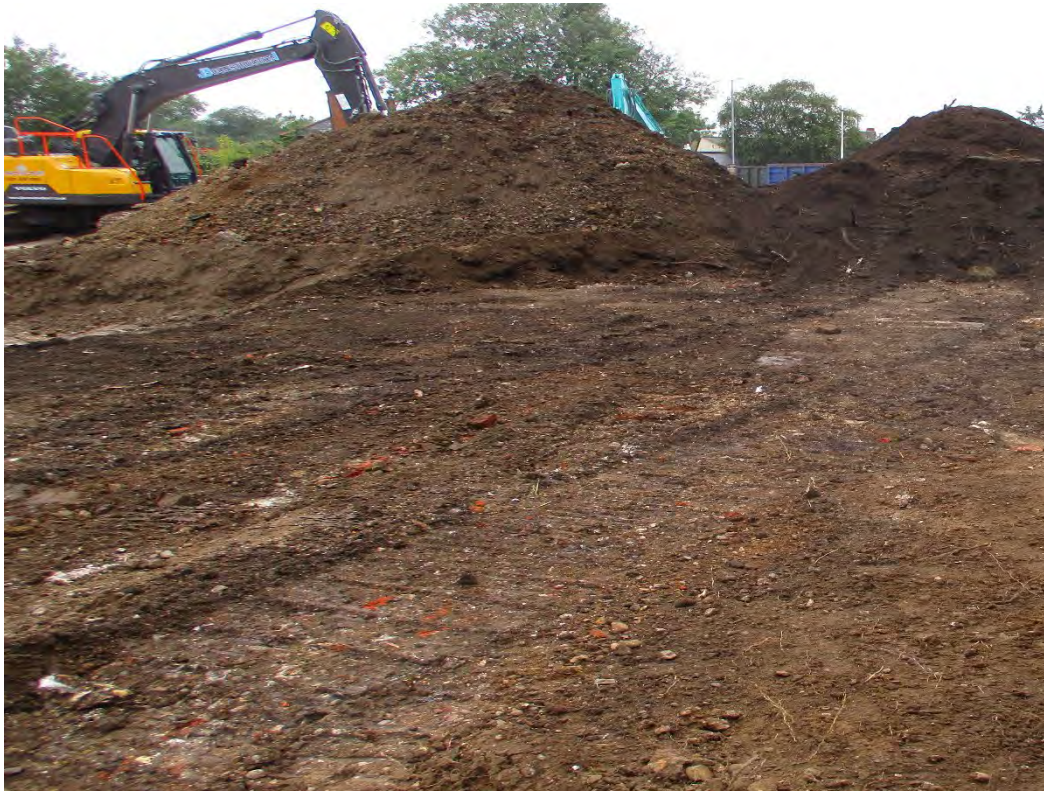
Fig. 12. Vegetation and topsoil strip for piling mat
