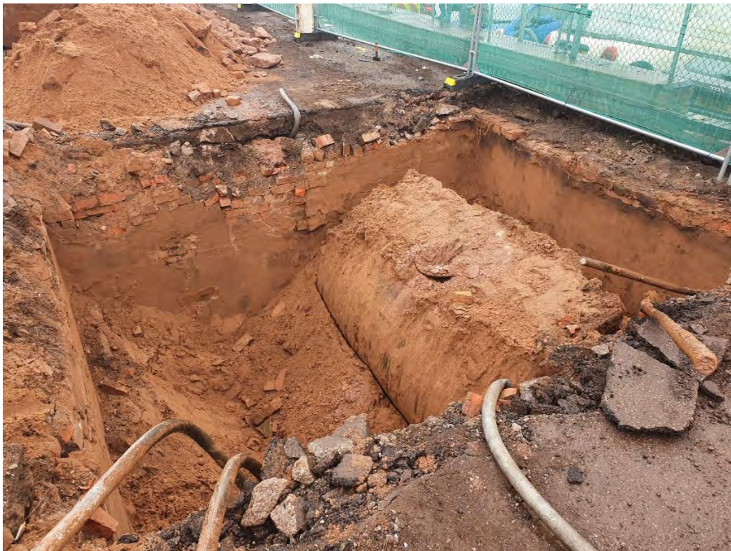
Fig. 10. Petrol tanks to west side of garage under removal
