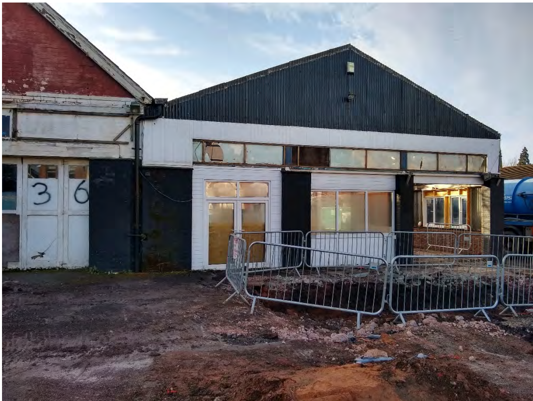
Fig. 4. Garage and forecourt area looking southwest
