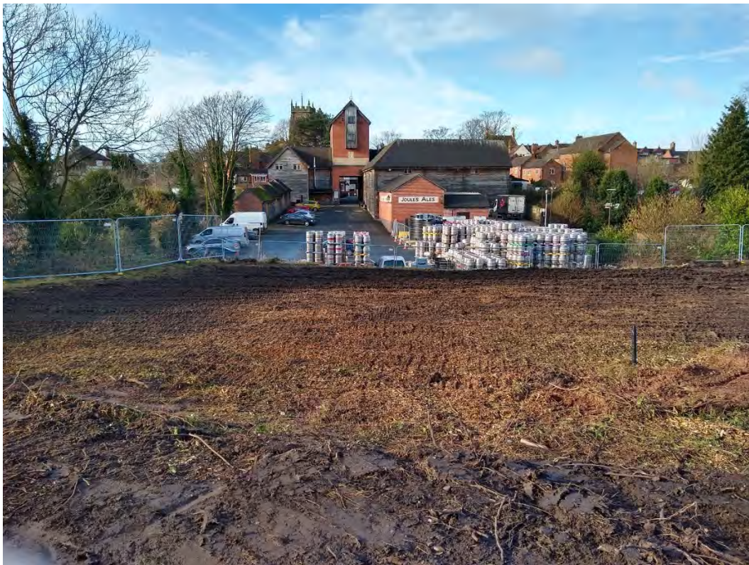
Fig. 8. Evidence of terracing – rear of plot, looking west towards Joules Brewery
