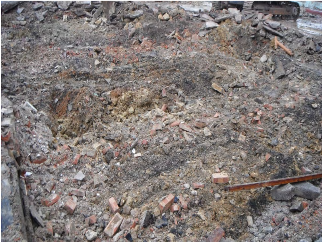
Fig. 11. Garage floor slab and sub-base under removal
