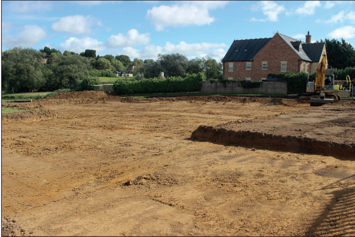
Area 1 during groundworks.
