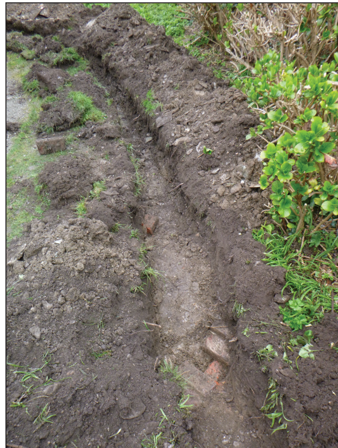
Trench 1 middle portion with wall 104 in the foreground, looking west
