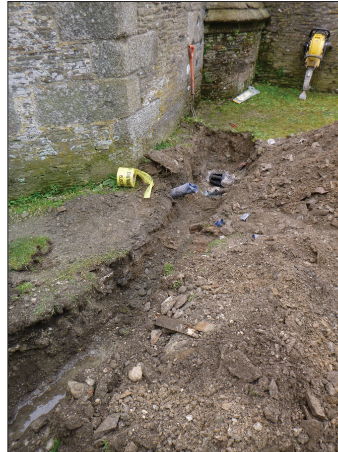
Trench 1 western end, looking south-west
