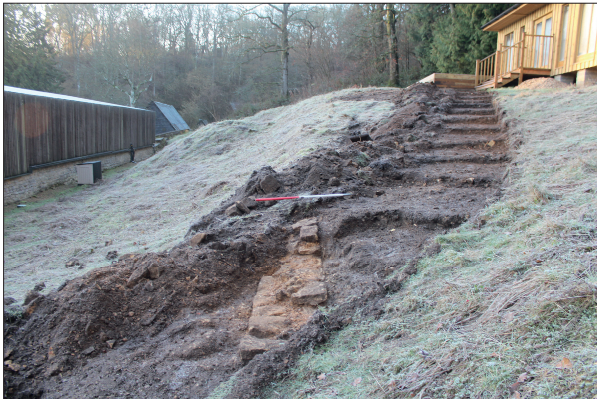
Wall 103, looking south (1m scale)
