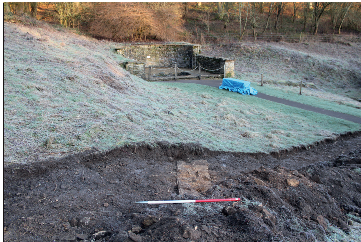
Wall 103, looking north towards Nymphaeum (1m scale)
