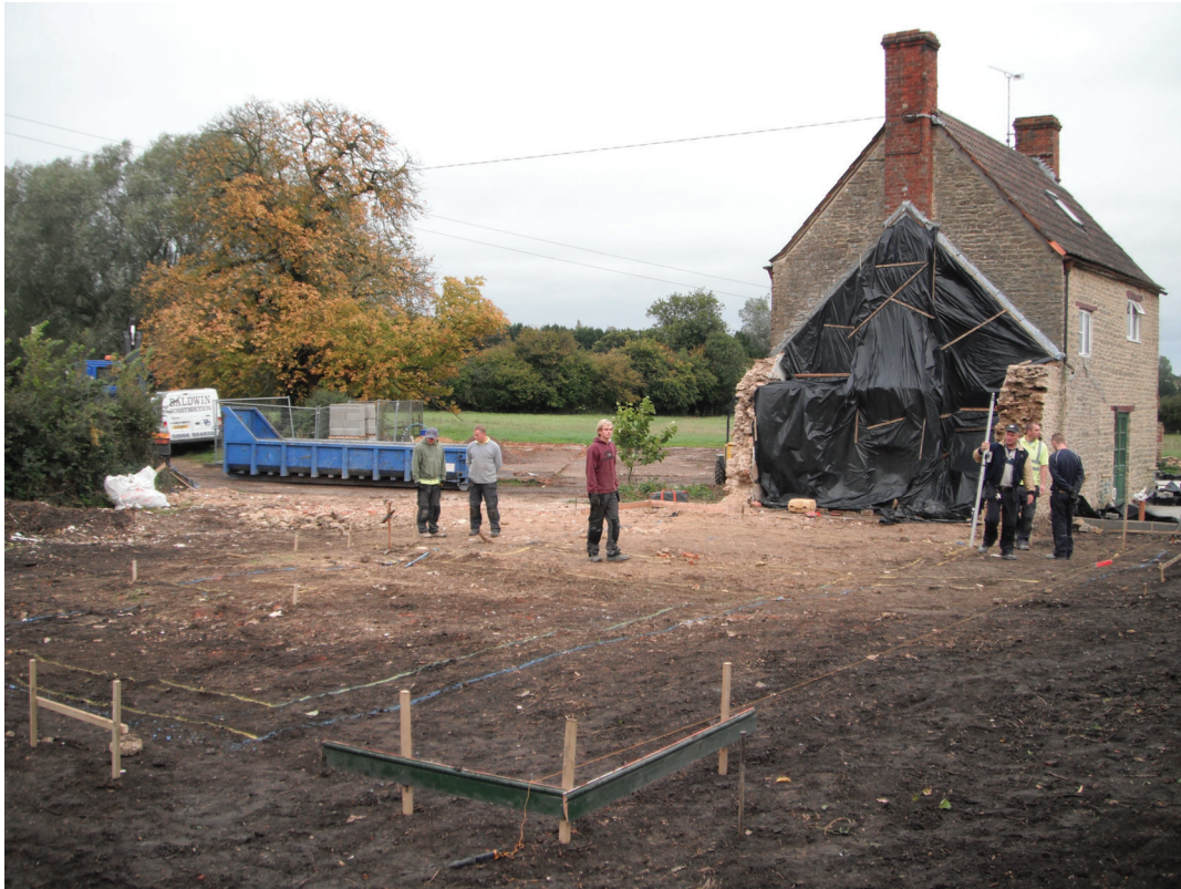
View across site before excavation of foundations
