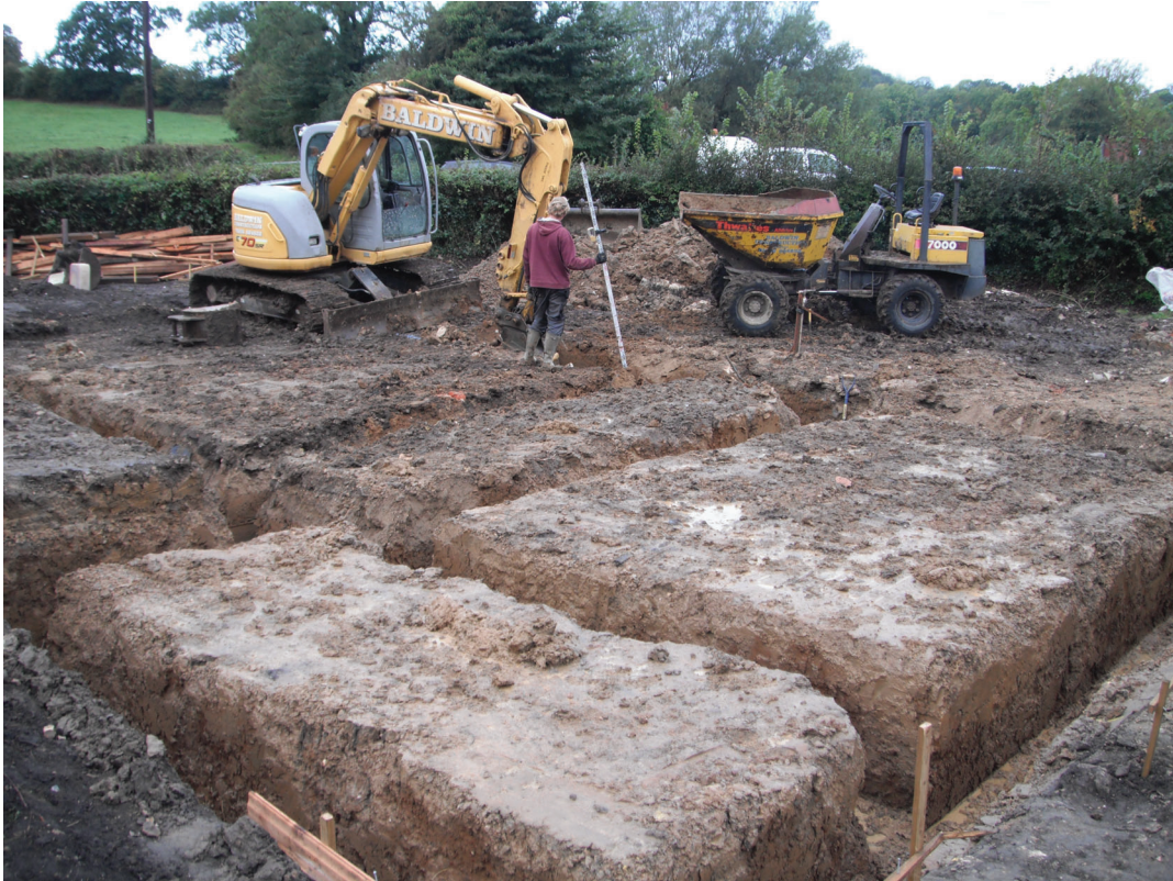
View across site during excavation of foundations
