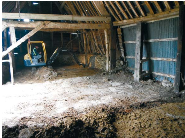
Area 1: ground reduction inside the barn, looking south-east
