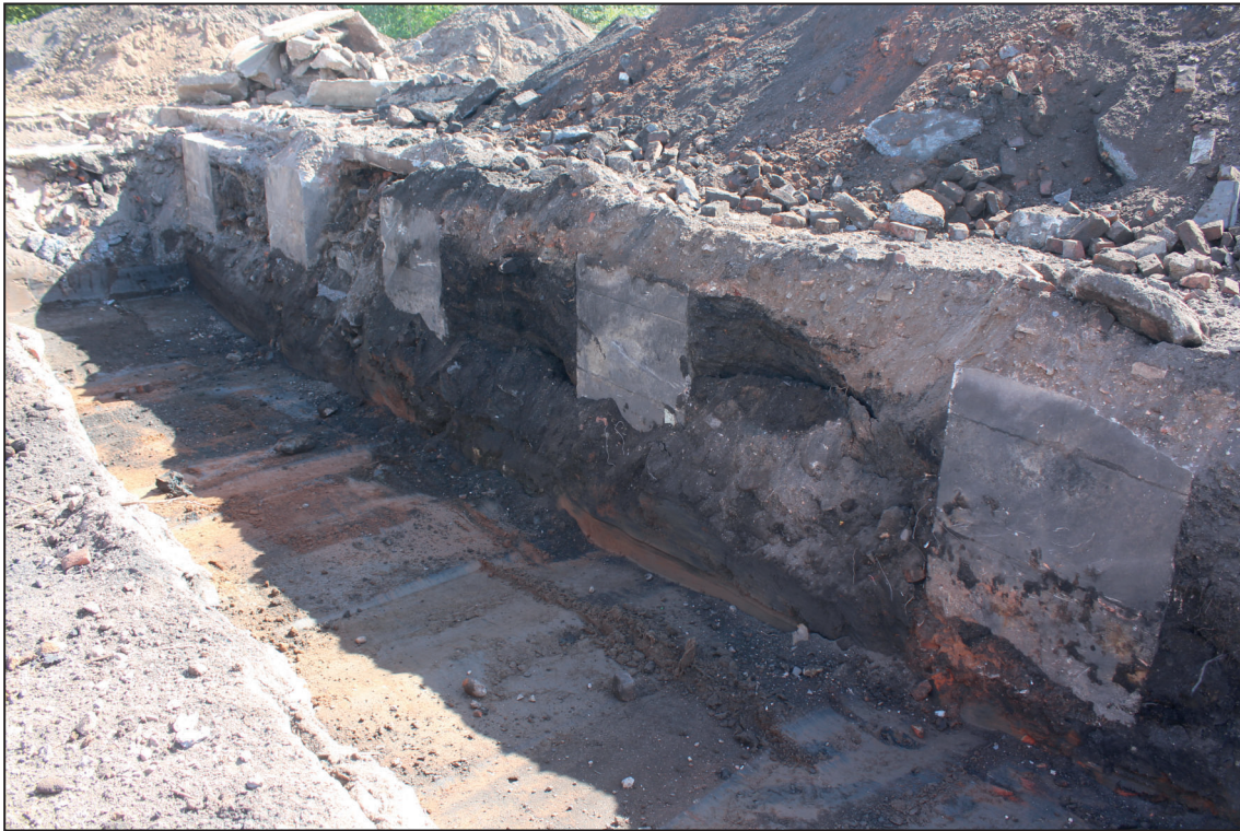
Concrete post-pads in south-eastern extent of Trench 16, looking south-east
