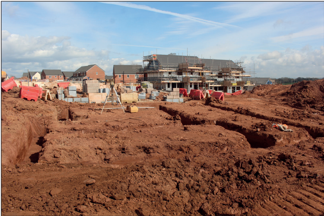
Plot 80, looking north-east
