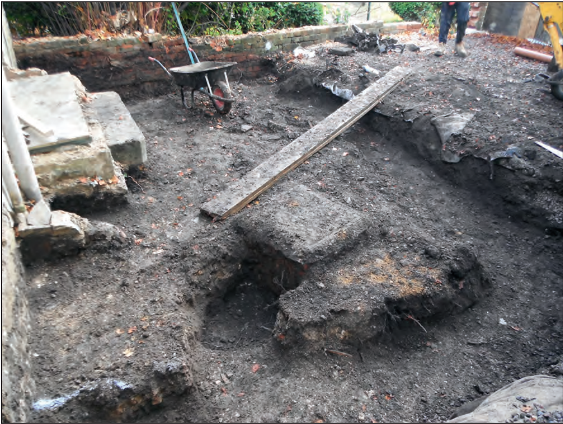
Working shot showing extent of observed groundworks, looking east
