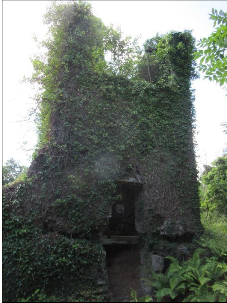
Figure 23.01 – North elevation of Engine House.
