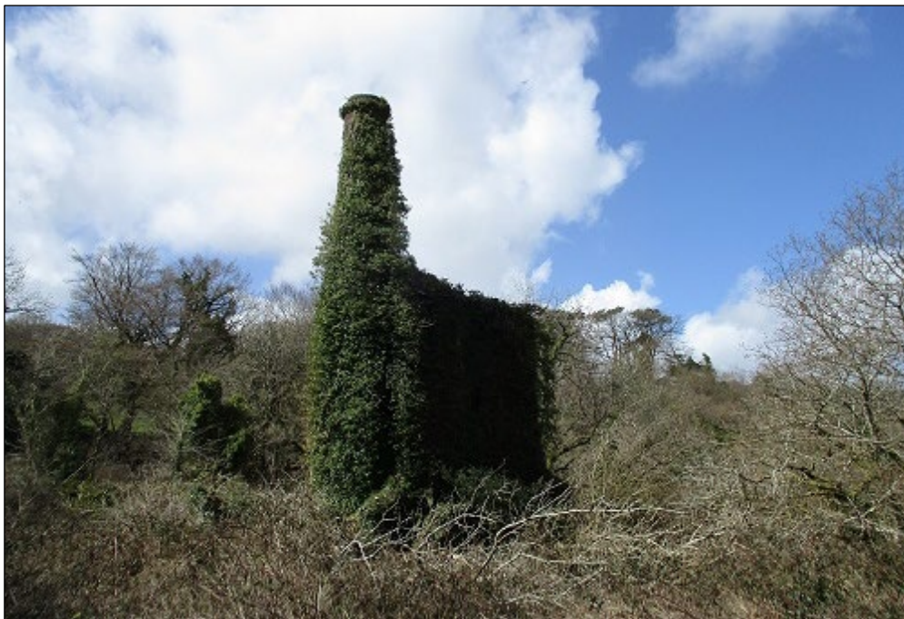
Photograph 1. Holmbush Engine House looking north-west
