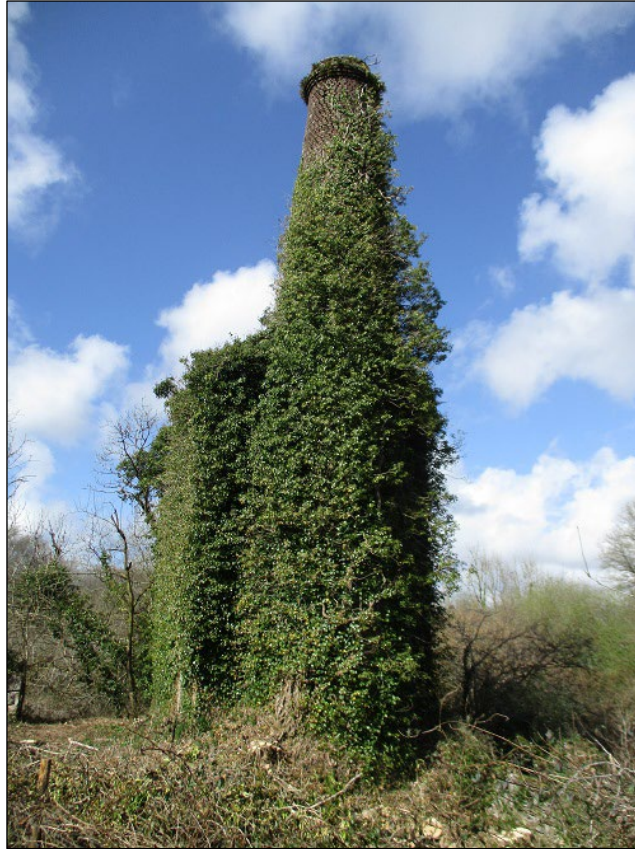
Photograph 19. Boiler House Chimney looking north-east
