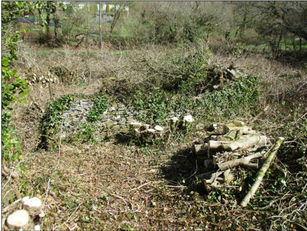
Photograph 16. West wall of Boiler House looking south-east from atop platform
