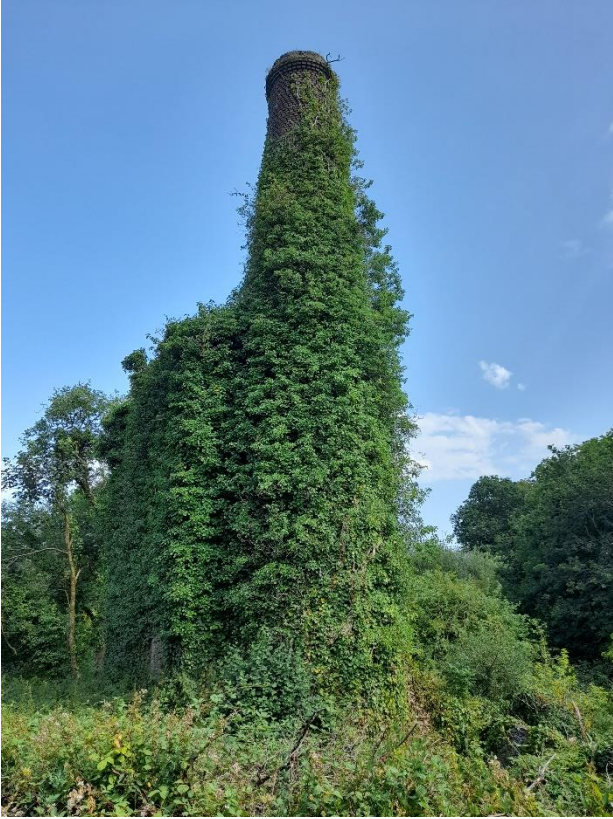
6.The Chimney and Engine House, viewed from the south
