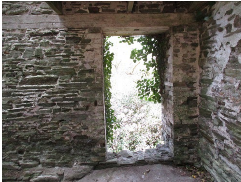
Photograph 6. Door in east wing wall to Boiler House
