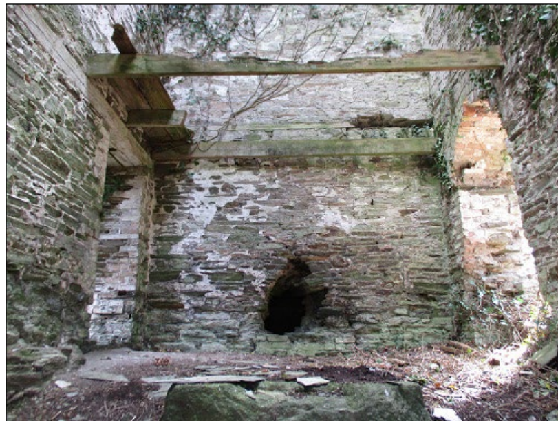
Photograph 8. Gable end wall opening to chimney flue
