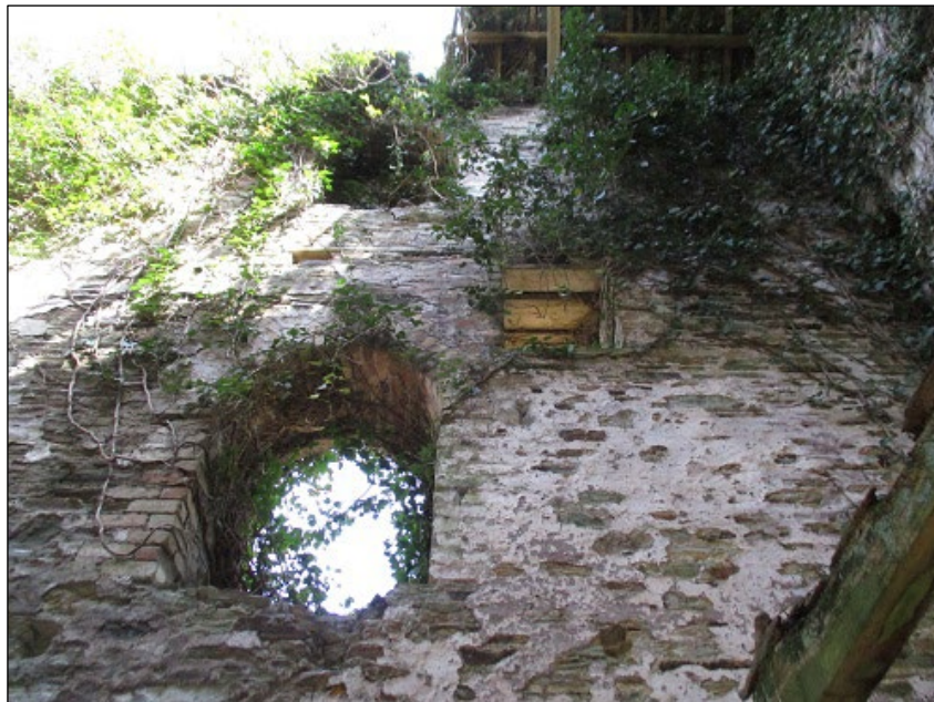
Photograph 7. Internal elevation of west wing wall first and second floors
