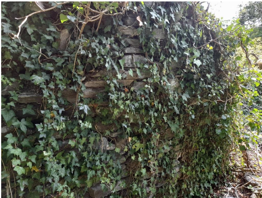
9. Part of the Boiler House wall left in situ
