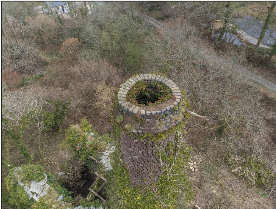
Figure 25.04 – Chimney head and open jointed brickwork.
