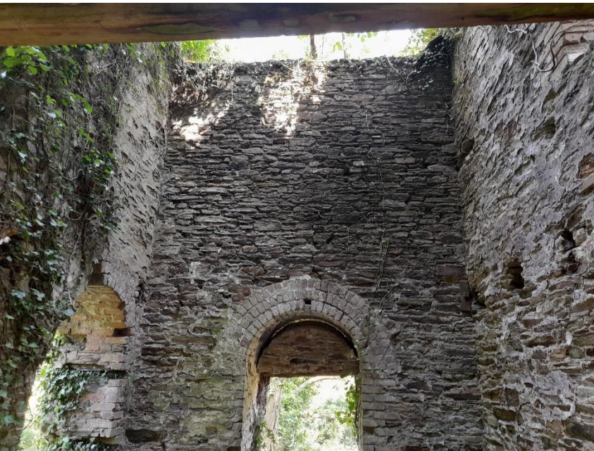
7.The interior of the Engine House
