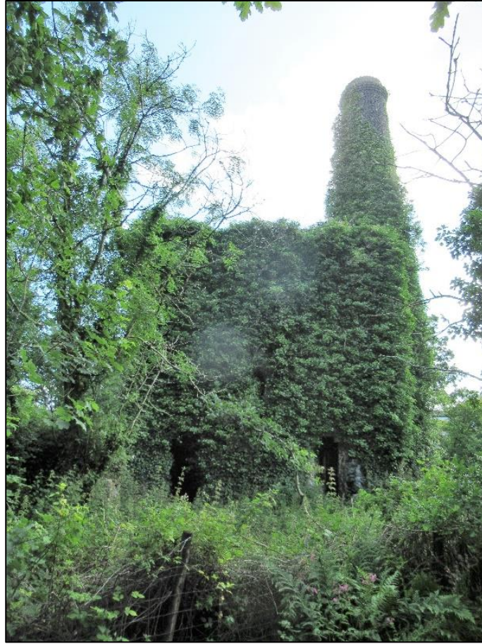
Figure 23.02 – West elevation showing two lower-level openings
