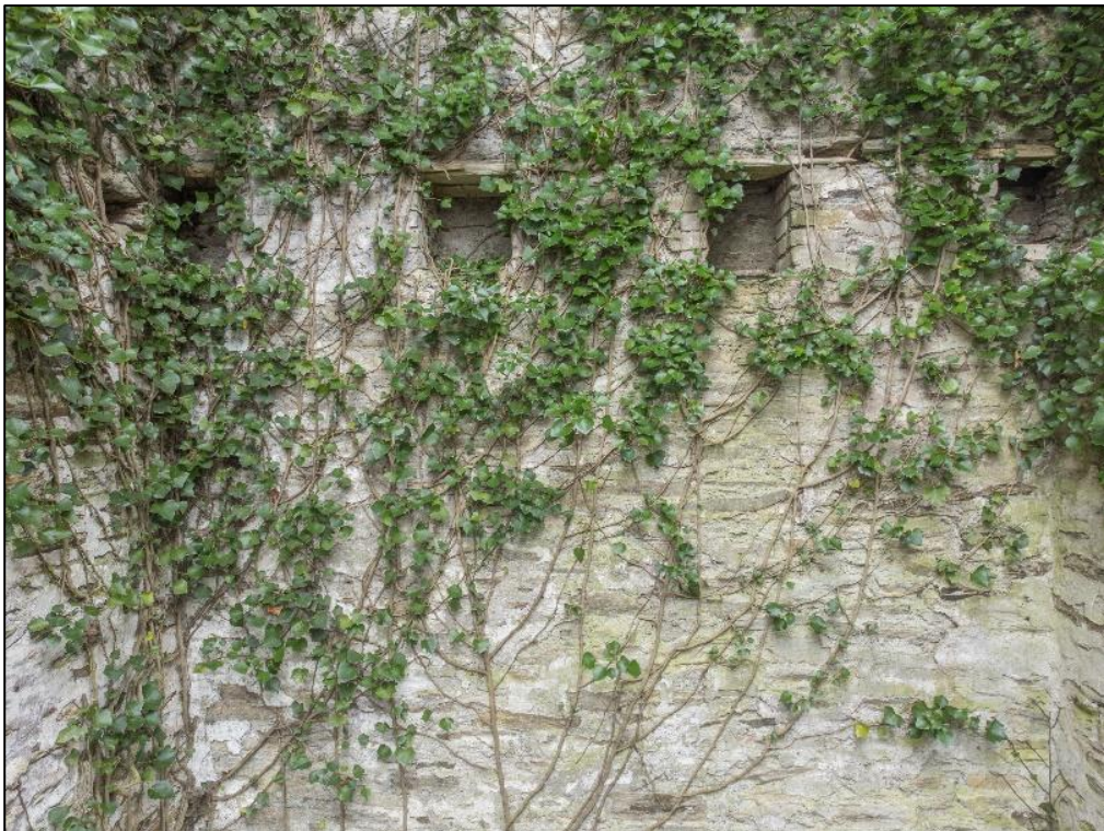
Figure 23.11 – Four high-level recessed voids.
