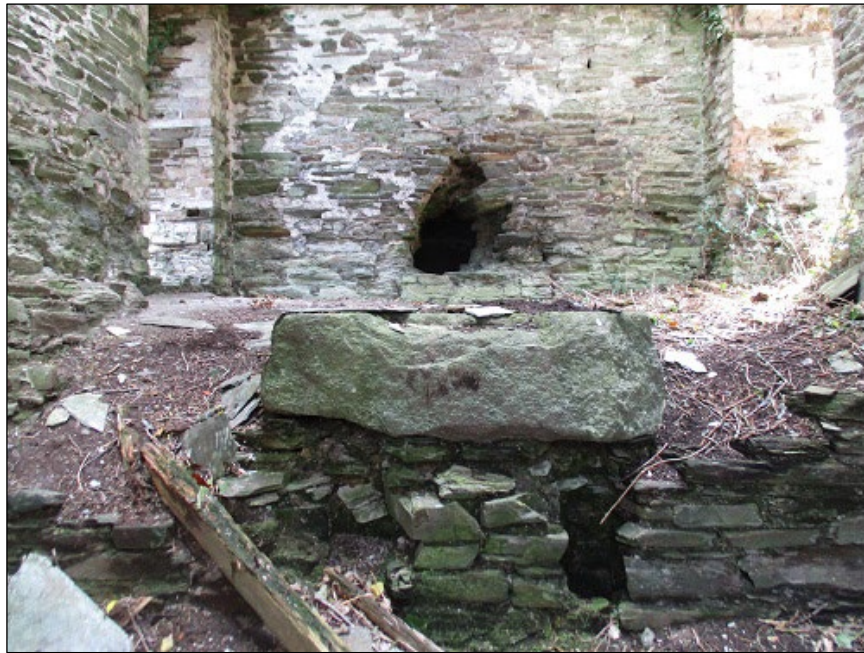
Photograph 9. Access bolt holes beneath the cylinder bedstone
