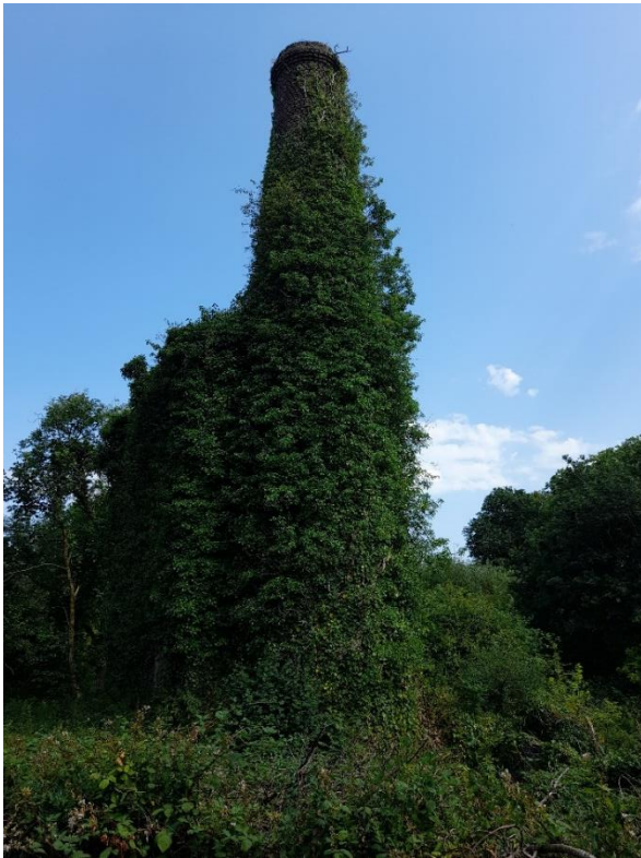
2. Engine House and chimney
