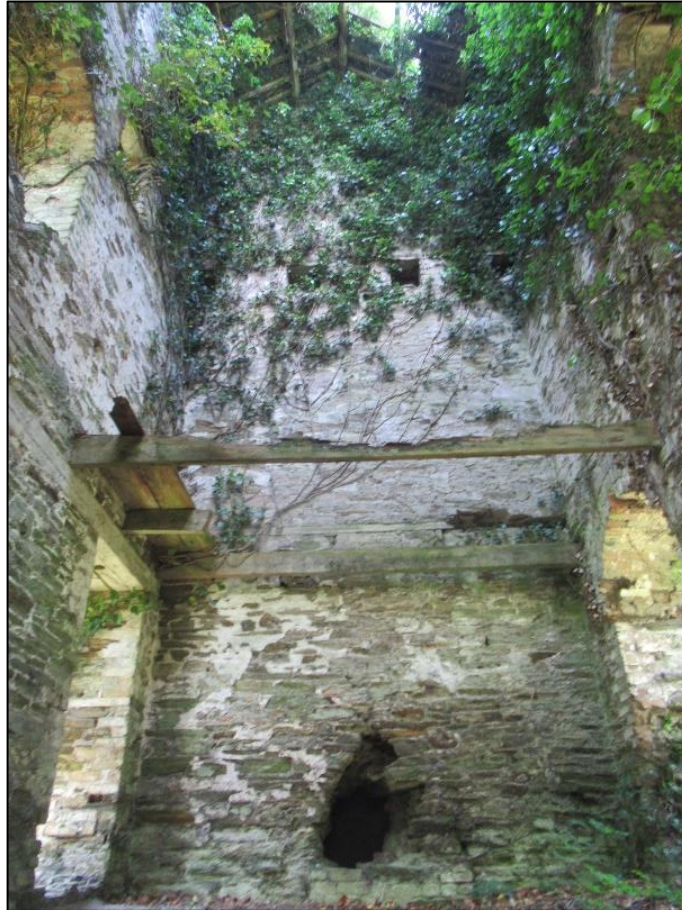
Figure 23.10 – Internal of south elevation and remaining floor structure.
