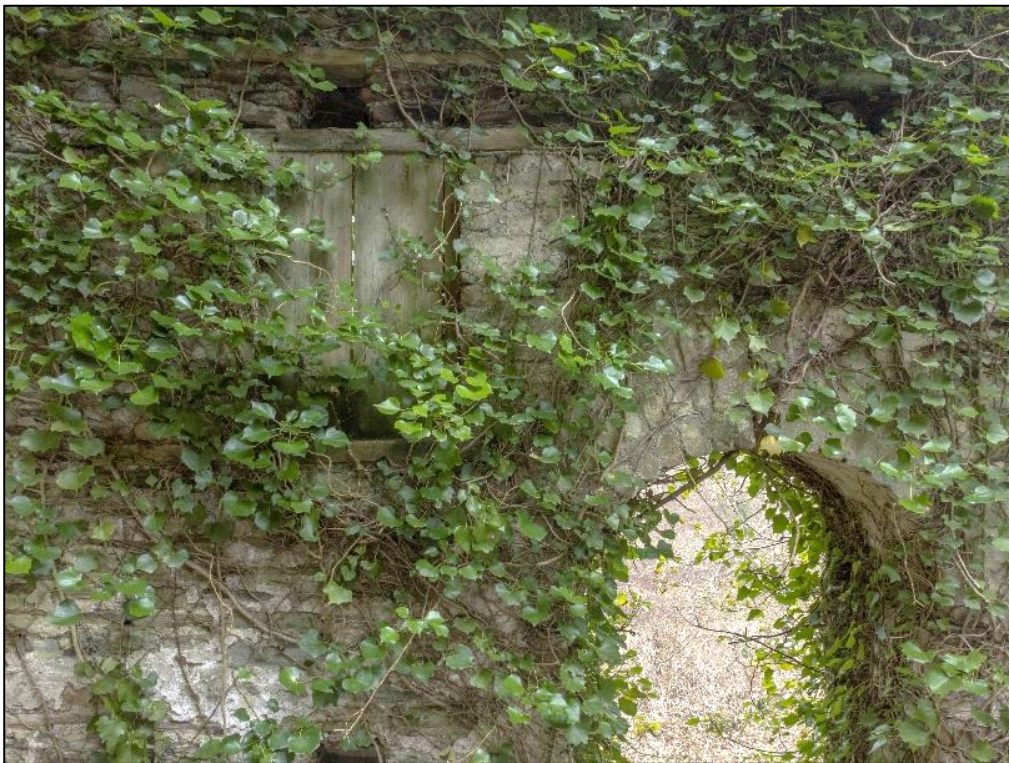
Figure 23.03 – Boarded opening in west elevation
