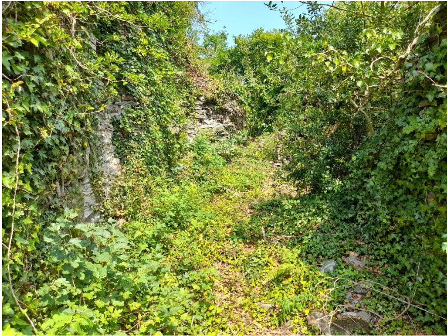
8. The Boiler House view south to north
