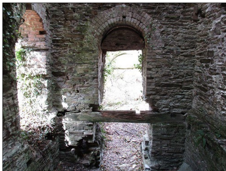
Photograph 2. Plug door looking north from within the interior
