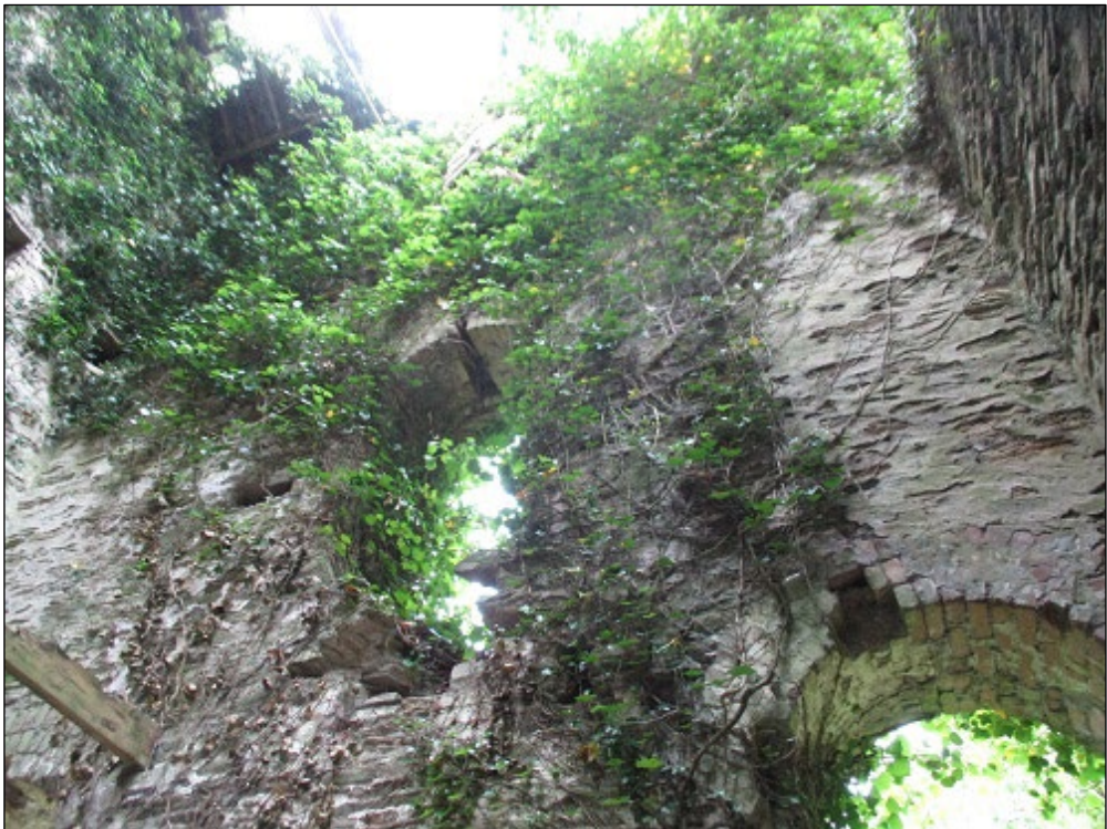
Photograph 5. West wing wall interior elevation first and second floors
