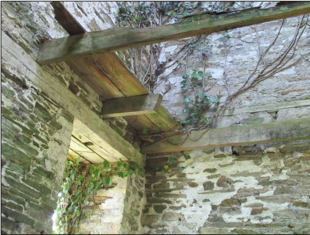
Figure 23.09 – Internal of east elevation intermediate opening with timber lintels.
