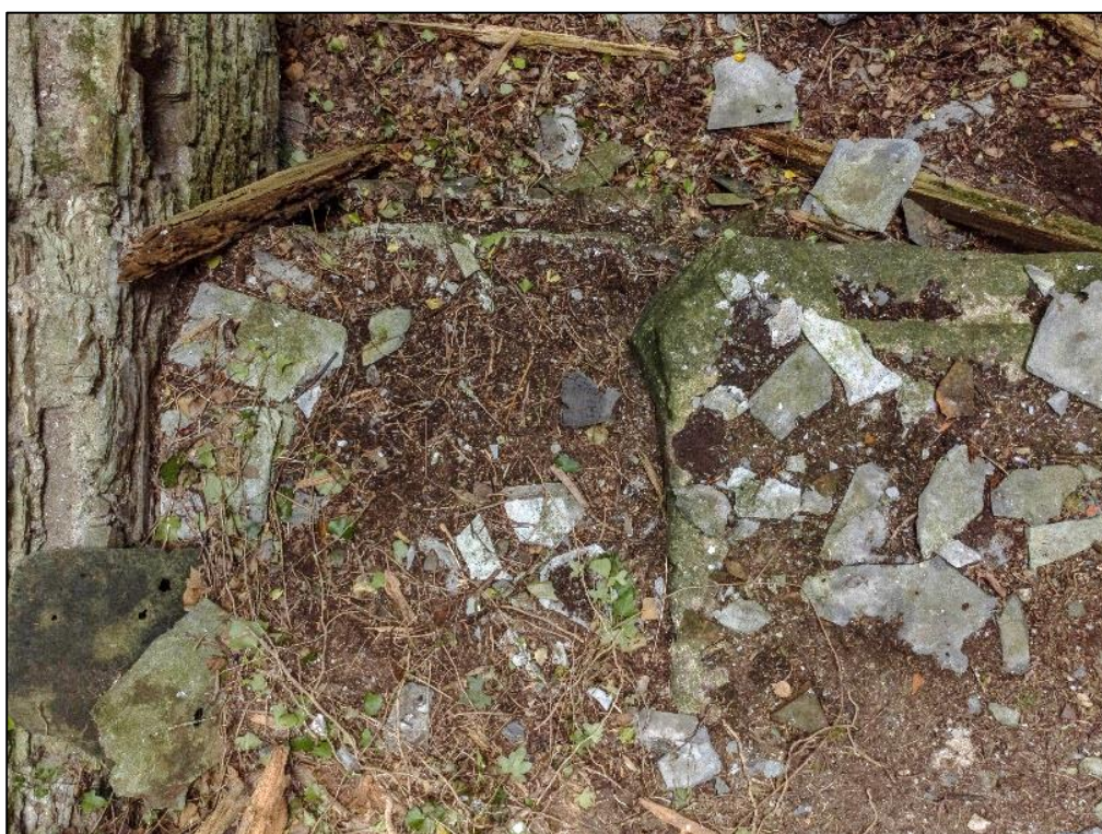
Figure 23.14 – Fallen roof slates on the floor of the Engine House
