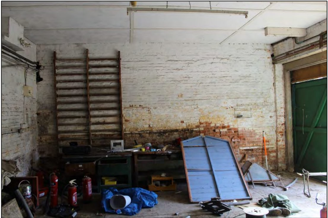
Photo 52: Overview of Room C4, looking south-east
