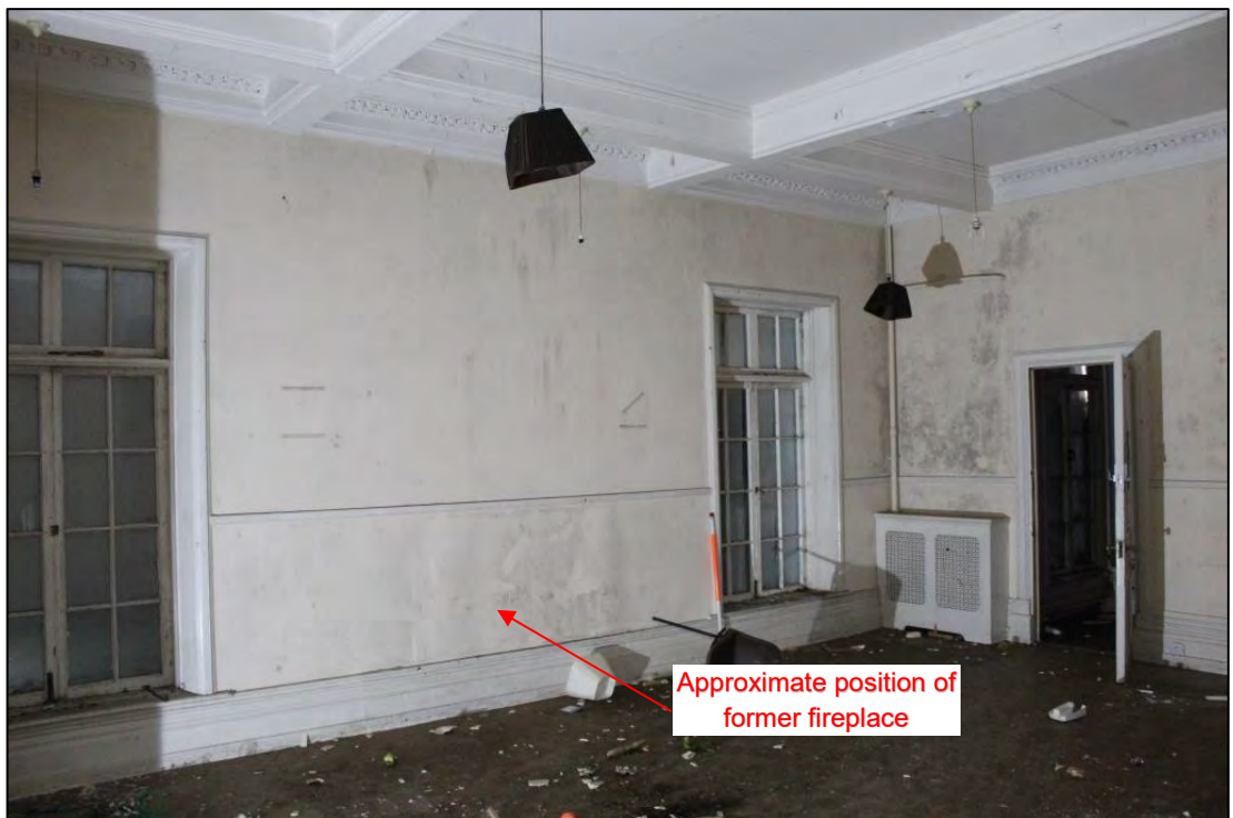
Photo 21: Overview of Room 5, looking west
