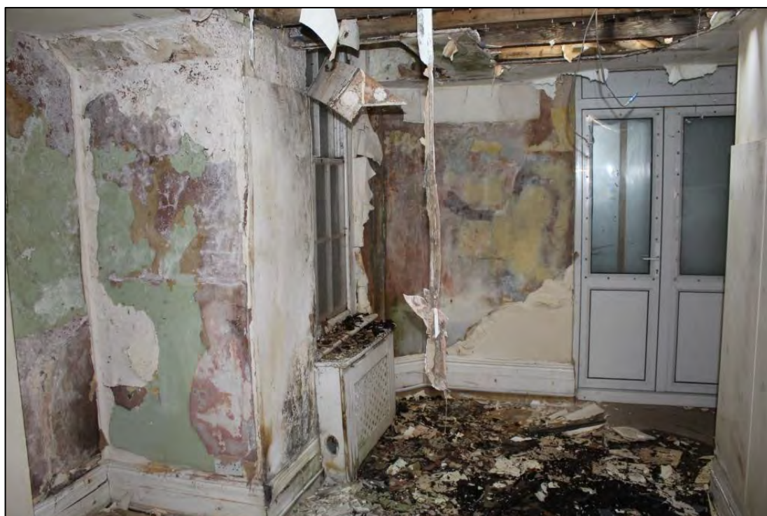
Photo 29: Overview of Room 26, looking south-east
