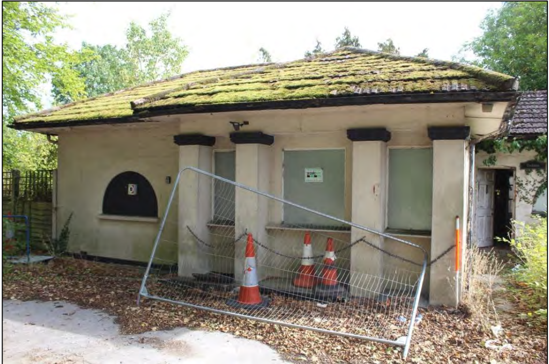
Photo 67: Northern elevation of Trelawn
