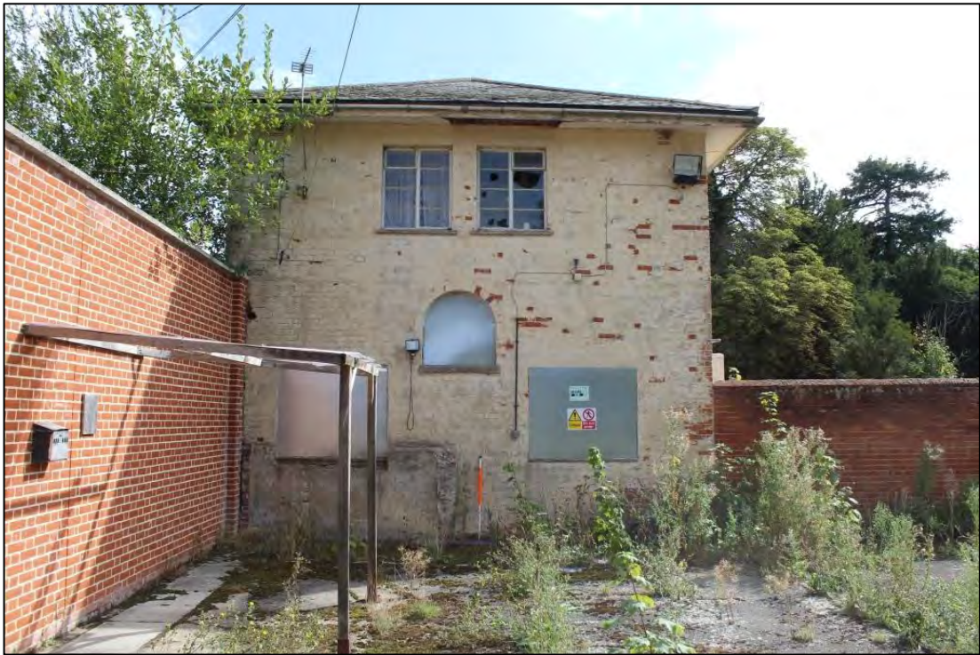
Photo 49: Overview of north-western elevation
