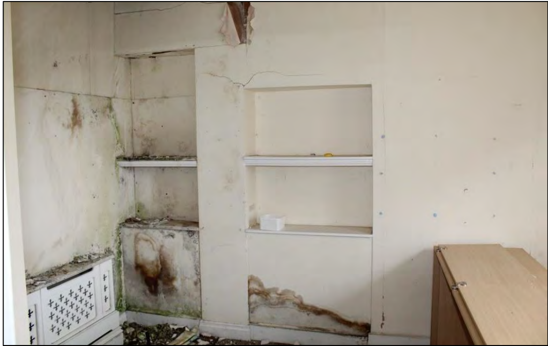
Photo 38: Recessed areas within Room 45, looking north-west
