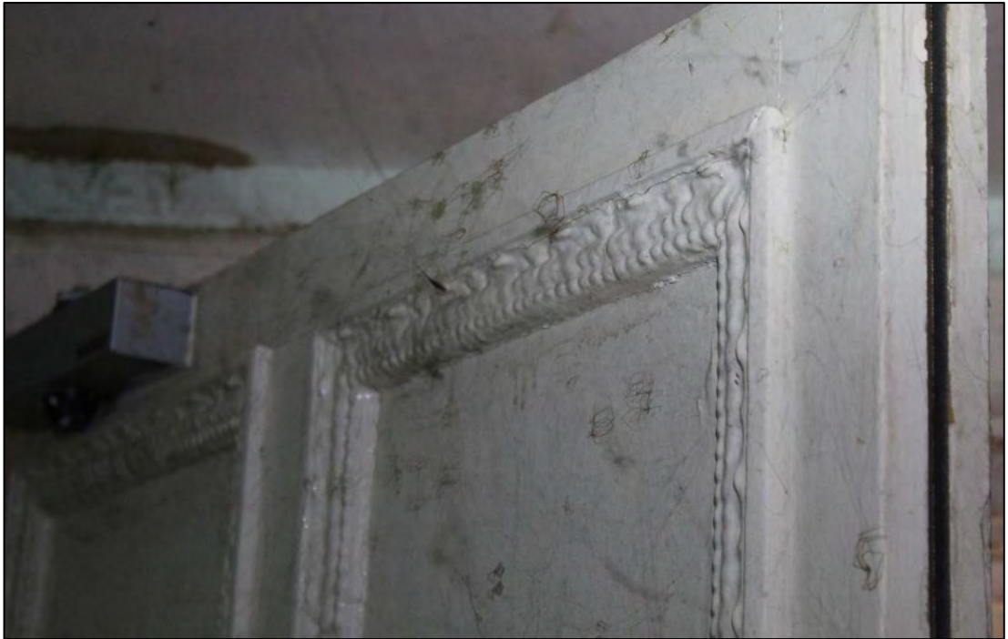
Photo 30: Detail of decorative elements on door to Room 25
