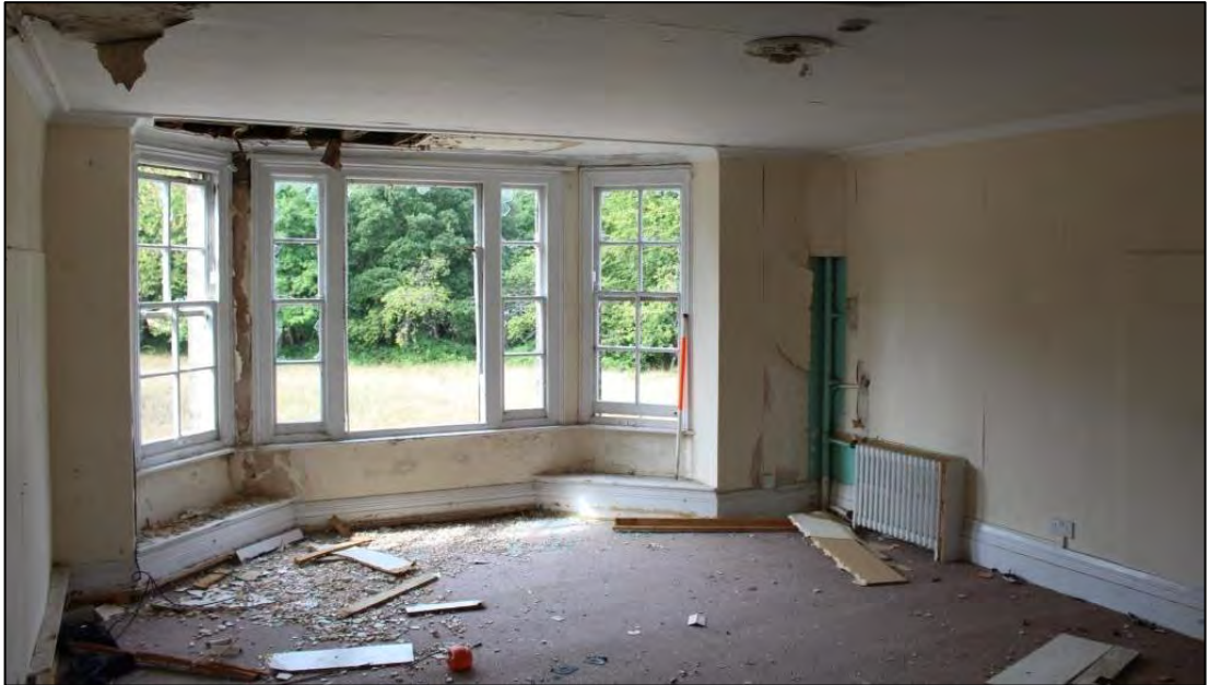
Photo 35: Overview of Room 38, looking west
