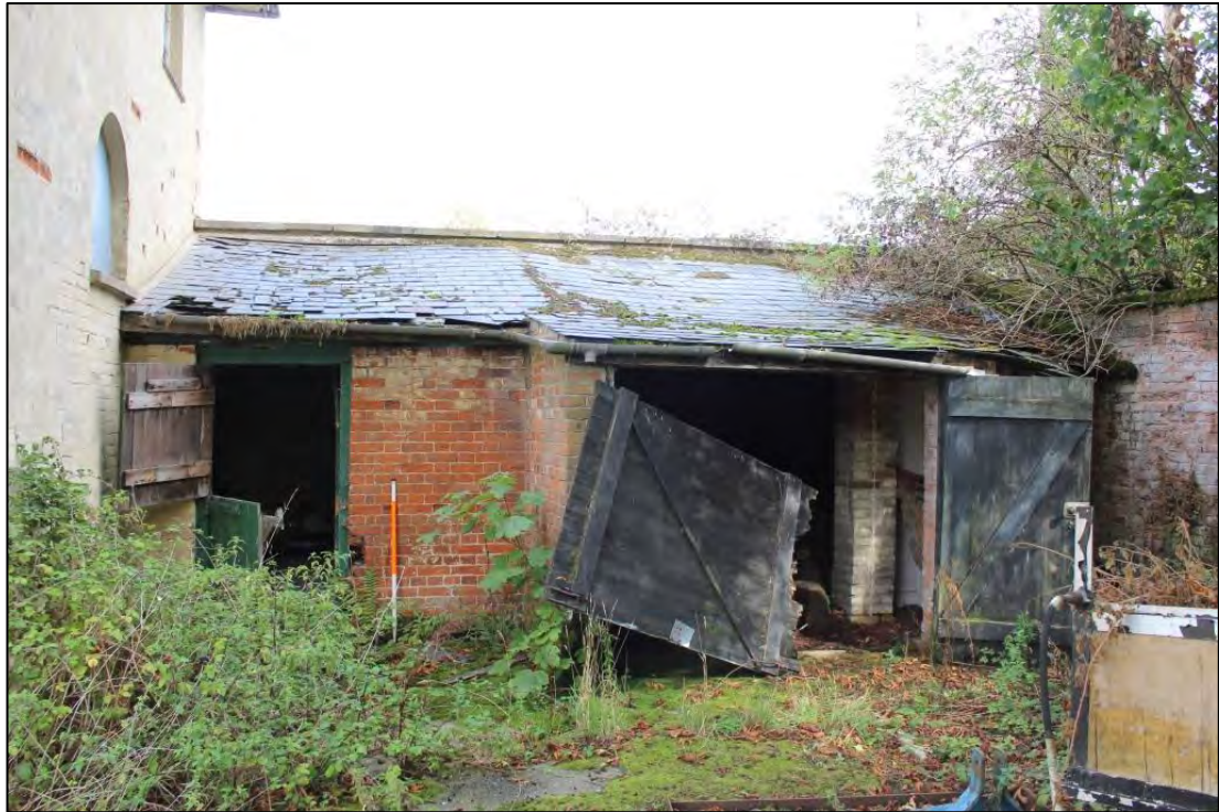
Photo 66: Outbuilding abutted to the south-eastern elevation of the coach house
