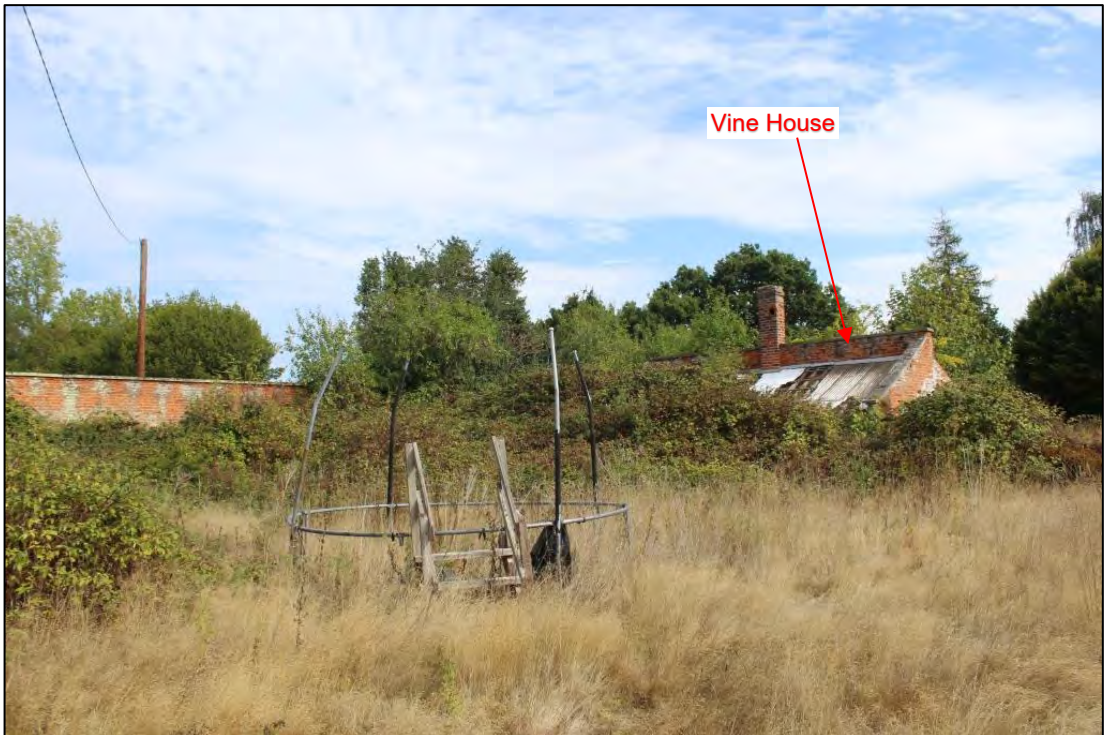
Photo 64: View of north-eastern wall alignment and the 'Vine House', looking south-east from inside the walled garden
