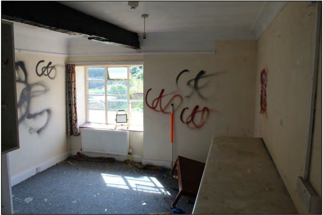
Photo 57: Overview of Room C13
