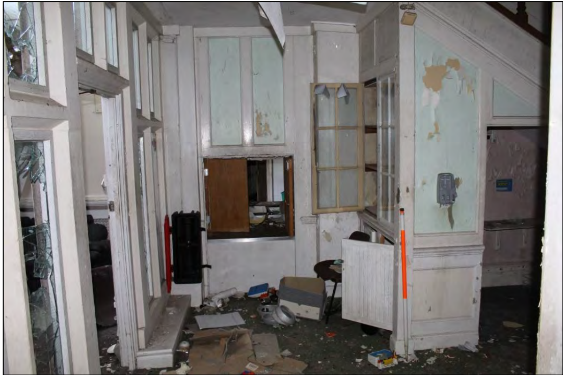
Photo 23: Overview of Room 11, looking north-east
