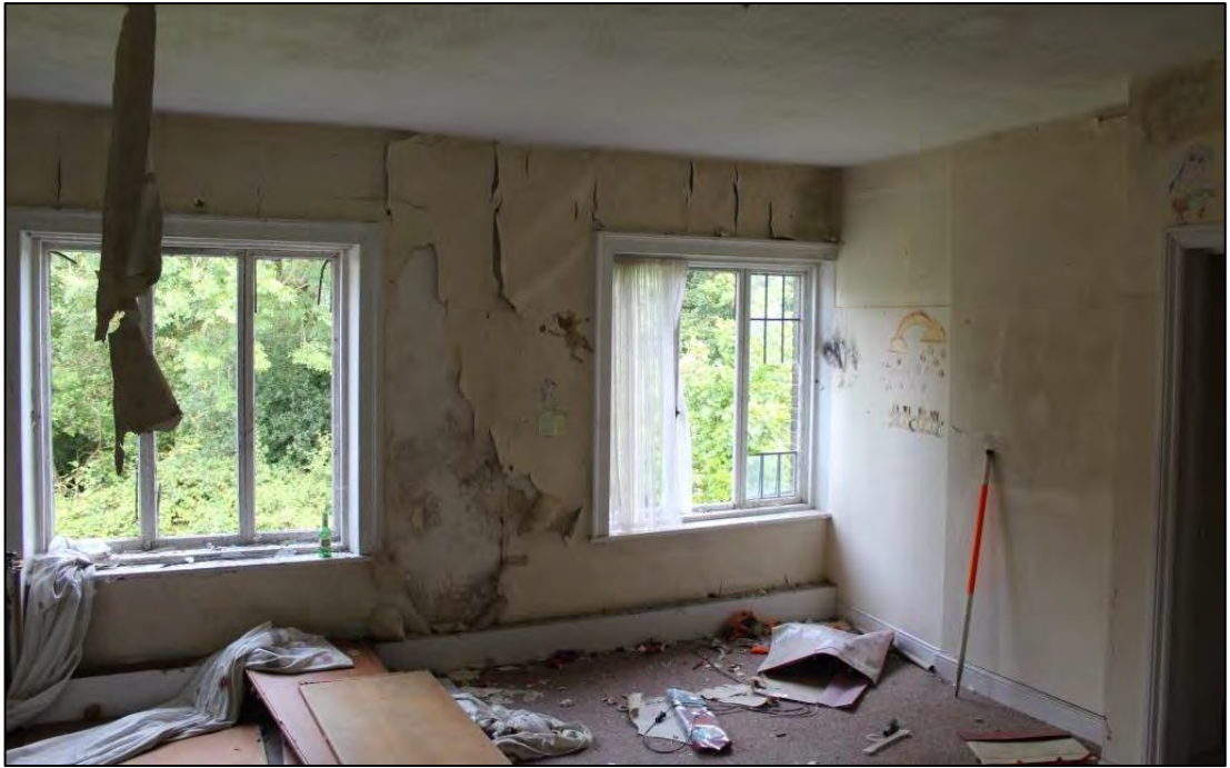
Photo 41: Overview of Room 52, looking north
