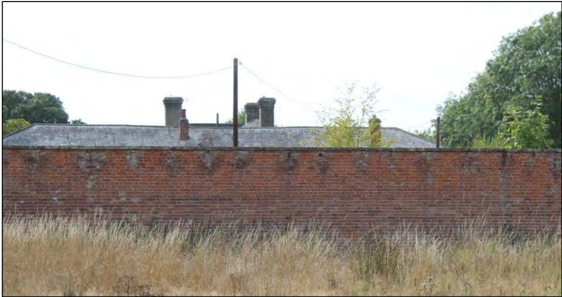
Photo 61: Section of the north-eastern wall alignment (external view)
