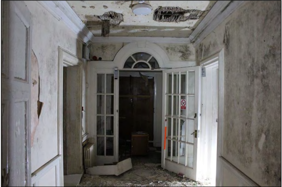
Photo 17: Overview of Room 3, looking south-west
