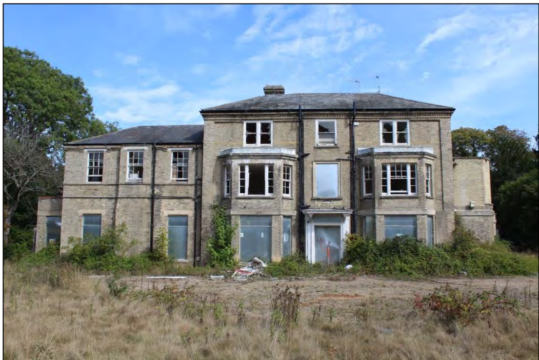
Photo 1: South-western elevation of the house
