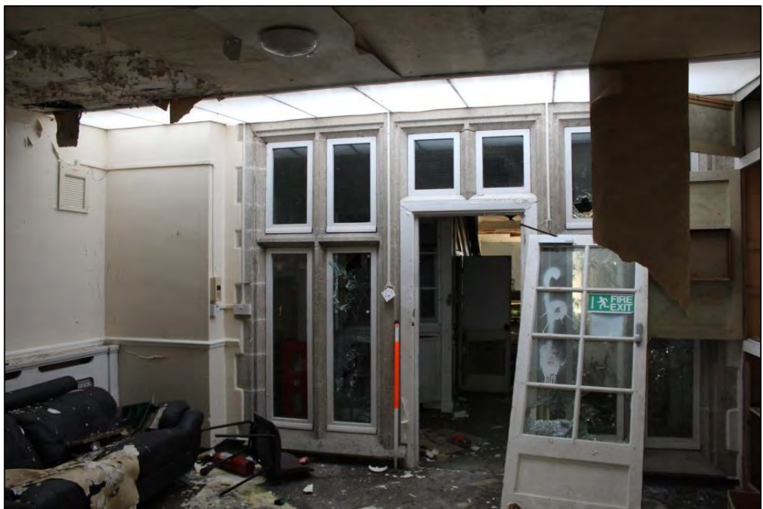
Photo 22: Overview of Room 10, looking south-east towards Room 11
