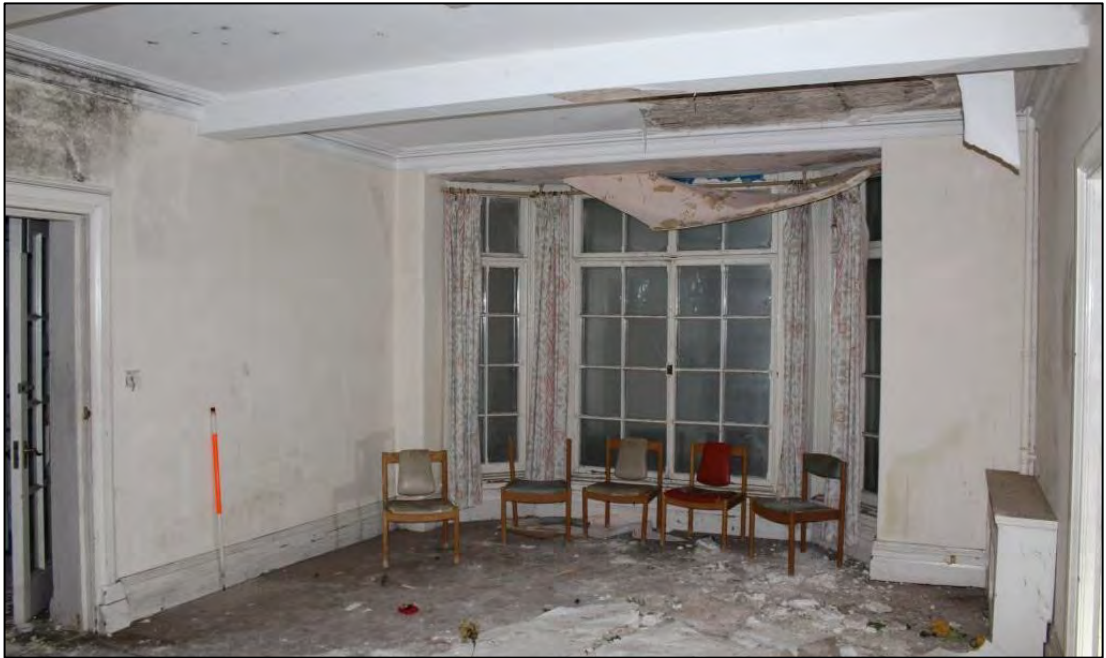
Photo 18: Overview of Room 4, looking south-west
