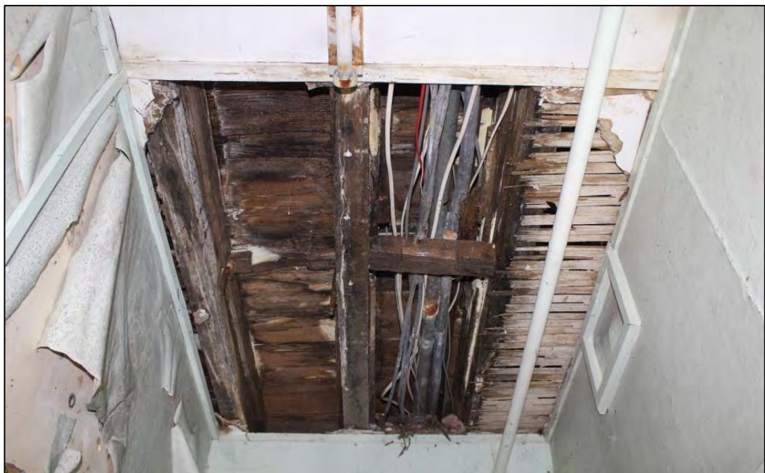
Photo 28: Detail of ceiling construction, Room 21
