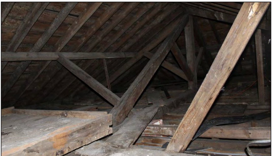
Photo 46: Detail of roof structure
