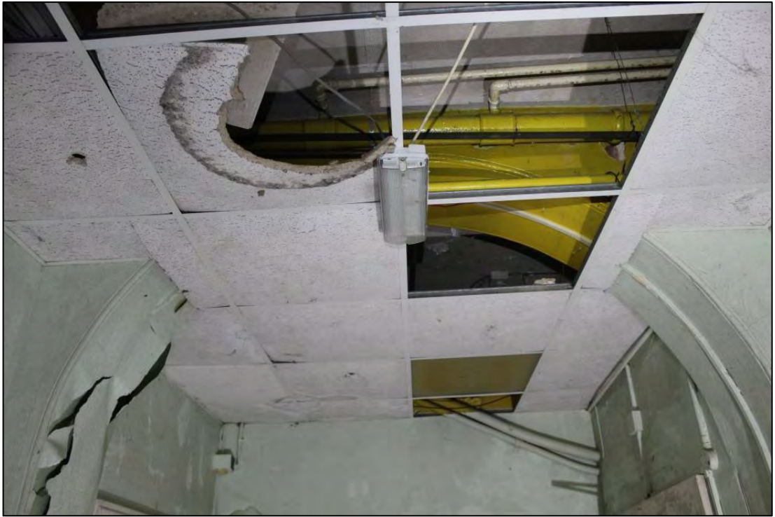
Photo 25: Detail of archway within Room 18
