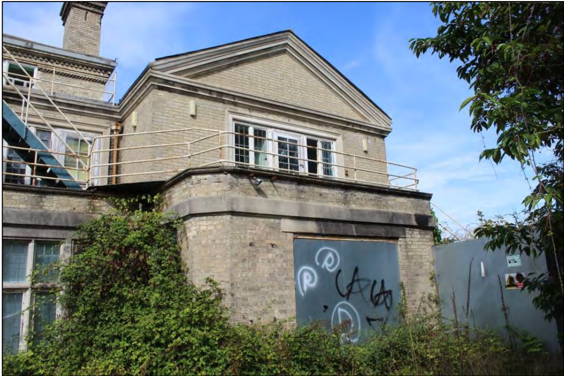
Photo 6: Eastern extent of south-eastern elevation
