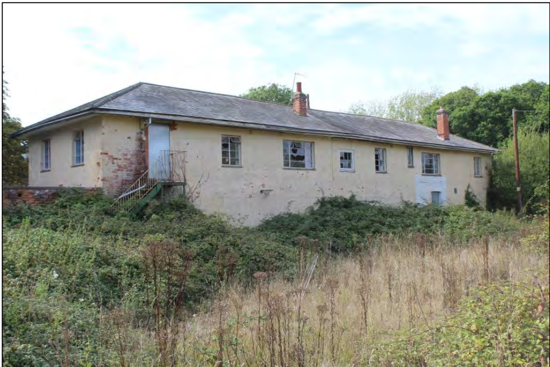
Photo 50: Overview of north-eastern elevation
