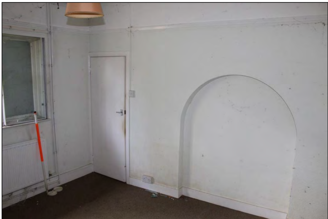
Photo 71: Arches recess within Room T3
