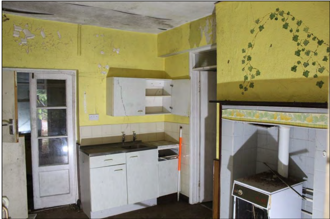
Photo 70: Overview of Room T1, looking south
