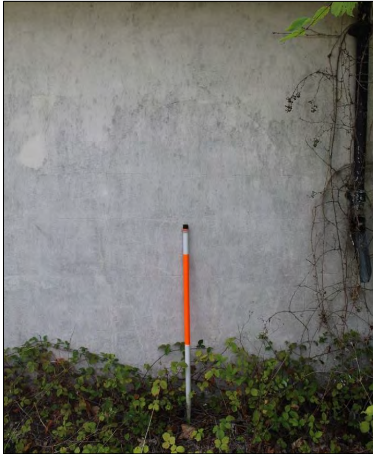
Photo 69: Arch within eastern elevation
