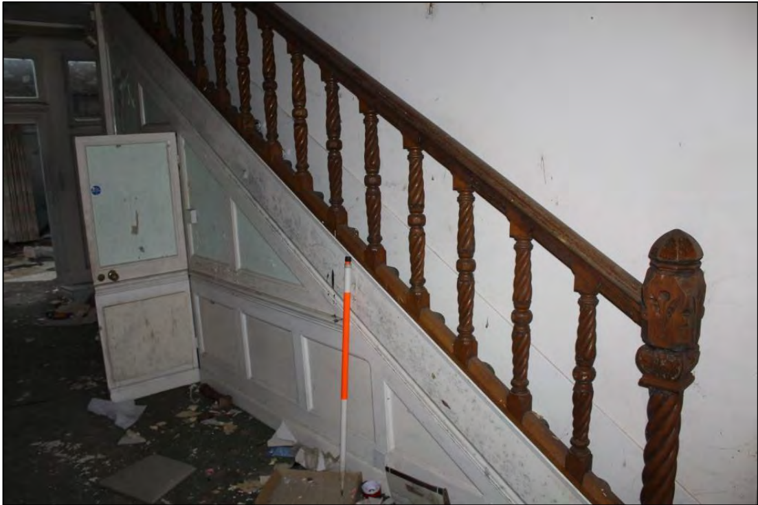
Photo 14: Detail of staircase elements
