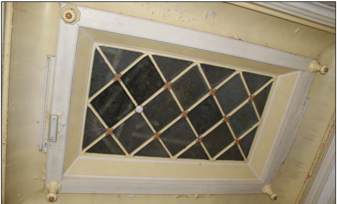
Photo 42: Panel above Room 53
