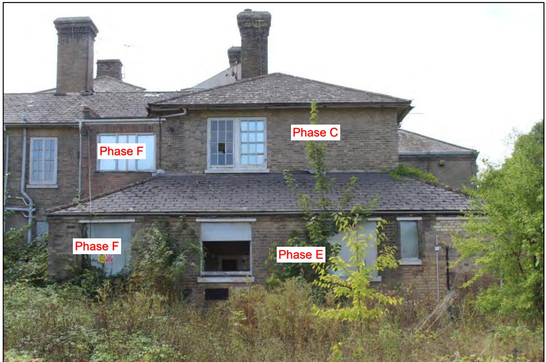
Photo 8: Northern extent of north-eastern elevation
