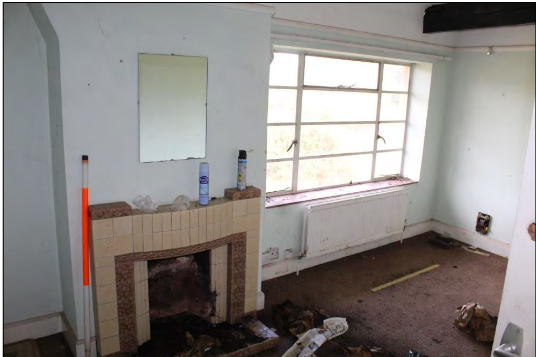
Photo 56: Overview of Room C8, looking east
