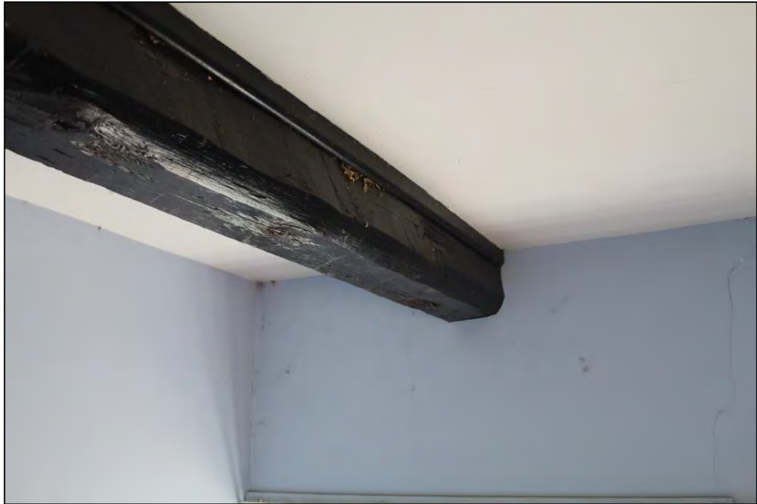
Photo 59: Detail of chamfered beam in Room C10
