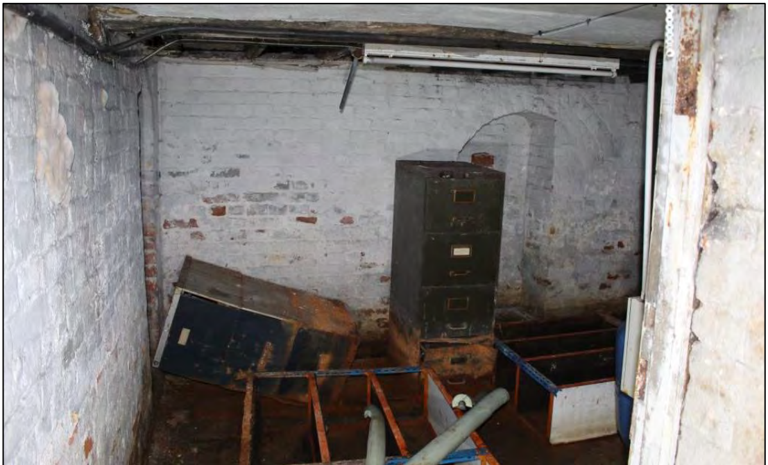
Photo 31: Overview of Basement (Room 31), looking west
