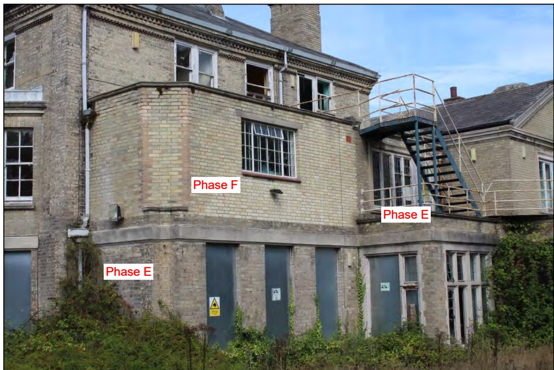
Photo 5: South-eastern elevation of the house
