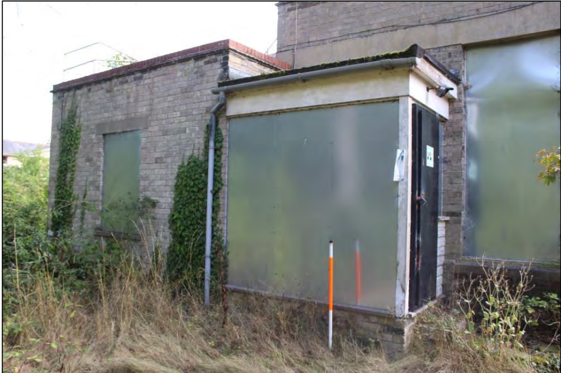
Photo 9: Partial view of north-western elevation
