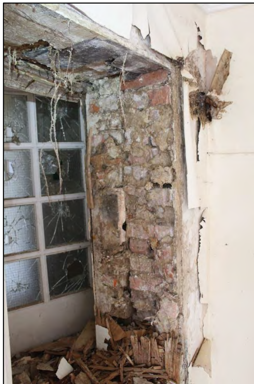
Photo 36: Detail of wall fabric within Room 38
