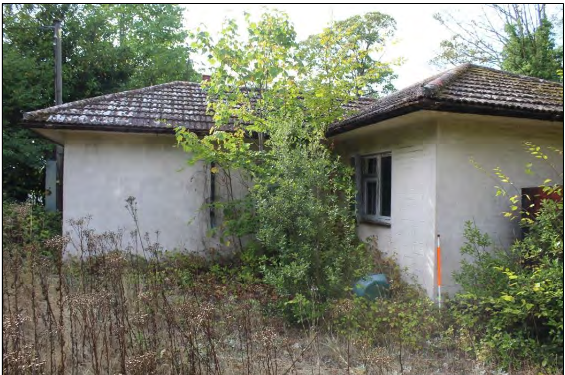
Photo 68: Eastern elevation of Trelawn
