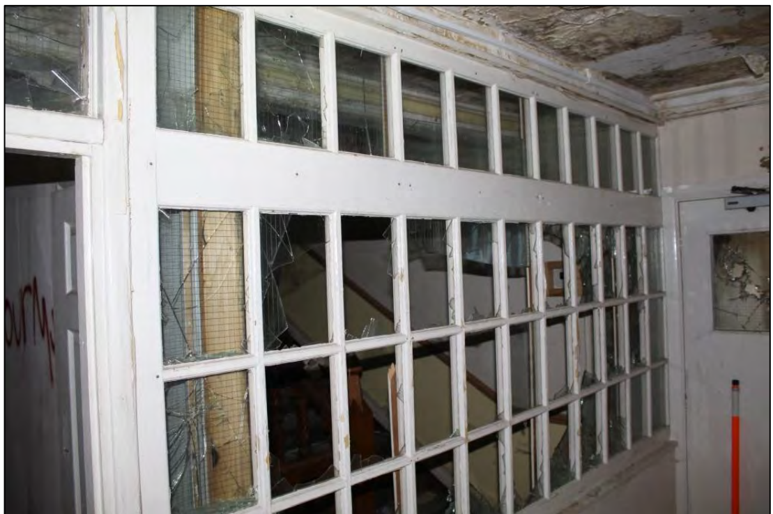
Photo 34: Overview of glazed screen in Room 37
