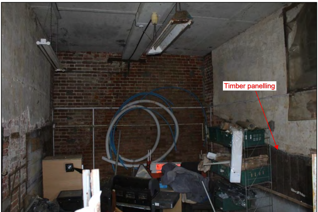
Photo 55: Overview of Room C7, looking north-east
