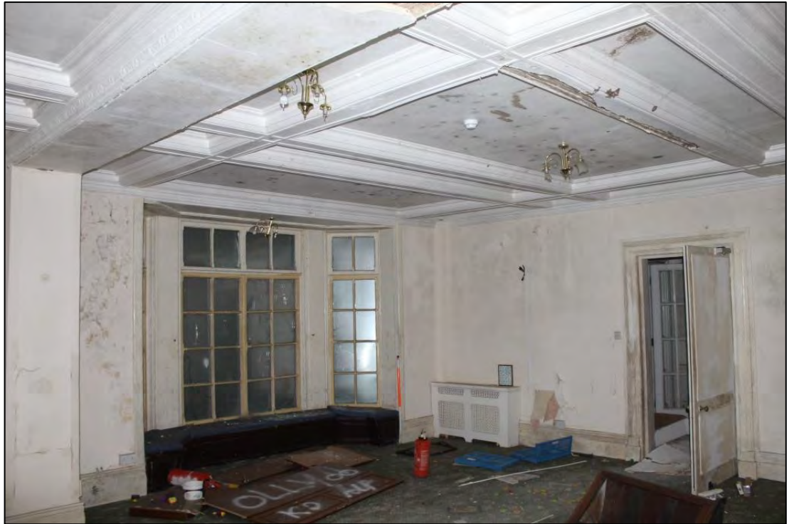
Photo 15: Overview of Room 15, looking west
