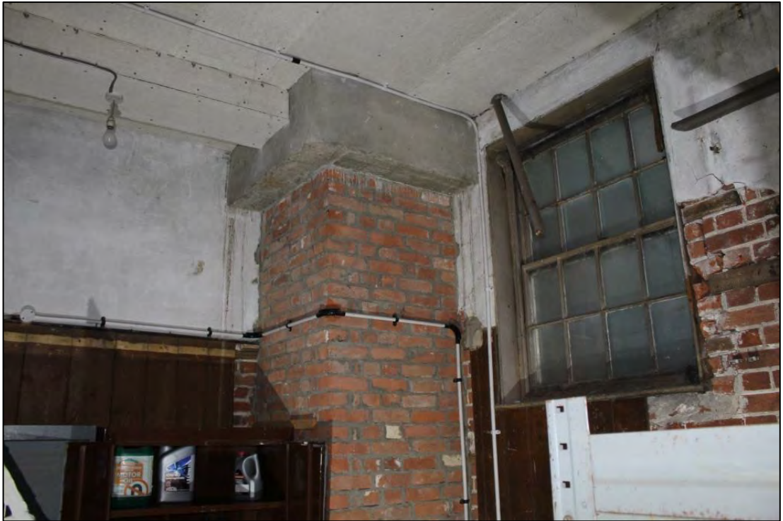
Photo 54: Overview of Room C5, looking north
