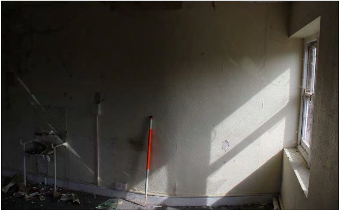
Photo 45: Partition between Rooms 58 and 59, viewed north-east from within Room 58
