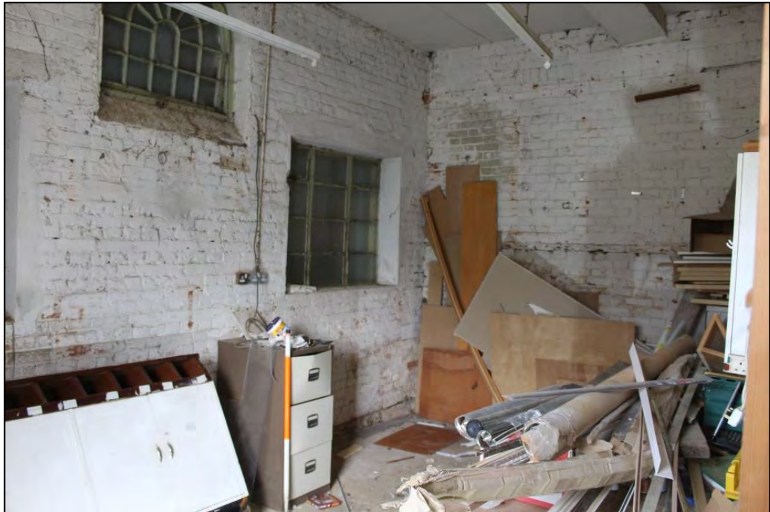
Photo 51: Overview of Room C2, looking north
