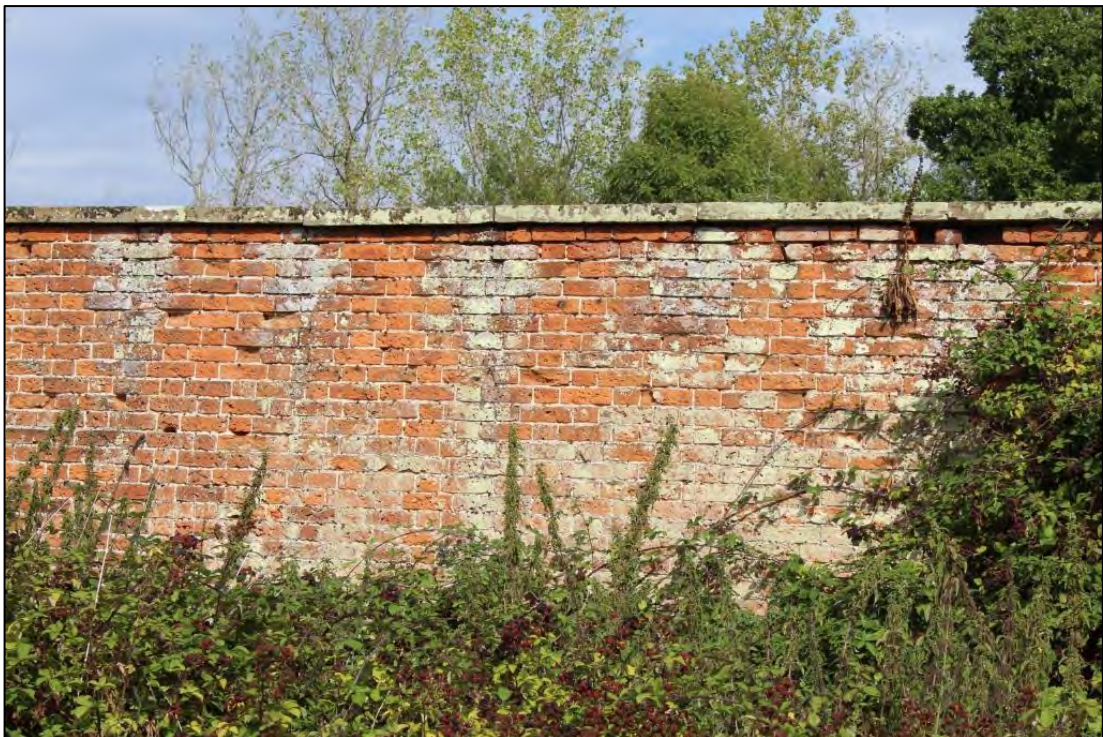
Photo 62: Section of the north-eastern wall alignment (internal view)
