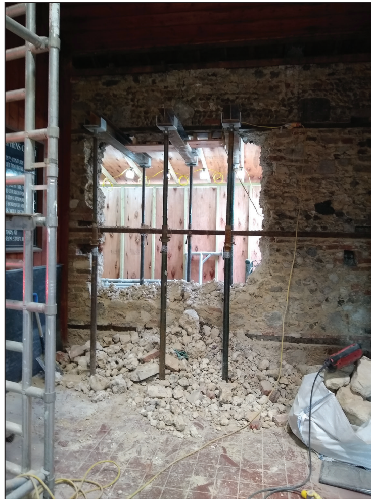
Removal of wall underway, looking north-west
