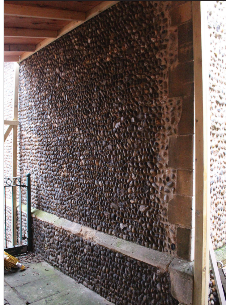
Exterior face of wall prior to removal, looking south-east
