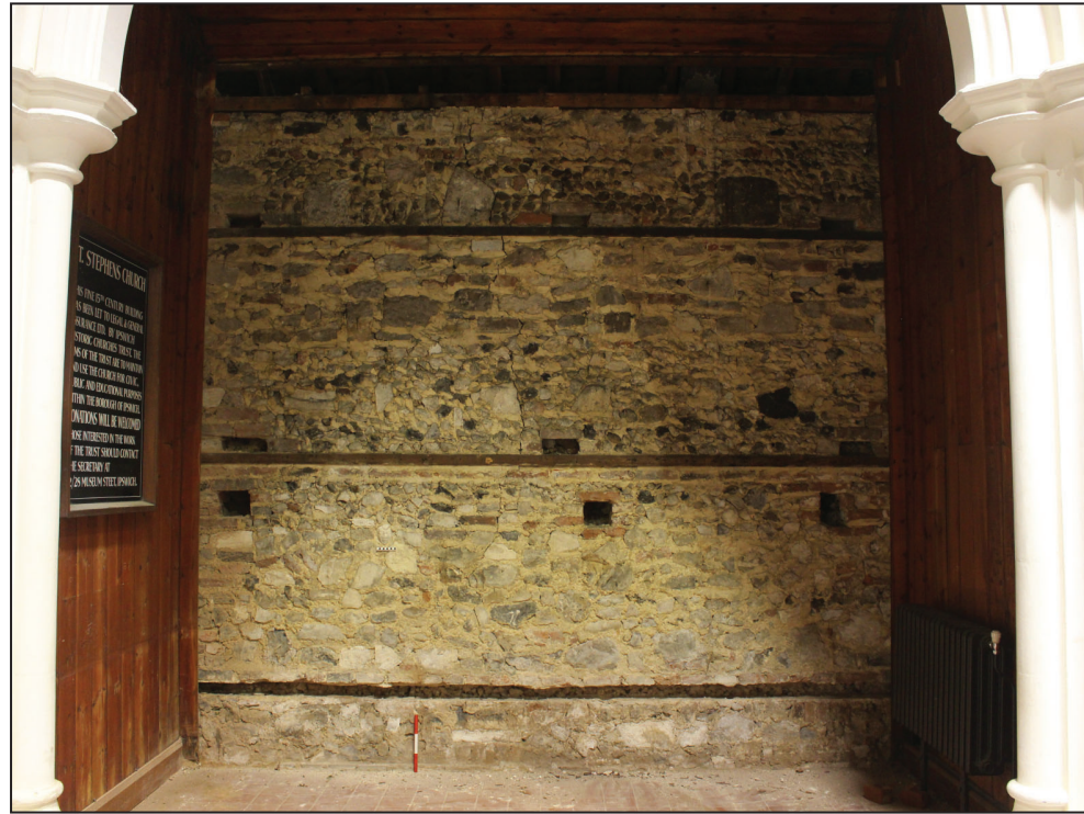
Interior face of wall prior to removal, looking north (0.3m and 0.1m scales)
