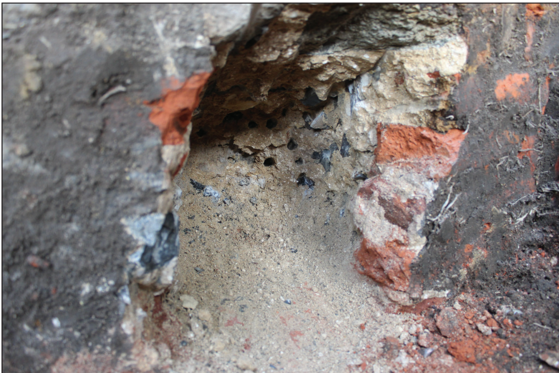
Drain trench excavation; foundation detail, looking north-east
