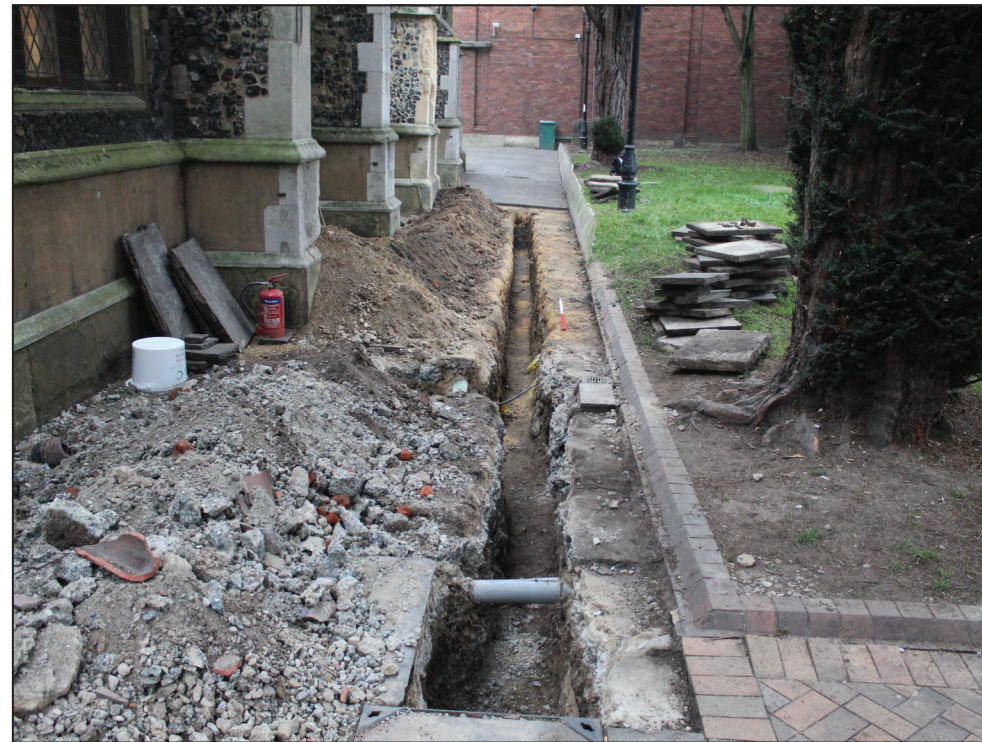
Drain trench, looking east (1m scale)
