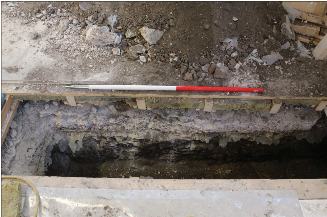
Drain trench, looking east (1m scale)
