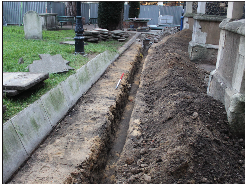
Drain trench, looking west (1m scale)
