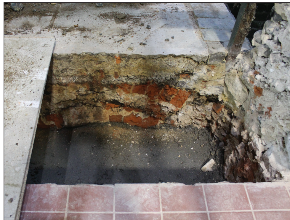
Vaulted brickwork beneath wall, looking north
