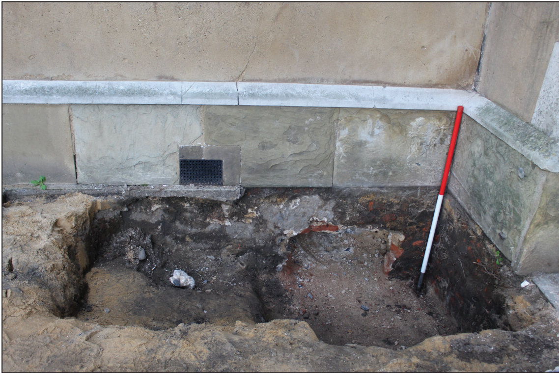
Drain trench excavation through foundation, looking north (1m scale)
