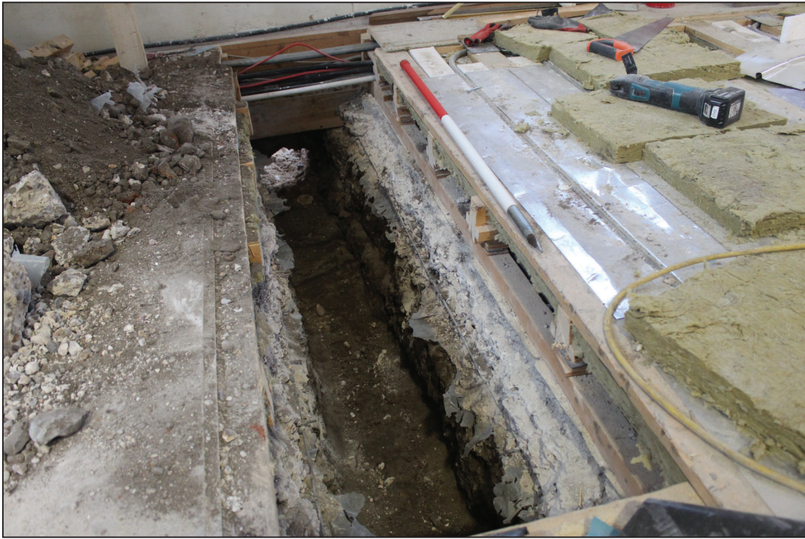
Drain trench, looking south (1m scale)
