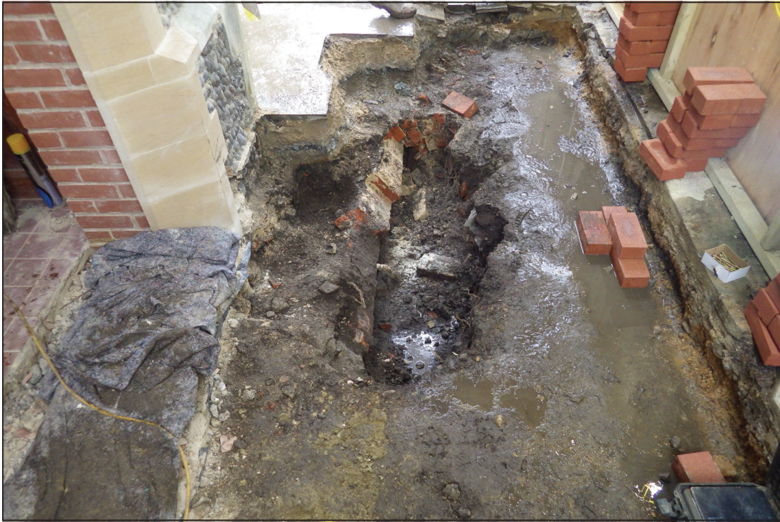
Exposed burial vault, looking west
