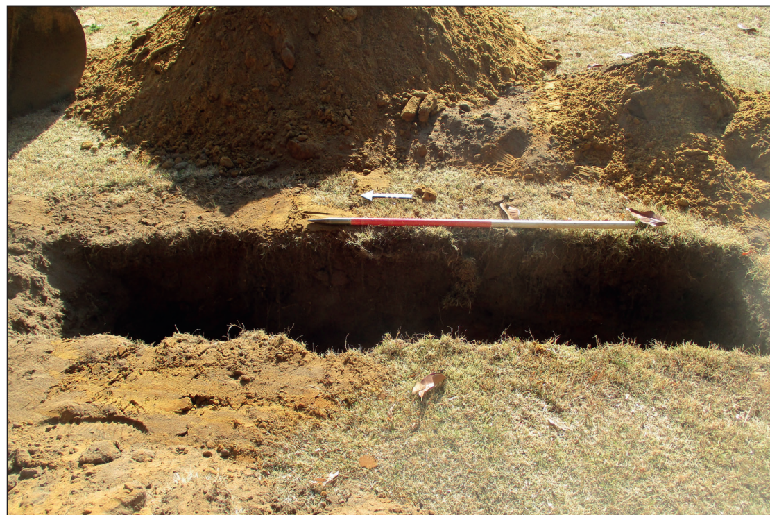
Trench 1, looking east (scale 1m)
