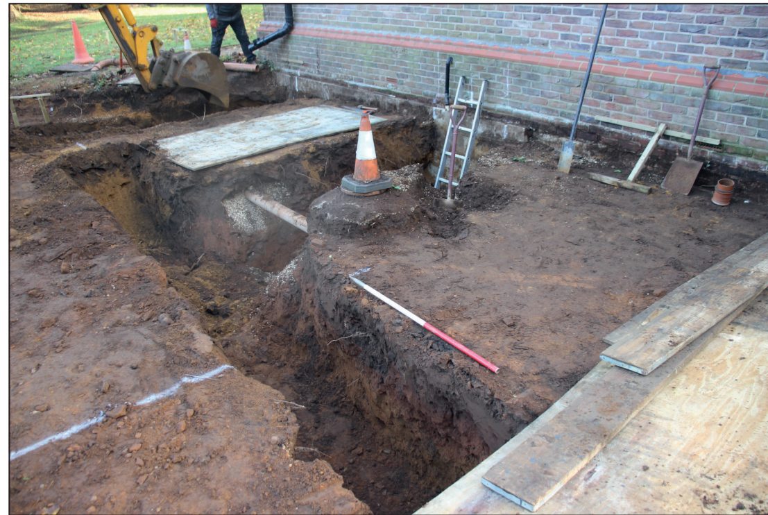
Trench 3, looking east (scale 1m)
