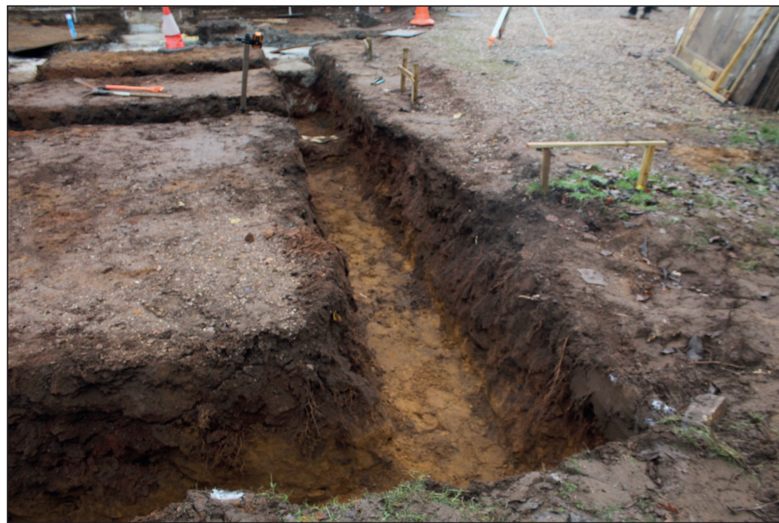
Trench 4, looking south-west
