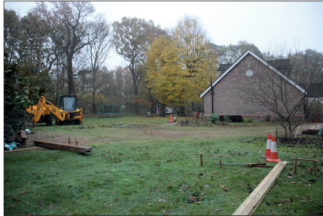
Site pre-excitation, looking south-east
