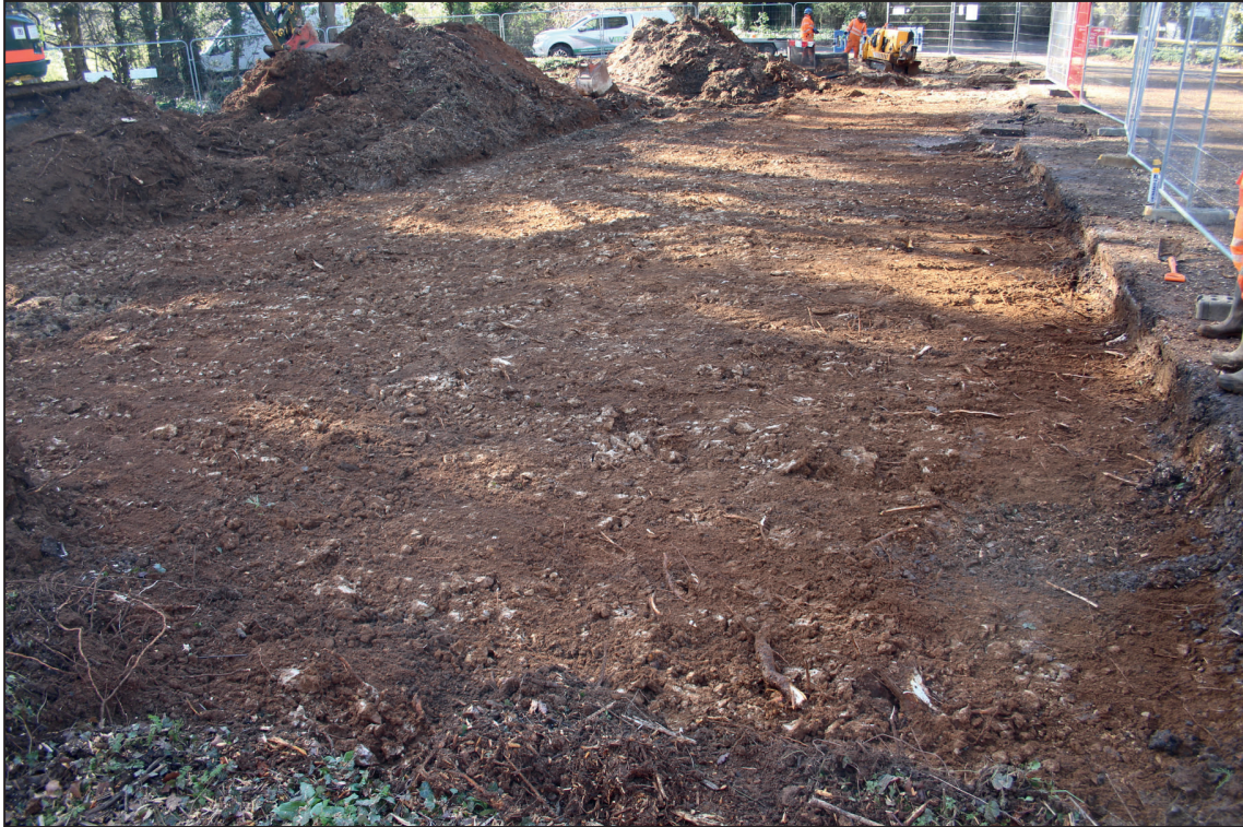
Monitored groundworks, looking west
