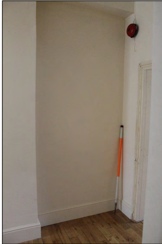
Photo 31: Former doorway between Rooms 3 and 13, viewed from Room 13
