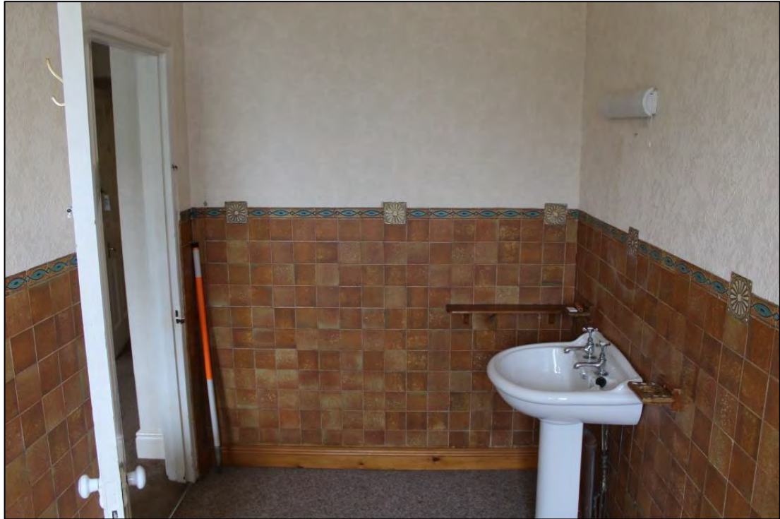
Photo 44: Detail of tiling in the ensuite of Room 36
