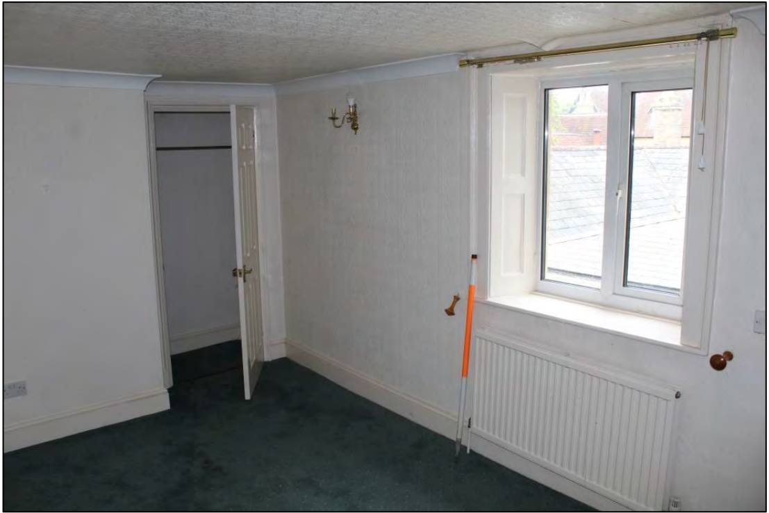
Photo A27: Room 41, looking south-west
