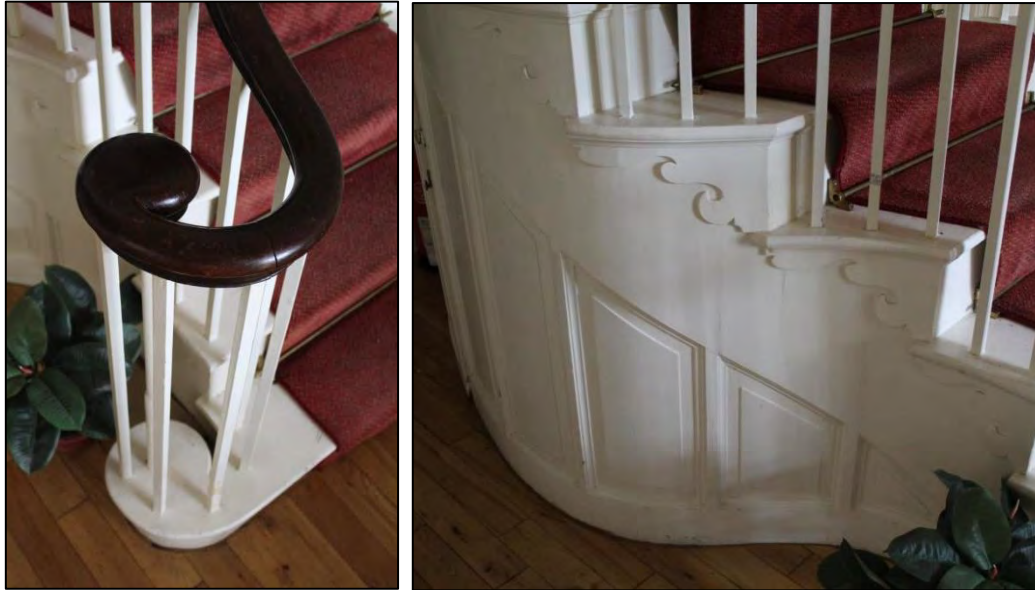
Photos 19 and 20: Curved handrail end and decorated tread end
