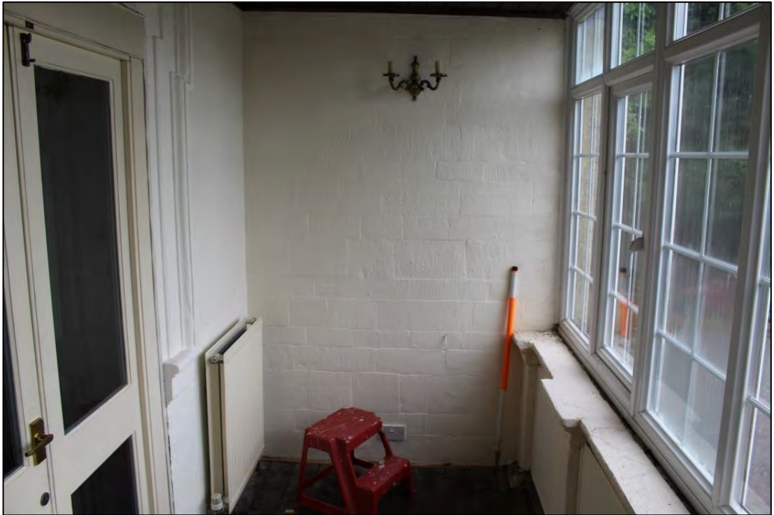
Photo A21: First floor balcony, looking south-east
