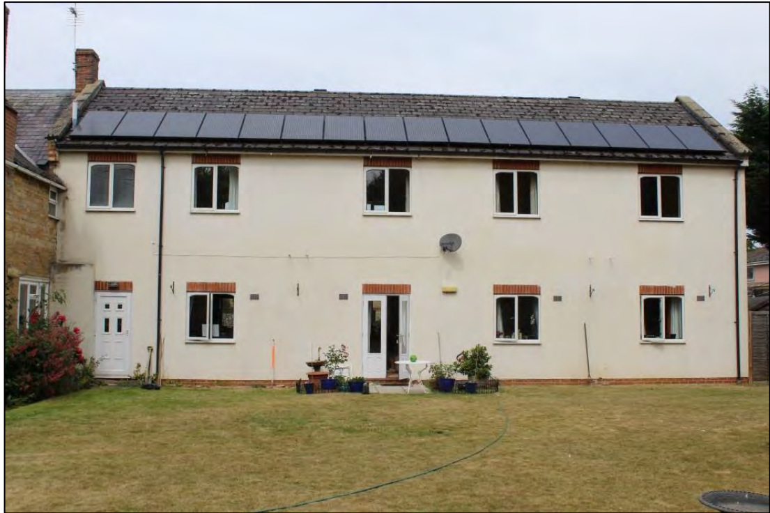
Photo 8: Phase F extension, looking west
