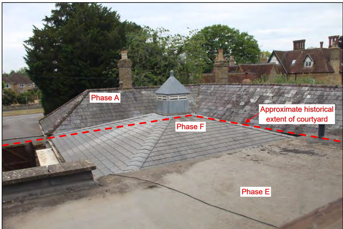
Photo 10: Overview of former courtyard area
