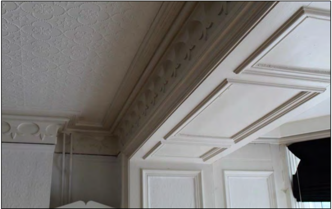
Photo 23: Detail of cornice in Room 4
