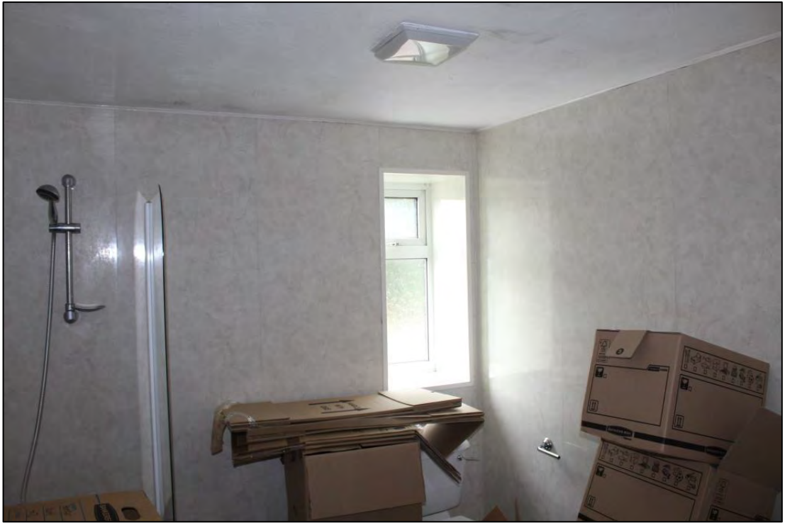
Photo A15: Room 21, looking south-west
