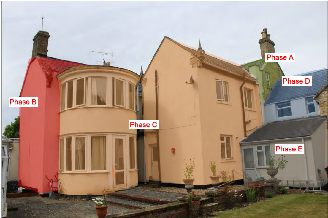
Photo 6: Overview of northern and north-eastern elevations
