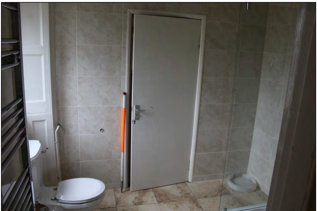
Photo A26: Rooms 39/40 bathroom, looking north
