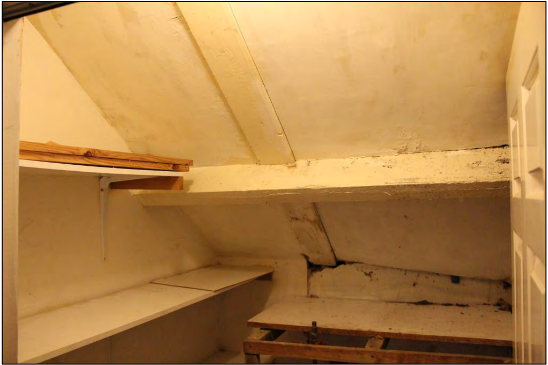
Photo A31: Detail of roof structure within former barn
