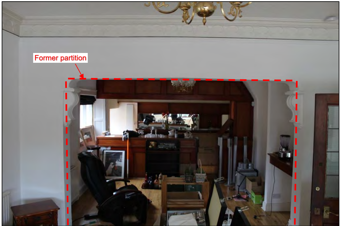
Photo 21: Overview of Rooms 4 and 5, looking north
