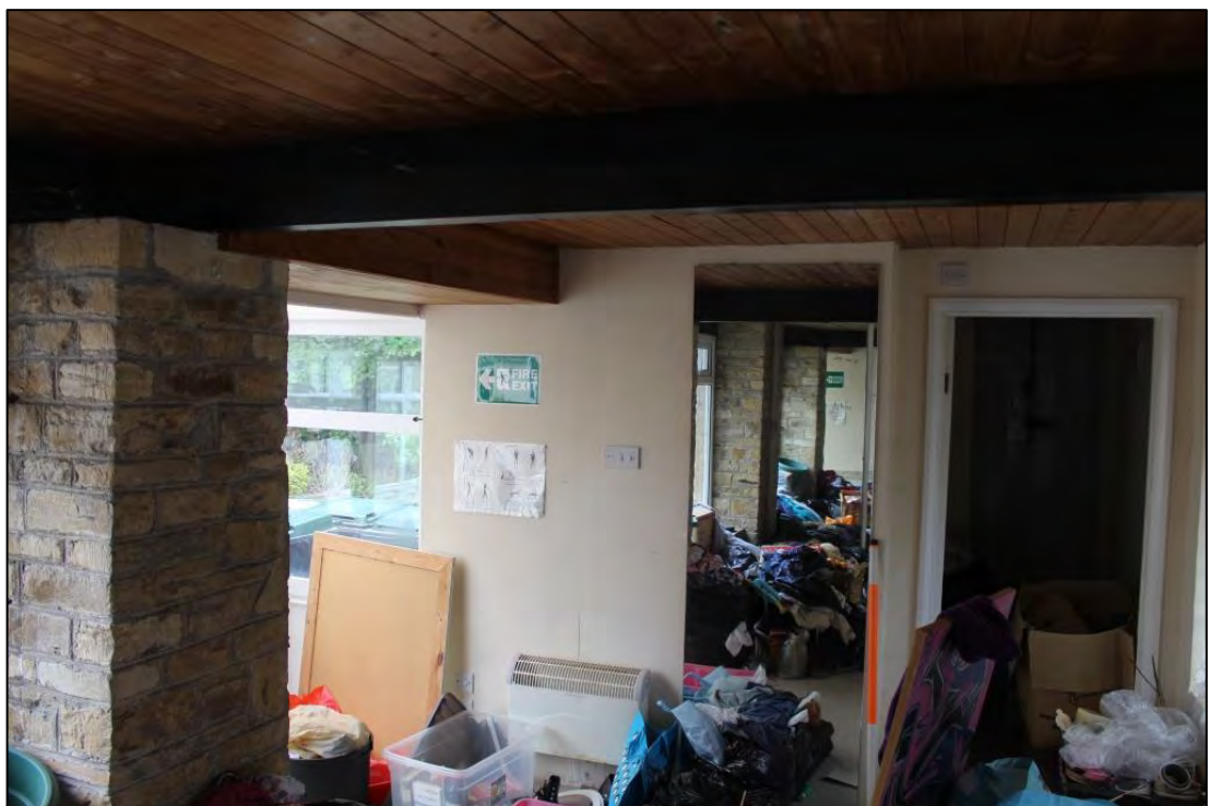
Photo A8: Room 10, looking south-east
