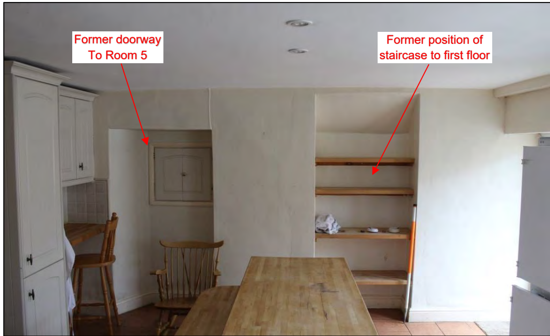
Photo 30: Overview of Room 12, looking south
