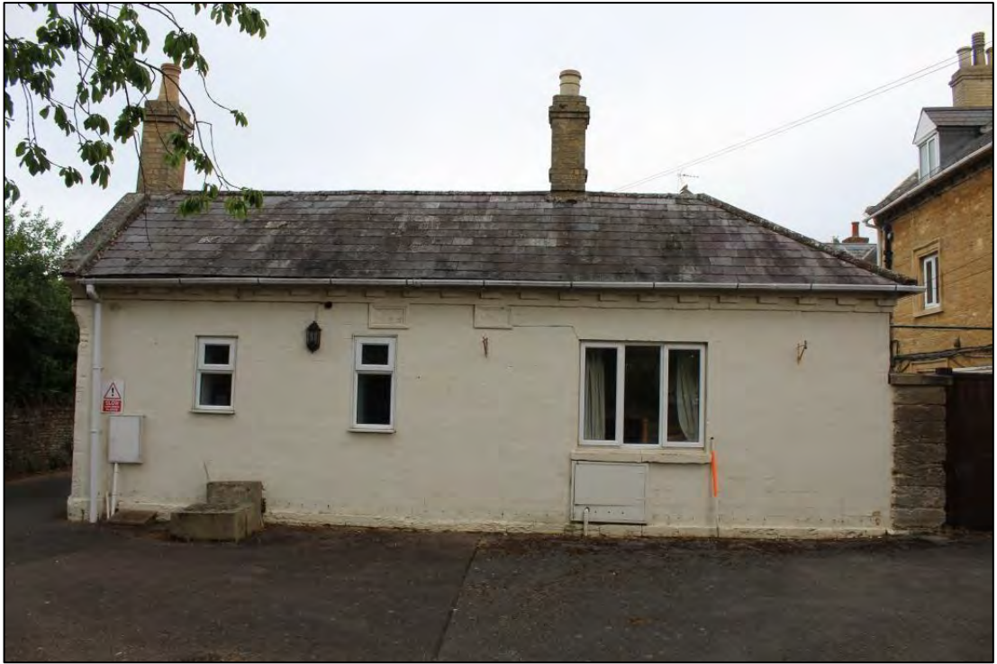
Photo 11: Southern elevation of stable block
