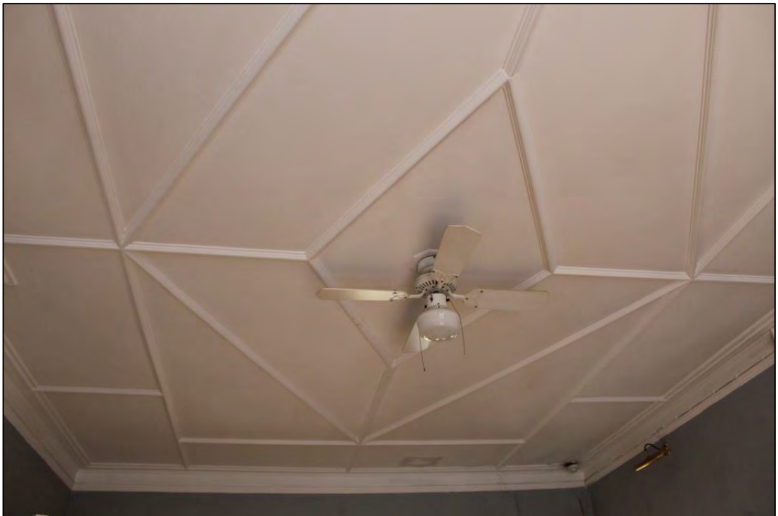
Photo A4: Ceiling detail in Room 6
