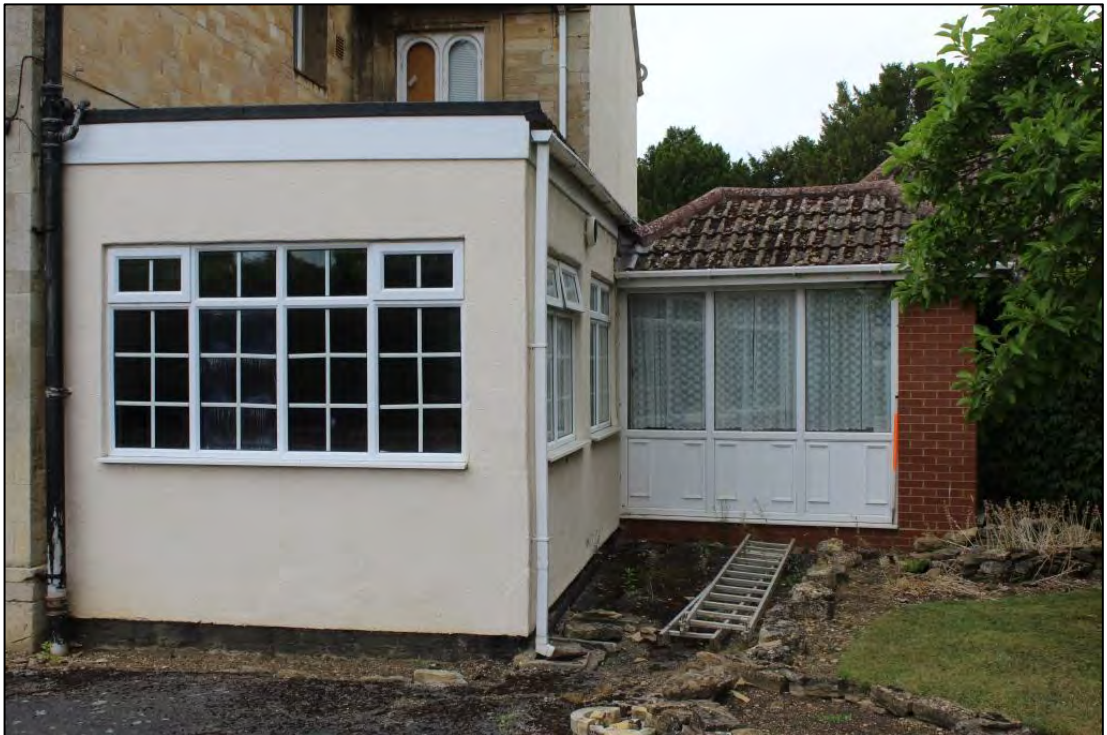
Photo 4: Eastern extensions to the building
