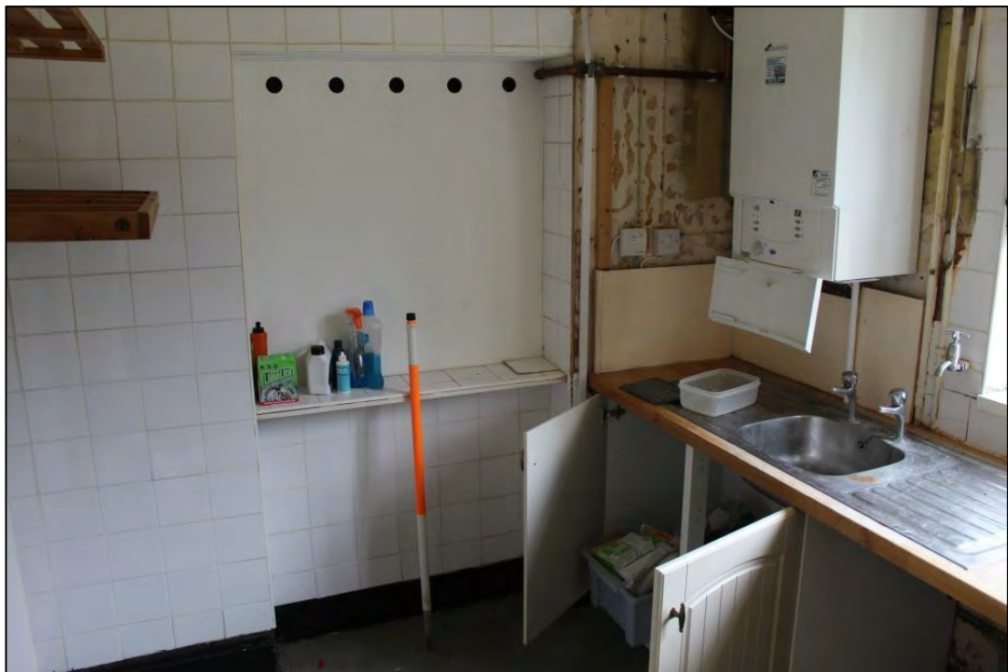
Photo 32: Overview of Room 14, looking north-west
