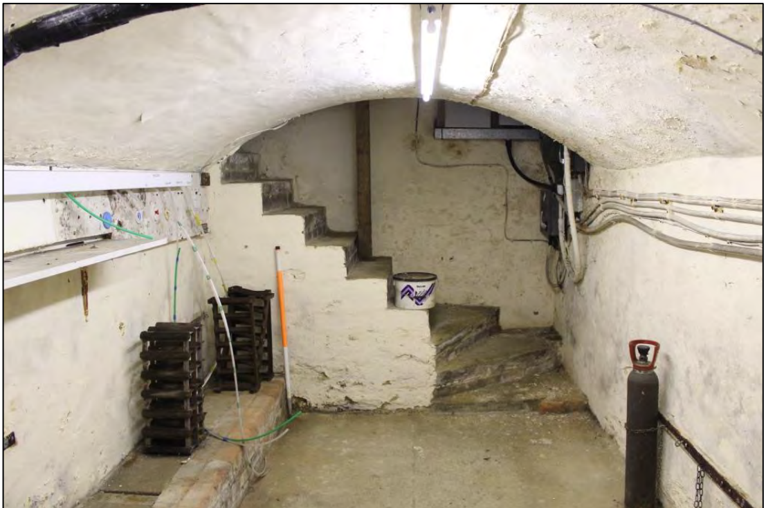
Photo A20: Room 52, looking south-west
