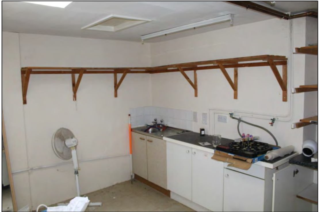
Photo A13: Room 18, looking north
