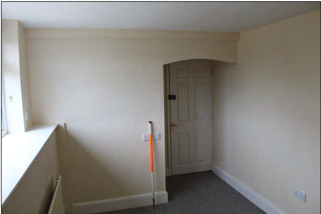
Photo A30: Room 46, looking south-east
