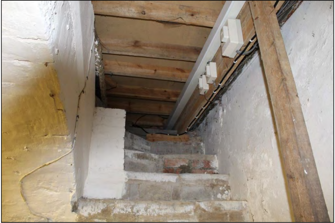
Photo 24: Former staircase leading to Room 5, viewed from within cellar (Room 52)
