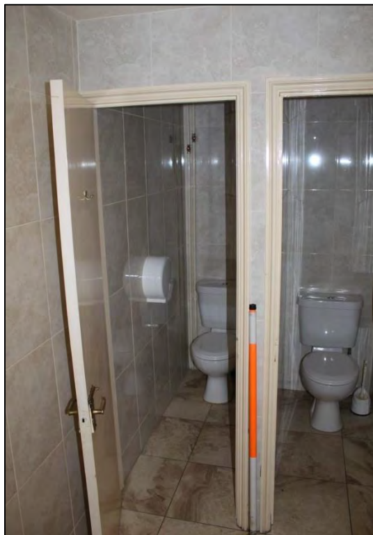
Photo A2: Room 3, looking south-east
