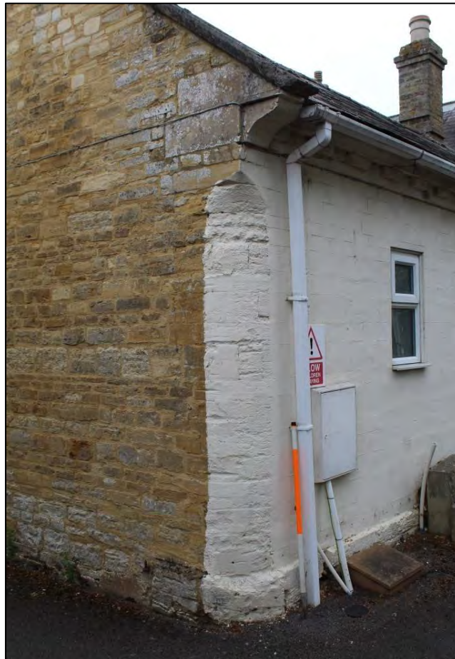
Photo 12: Detail of south-western corner of stables
