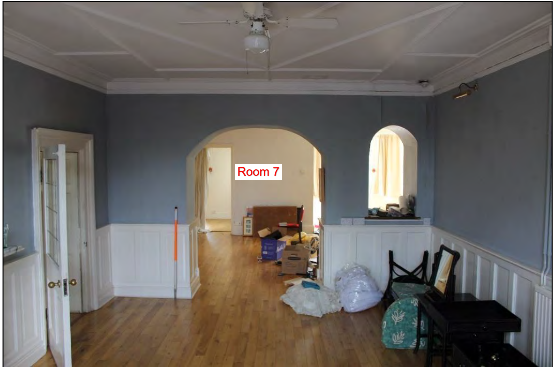
Photo 25: Overview of Room 6, looking north
