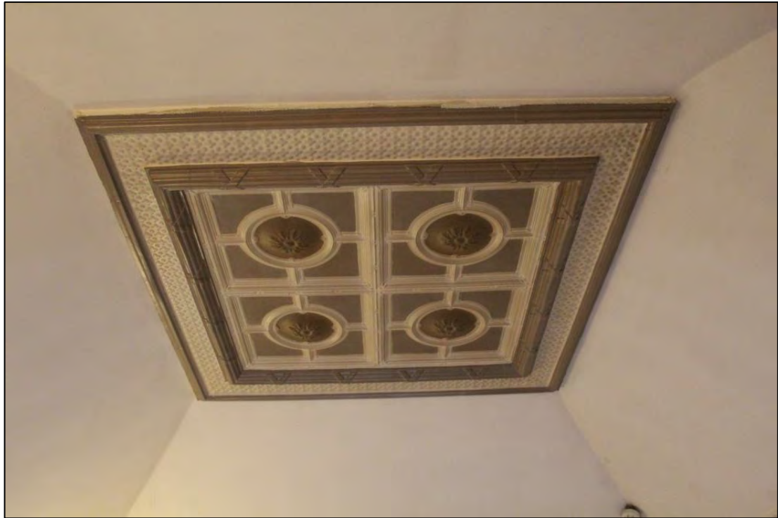
Photo 43: Detail of ceiling panel in Room 34
