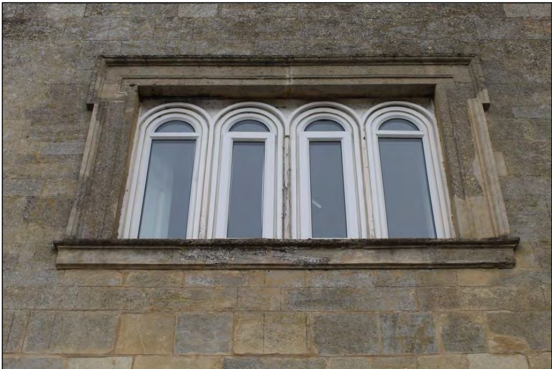
Photo 2: Detail of first floor window within southern elevation
