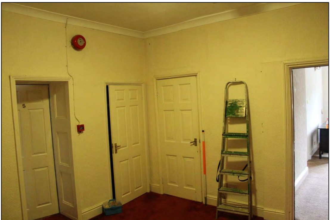
Photo A22: Room 35, looking north-west
