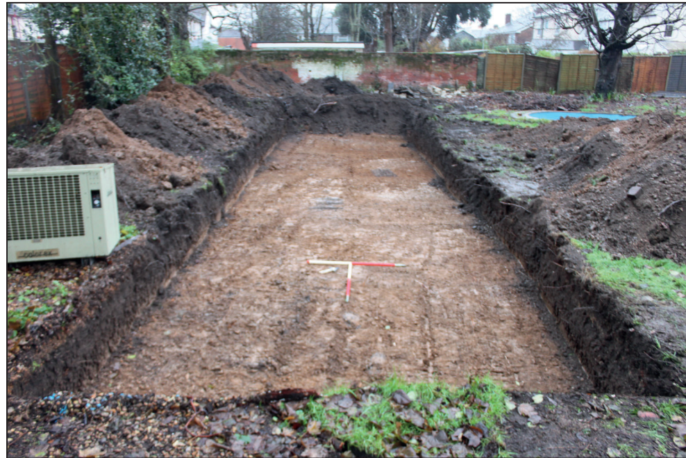
Watching brief area, looking north-west (1m scales)
