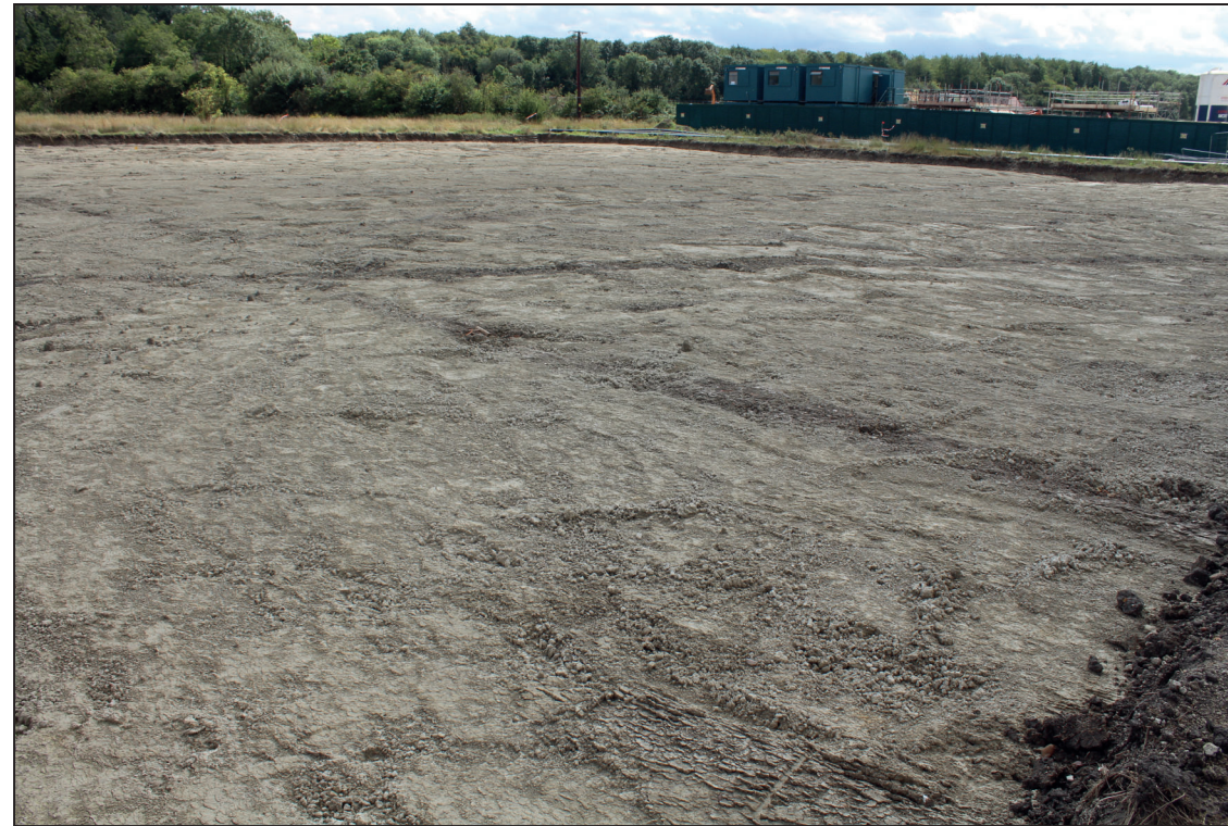
Overview of Area I, looking south-west
