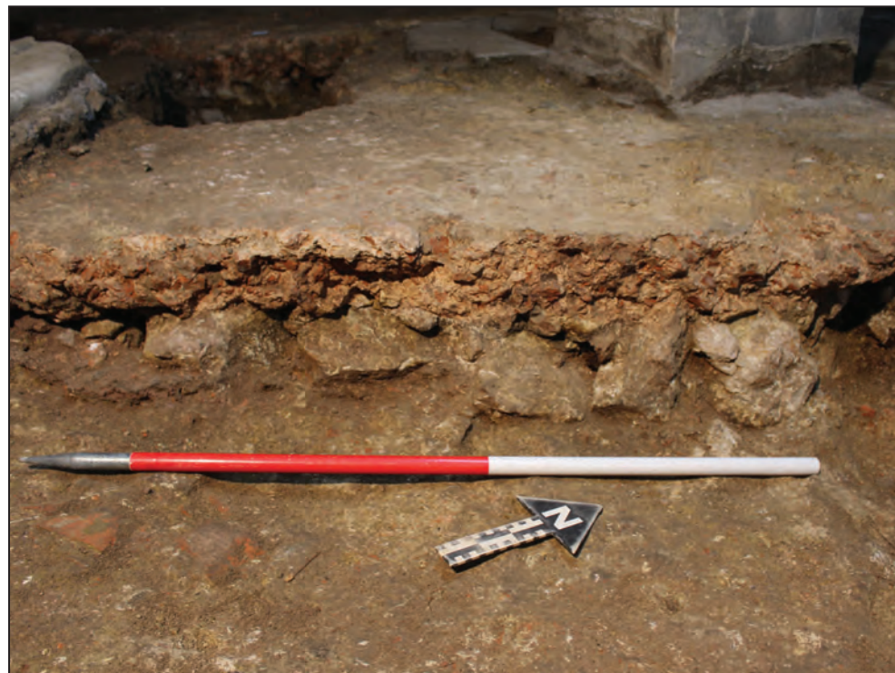
Photograph C: Opus signinum floor 183000/187035, looking north-west (1m scale)
