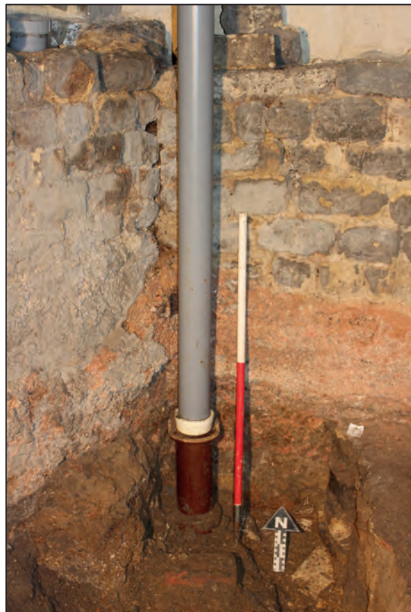
Photograph 1. Western butt joint of wall 2704, looking north (1m scale)
