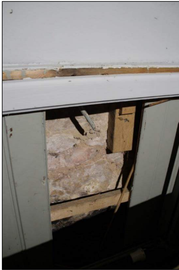
Photo 43 Stone masonry below modern tongue and groove wainscoting
