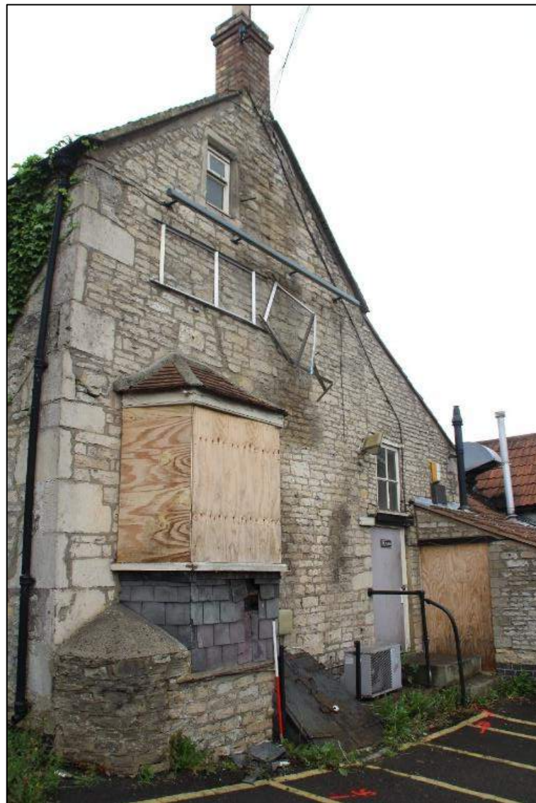
Photo 8 The northern elevation
