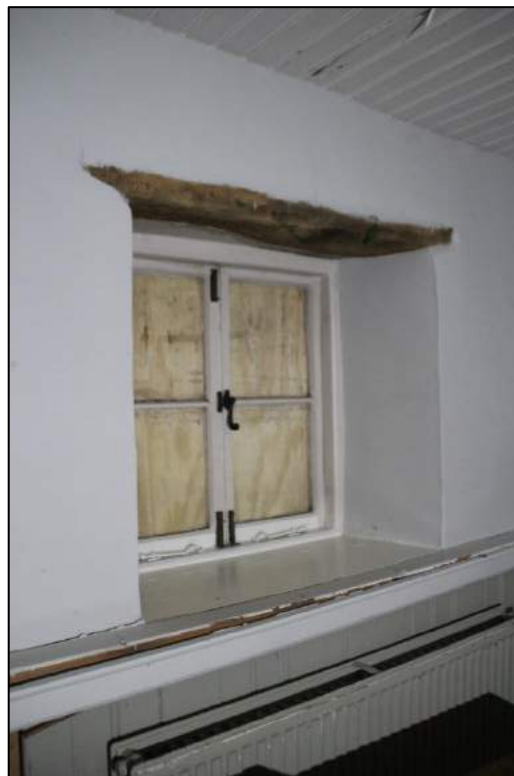
Photo 42 Window facing east in Room 8 with timber lintel
