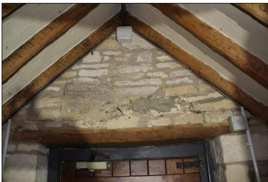
Photo 35 Detail of porch roof, looking east
