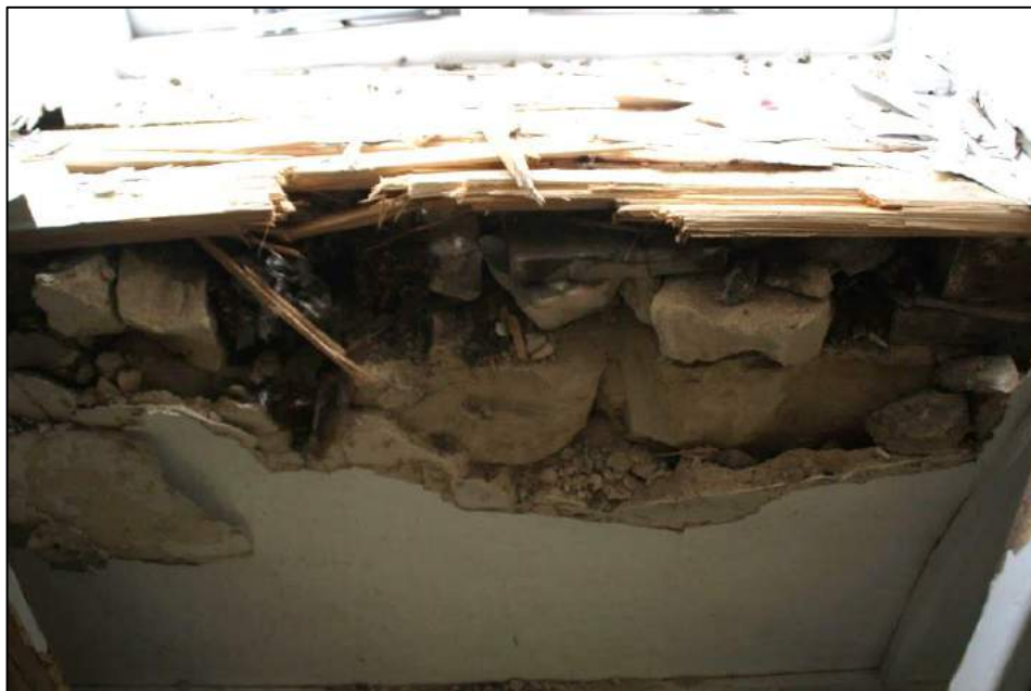
Photo 61 The window cill and masonry below in Room 14
