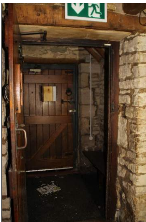
Photo 34 View of porch from Room 3
