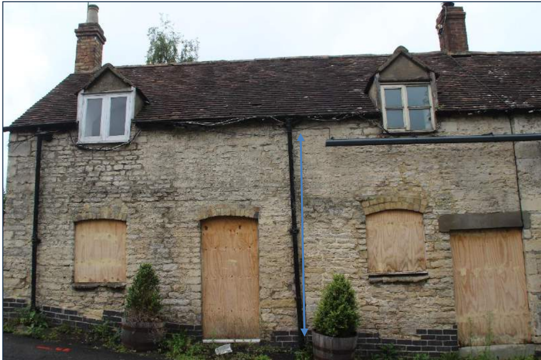
Photo 7 The southern section of the eastern façade (building junction annotated)
