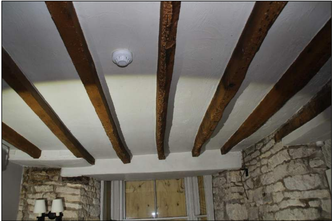
Photo 33 Detail of ceiling with exposed joists, Room 3
