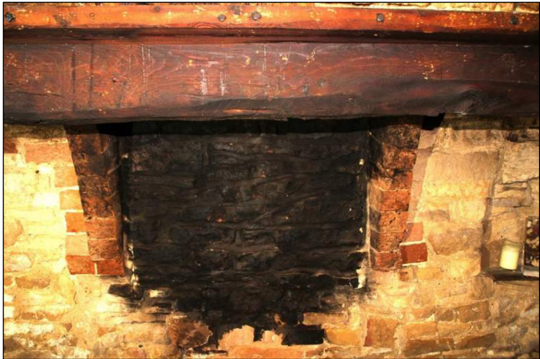
Photo 29 Detail of the fireplace lintel and brick consoles
