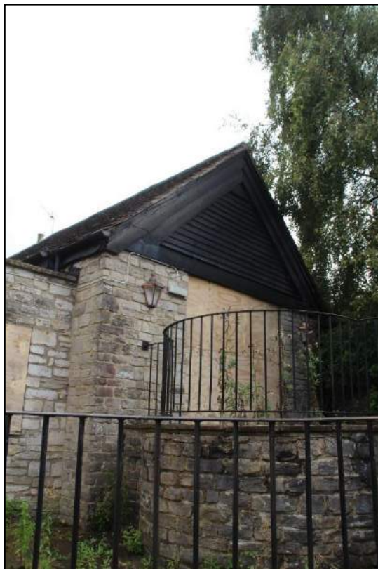
Photo 16 The 1996 entrance structure appended to the southern section of the historic Building
