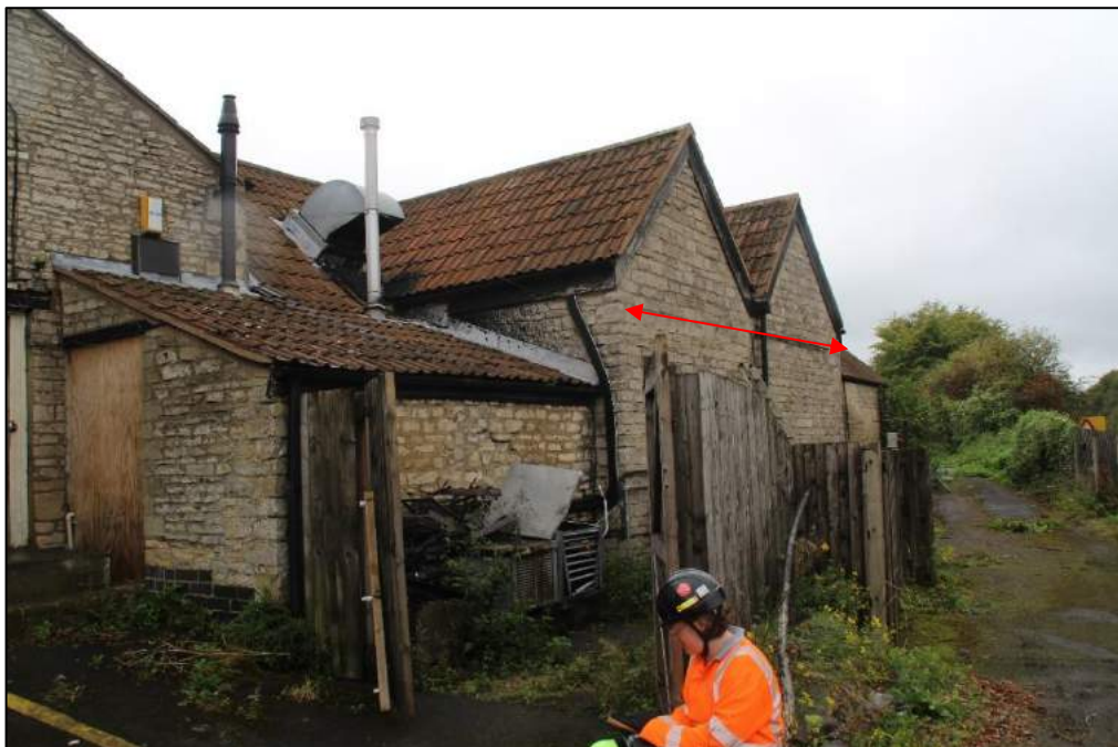
Photo 10 The two 1980s gabled structures (arrowed)
