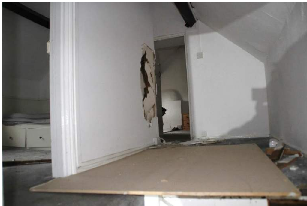
Photo 59 The upper lobby and Room 13 on the left
