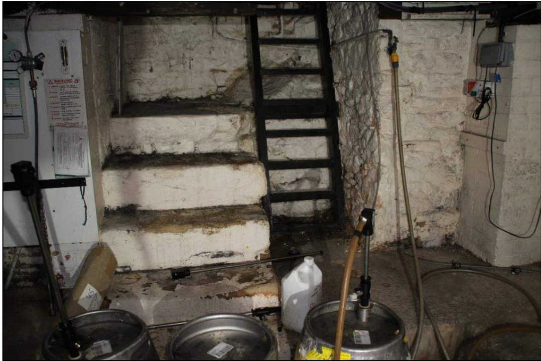
Photo 68 The southern wall of the cellar with infilled former stairway to the interior of the pub
