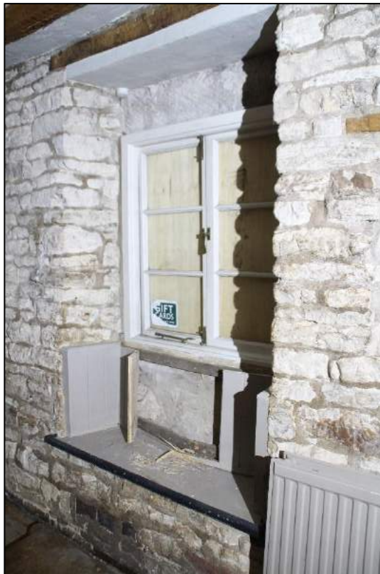
Photo 31 The north-western window in Room 3
