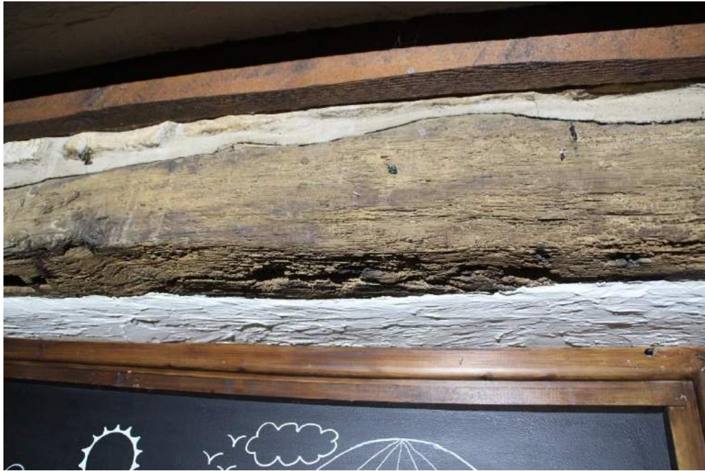
Photo 38 Historic reused timber in lintel of 1980s work
