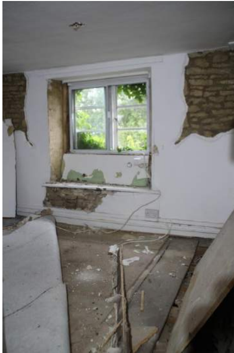
Photo 52 View of the window in Room 9
