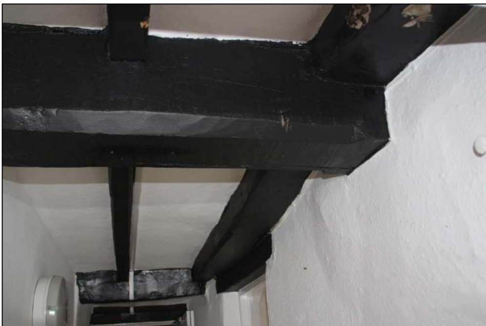
Photo 64 Section of a main beam, first floor corridor
