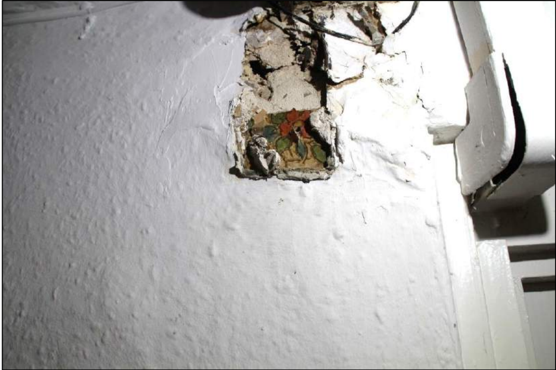
Photo 65 A remnant of historic wallpaper under modern wall coverings
