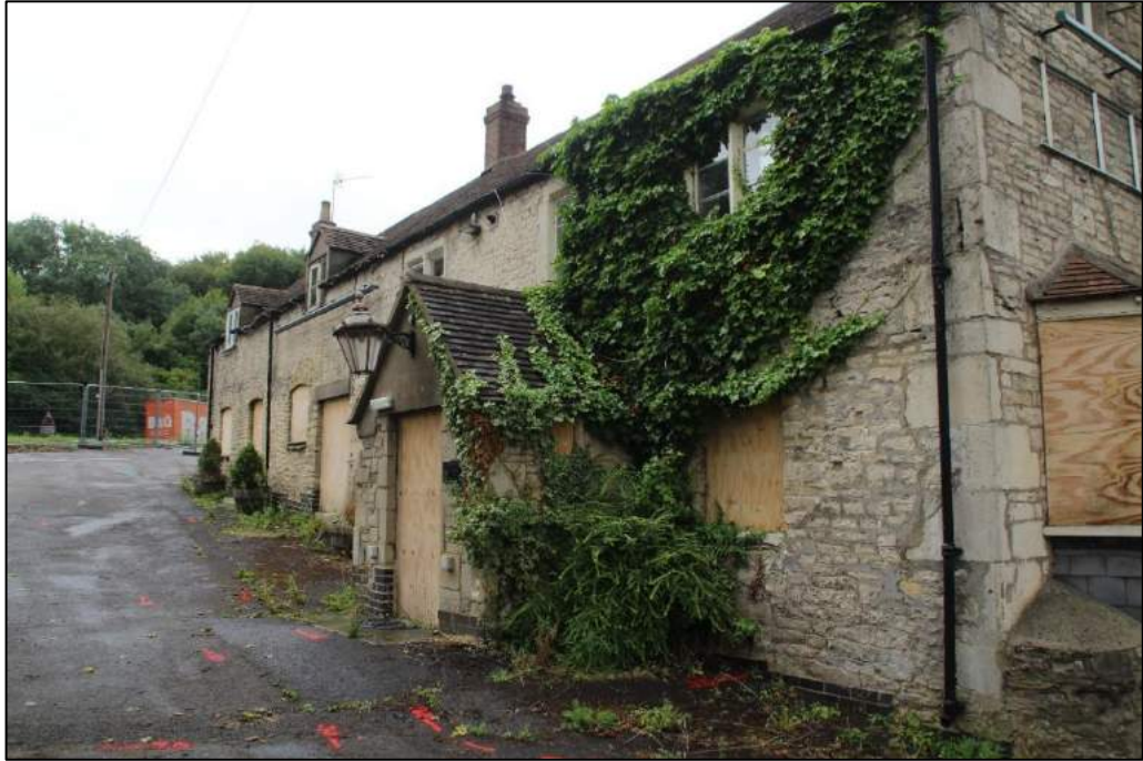
Photo 4 The front, eastern elevation, seen from the north
