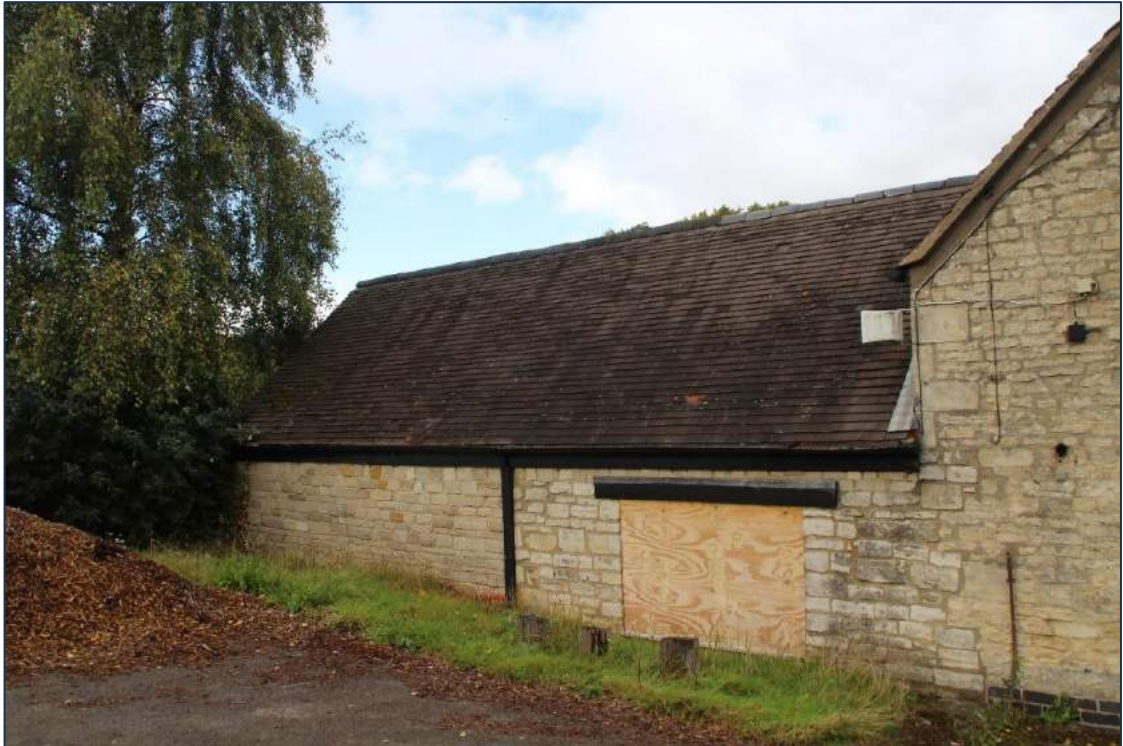
Photo 17 The western section of the southern elevation
