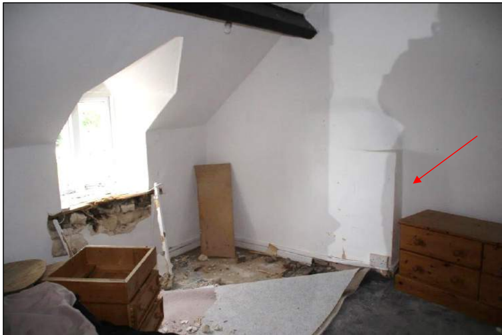
Photo 60 Room 14 with the gable linear feature, possible former fireplace
