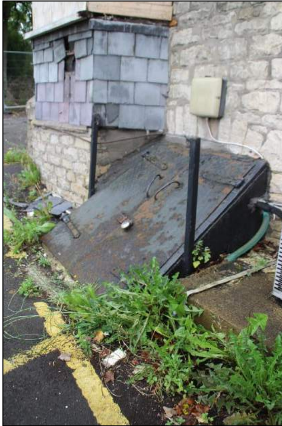
Photo 66 The cellar doors on the northern elevation
