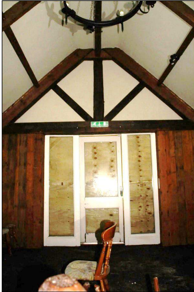
Photo 40 View looking west in the 1990s entrance hall
