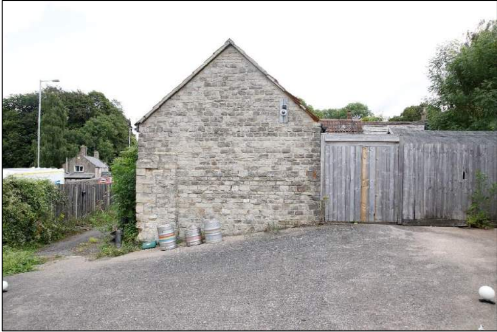
Photo 12 The western elevation of the east-west wing
