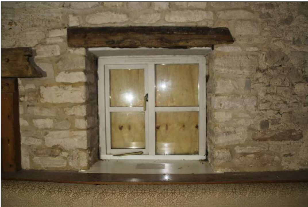
Photo 47 The east window in Room 7
