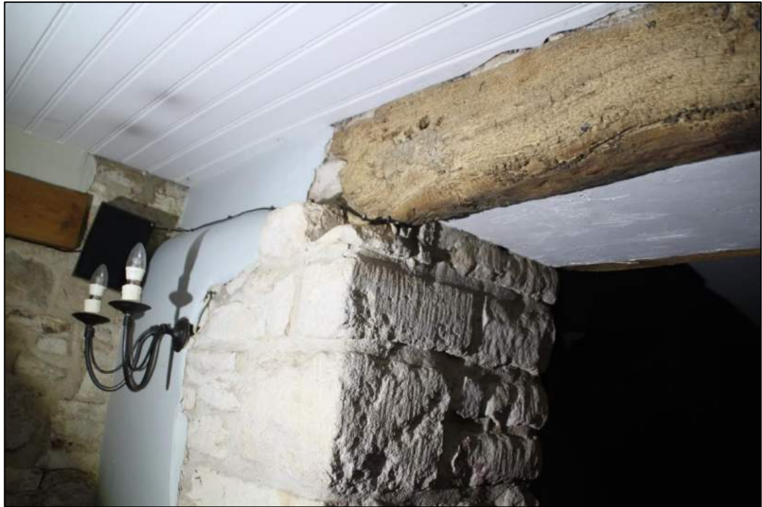
Photo 45 The opening between Rooms 7 and 8
