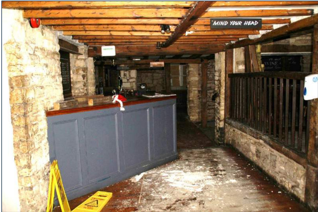
Photo 23 View looking east in Room 2
