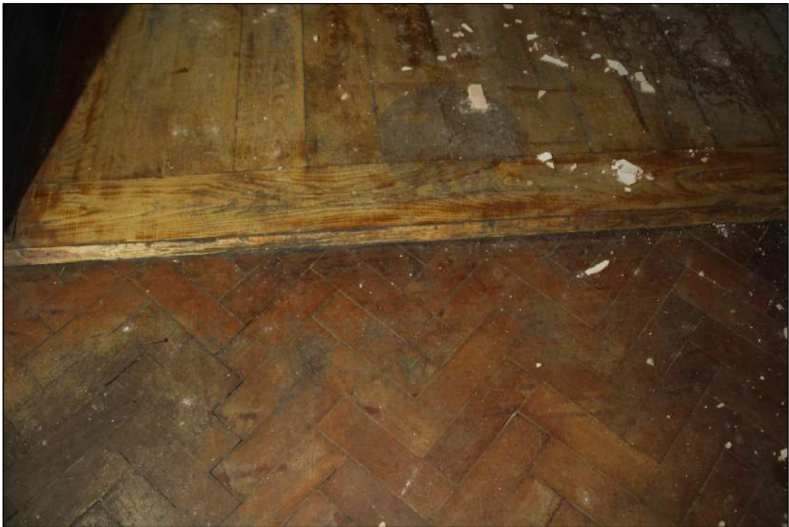
Photo 27 The flooring change in Room 3
