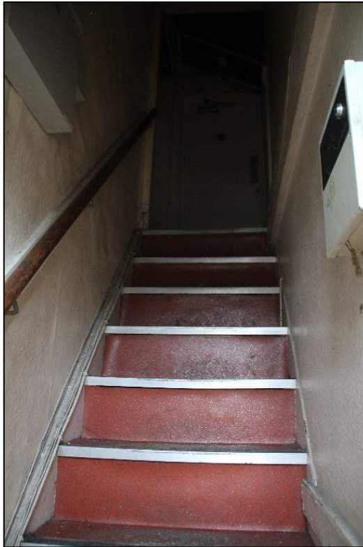
Photo 49 The stairs accessing the first floor
