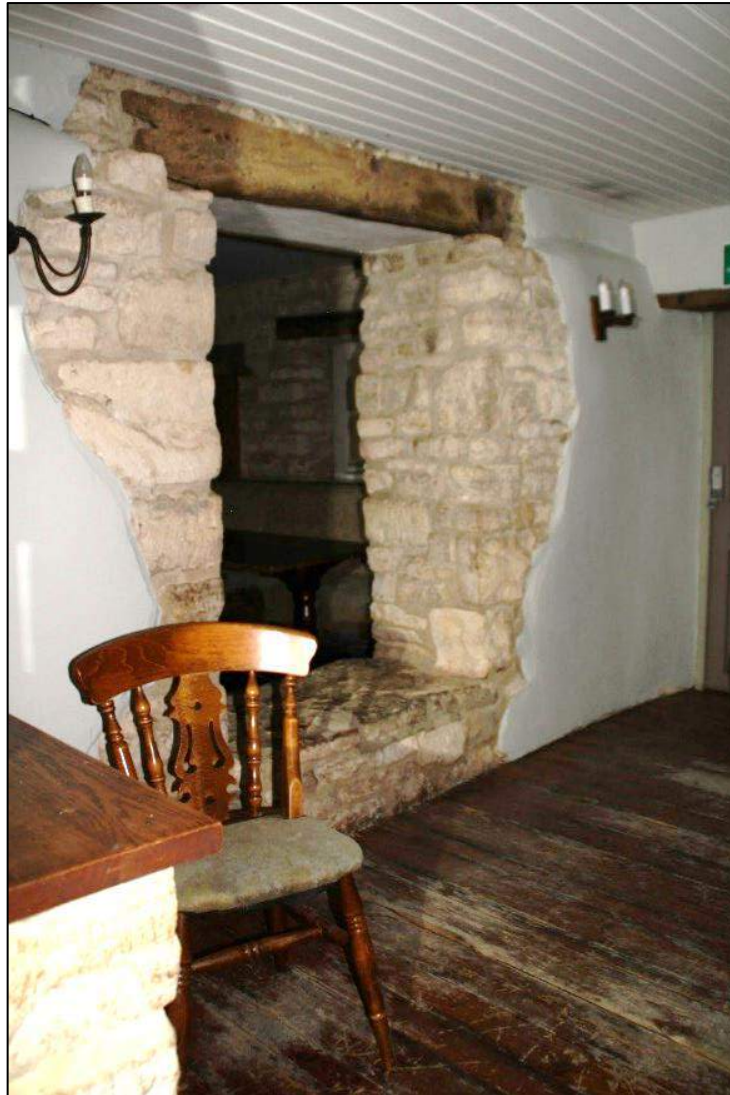
Photo 44 The opening between Room 7 and Room 8
