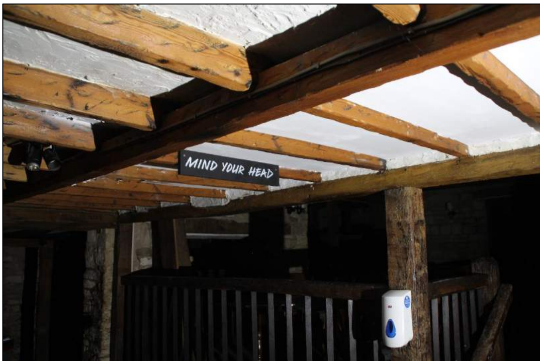
Photo 24 View of new distressed timbers in Room 2, constructed late 20th century
