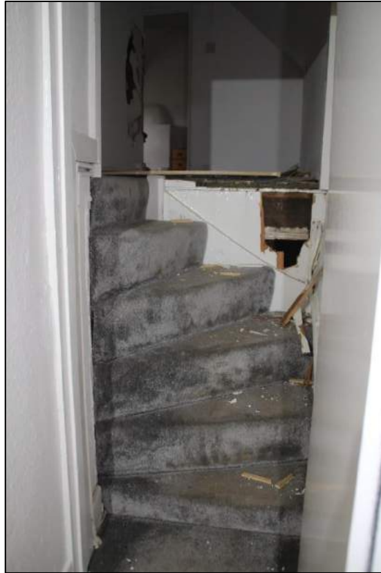
Photo 58 The small flight of stairs to Rooms 13 and 14
