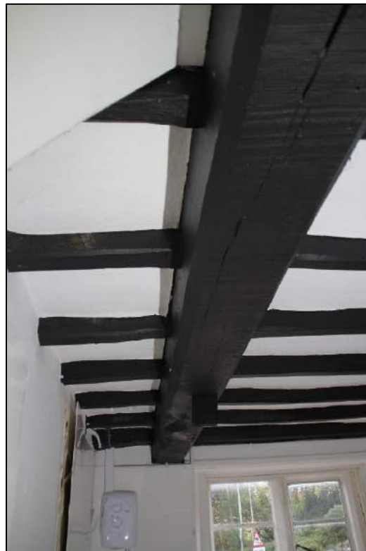
Photo 56 View of beam and exposed joists, Room 11
