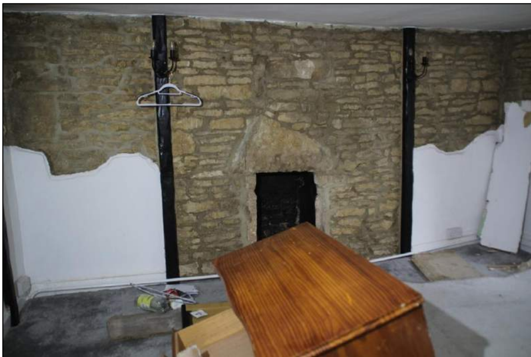
Photo 51 The northern room, first floor, looking north
