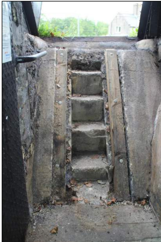
Photo 67 The cellar stairs with barrel slope
