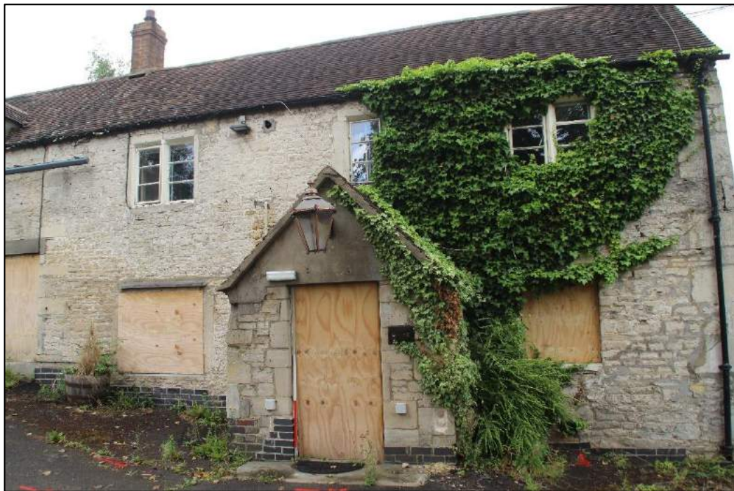
Photo 5 The front, eastern, elevation, seen from the east
