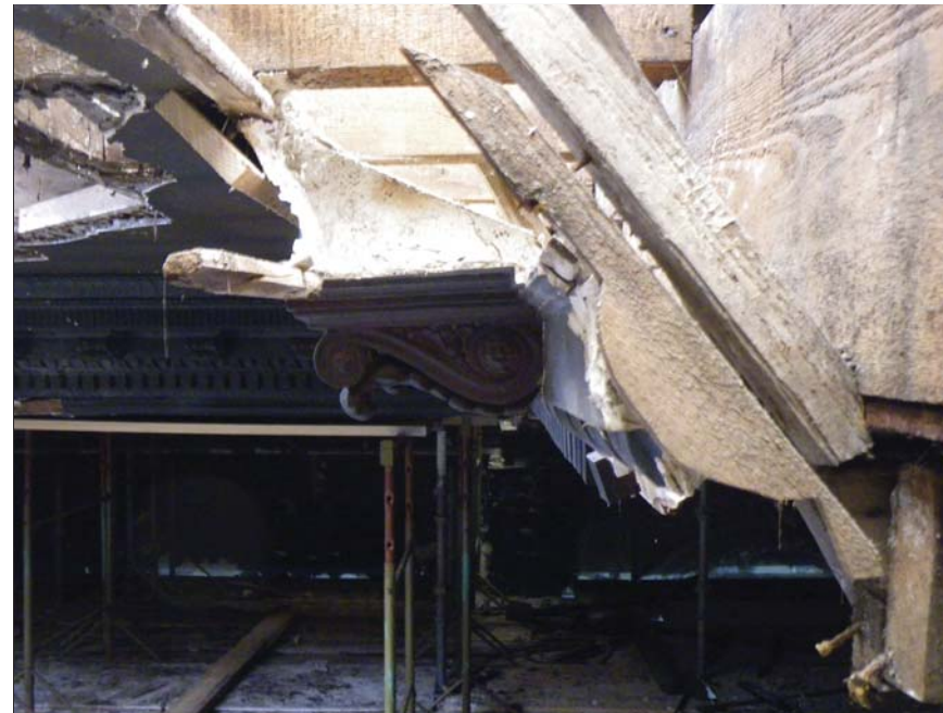
10 Detail of typical plasterwork attachments
