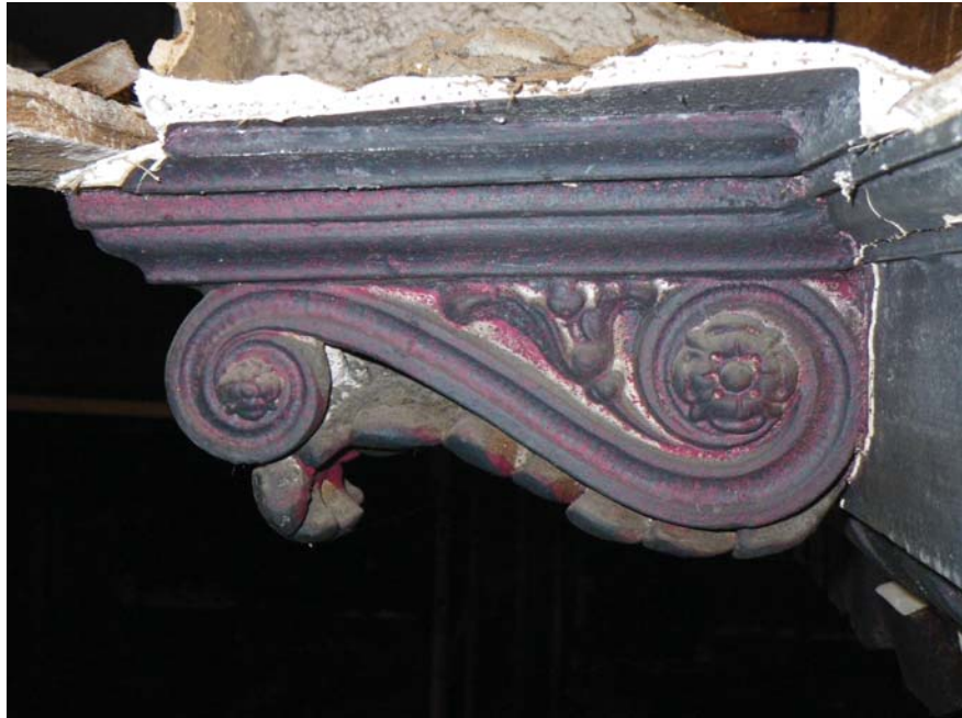
12 Detail of side of console bracket on ceiling beam
