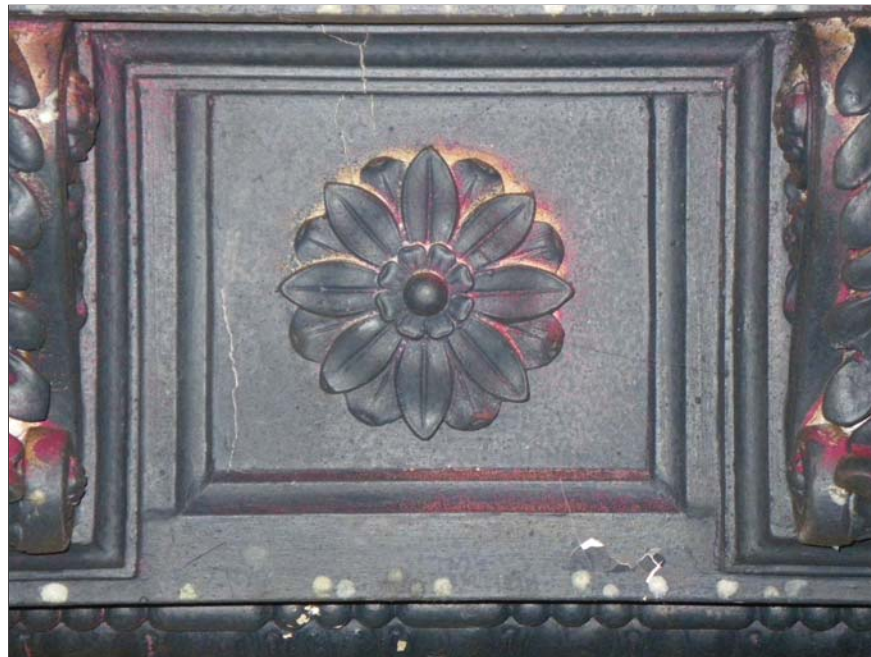
15 Detail of rose between console brackets on ceiling beam
