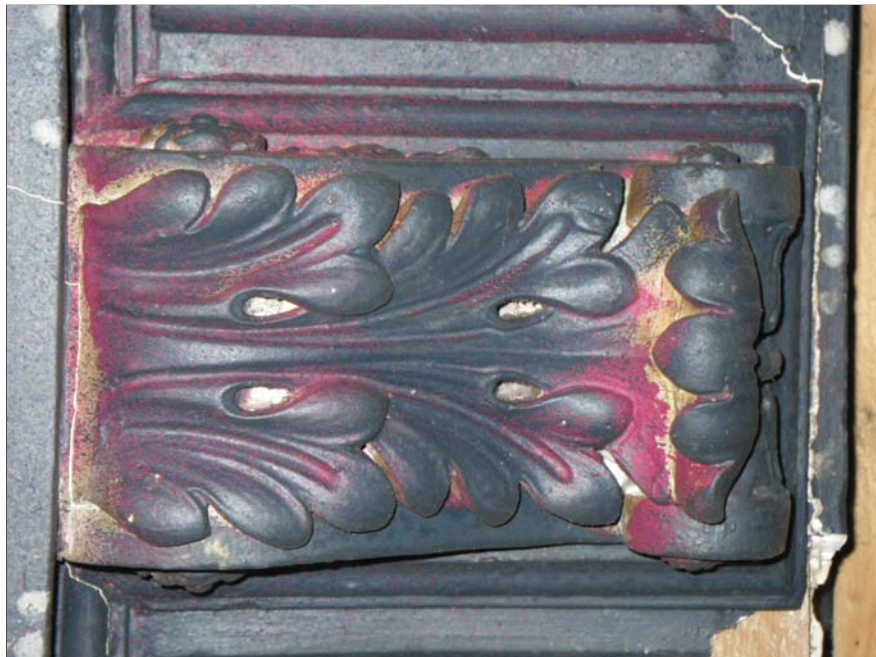
14 Detail of underside of console bracket on ceiling beam
