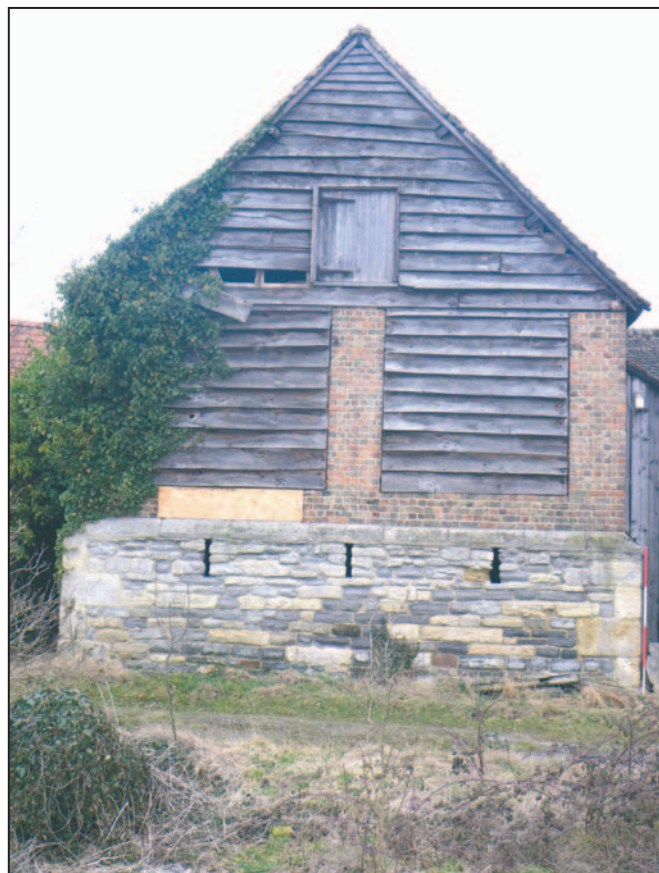
6 West elevation of Building 1, looking north. Scale 2m.
