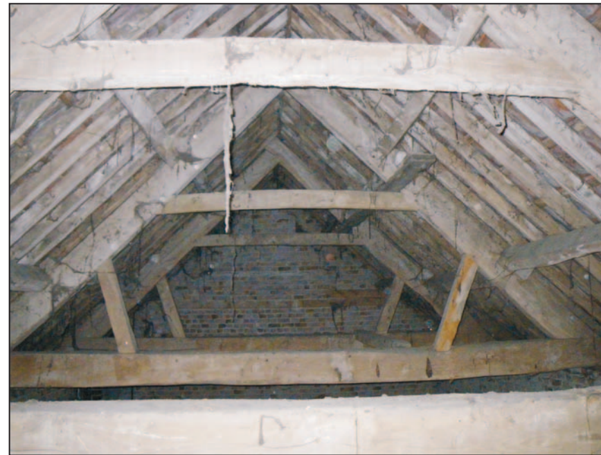
22 The roof structure in Building 2, Room 7, looking north.
