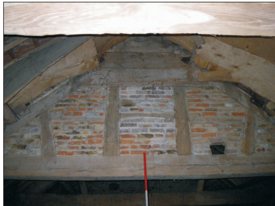
23 The in-filled Truss in Room 8, Building 3, looking north. Scale bar 0.5m.
