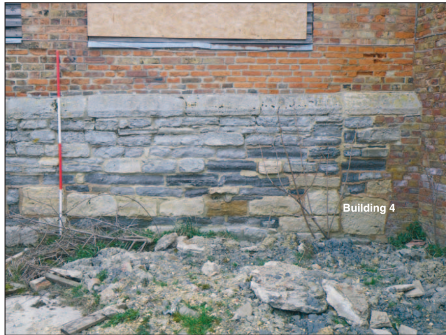
14 Fragment of Building 4 between Buildings 1 and 2, looking north-west. Scale 2m.
