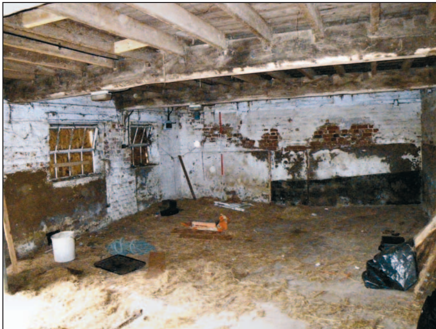
19 Room 1 in Building 2, looking north-west. Scale 2m.
