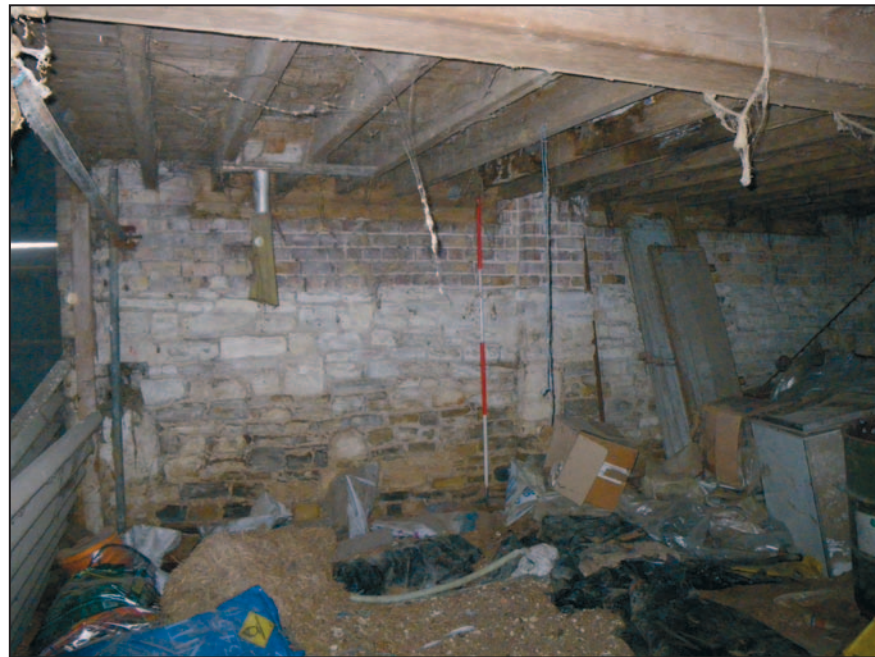
10 Interior of south wall of Building 1, looking south-west. Scale 2m.
