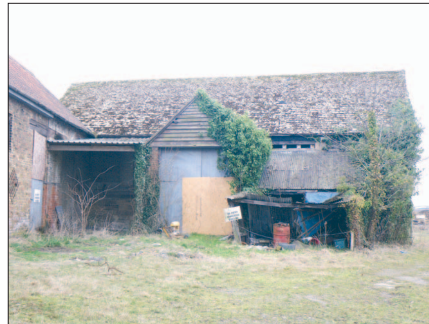
32 The lean-tos against the north side of Building 1, looking south.
