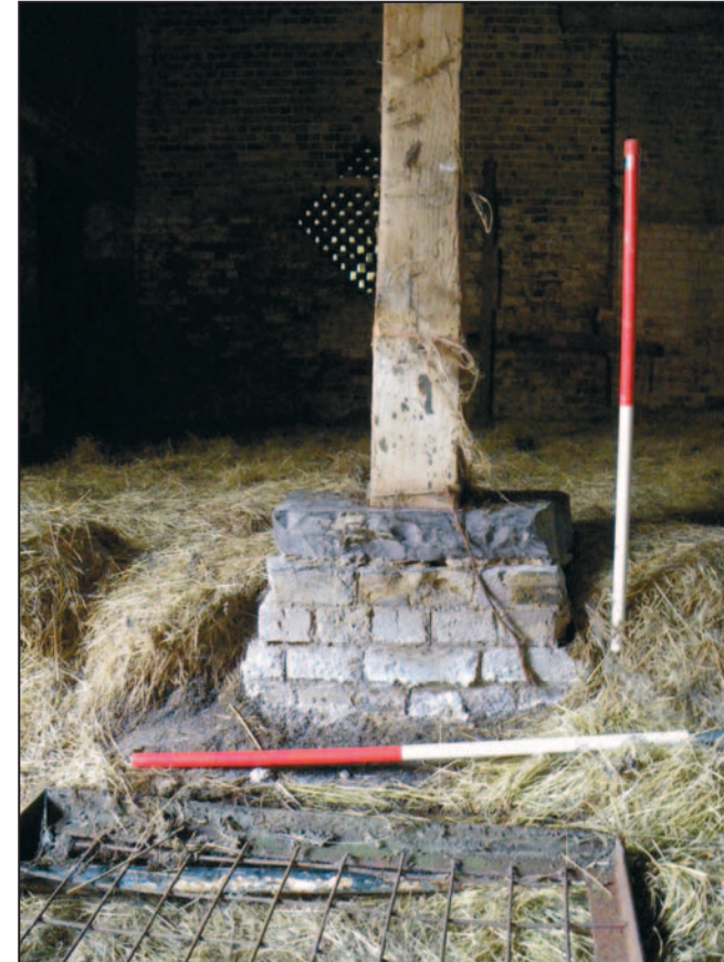
30 Fragment of east wall of Building 2 used as base of one of the southern arcade posts of Building 2/2a, looking west. Scales 1m.
