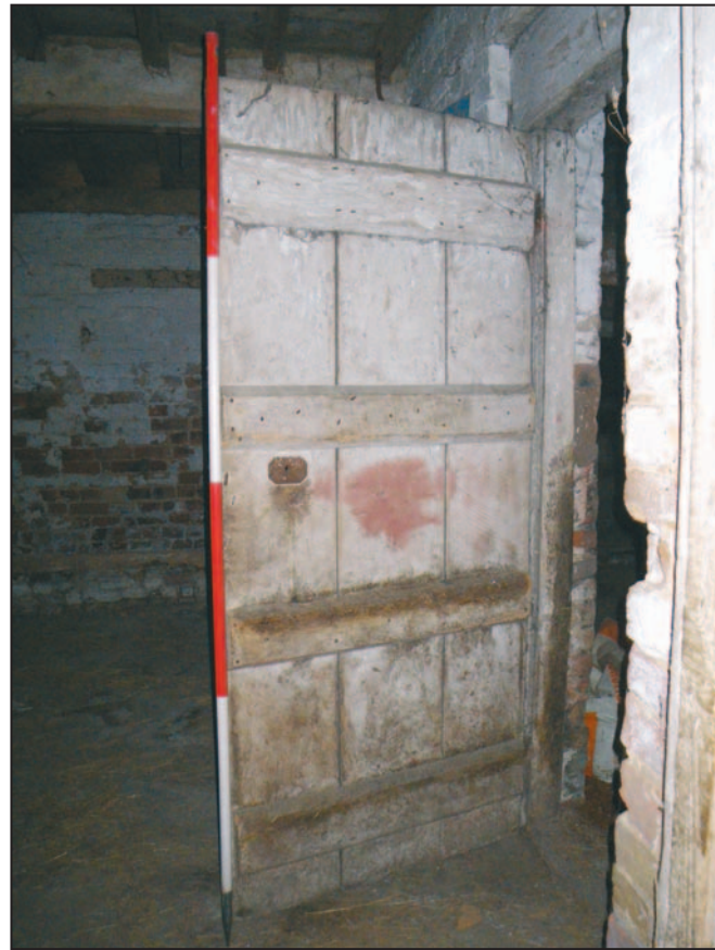
21 The early ledger door in Room 3. Scale 2m.
