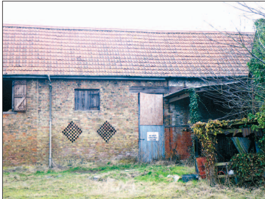
27 The west elevation of Building 2 and its junction with Building 3.
