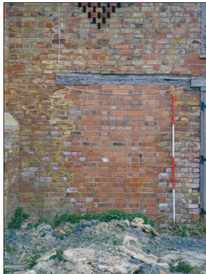
31 The blocked-in doorway in the south gable end of Building 2, looking north. Scale 2m.
