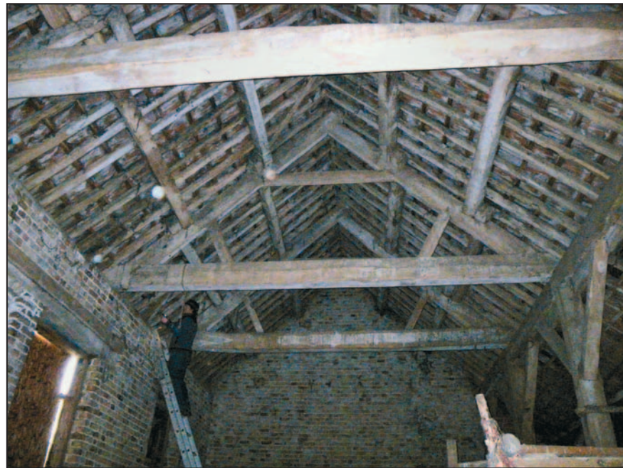
29 The roof timbers of Building 2, looking north.
