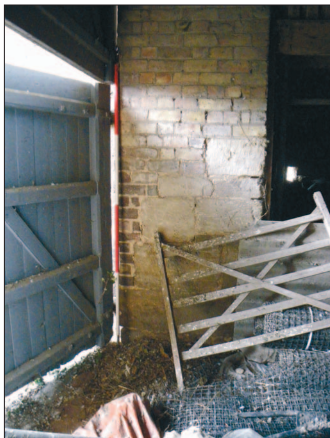
8 Quoins to the south entrance in Building 1, looking west. Scale 2m.
