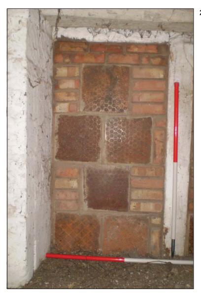
27 Two types of malting kiln floor bricks used to block windows in the stair tower in Building 1. Scales 1m
