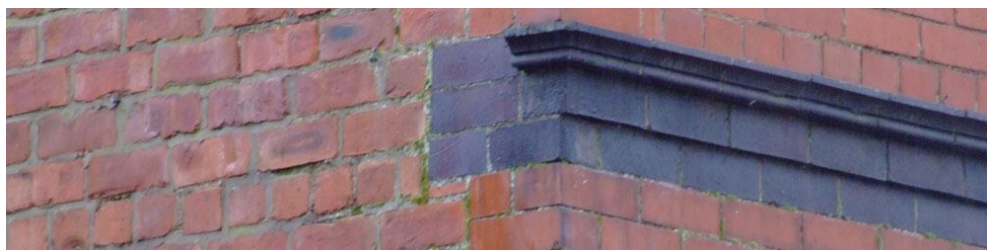
PLATE 9:BLACK GLAZED BRICK CORNICE DETAIL ON SOUTH FASCADE
