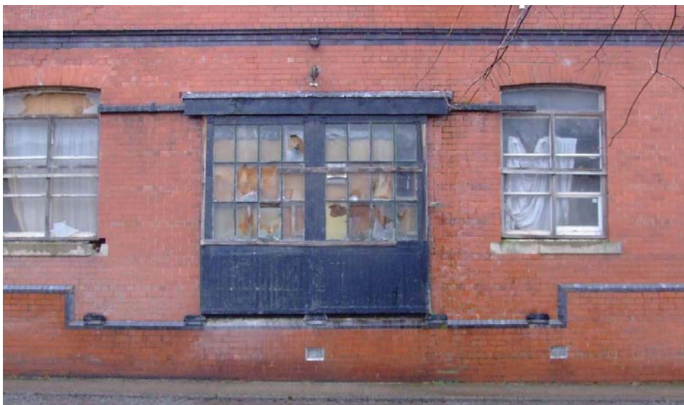
PLATE 7: CENTRAL GOODS DOOR, TYPICAL WINDOW AND PLINTH - SOUTH ELEVATION
