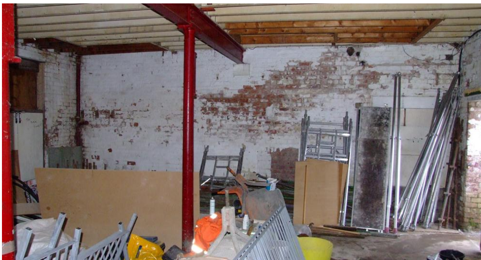
PLATE 15: ROOM 3 SHOWING SANDSTONE CORBEL FOR I-BEAM SUPPORT AND CONCRETE FLOOR - WEST
