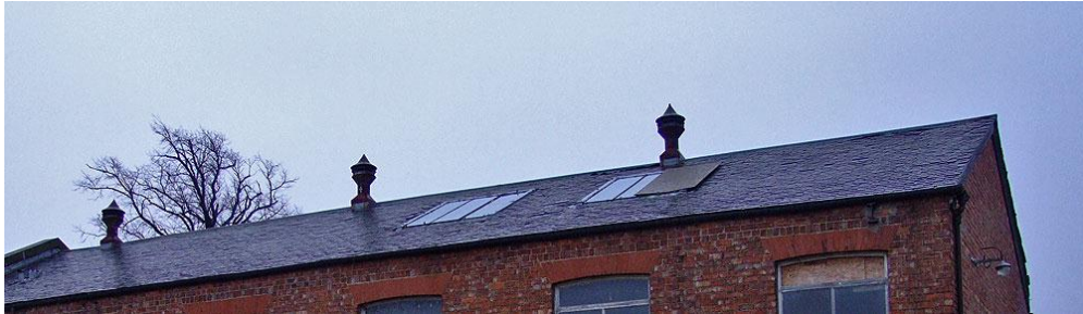
PLATE 13: SLATE ROOF. ROOF LIGHTS AND VENTILATION COWELS
