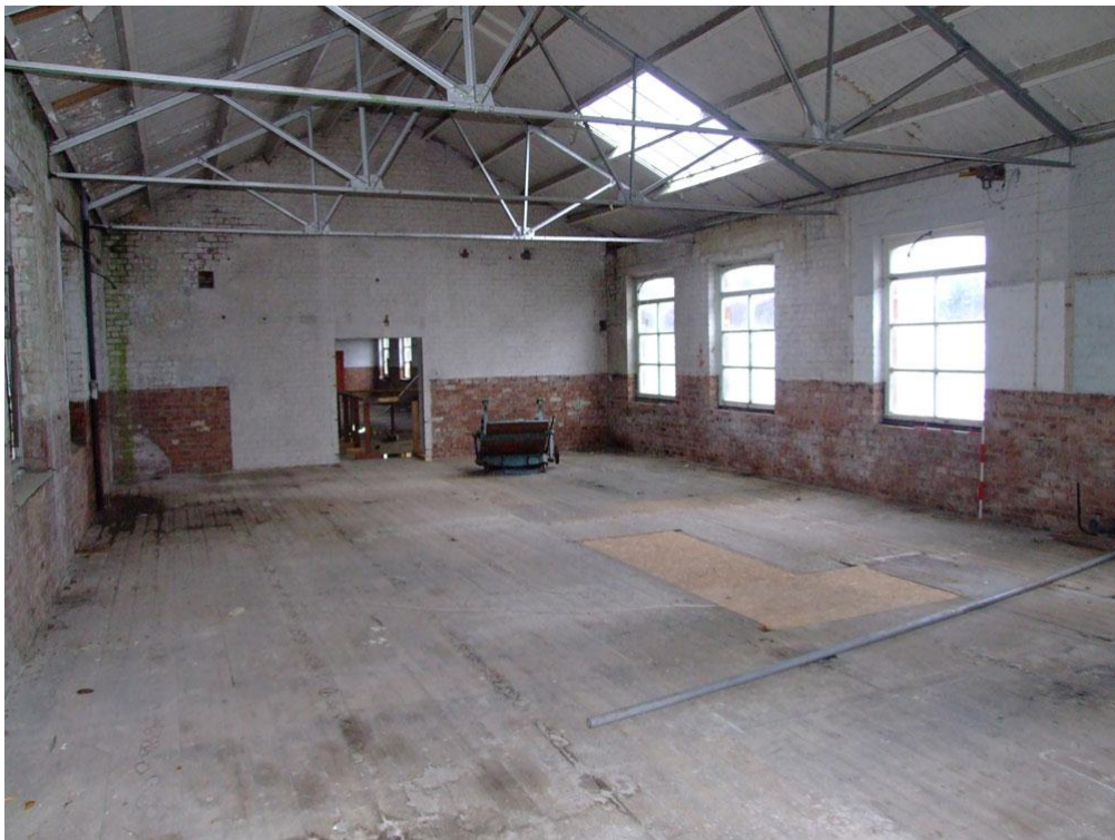
PLATE 19: ROOM 2 WITH ROOM 1 BEYOND. NOTE FLOOR SCARS OF INTERNAL DIVISIONS AND LOCATION OF STAIRS TO GROUND FLOOR ( COVERED IN NEW BOARD) ABOVE IS THE CAST IRON CANTILEVER TRUSS ROOF SUPPORT
