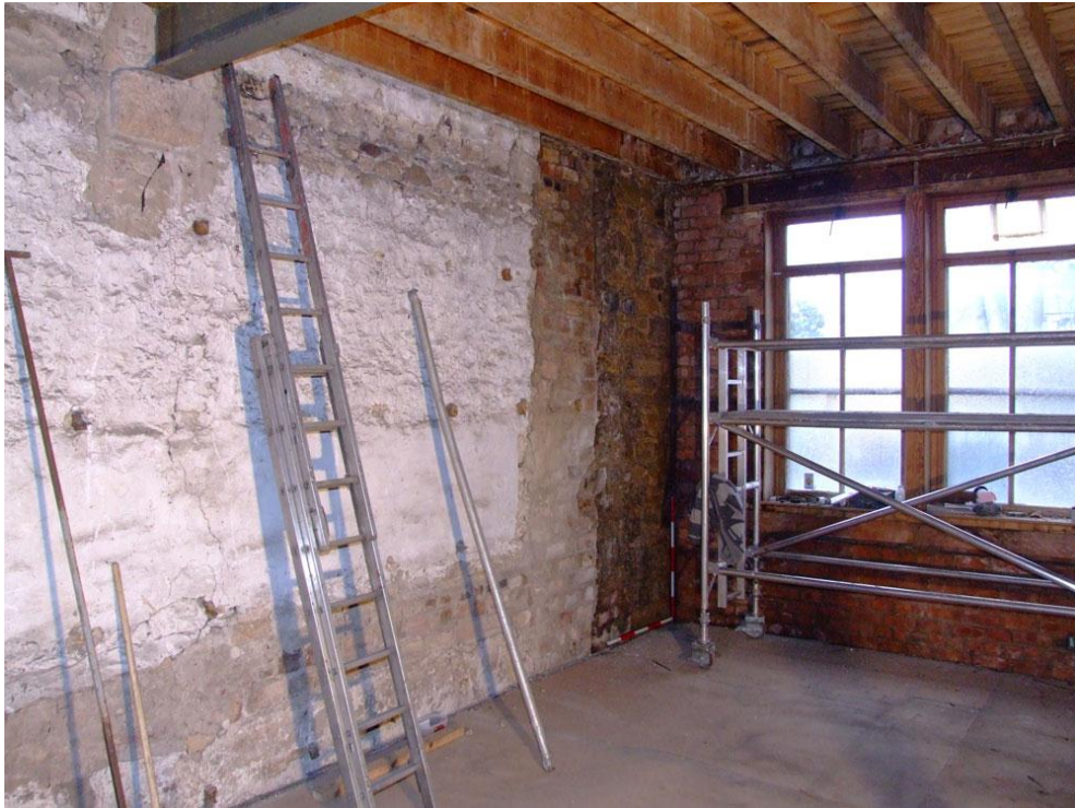
PLATE 17: INTERIOR - SHOWING READR WALL OF COTTAGE AND REPAIRED FLUE IN BRICK.
