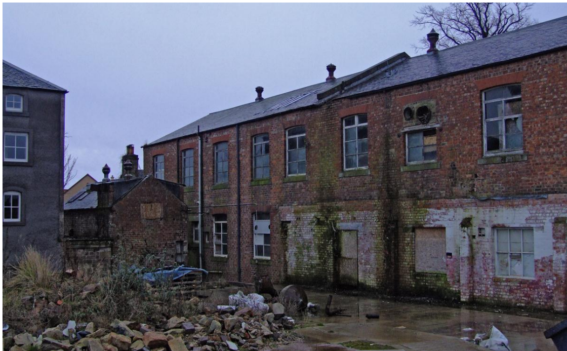
PLATE 3: REAR ELEVATION OF CHEVIOT HOUSE MILL, WITH THE WEST MILL TO THE LEFT AND BETWEEN THE TWO STRUCTURE THE PATERSON MILL ENGINE SHED. THE MILL LADE RUNS THROUGH THE SITE, BENEATH THE COURTYARD.
