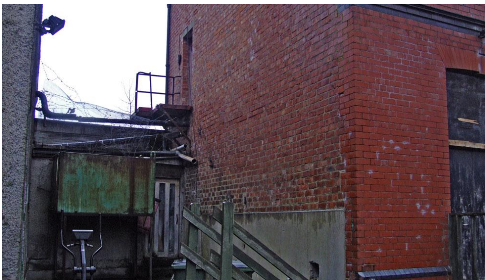
PLATE 12: WEST GABLE, WITH STAIRWAY SCAR AND 1ST FLOOR FIRE EXIT.
