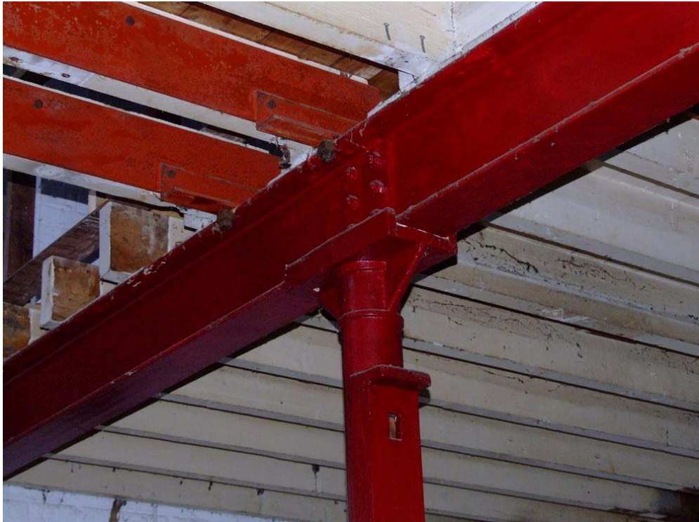
PLATE 14: DETAIL OF PILLAR CAPITAL, WITH FITTING AND ADDITIONAL FLANGES. NOTE UPPER ADDITIONAL TRUSS SUPPORTS TO LEFT.
