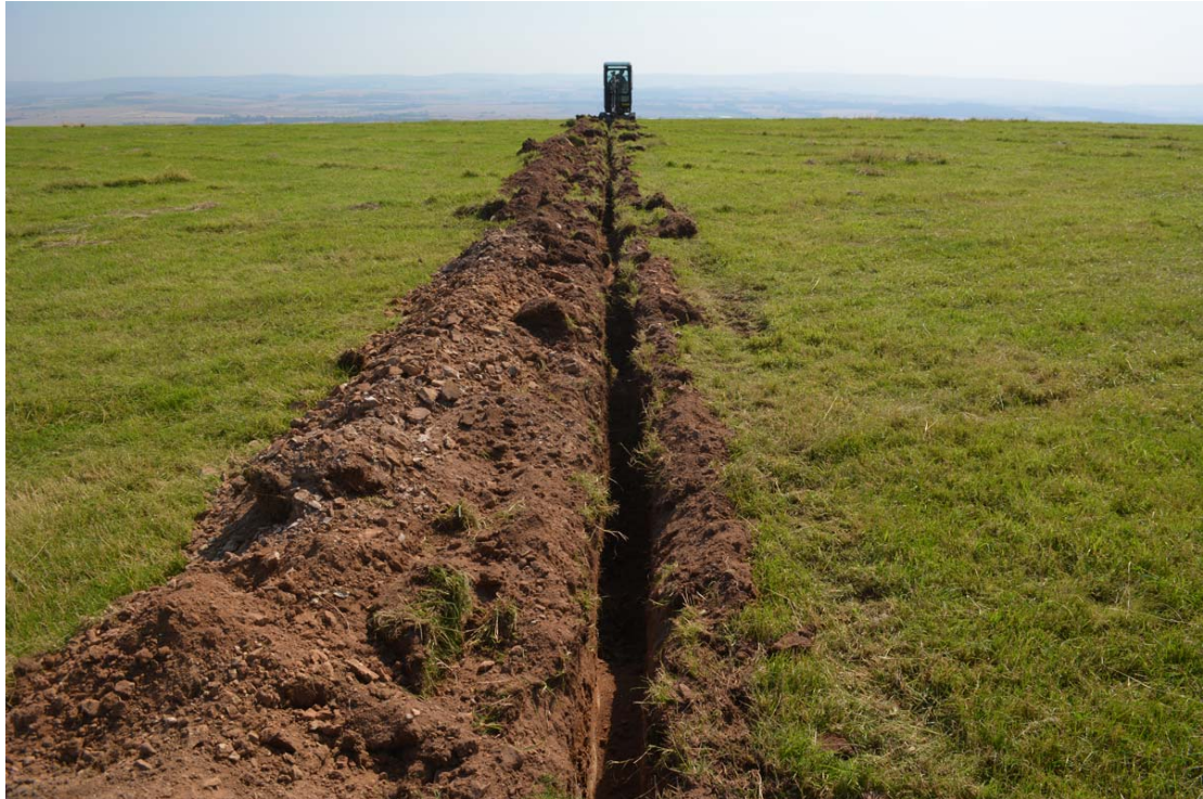
Plate 2 – Cable Trench – post excavation
