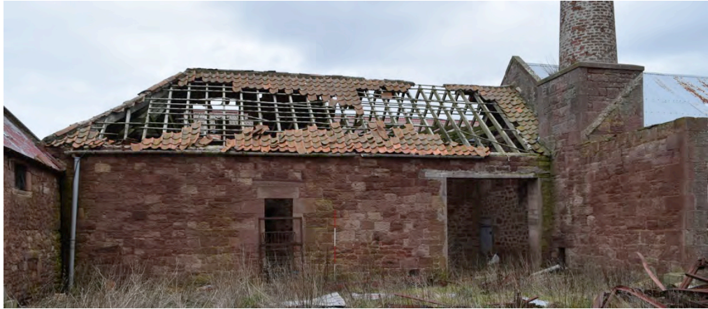
Plate 6: Yard 2; west exterior range– with partially collapsed pantile roof; wide entry and a tall window.
