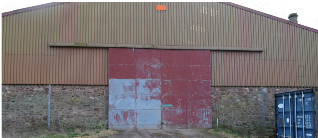
Plate 2: Yard 2— view of portion of the north exterior elevation, with wide entry and coursed rubble wall.
