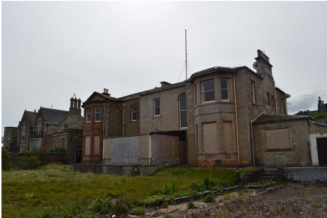
Plate 3: The rear North elevation with later 1895 extension (note pedimented façade) and later canted bay in red sandstone to left; original build centrally and single-story west wing to right.
