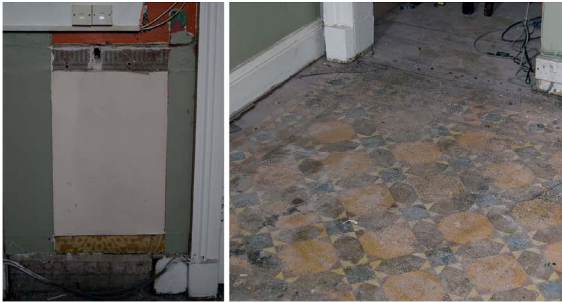
Plate 7: Room 3– detail of decorative paint scheme (left) and floor tiles (right).
