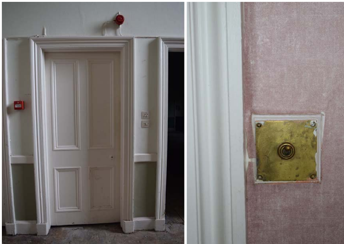
Plate 13: Left—Typical door surround; right—earlier 20th century brass light switch in Room 42.
