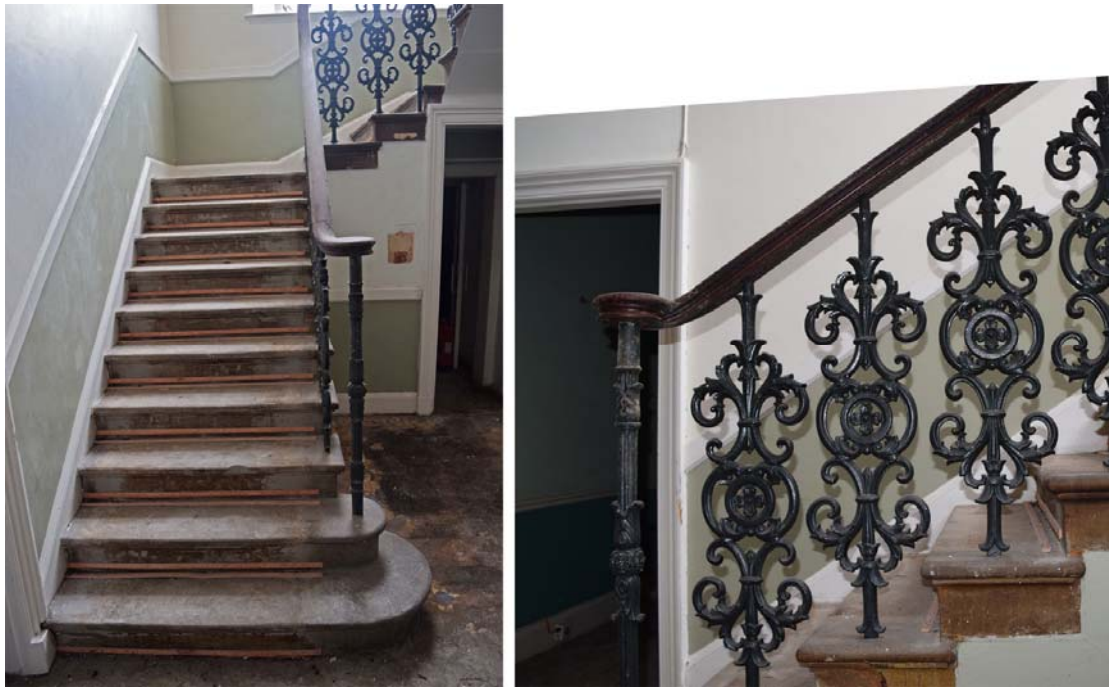
Plate 6: Left, Main stairs (Room 7); right, detail of ornate ironwork on the main staircase.
