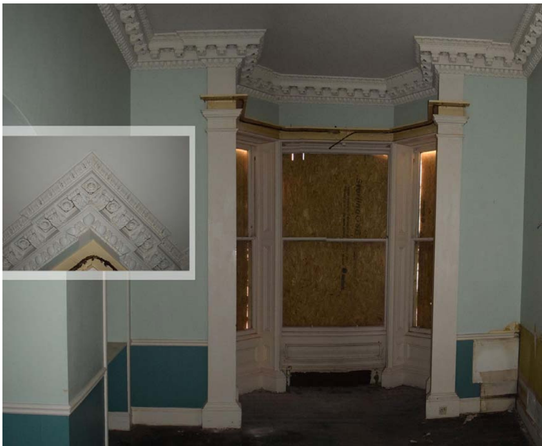
Plate 8: Room 6, detail of the south elevation, with canted bay and decorative surrounds; inset– detail of ornate cornice.
