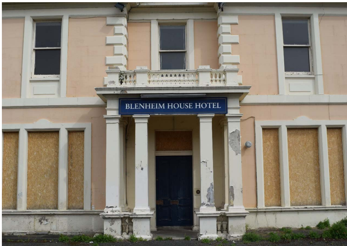
Plate 5: Detail of the exterior porch (Room 1) on the principal south elevation.
