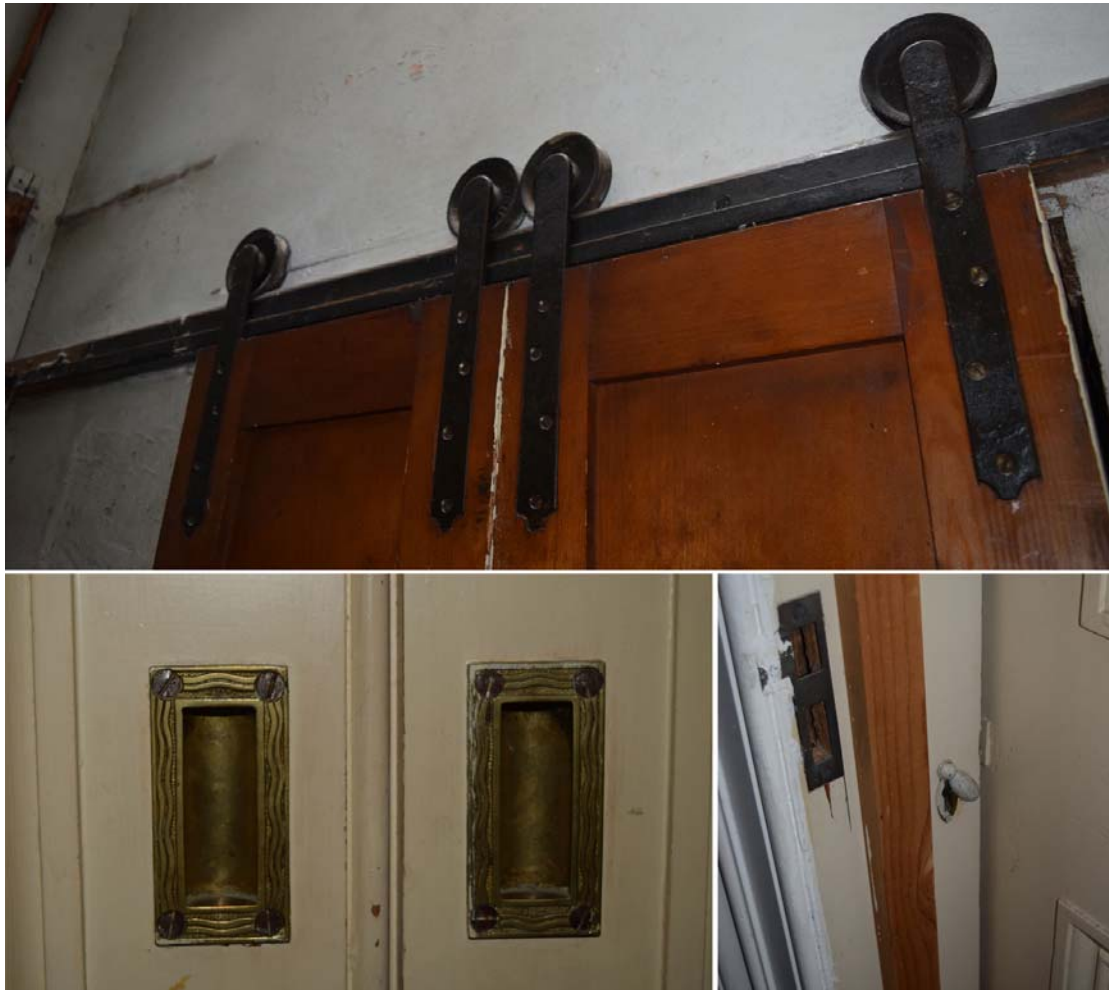
Plate 10: Room 51, with cast iron hanging rollers, inset brass door fittings and side mounted locking.
