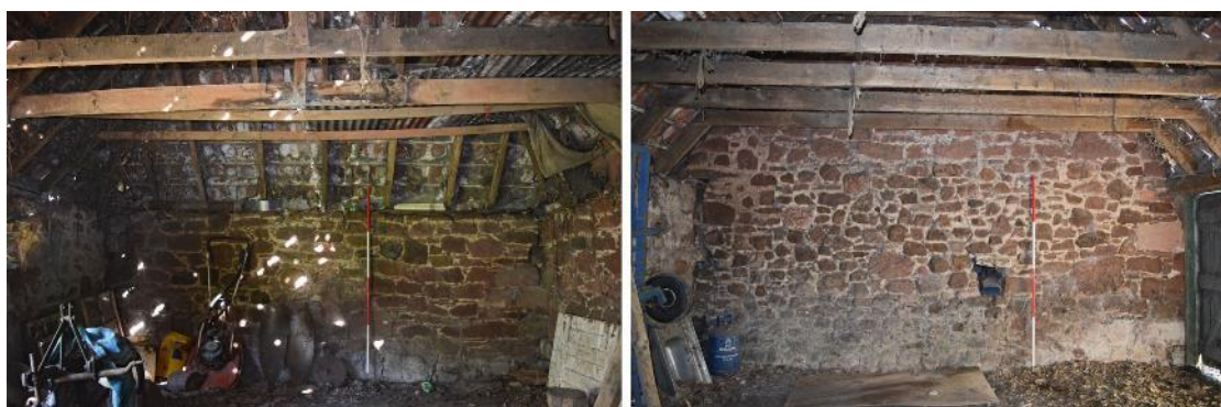
Plate 41: Room 3.1, Left– N elevation formed by boundary wall; with sloping piended roof; Right– S elevation with opening [040].
