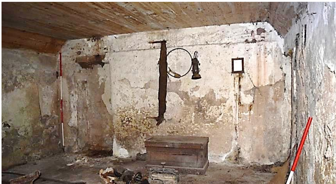
Plate 15: N elevation of Room 4.1, with line for the original roof trusses and recess [017] on the left.
