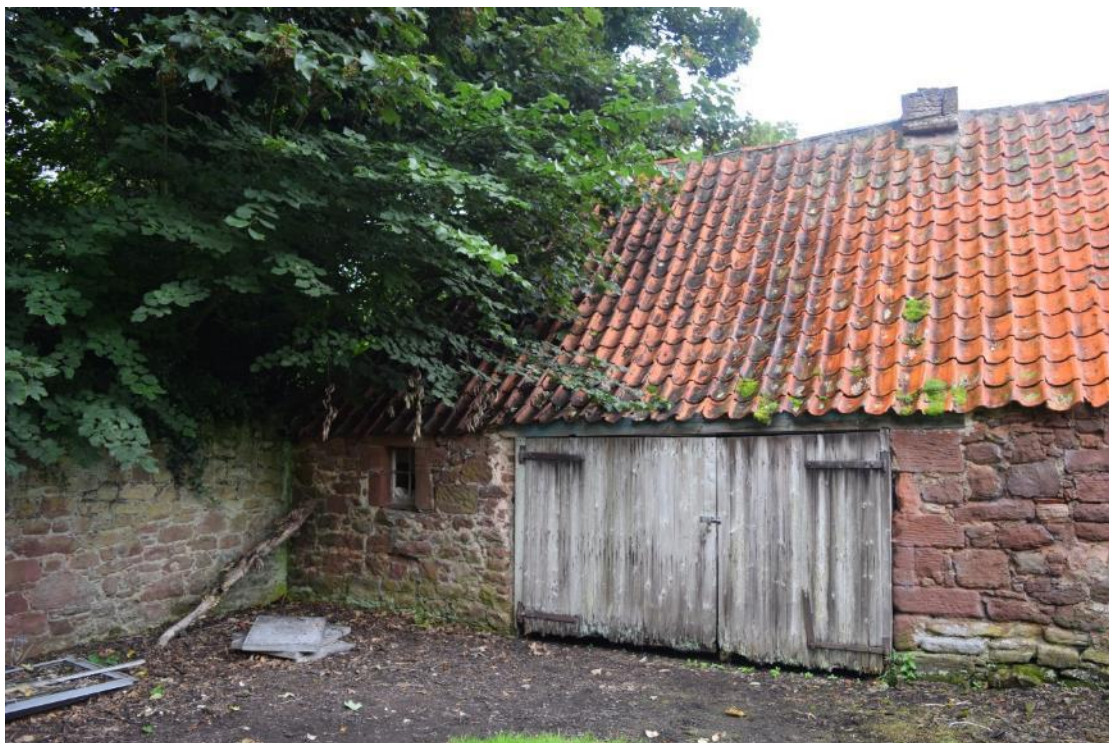
Plate 27: W elevation of Structure 3, with wide double entrance [012] and window [013].
