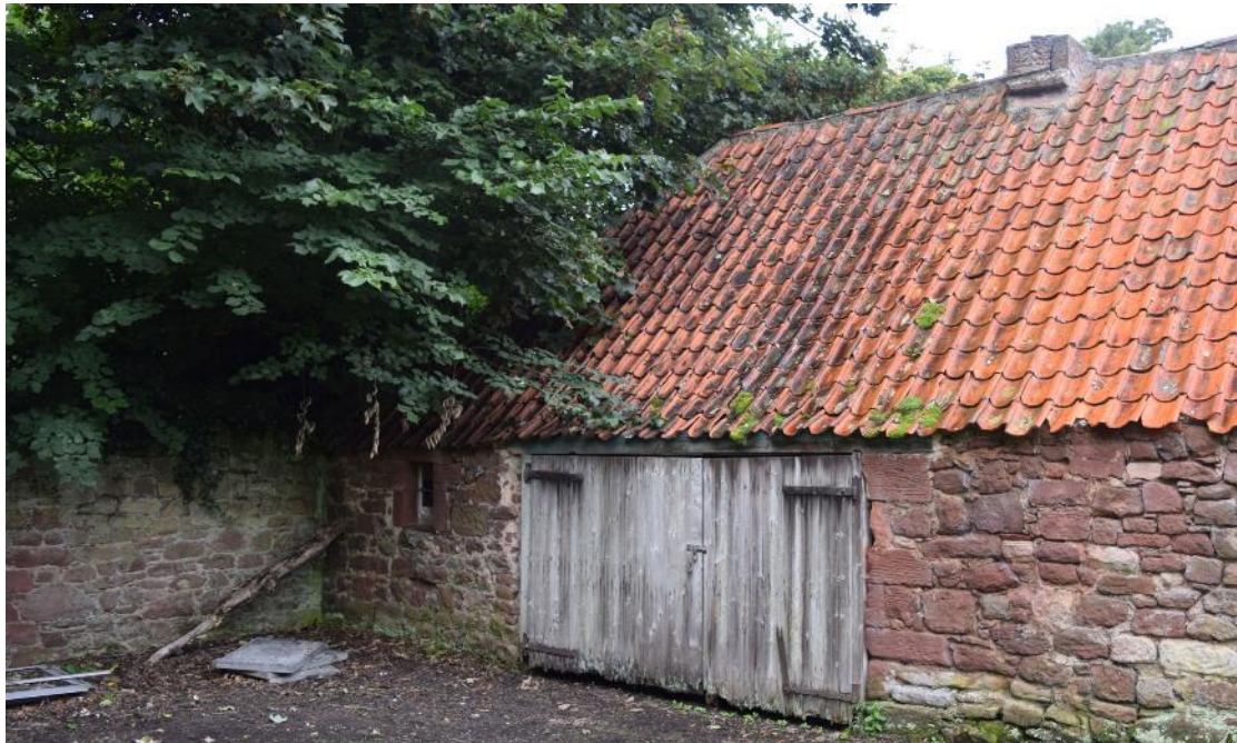
Plate 23: The N end of the E range, showing piended roof of Structure 3 (left) and joint between the N wall of Structure 3 and the boundary wall.
