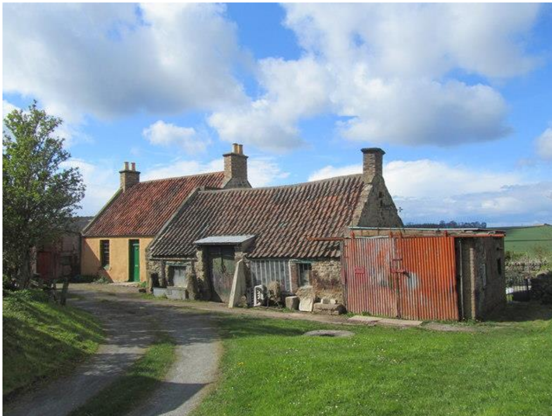
Plate 44: Early 18th century Smithy at Cousland, with later alterations; note the large window next to the central entrance, which served to provide increased light for the smithy workshop (© Copyright C.L.T Smith and licensed for reuse under this Creative Commons Licence )
