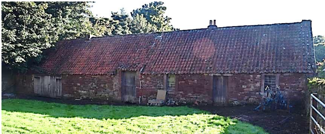
Plate 24: The principal W elevation of the E range, with openings [008-013].
