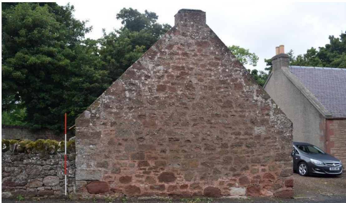
Plate 22: S gable end of Structure 1, surmounted by a low chimney [041].
