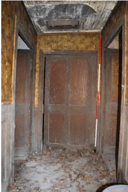
Plate 32: Structure 1, Room 1.1– Left: door [024] into Room 1.2; also note the small roof hatch in the lath ceiling and panelled walls; right: wallpaper and newspapers on the panelling of S elevation.
