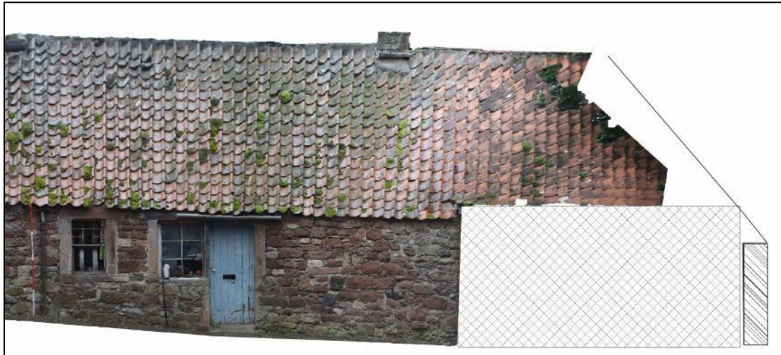
Plate 30: E elevation of Structure 2, with windows [036] and [035]; also note entrance [047] and later timber structure added to the façade (cross-hatched area).
