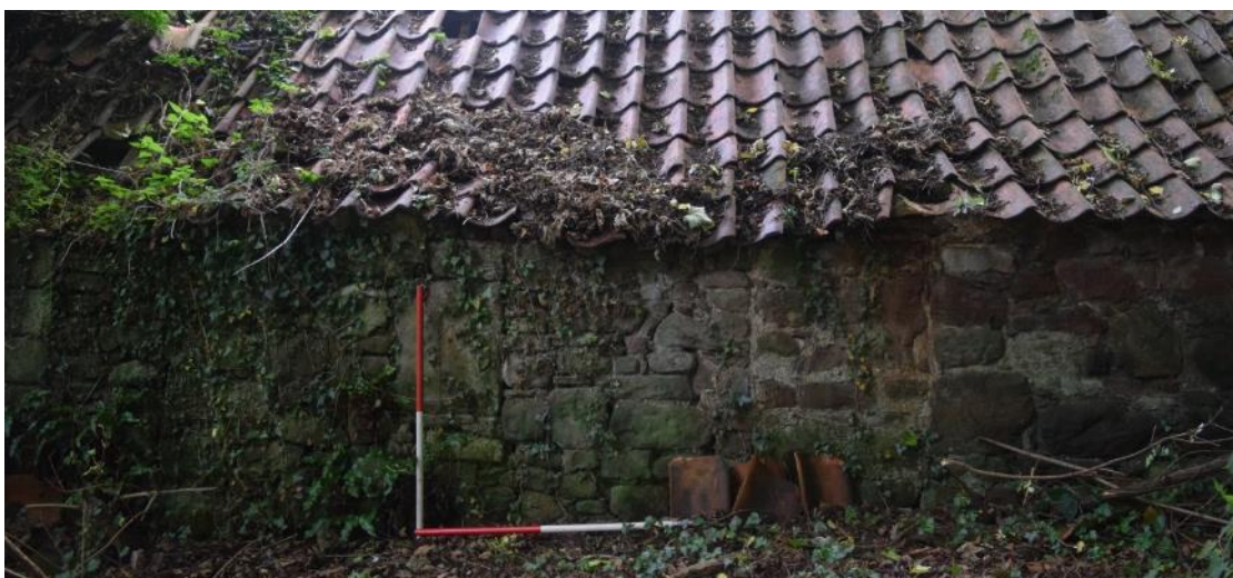
Plate 12: Structure 5, partial W elevation with blocked large opening [020].
