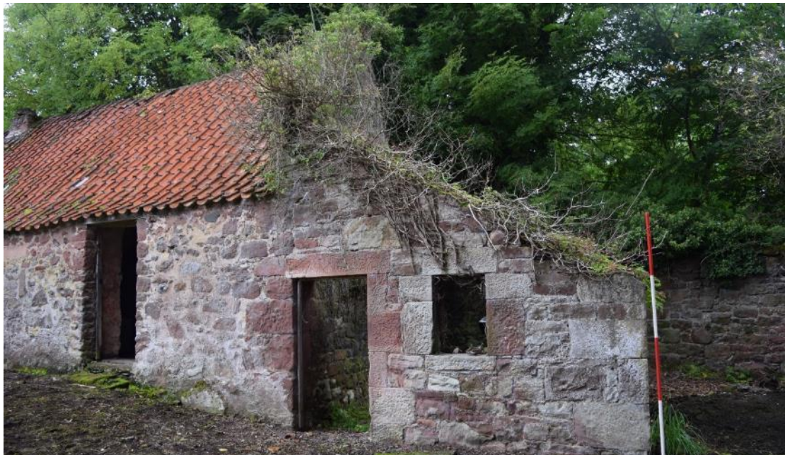
Plate 10: E elevation of Structure 6, with entrance [006] and window [007].
