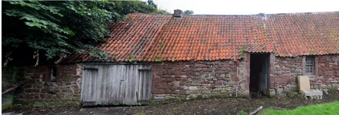
Plate 26: W elevation of Structure 2, with tall entrance [011]; Structure 3 to left.
