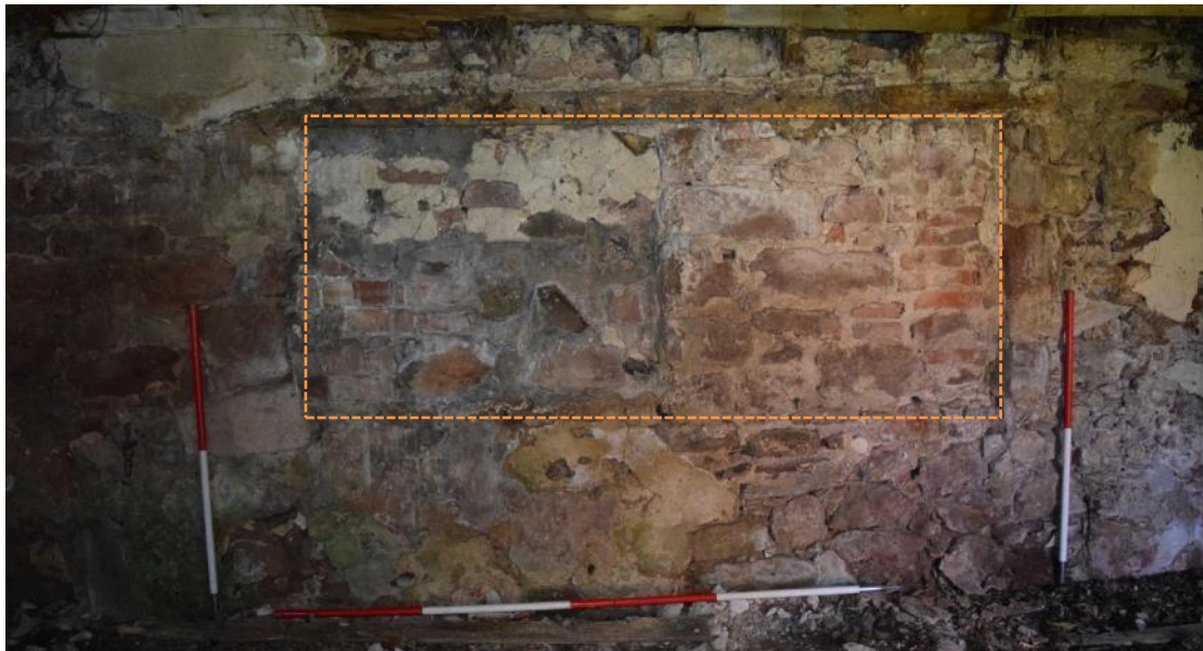
Plate 17: Partial W elevation of Room 5.1, showing large blocked opening [020].
