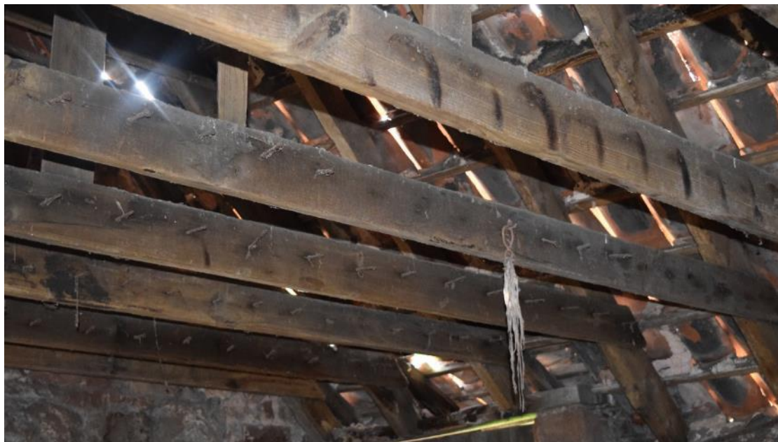
Plate 39: A-frame roof with kingposts; Room 2.1, with nails and horseshoe scorch marks on the lower cross beams.
