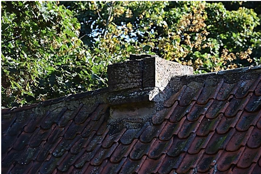
Plate 31: Detail of the chimney stack [043], with projecting chamfered drip stone.
