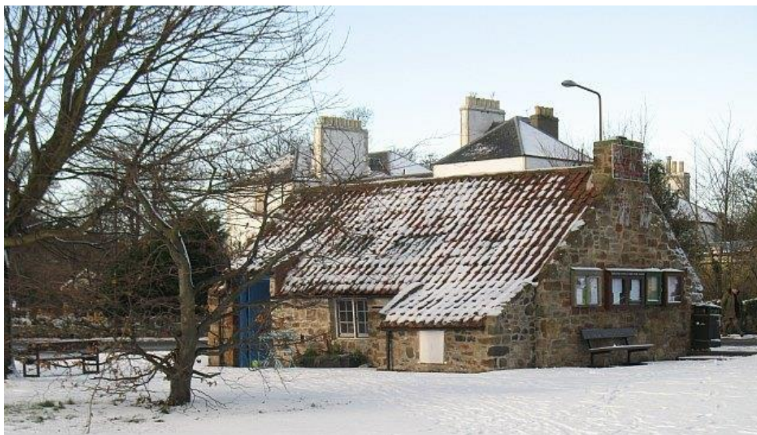
Plate 4: Gullane Old Smiddy; note the low extension at the front for the bellows © Copyright Richard Webb and licensed for reuse under this Creative Commons Licence .
