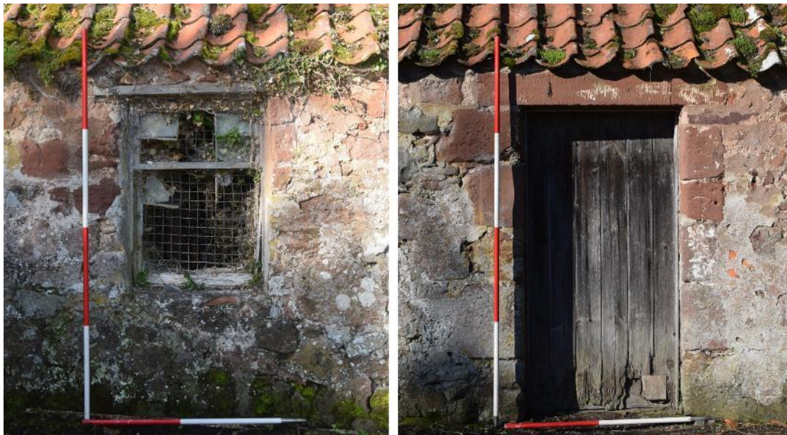
Plate 8: Structure 4, E elevation (partial) with window [001] and entrance [002].
