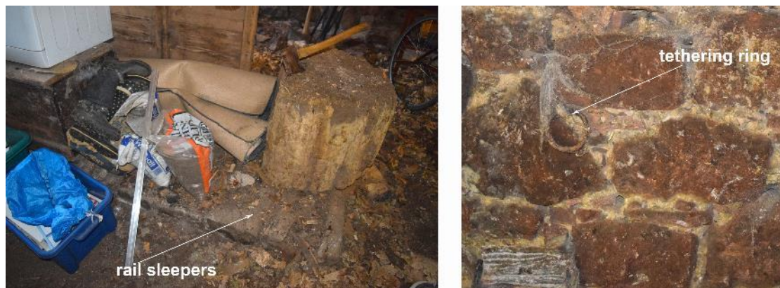
Plate 38: Room 2.1, detail of sleeper beam flooring (left) and iron 'tethering' ring on the S elevation (right).
