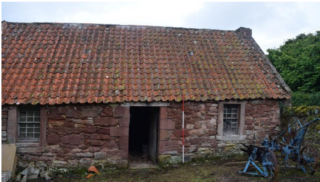
Plate 25: W elevation of Structure 1, with windows [008] and [010] and entrance [009].
