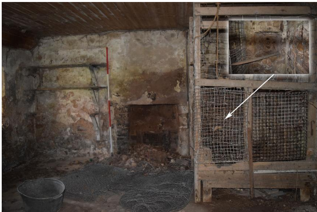
Plate 14: S elevation of Room 4.1, with shelving unit to left and fireplace [014] to right; also note the 'cage' construction and blocked opening [015] in the corner (detail).
