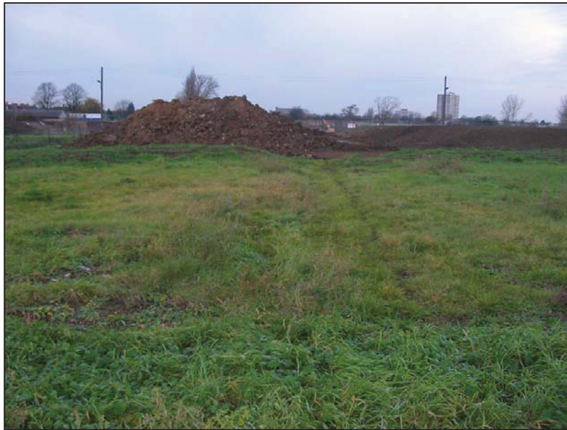
Plate 1: Looking northwest over survey area showing the large spoil heap situated over the western edge of the survey area
