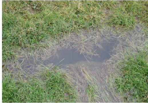
Plate 2. Water spring presumably being supplied from the leaking dam.
