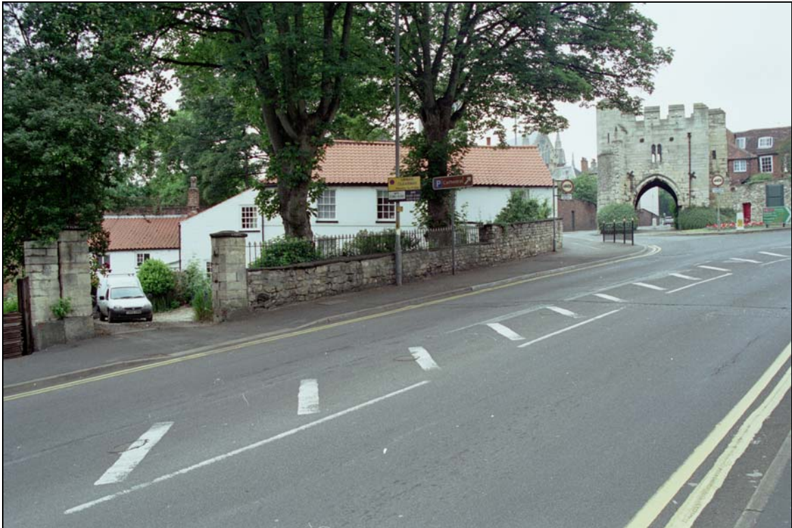
Plate 1: General view of Pottergate Lodge (with Pottergate Arch to right) - looking generally north-west
