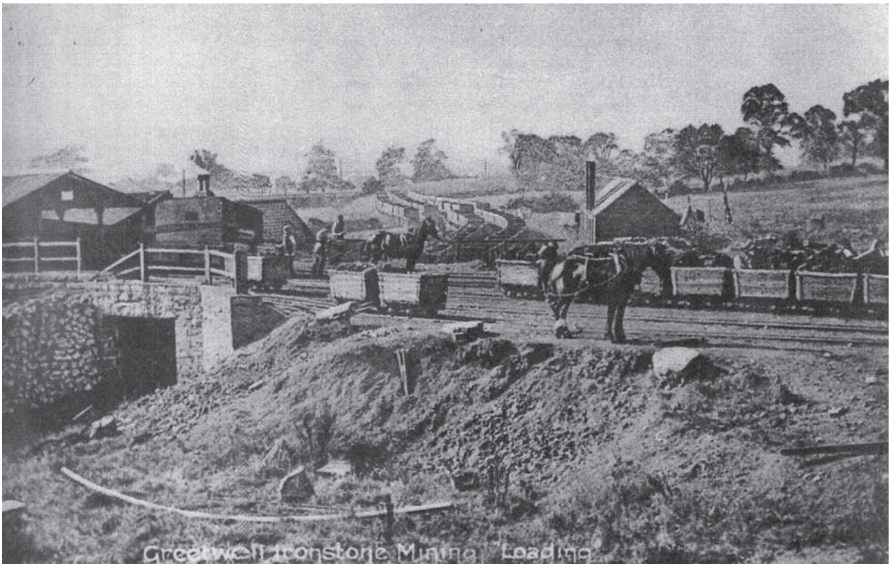
Figure 5. Old photo c. 1920s showing horse-drawn tramways transporting ironstone from the Greetwell Ironstone Mines at the Monks Abbey Sidings, Allenby Estate. (Maurice Hodson - Lincoln City Museum archives).
