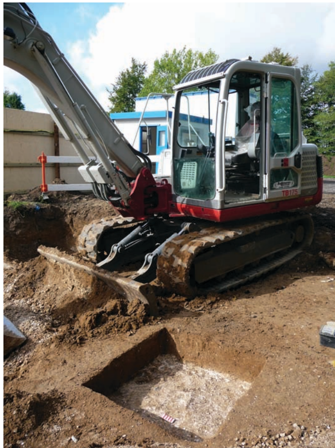
Figure 4. Photographs of F.2 (top) and Test Pit 1 (bottom) - both looking North
