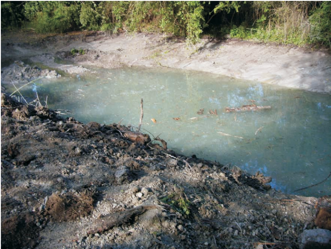
Figure 5. Eastern arm of the moat during cleaning and silt pond post-cleaning
