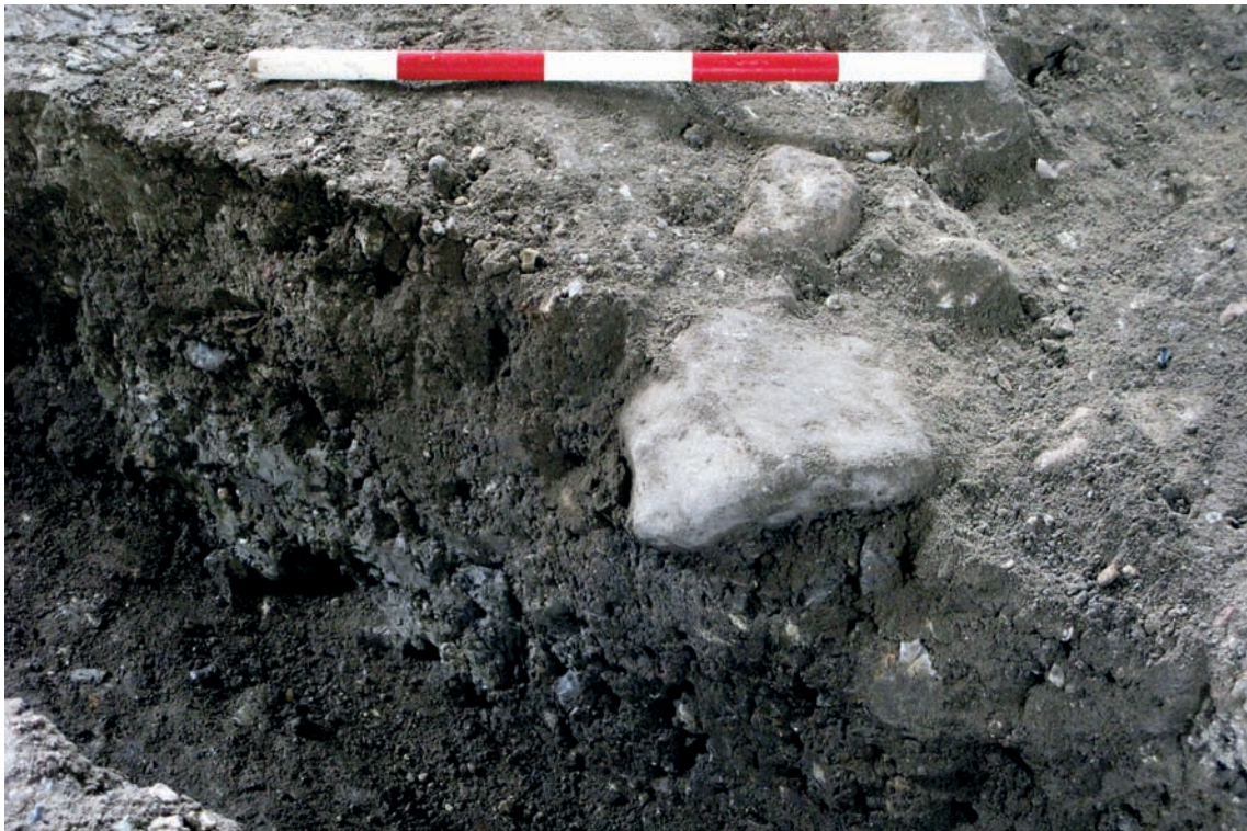
Figure 11. Views of stone-built foundation F.101 (top left), mortared tile foundation F.100 (top right), and clay sill pad F.102 (bottom)
