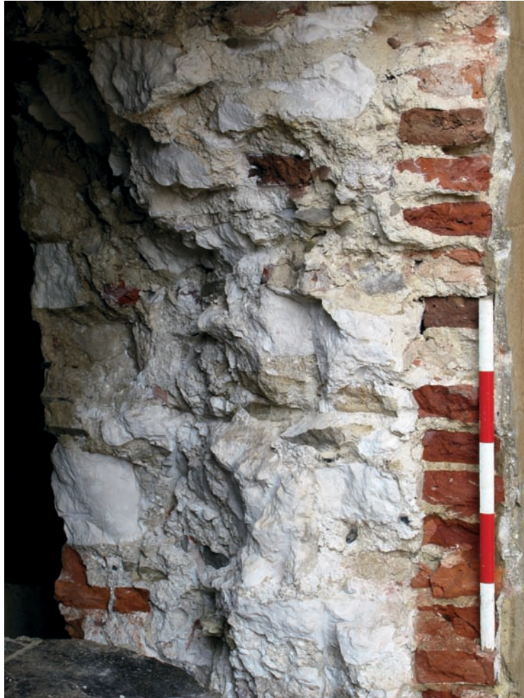
Figure 5. Cross-section of the south wall of the Porter's Lodge
