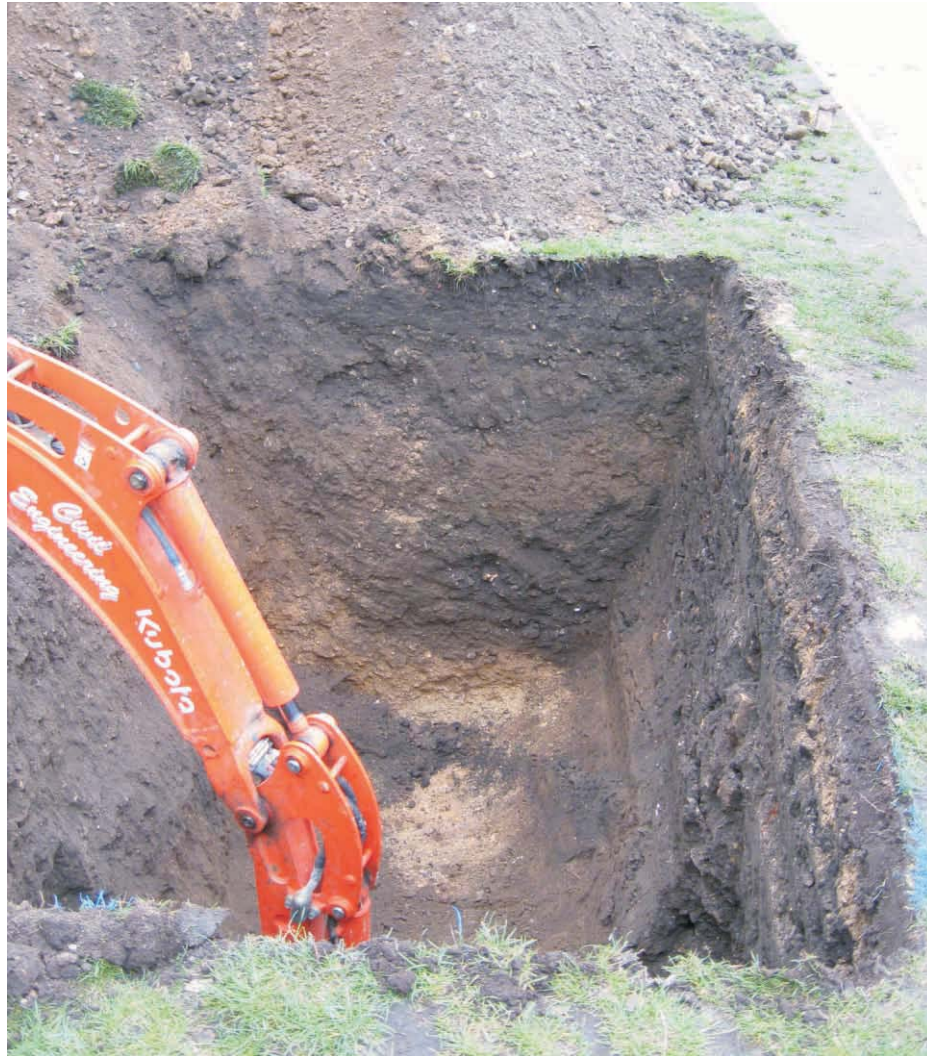
A. Southwest facing section of soakaway
