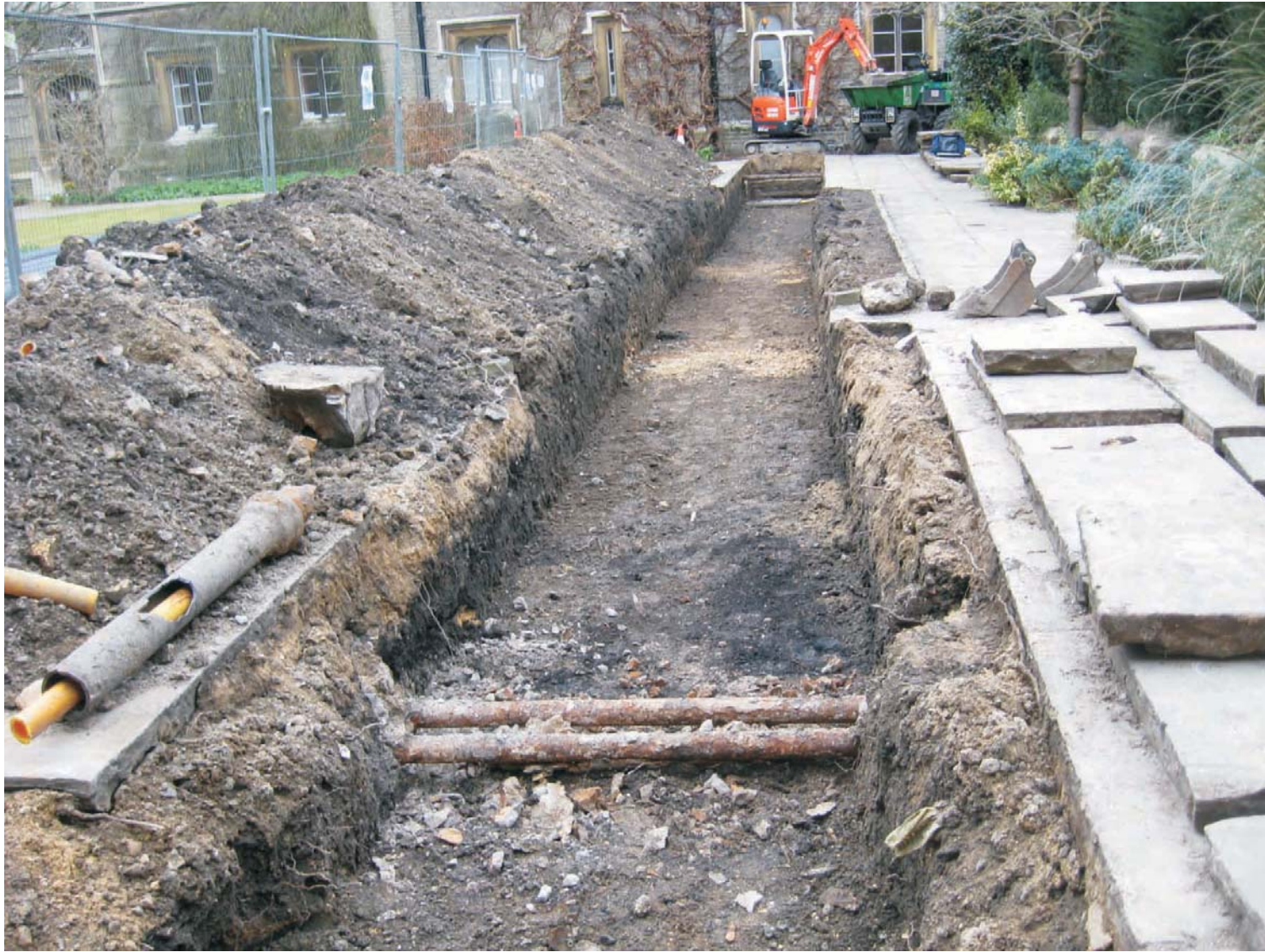
Figure 3. Area 1, pipe trench, looking south-east, taken during early stages of excavation
