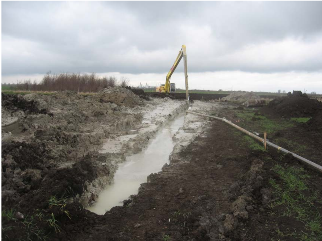
Figure 2: Photograph of Cut-Off Wall and Up-Cast Deposits Covered in Bentonite Slurry.
